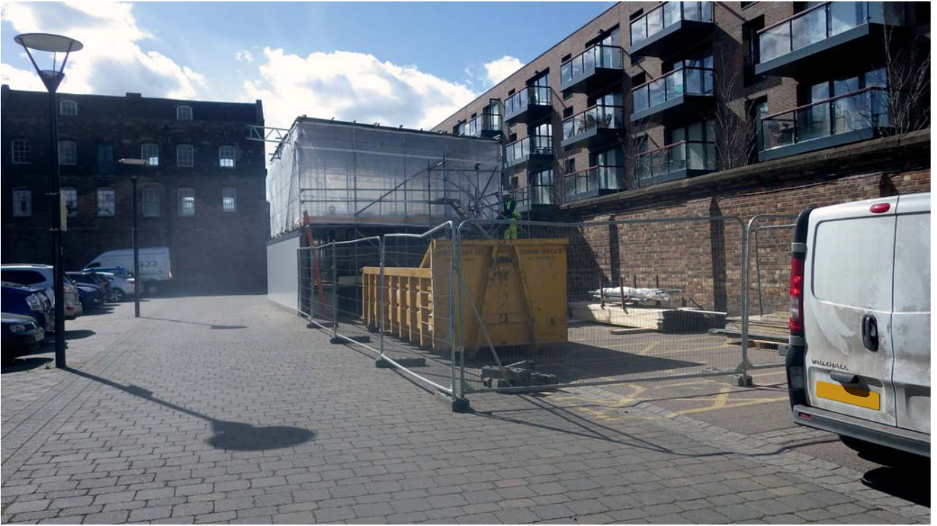
Figure 2: The soil block in its final location
