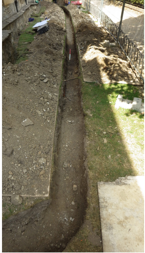
Plate 2: Trench 3 excavated, view to north
