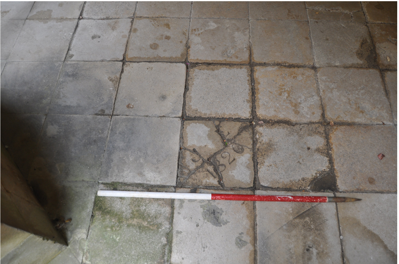
Plate 7: Initialled stone floor tile by Test Pit 3, view to west
