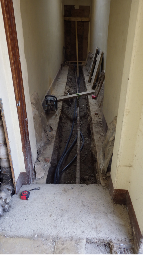
Plate 1: Trench 2 excavated, view to south
