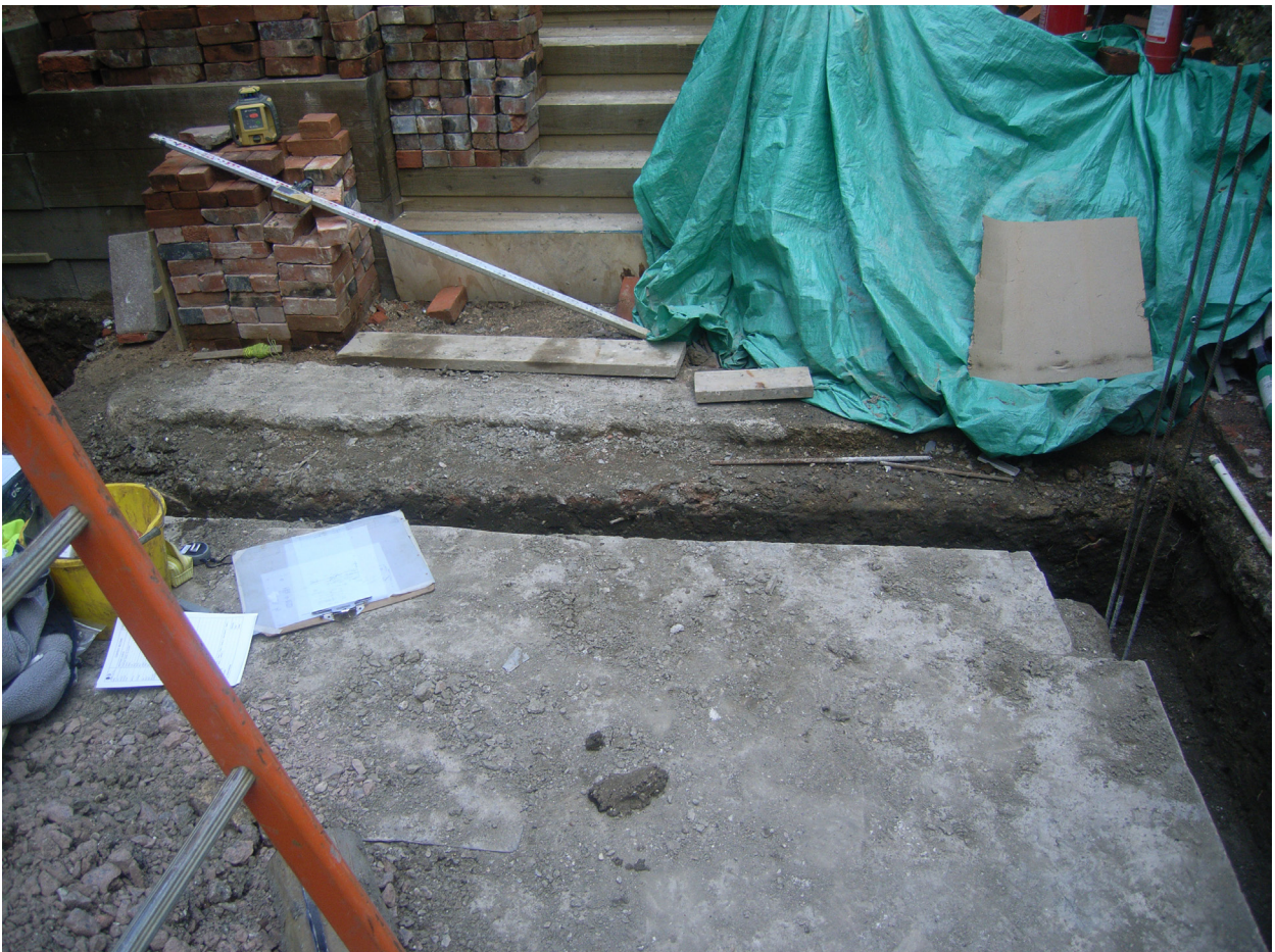
Plate 6: General view of ground beam trench
