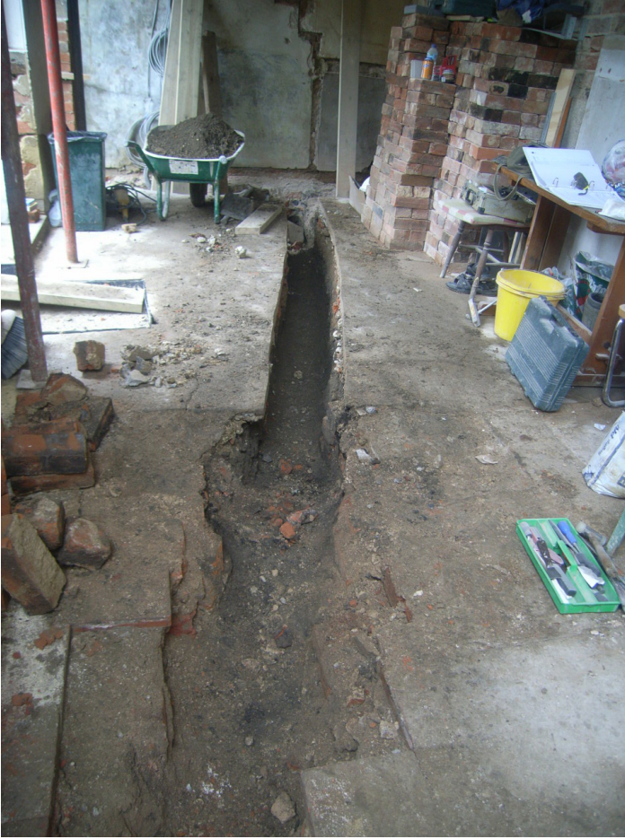
Plate 5: General view of ground beam trench
