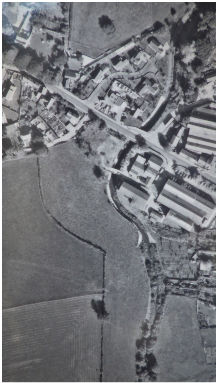
Plate 7: After construction works of the River Boyd 1980
