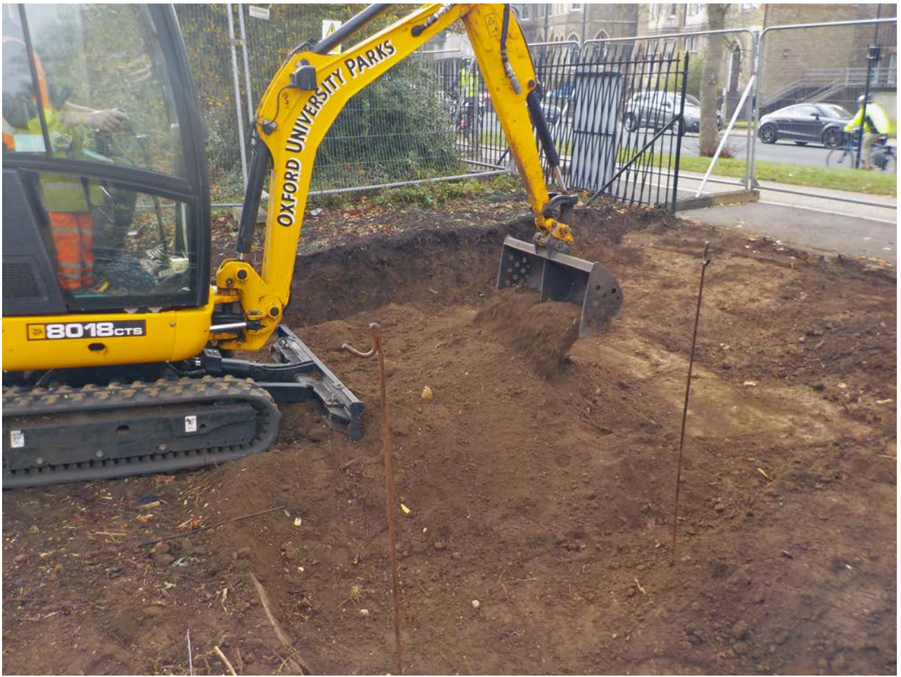
Plate 1: Ground reduction in progress, looking south-west
