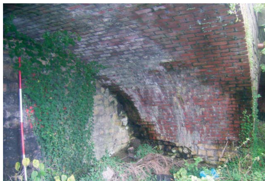
Plate 20: Interior of Vault 13
