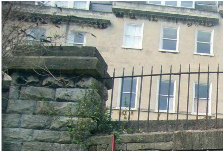
Plate 21: Wall to south of Vault 13 and later pier
