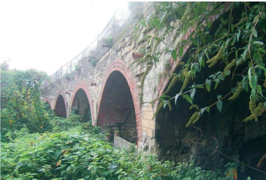
Plate 7: Arch face of Vaults 3, 4, 5 and 6
