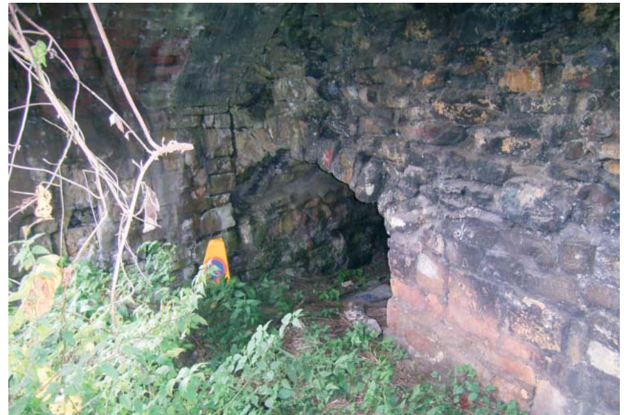
Plate 6: Passage in Vault 3
