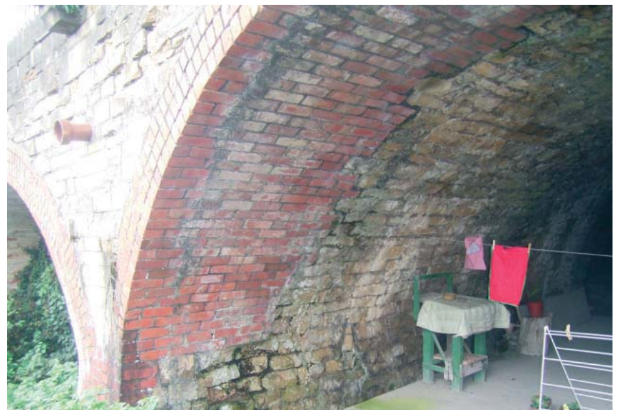
Plate 8: Interior of Vault 4
