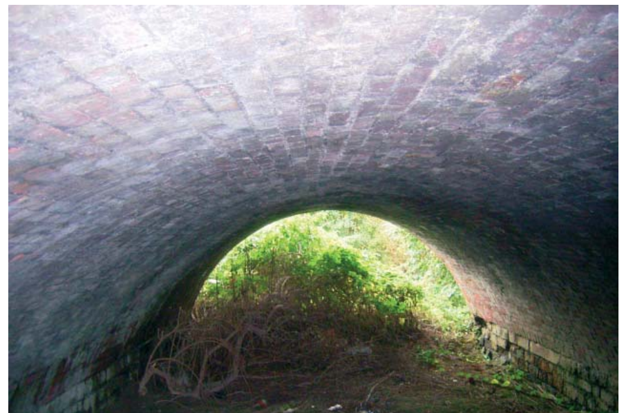
Plate 12: Interior of Vault 7
