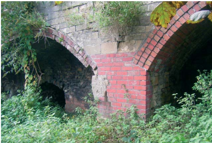
Plate 3: Pier between Vaults 2 (to right) and 3
