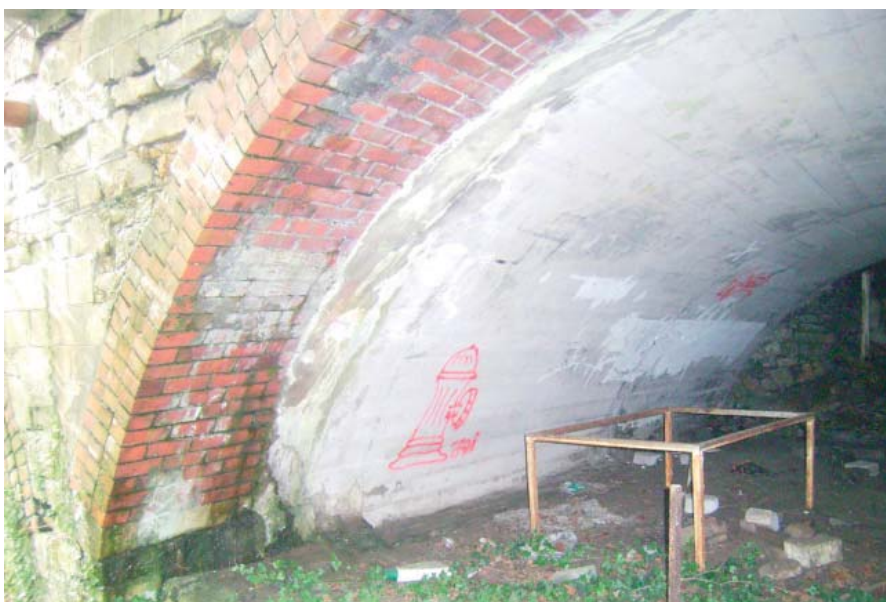
Plate 19: Vault 12 showing concrete arch and brick face
