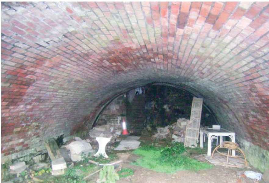
Plate 11: Interior of Vault 6
