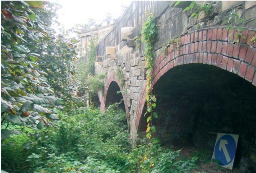
Plate 1: Face of Vault 1 in foreground
