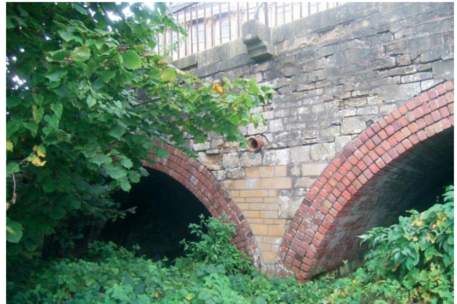
Plate 14: Face of pier between Vaults 7 (to right) and 8
