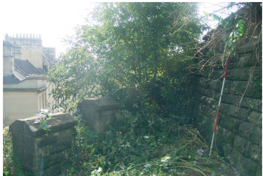
Plate 24: Junction between viaduct and Hedgemoad retaining wall
