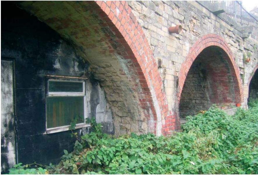
Plate 9: Face of Vaults 5 (to left) and 4
