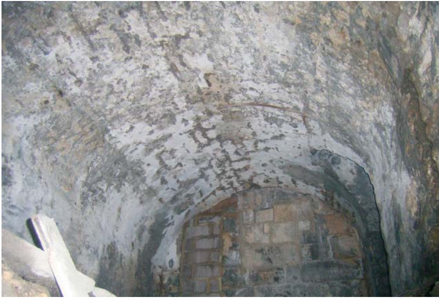
Plate 13: Basement room of house beyond Vault 7
