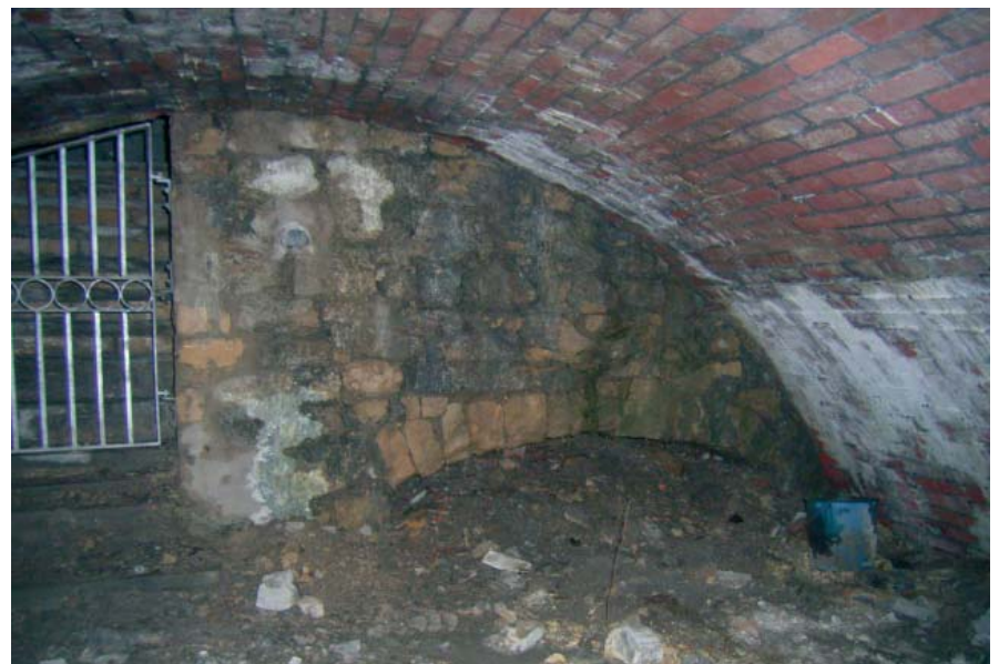
Plate 16: Rear wall of Vault 9 showing relieving arch
