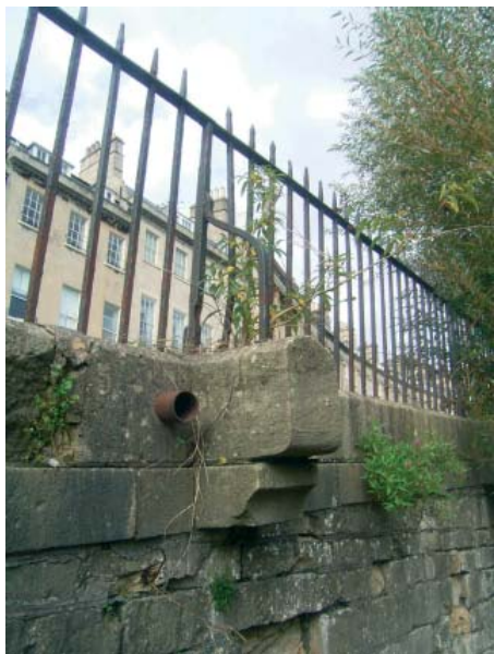
Plate 23: Corbel supporting iron railing
