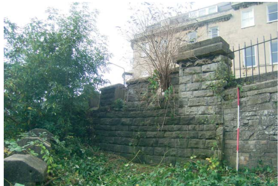
Plate 22: Later pier and wall at south end of viaduct
