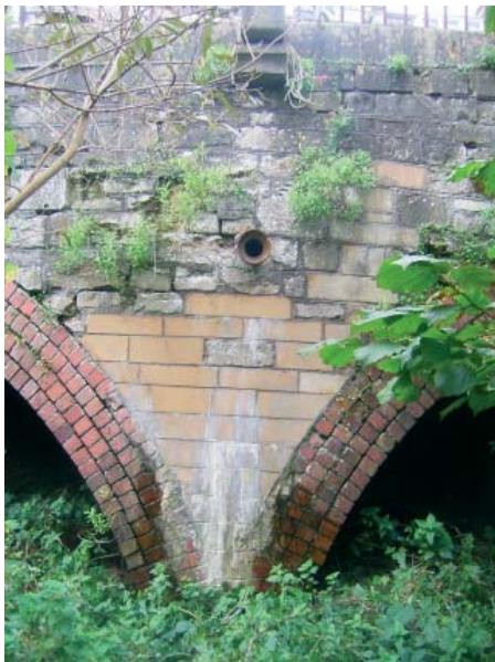
Plate 15: Vault 9 (to right) and 10
