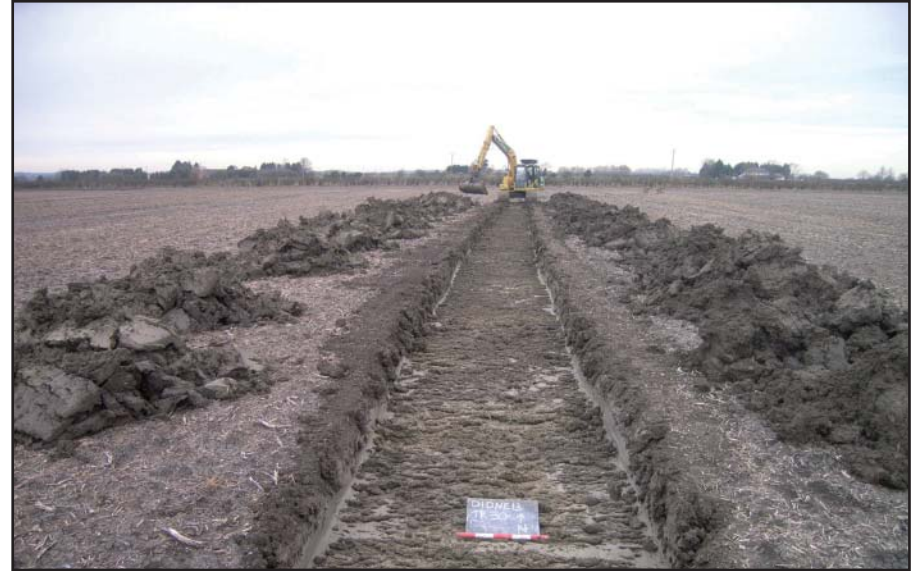
Plate 10: Trench 30 looking north
