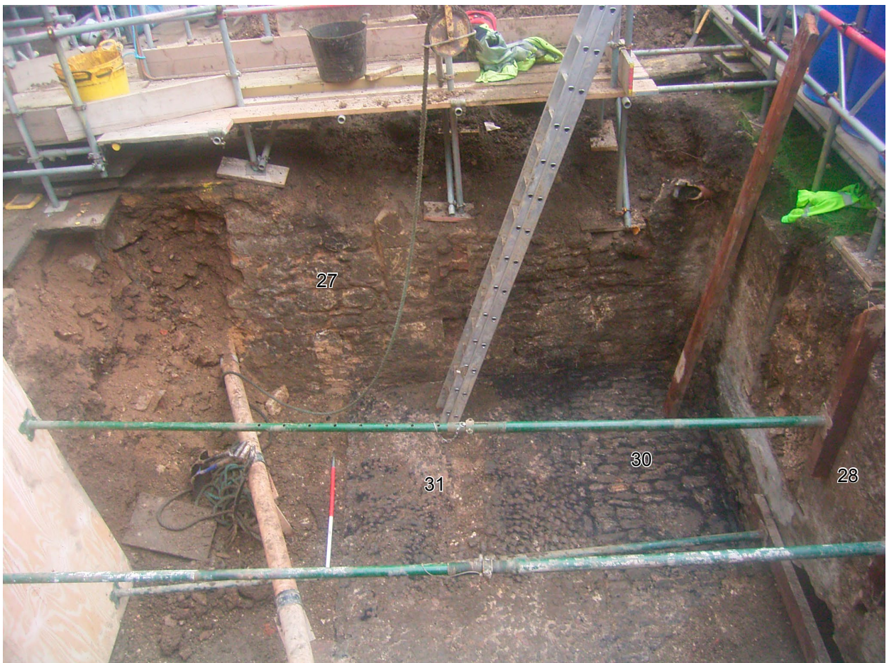
Plate 2: East wall of crane base cellar
