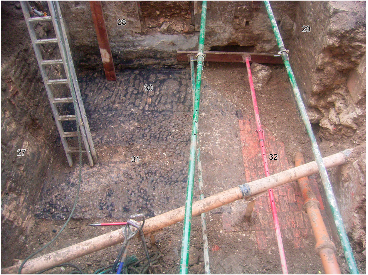
Plate 3: Crane base cellar floor
