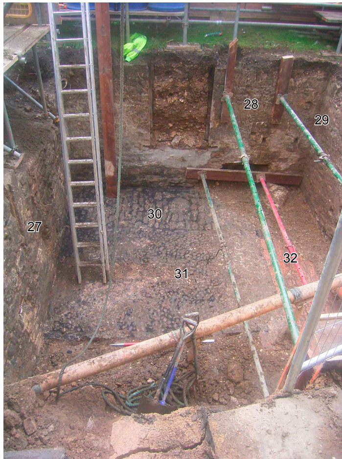
Plate 1: Lightwell in south wall of crane base cellar
