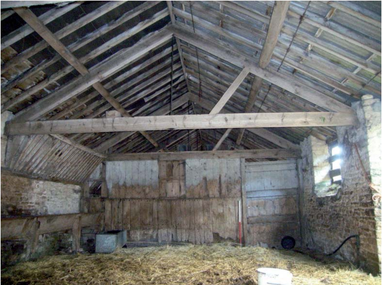
Plate 47: Barn 5; Partition dividing the Easternmost and Central Stable/Loosebox
