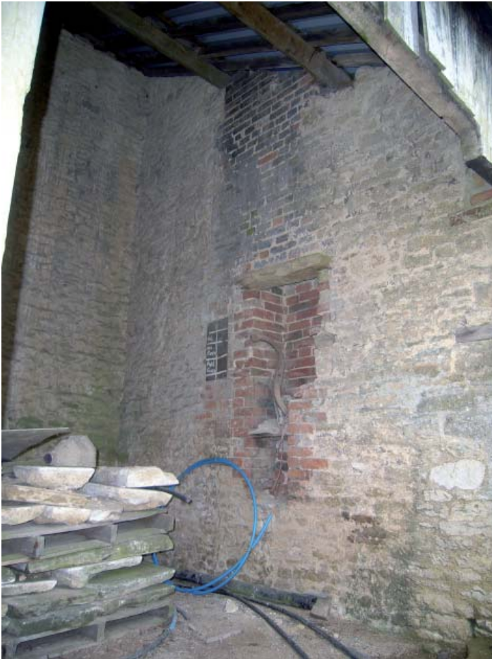
Plate 21: Barn 2; Farrier's Workshop
