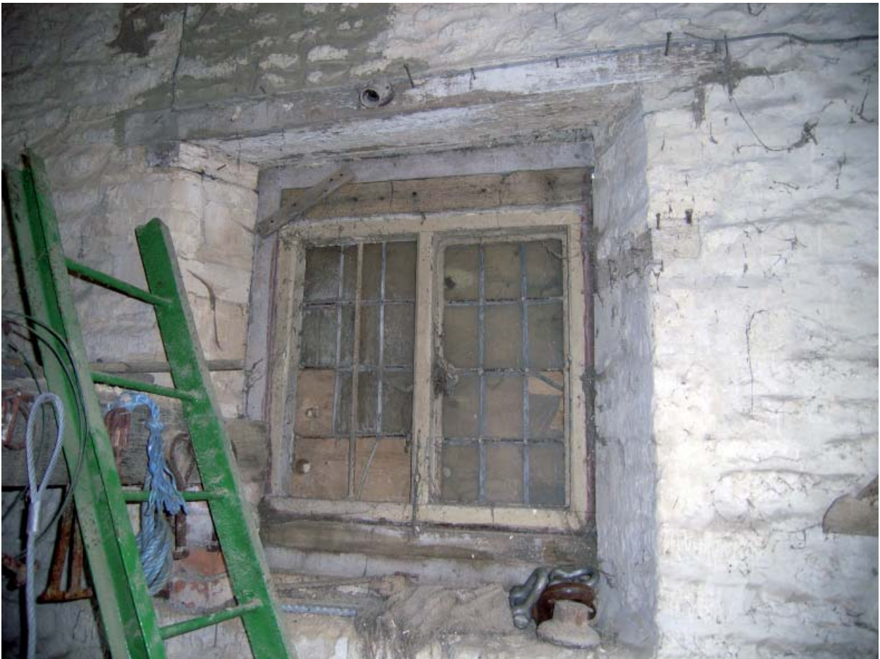
Plate 20: Barn 2; Warming Room window
