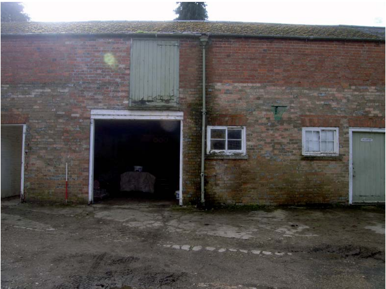
Plate 2: Farmhouse building; detail of first floor addition and pitching door; north elevation
