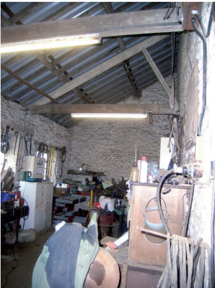
Plate 18: Barn 2; Roof truss in the General Workshop
