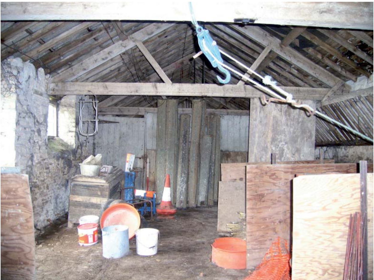
Plate 48: Barn 5; Central Stable/Loosebox showing makeshift stalls
