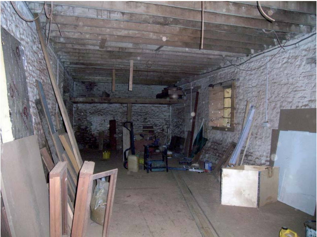
Plate 24: Barn 2; Modern Carpenter's Shop, ground floor looking east
