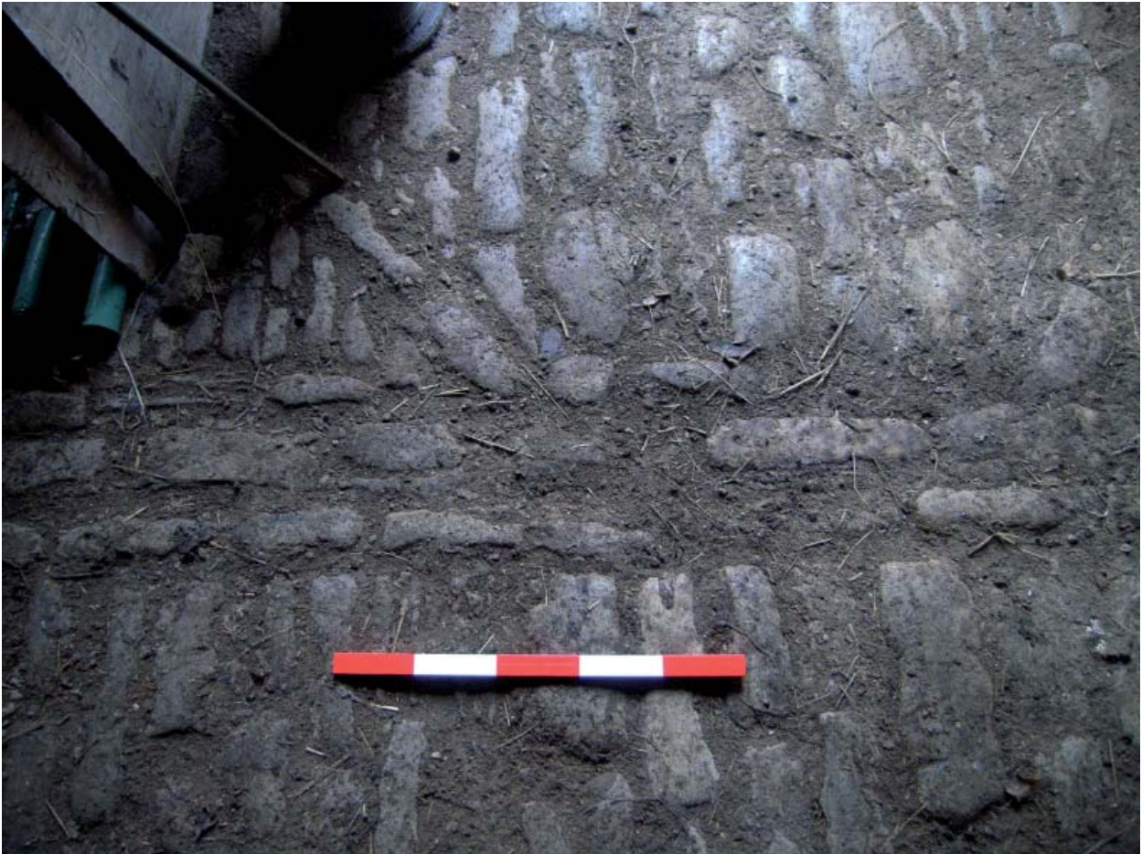
Plate 49: Barn 5; Central Stable/Loosebox floor detail
