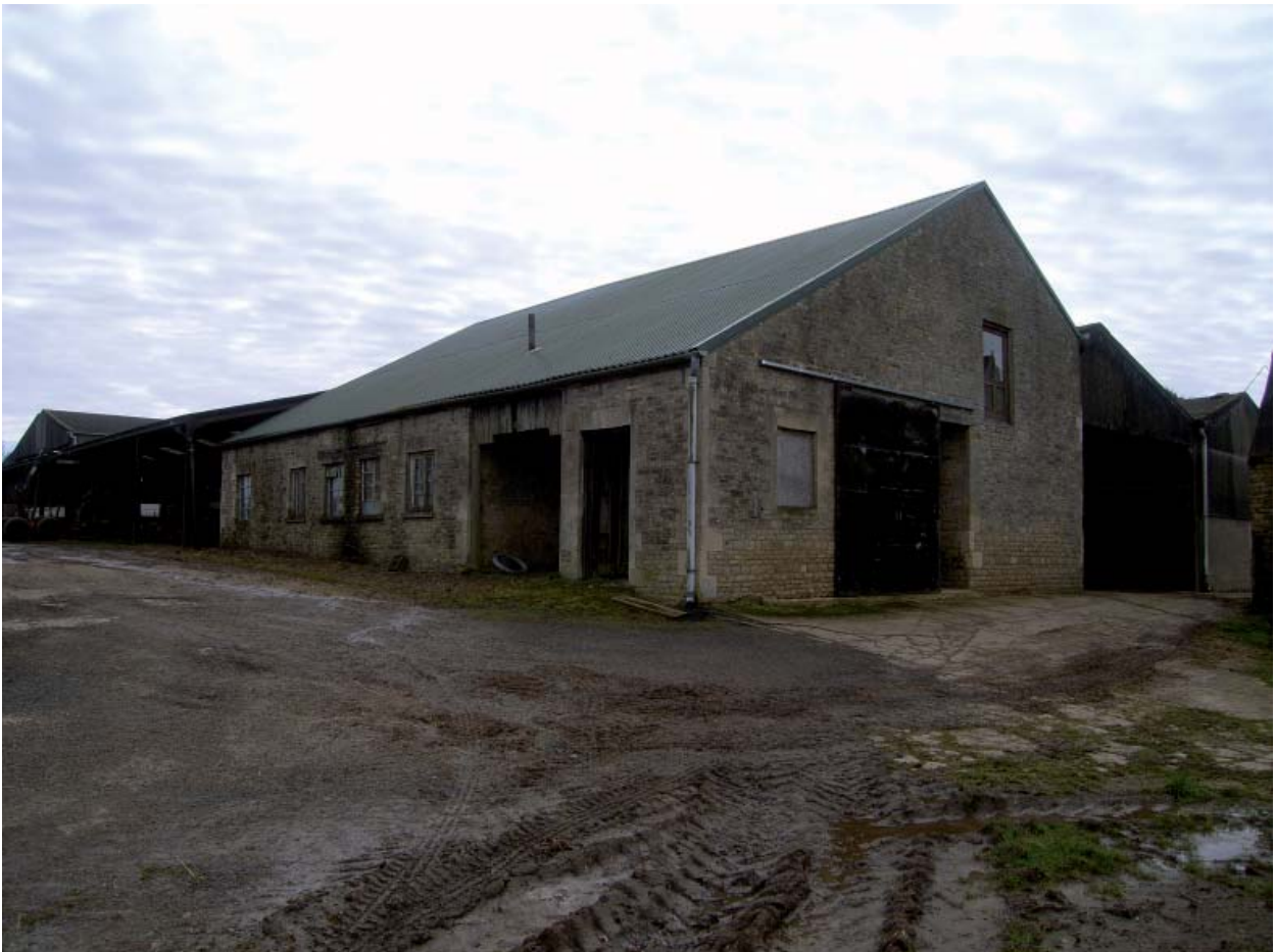
Plate 10: Barn 2; north and west elevations
