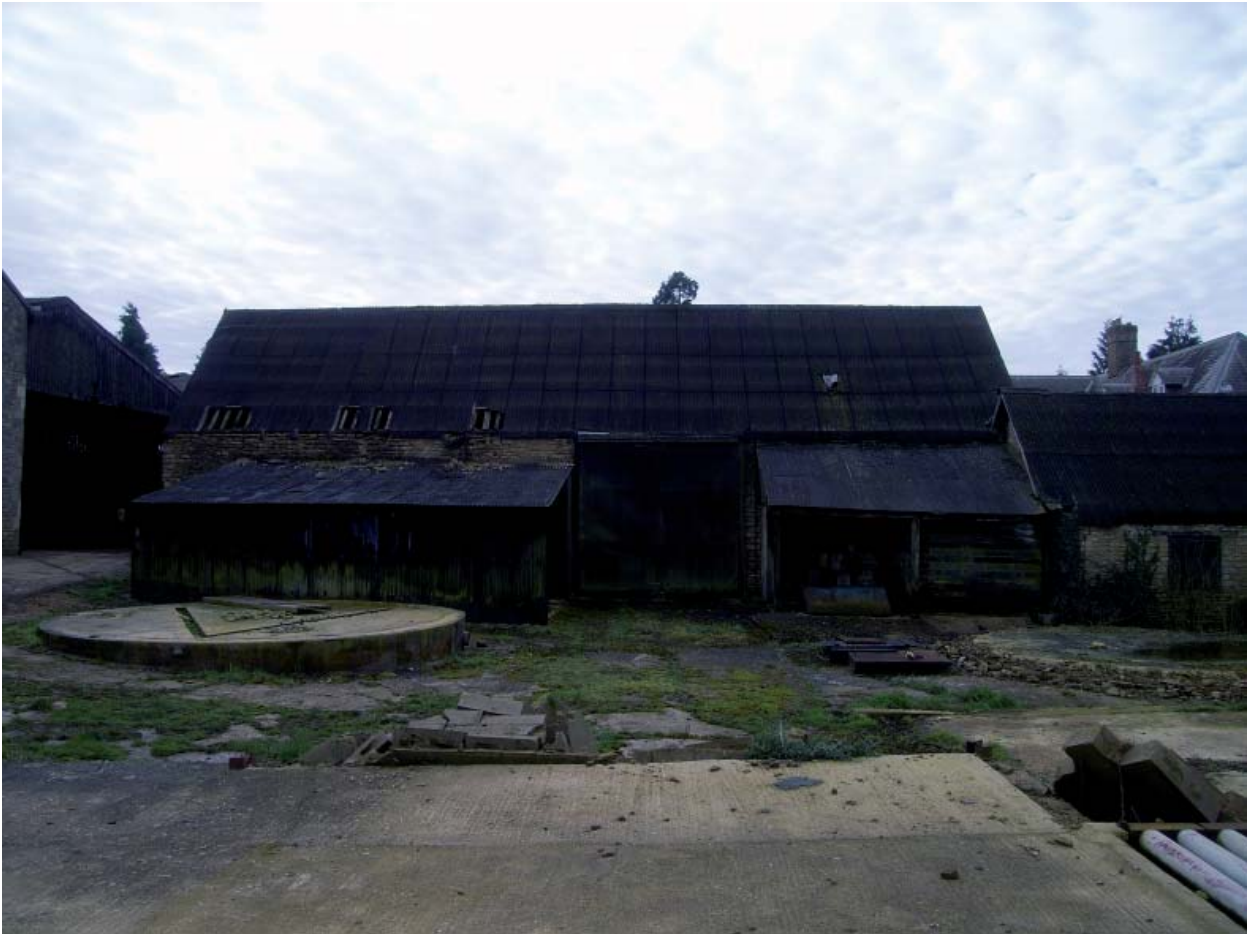
Plate 31: Barn 3; north elevation
