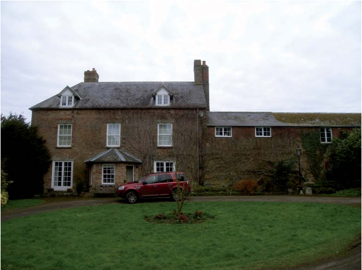
Plate 1: Main farmhouse building; south elevation
