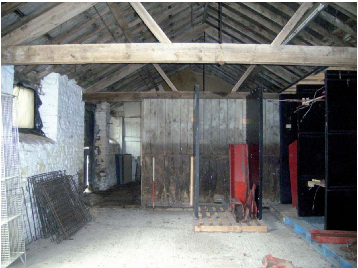
Plate 50: Barn 4 & 5; Partition of Store at west end of Barn 5 and Large Store of Barn 4
