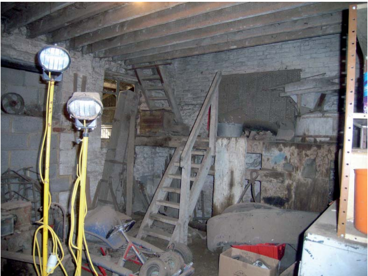
Plate 28: Barn 2; Mill House steps and landing looking west
