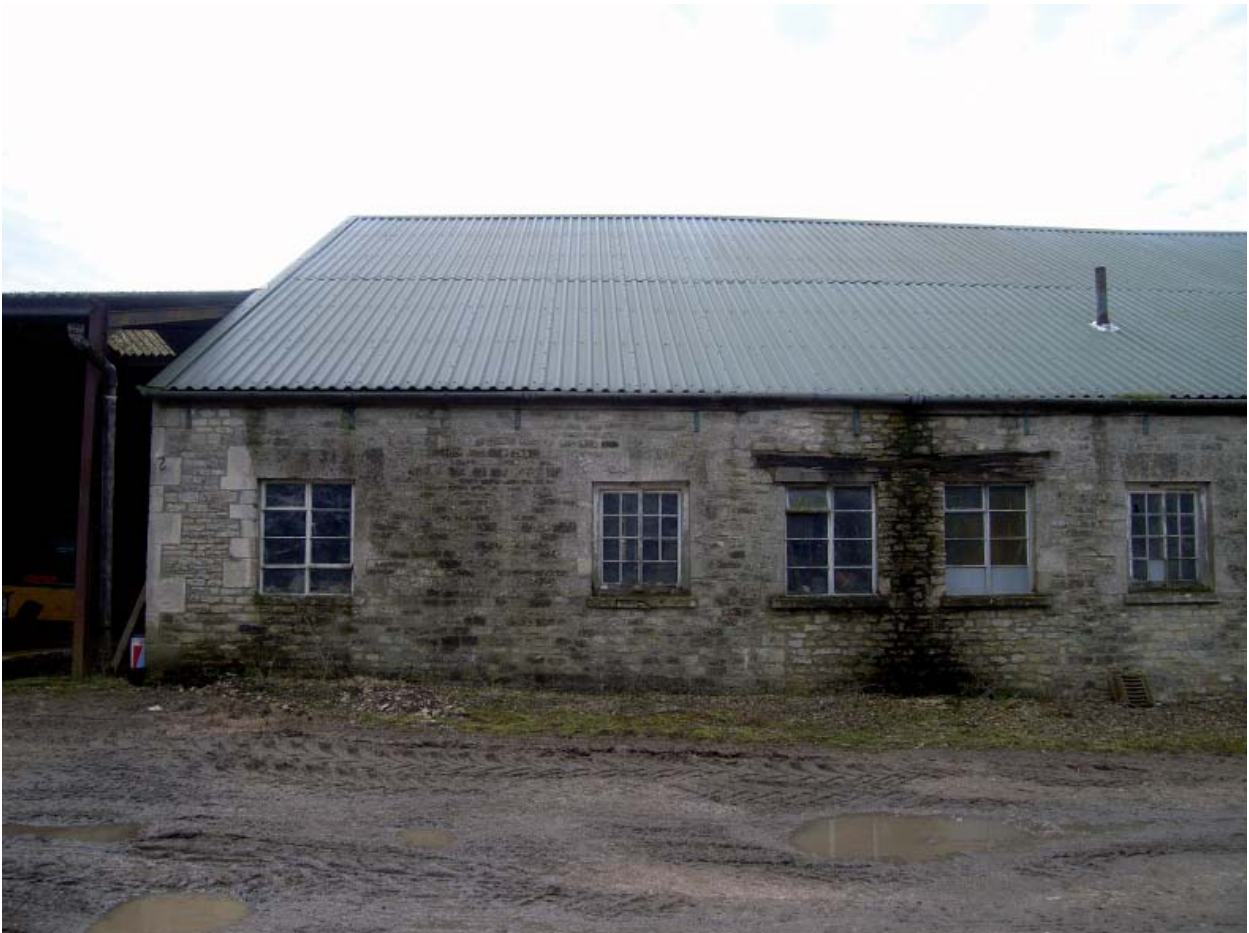
Plate 14: Barn 2; east end of north elevation
