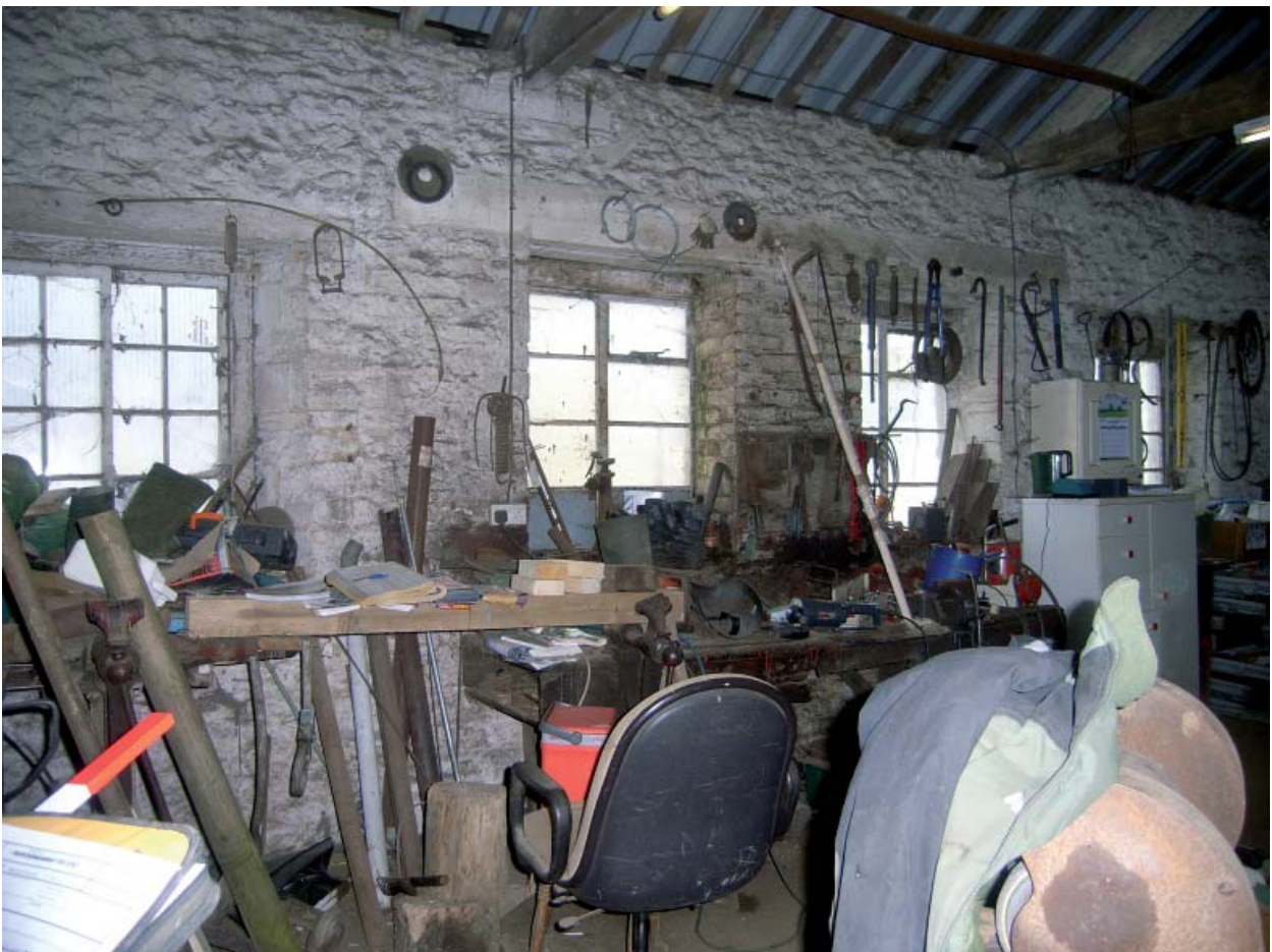
Plate 22: Barn 2; General Workshop showing blocking of large opening
