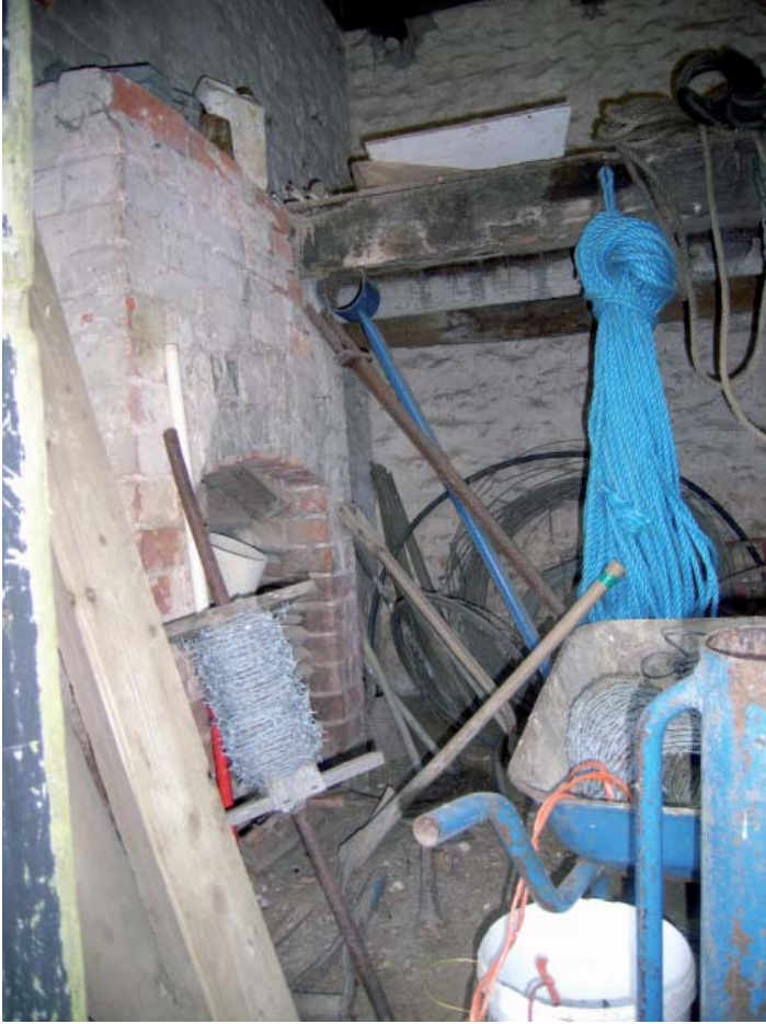
Plate 19: Barn 2; fireplace in the Warming Room
