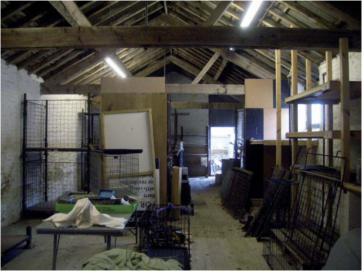
Plate 51: Barn 4; General Shot looking west
