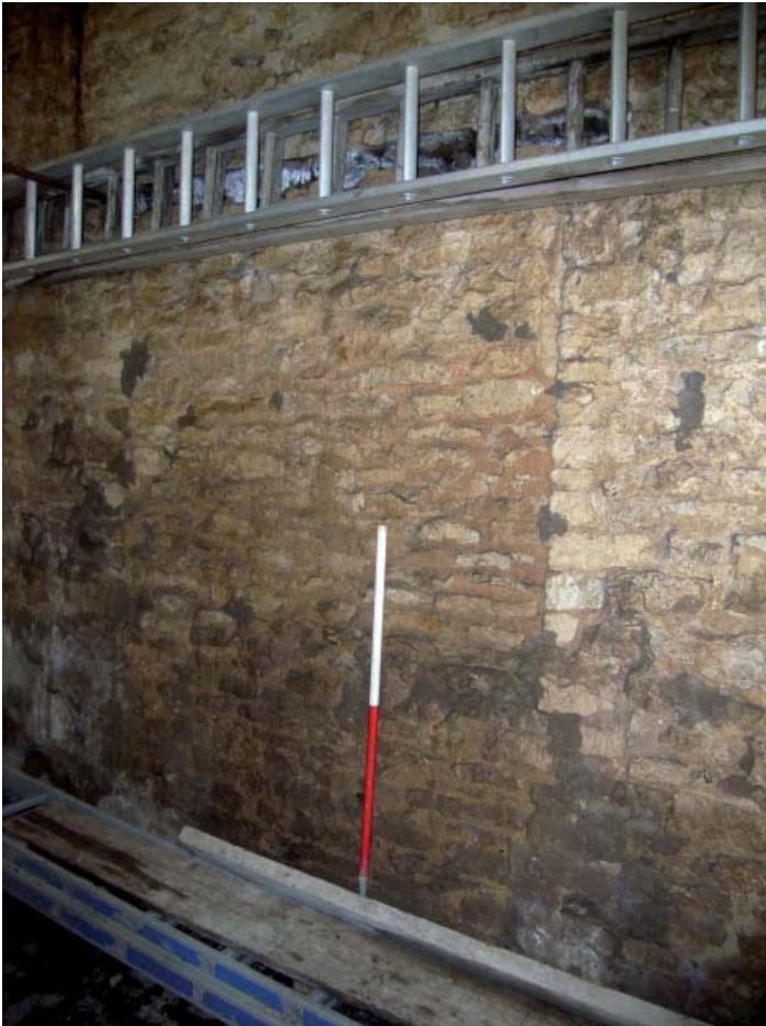
Plate 33: Barn 3; blocked doorway in the south wall
