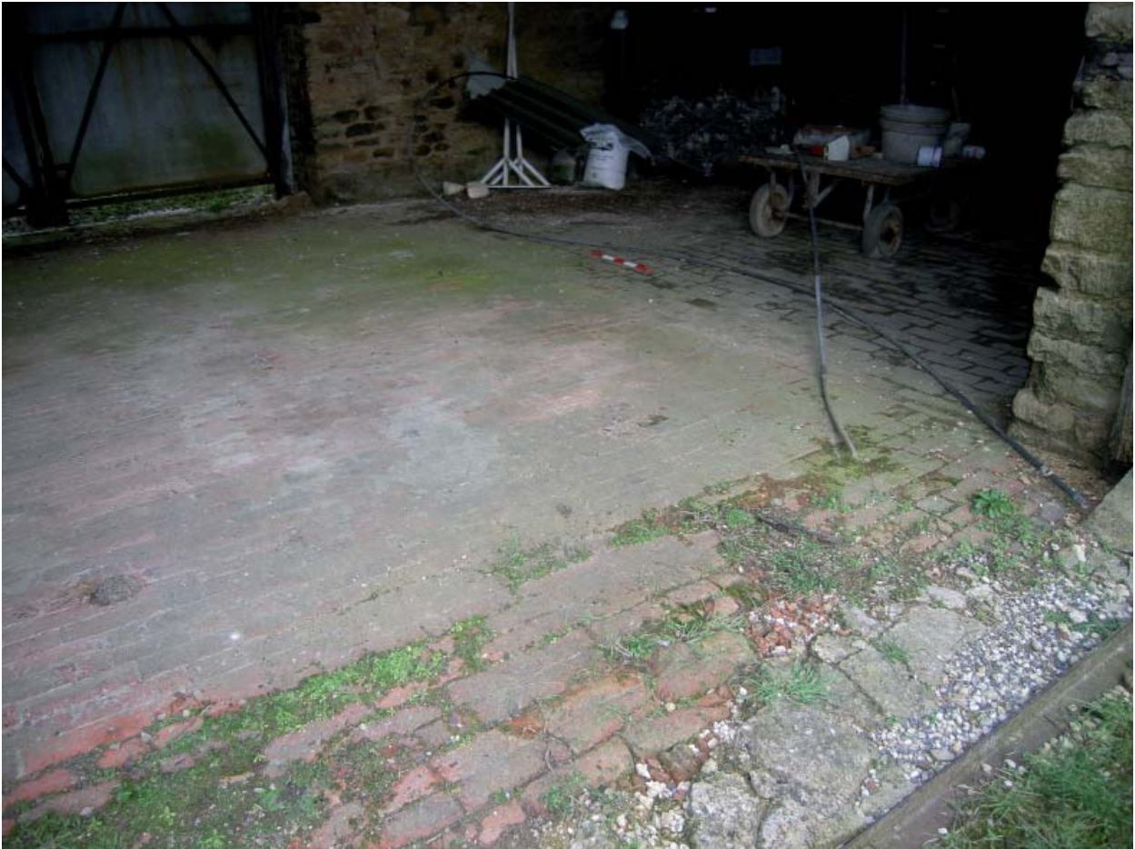
Plate 39: Barn 3; threshing floor and storage bay floor looking north east
