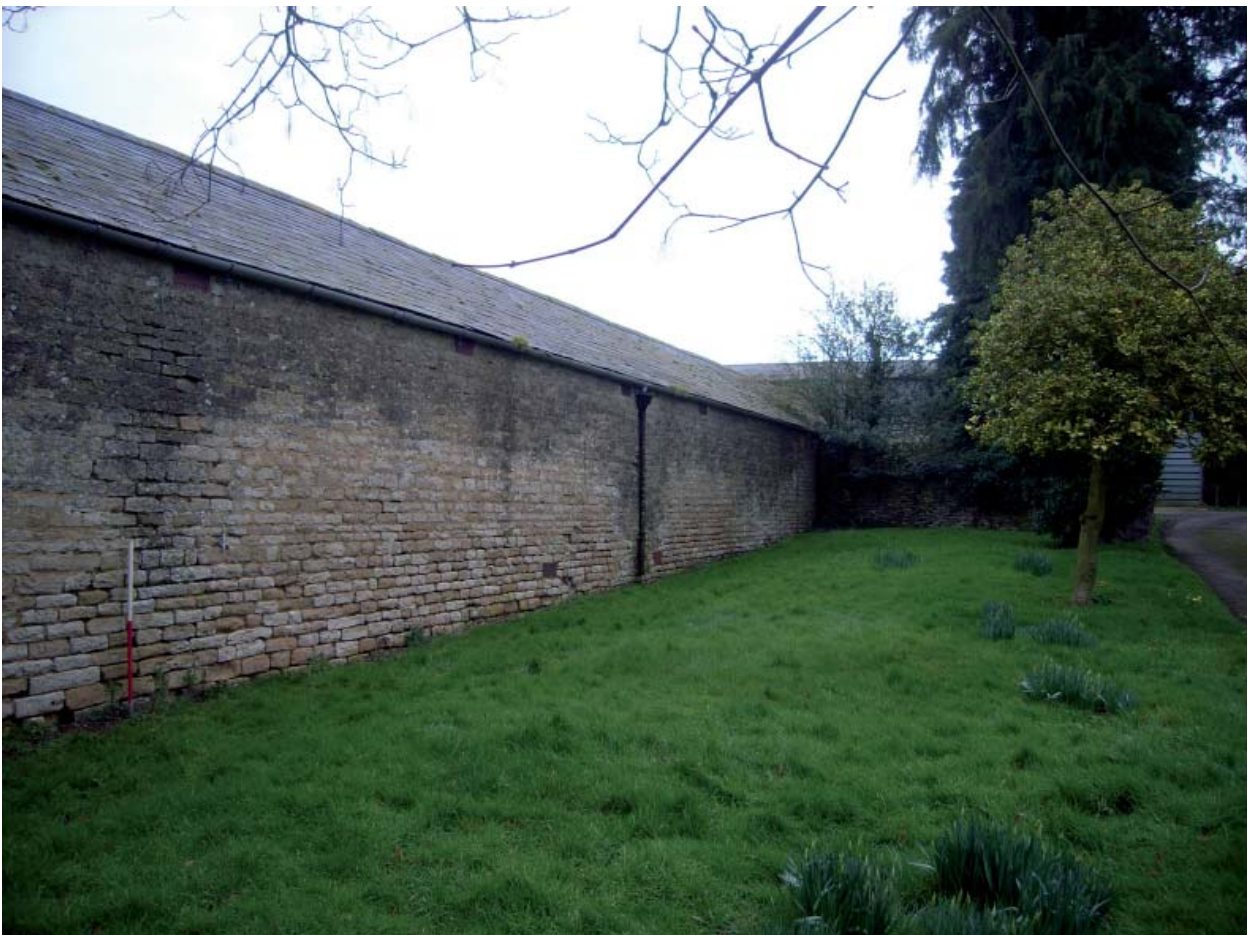
Plate 40: Barn 5; south elevation looking north east
