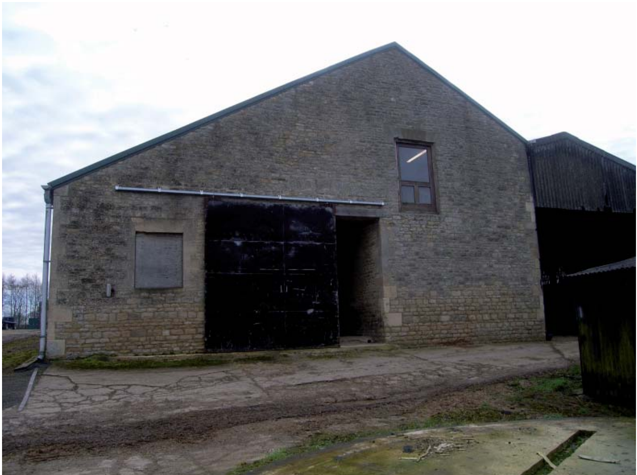
Plate 12: Barn 2; west elevation
