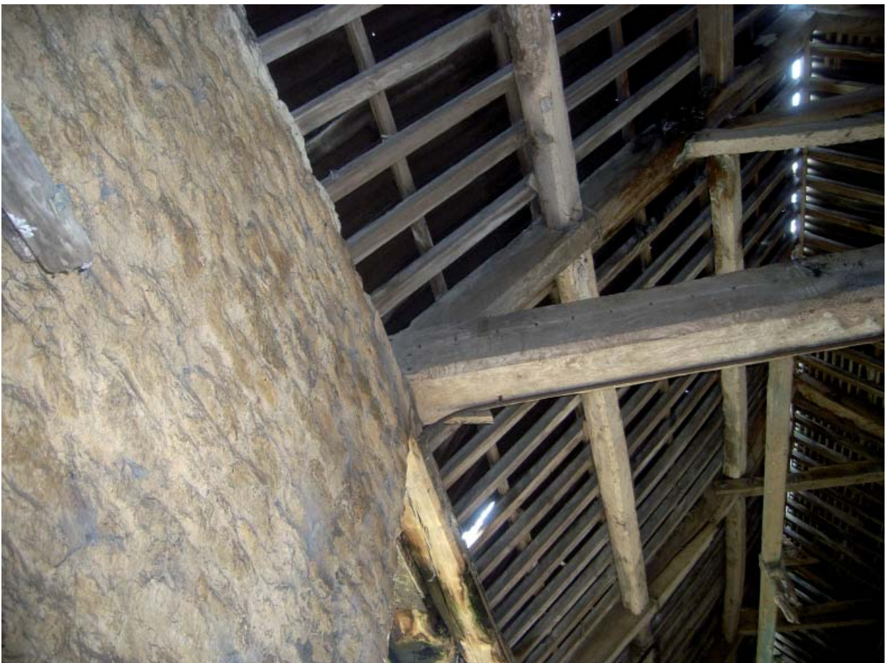
Plate 38: Barn 3; stopped chamfered tie-beam
