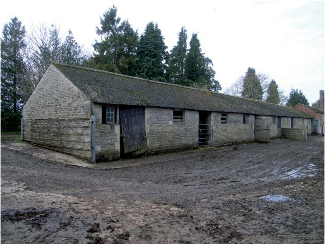
Plate 41: Barn 5; east and north elevations looking south west
