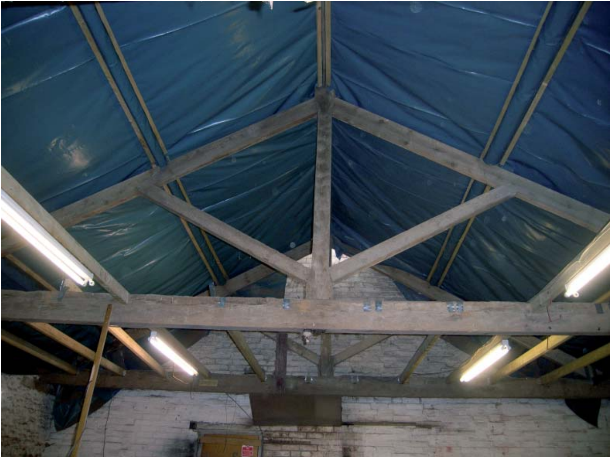
Plate 17: Barn 2; Roof truss in Modern Carpenter's Workshop
