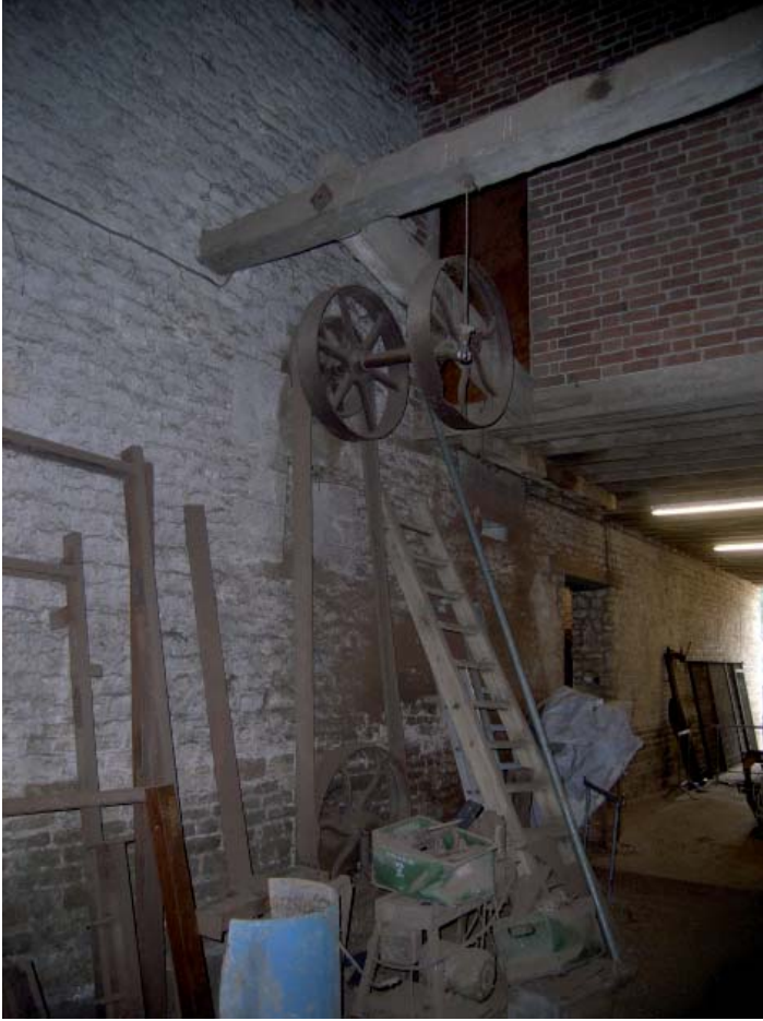
Plate 29: Barn 2; drive machinery between the Mill House and Passageway
