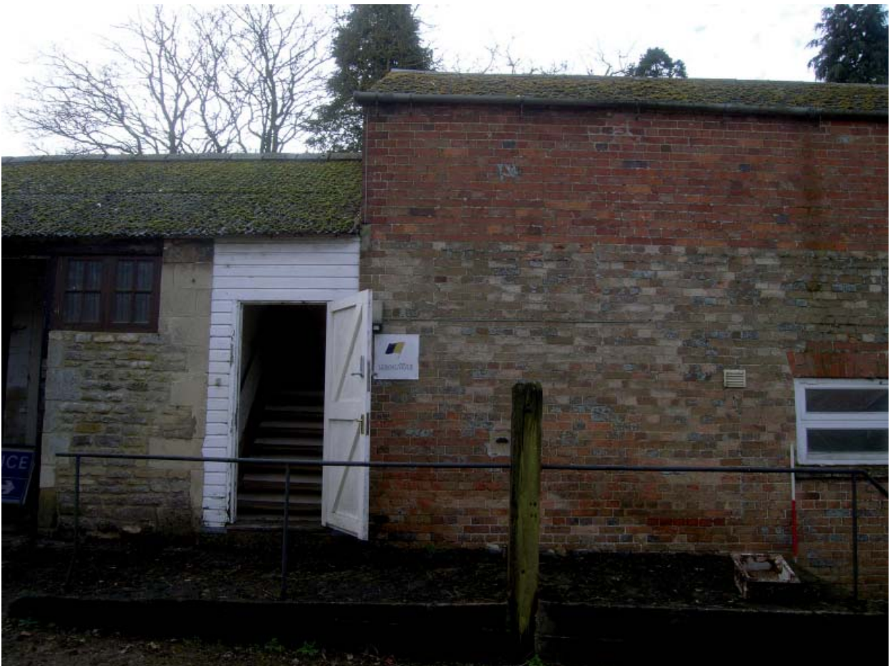
Plate 42: Barns 4 & 5; join between the block and the farmhouse on the north elevation
