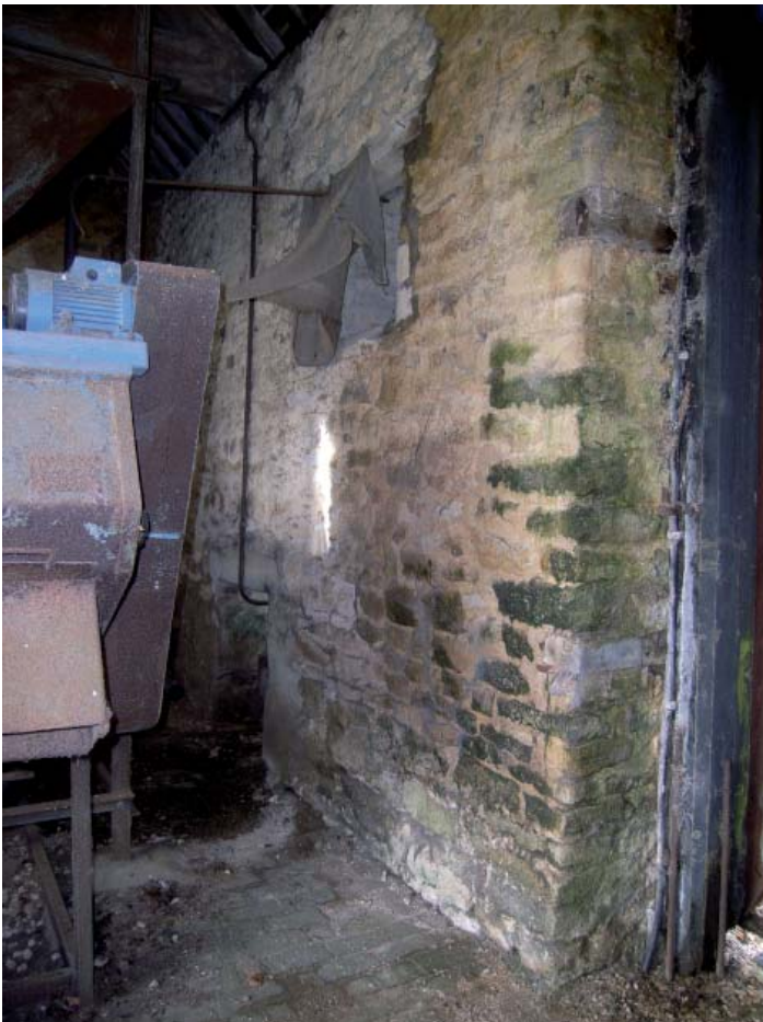
Plate 34: Barn 3; opening for modern machinery in the north wall
