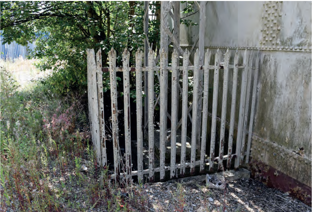
Plate 56: Enclosure at base of staircase of Holder 115
