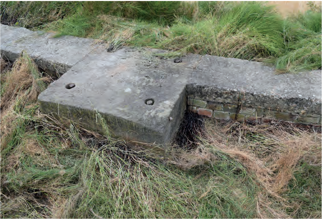
Plate 91: Details of base of former gasholder to north of site
