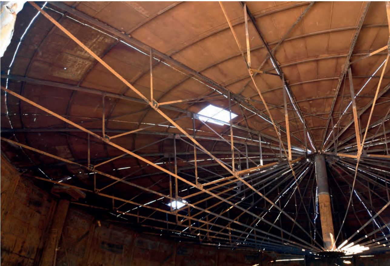
Plate 74: Crown structure in 115 during demolition
