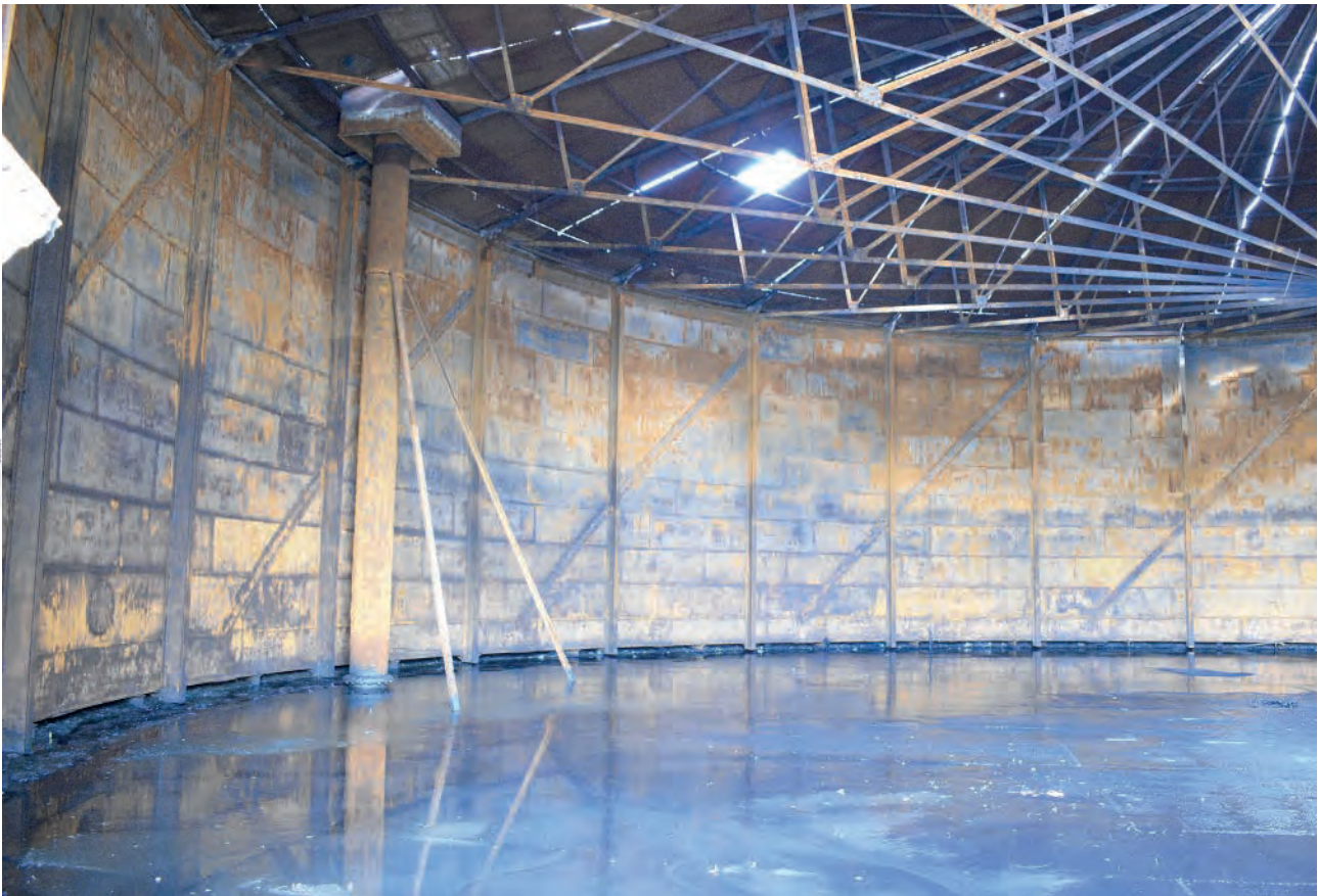
Plate 76: Interior of Holder 115 during demolition
