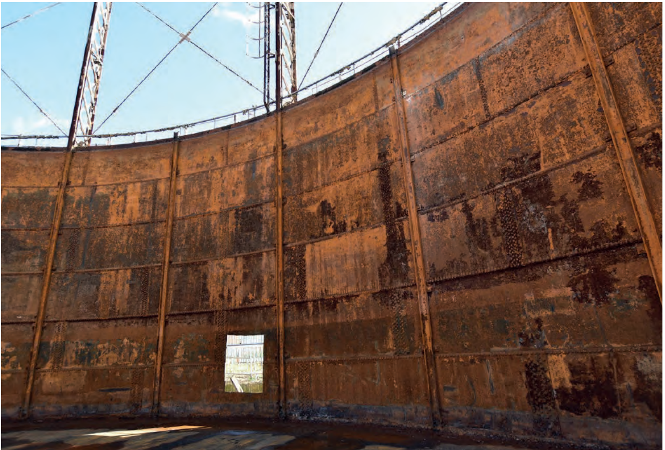
Plate 35: Holder 114 during demolition, after removal of crown
