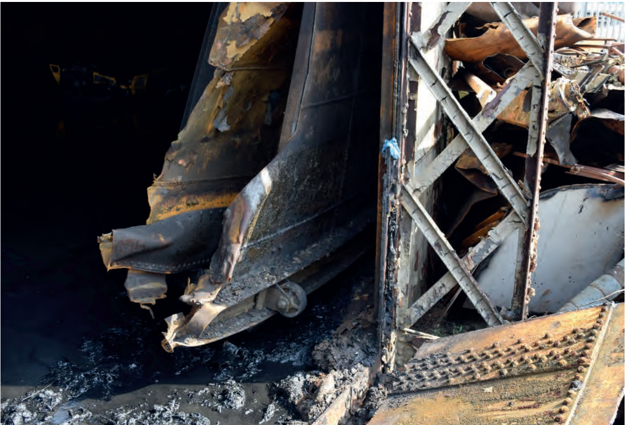
Plate 37: Detail during demolition showing guide rollers
