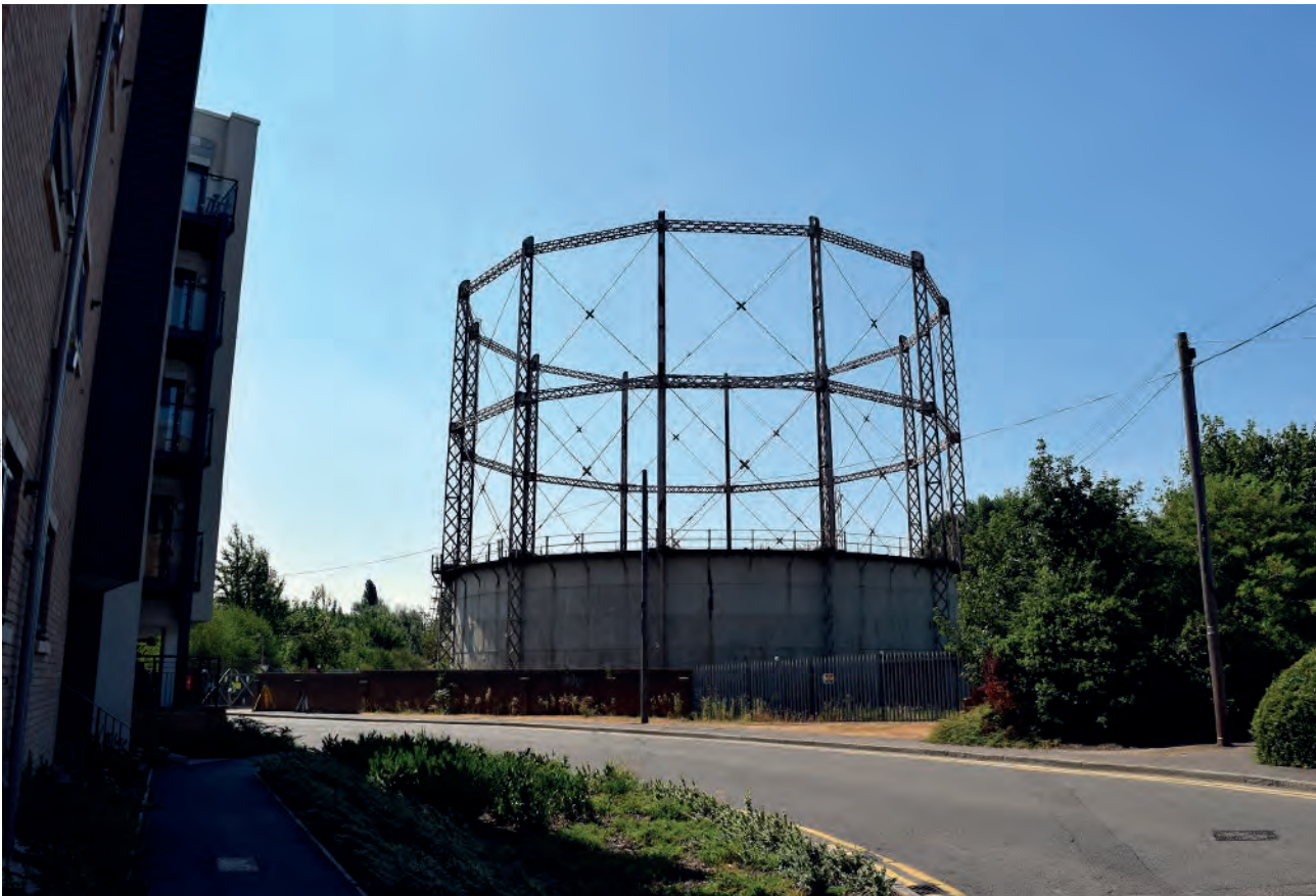
Plate 1: Holder 114 from north on Wharf Road
