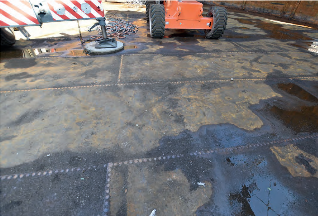
Plate 39: Riveted plates to floor of Holder 114
