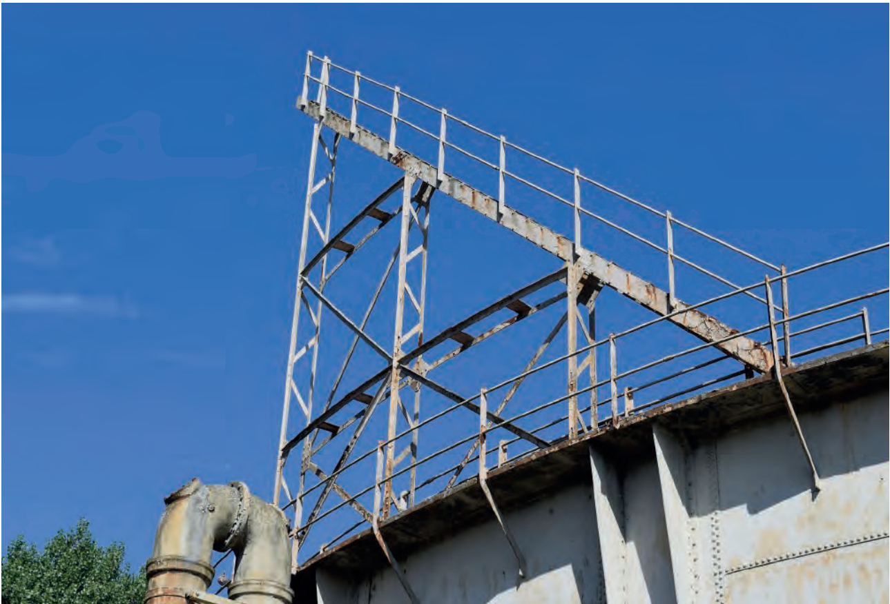
Plate 55: Ladder on top of tank of Holder 115
