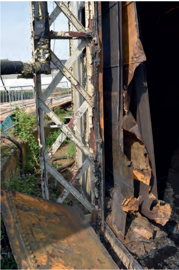
Plate 42: Detail during demolition
