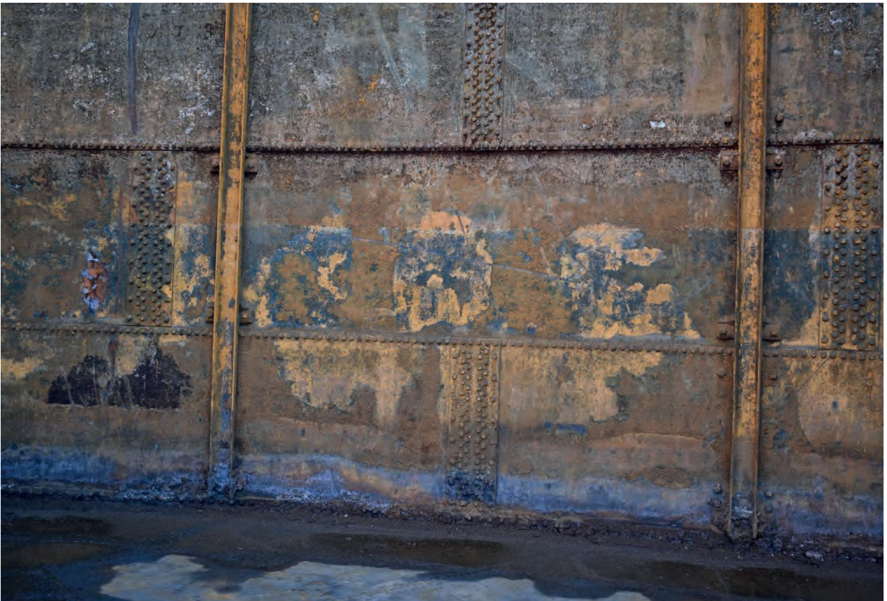
Plate 41: Internal face of inner lift during demolition
