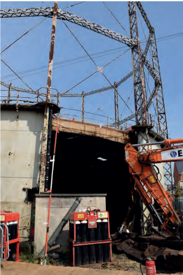
Plate 44: Opening formed in side of Holder 114
