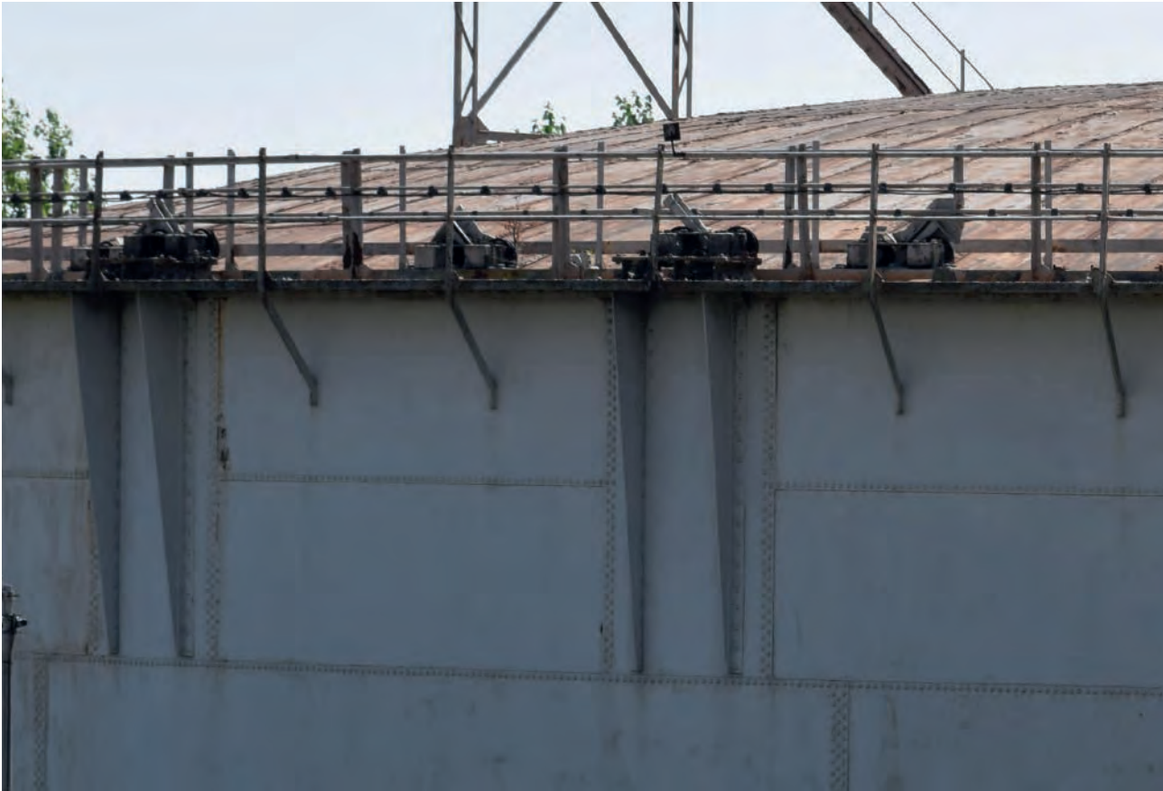
Plate 51: Detail of guide rollers on top of Holder 115
