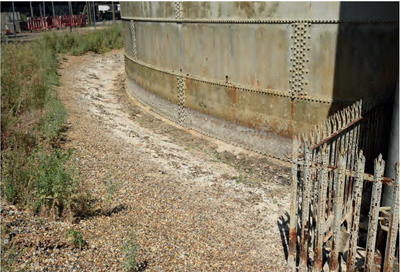
Plate 53: Depression around Holder 115, SW side
