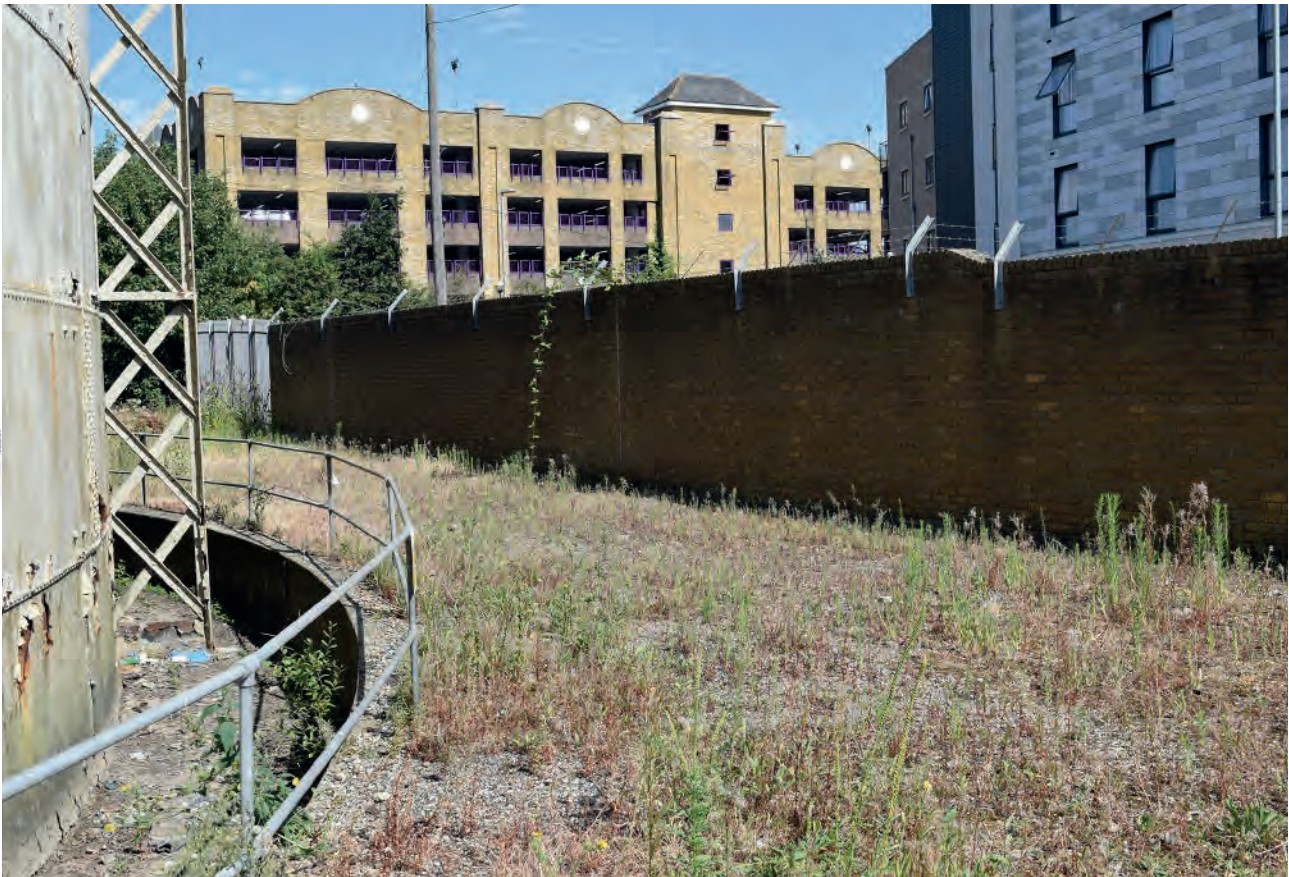
Plate 26: Boundary wall to north-east of Holder 114
