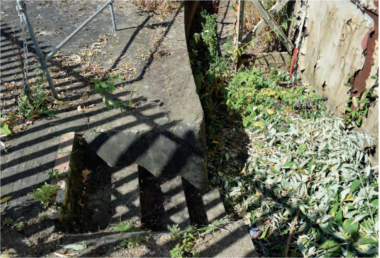
Plate 24: Steps into trench around Holder 114
