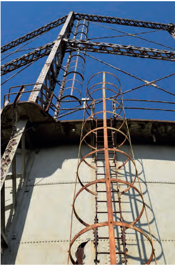
Plate 17: Ladder to east side of Holder 114
