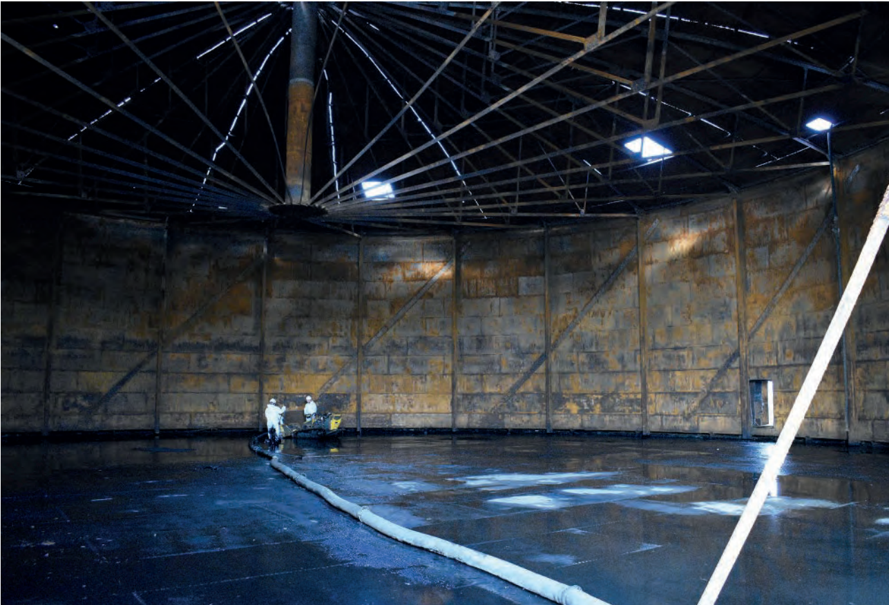
Plate 75: Interior of Holder 115 during demolition
