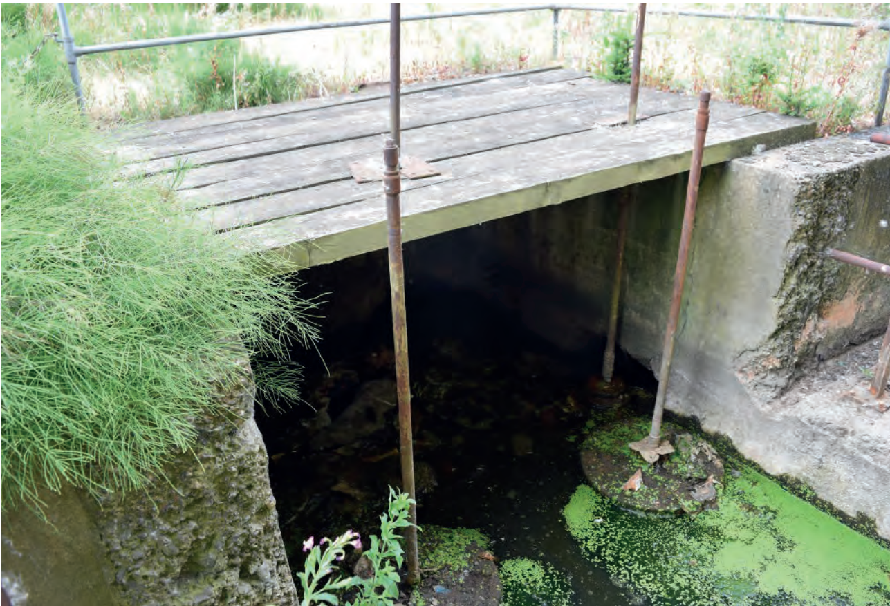
Plate 83: Valve pit to north of Holder 114
