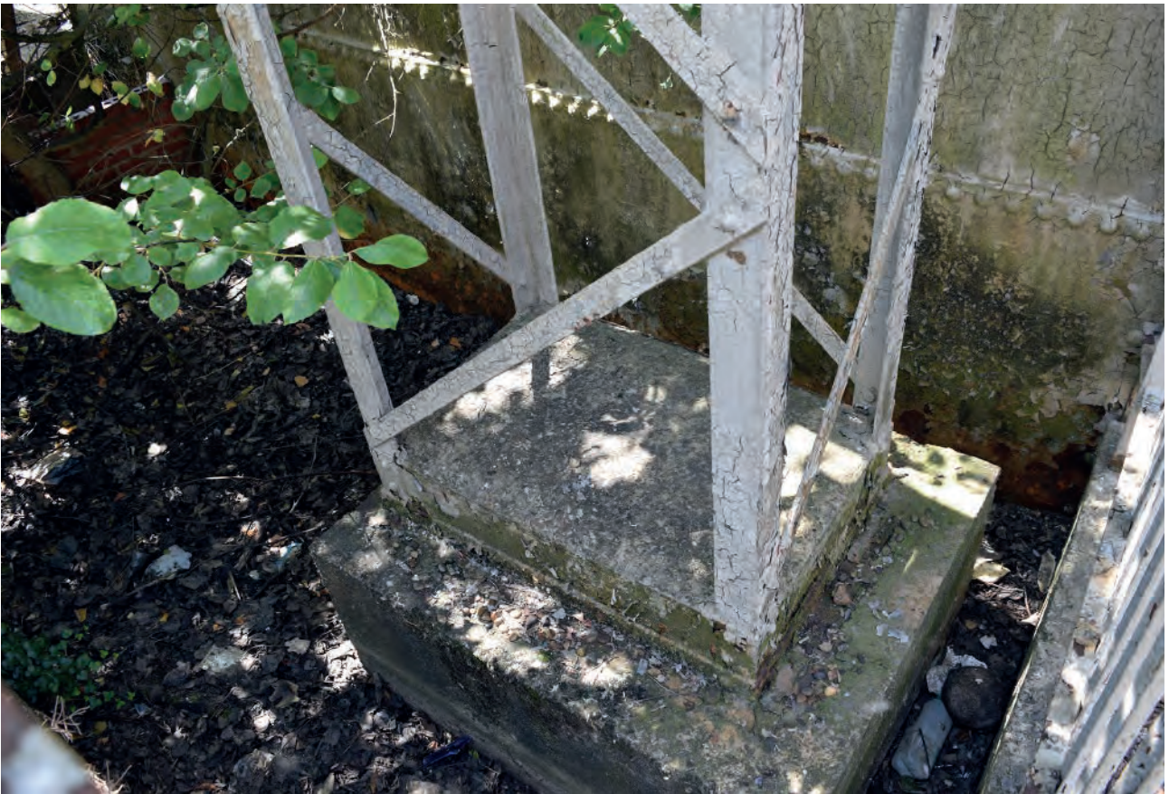
Plate 60: Stanchion supports for Holder 115 staircase
