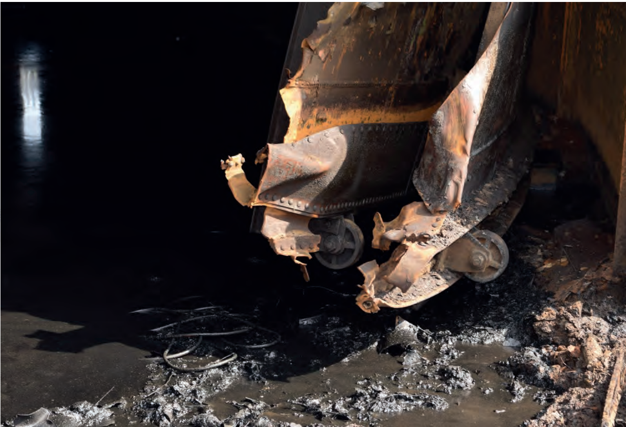
Plate 38: Detail during demolition showing guide rollers
