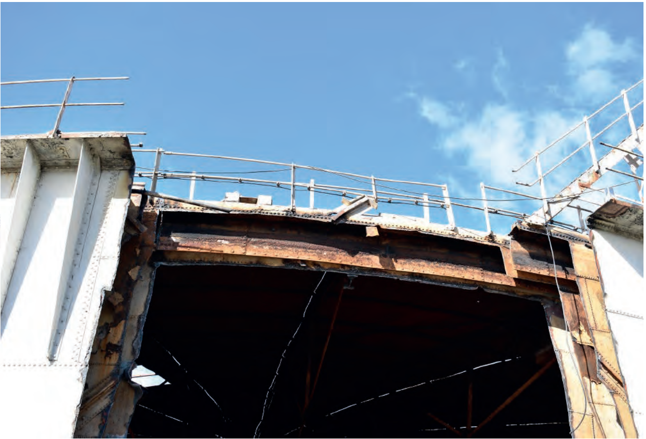
Plate 72: Opening created in 115 during demolition
