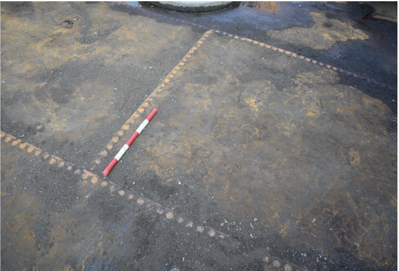
Plate 40: Riveted plates to floor of Holder 114
