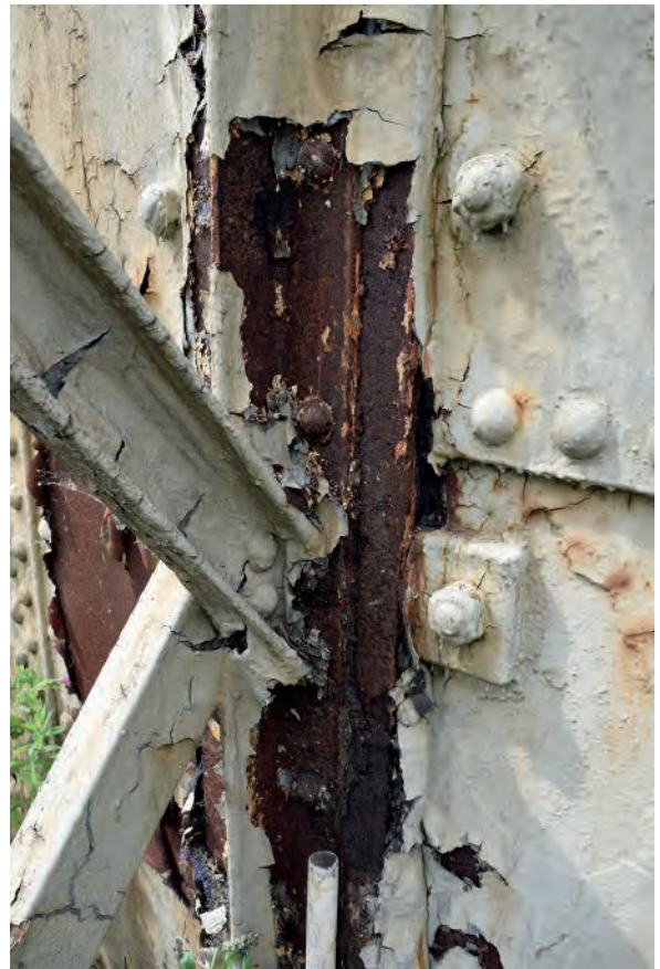
Plate 22: Detail of standard fixed to tank (Holder 114)
