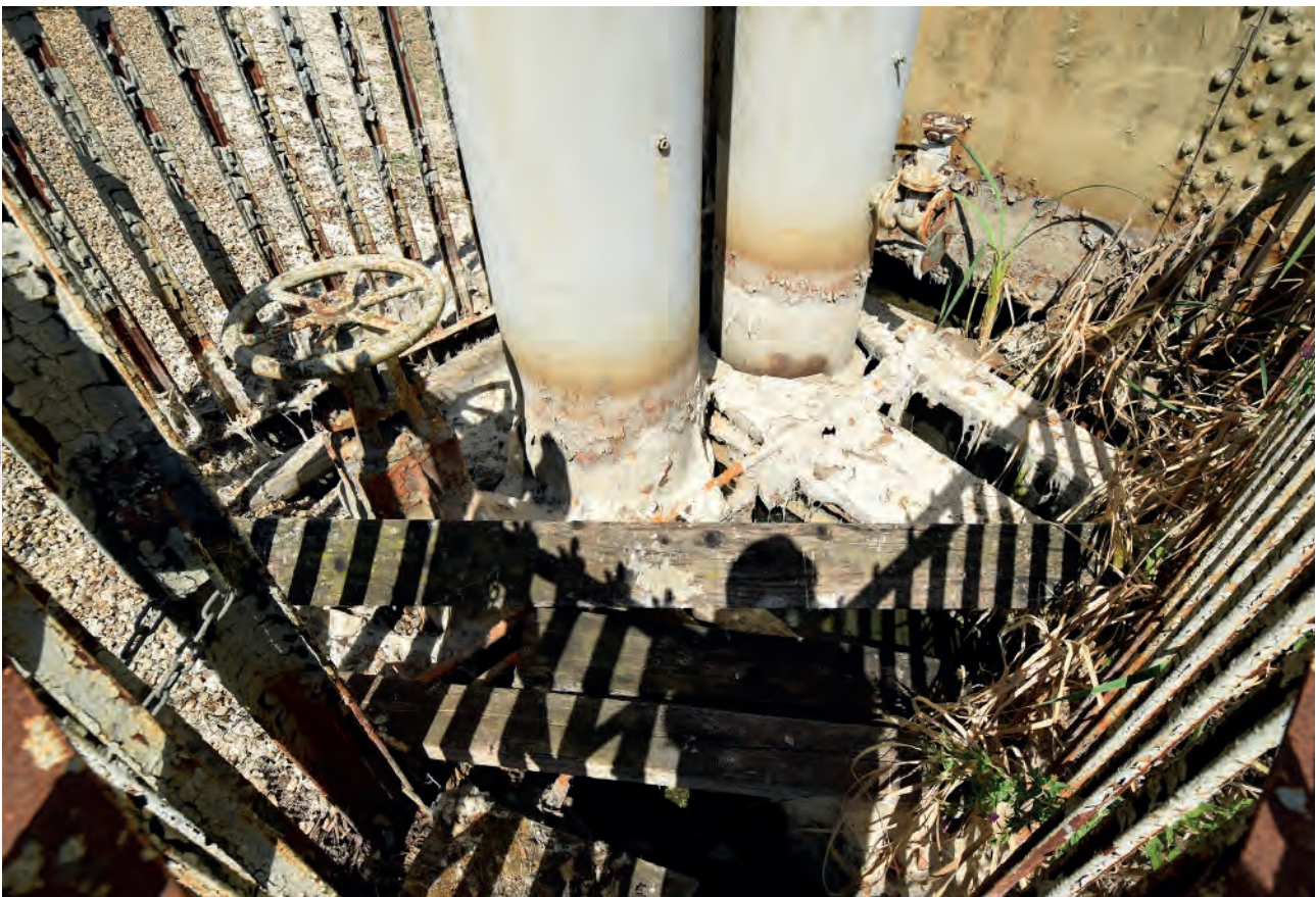
Plate 58: Valve pit to south side of Holder 115
