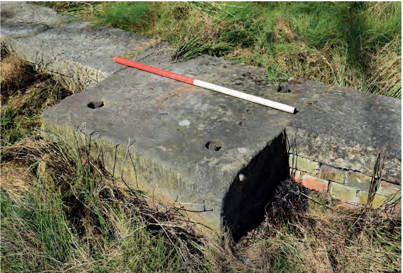
Plate 92: Details of base of former gasholder to north of site
