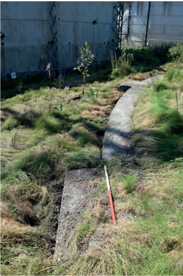
Plate 93: Details of base of former gasholder to north of site
