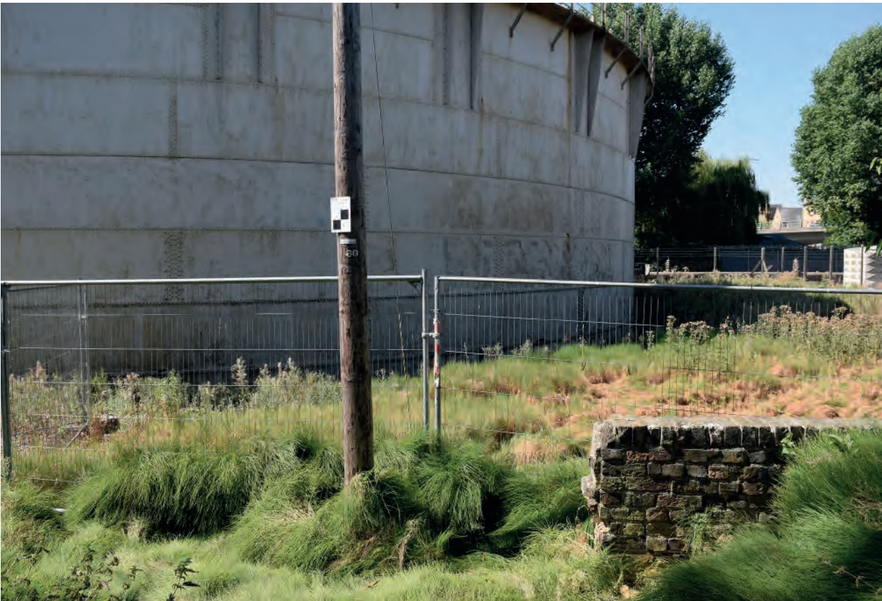
Plate 81: Boundary wall between holders
