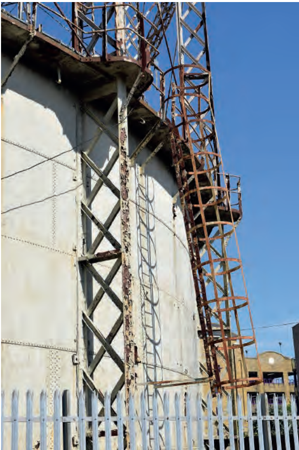
Plate 15: Ladder to side of Holder 114
