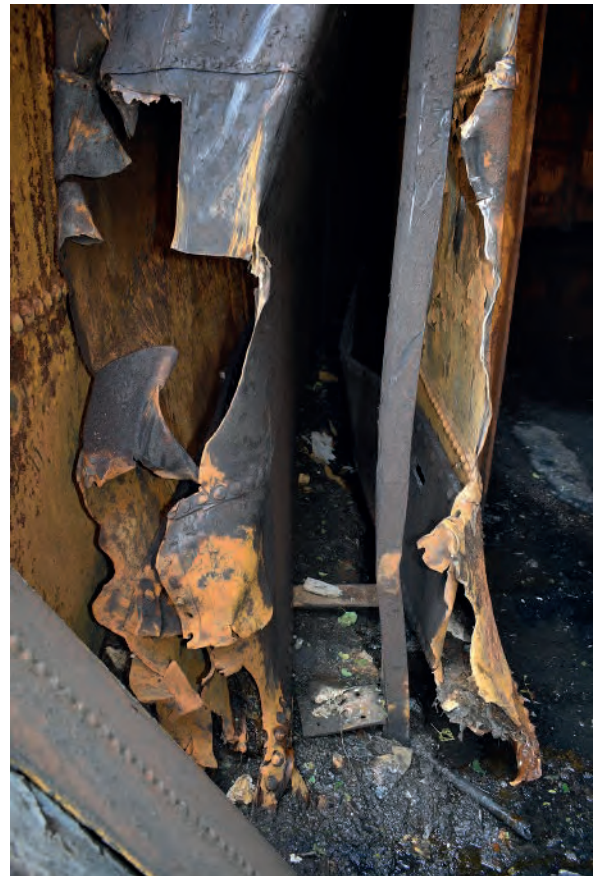
Plate 68: Detail of lifts during demolition of Holder 115
