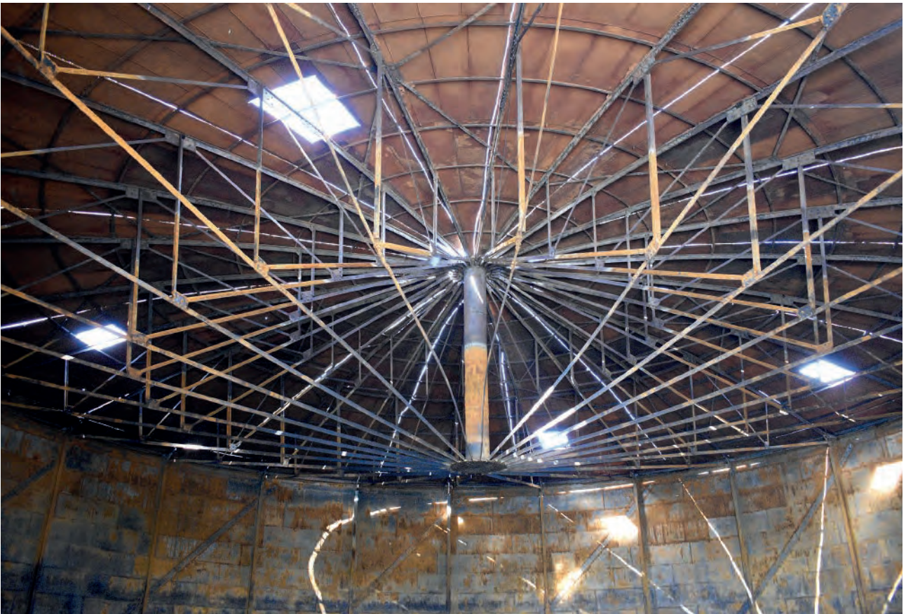
Plate 73: Crown structure in 115 during demolition
