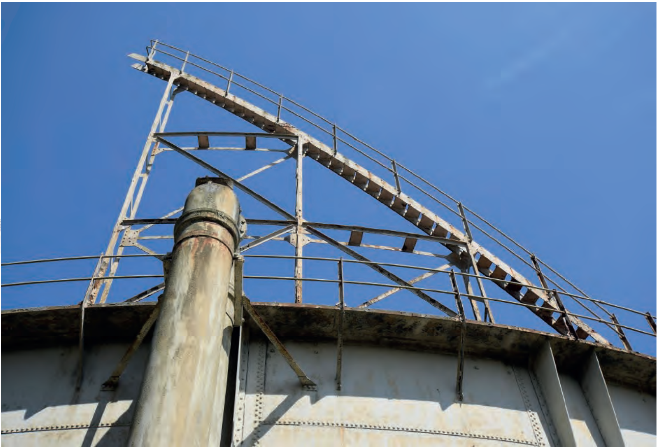
Plate 54: Ladder on top of tank of Holder 115
