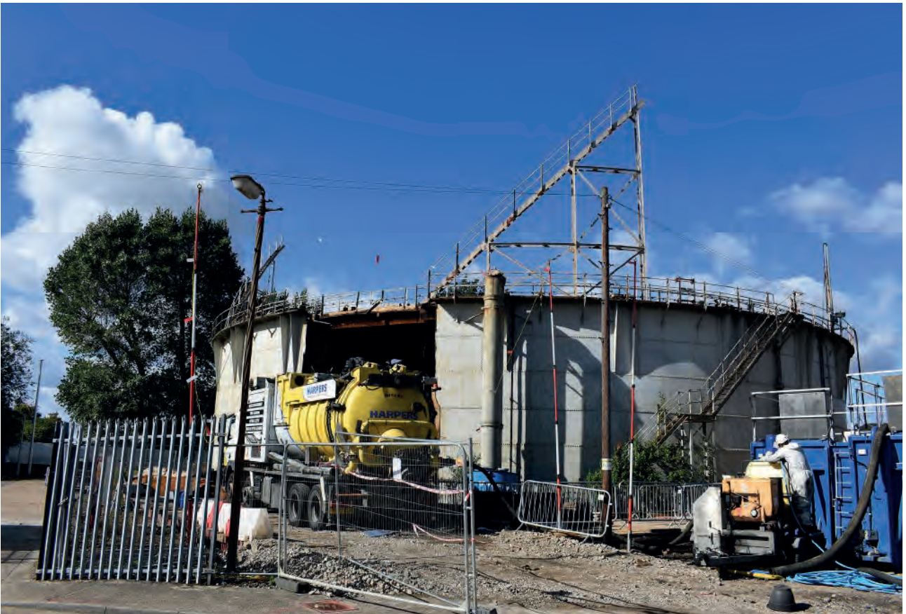
Plate 71: General view of Holder 115 during demolition
