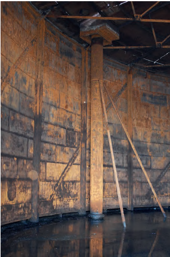
Plate 77: Vertical pipe in Gasholder 115
