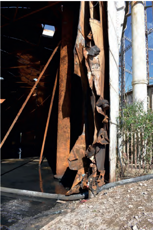
Plate 69: Detail during demolition of Holder 115
