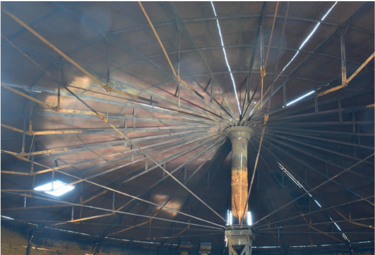
Plate 27: Crown structure to Holder 114
