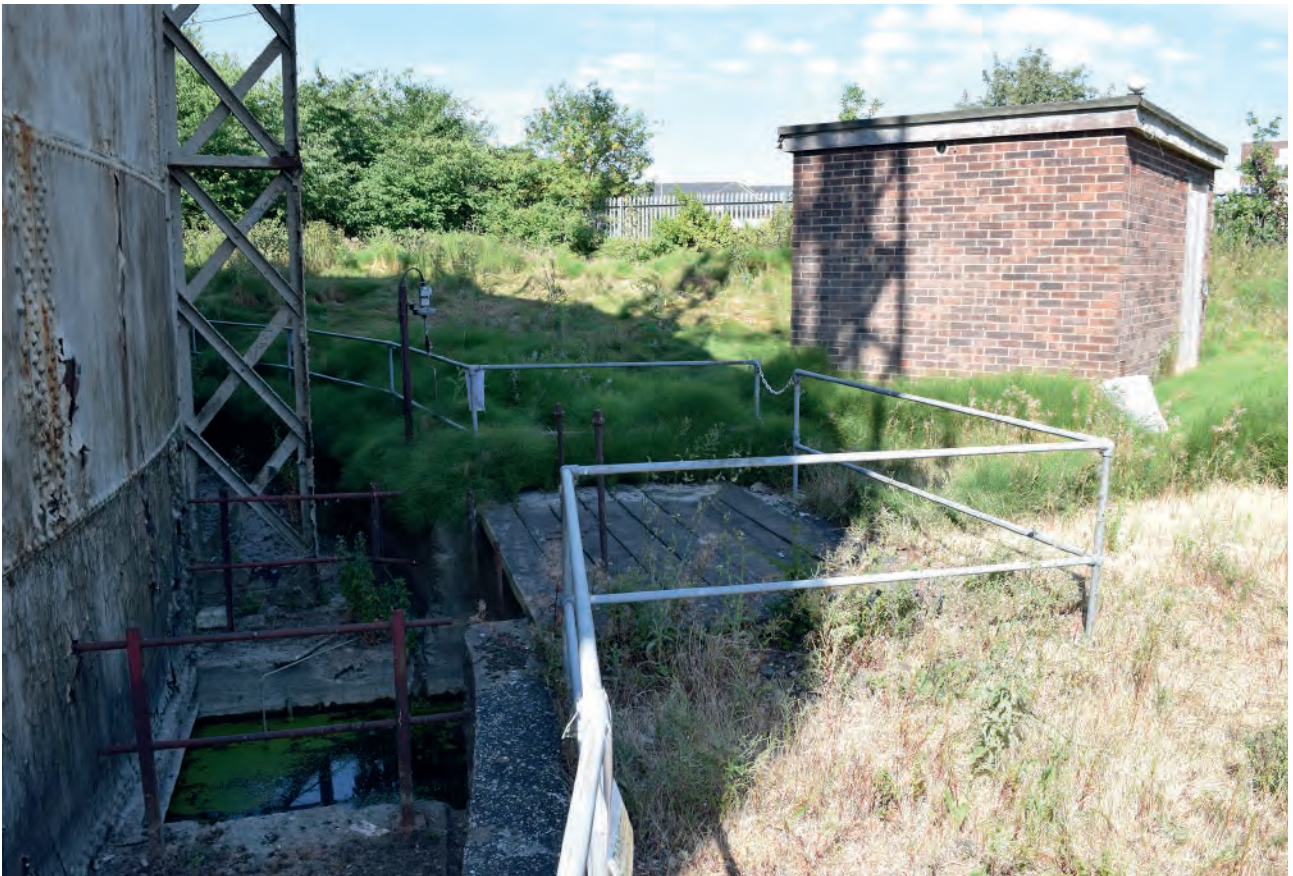
Plate 23: Valve pit and building to north side of Holder 114
