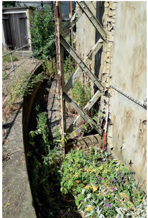
Plate 20: Base of standard (Holder 114)
