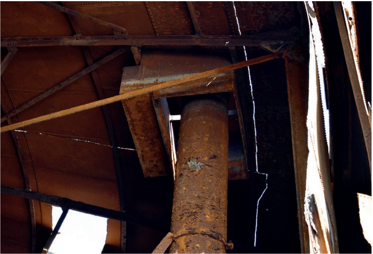
Plate 79: Detail of head of pipe within Holder 115
