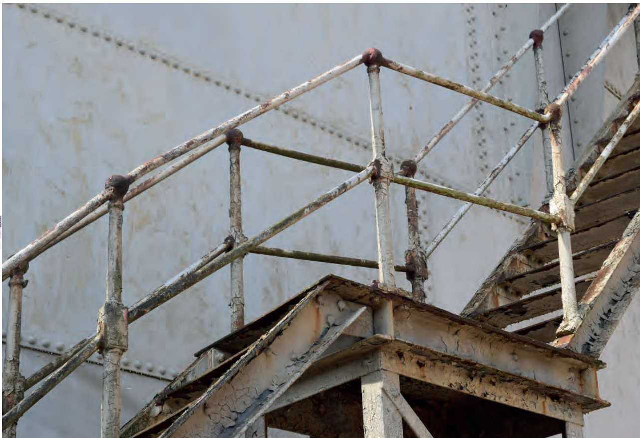
Plate 62: Detail of stairs to east side of Holder 115
