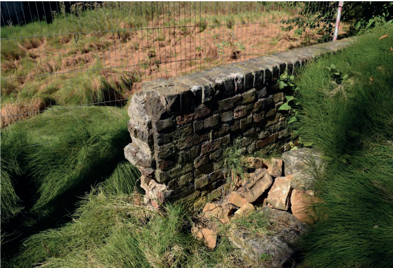
Plate 82: Boundary wall between holders
