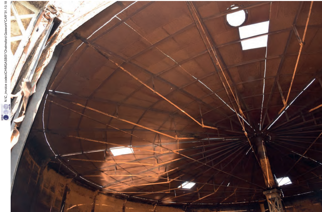
Plate 30: Crown structure to Holder 114
