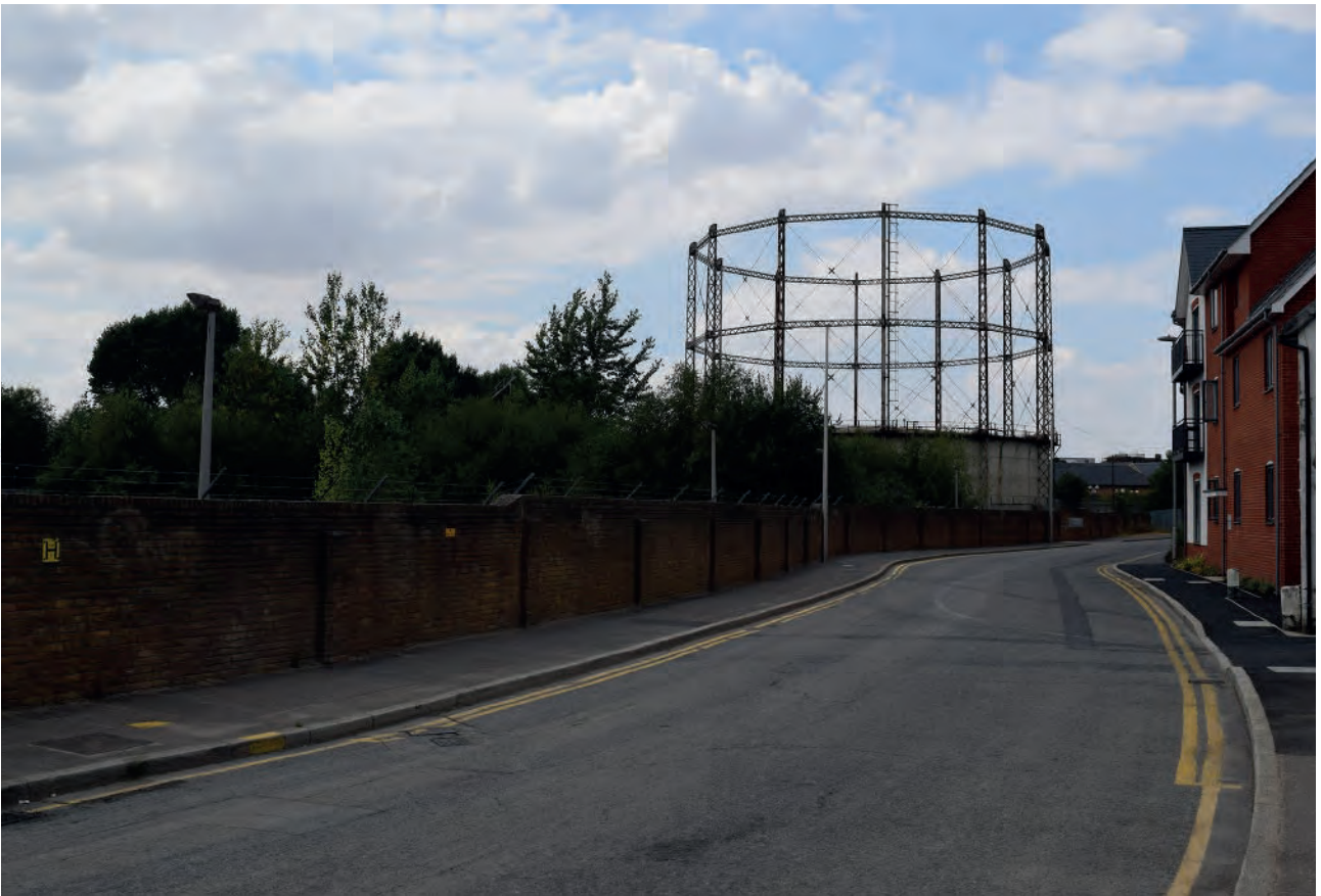
Plate 5: General view of Holder 114 from south-east
