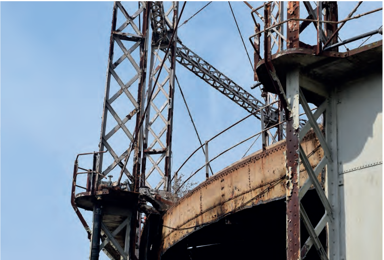
Plate 36: Detail during demolition
