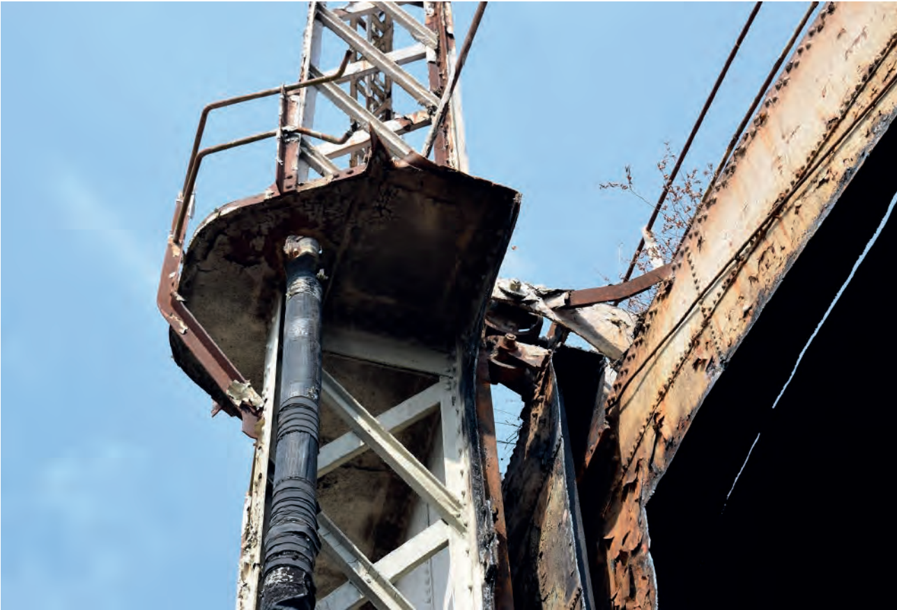
Plate 33: Detail of standard during demolition of Holder 114
