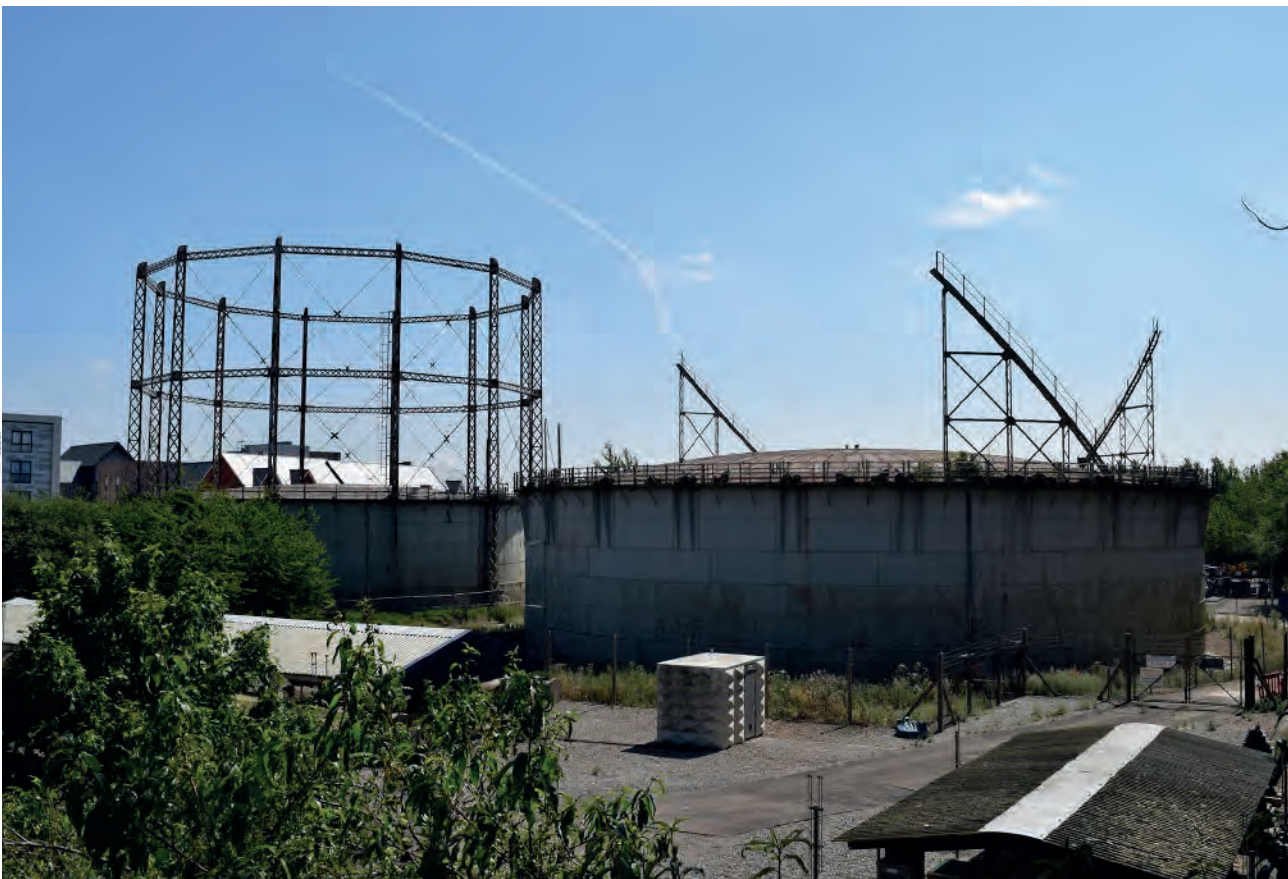
Plate 46: General view of holders from flyover to west
