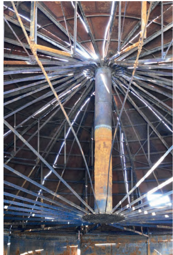
Plate 78: Central shaft within Holder 115
