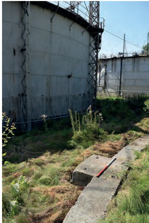
Plate 95: Details of base of former gasholder to north of site
