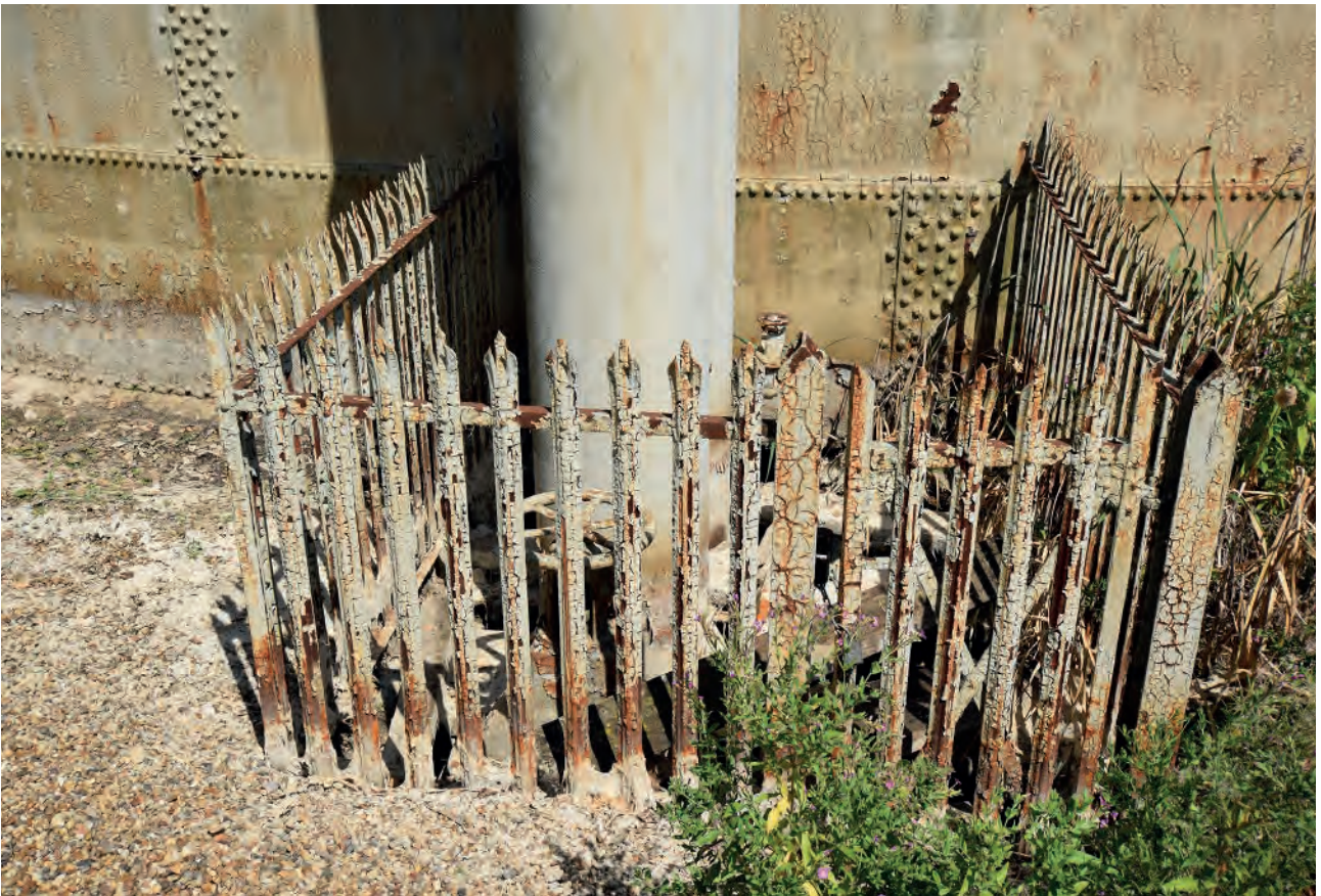
Plate 57: Enclosure around pipes and valve pit to south of 115
