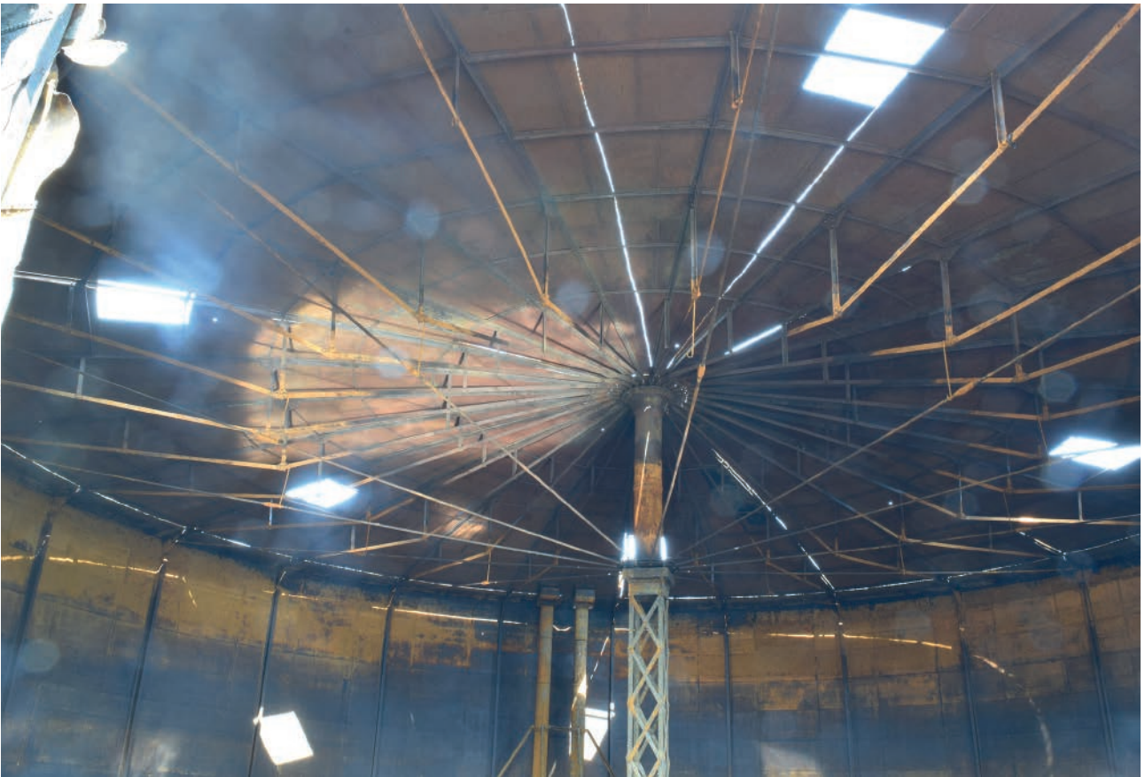
Plate 28: Crown structure to Holder 114
