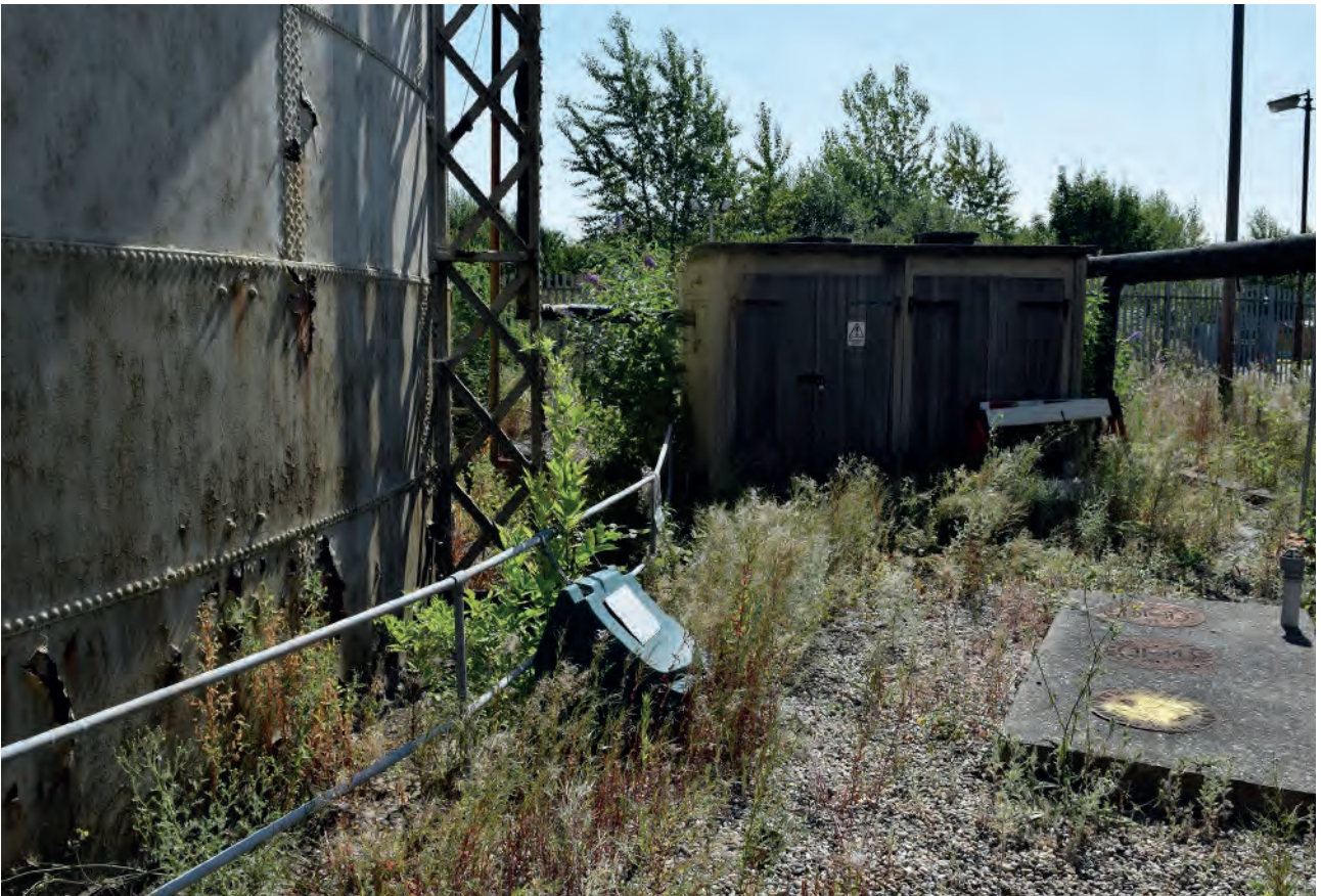
Plate 25: Boiler house to south side of 114
