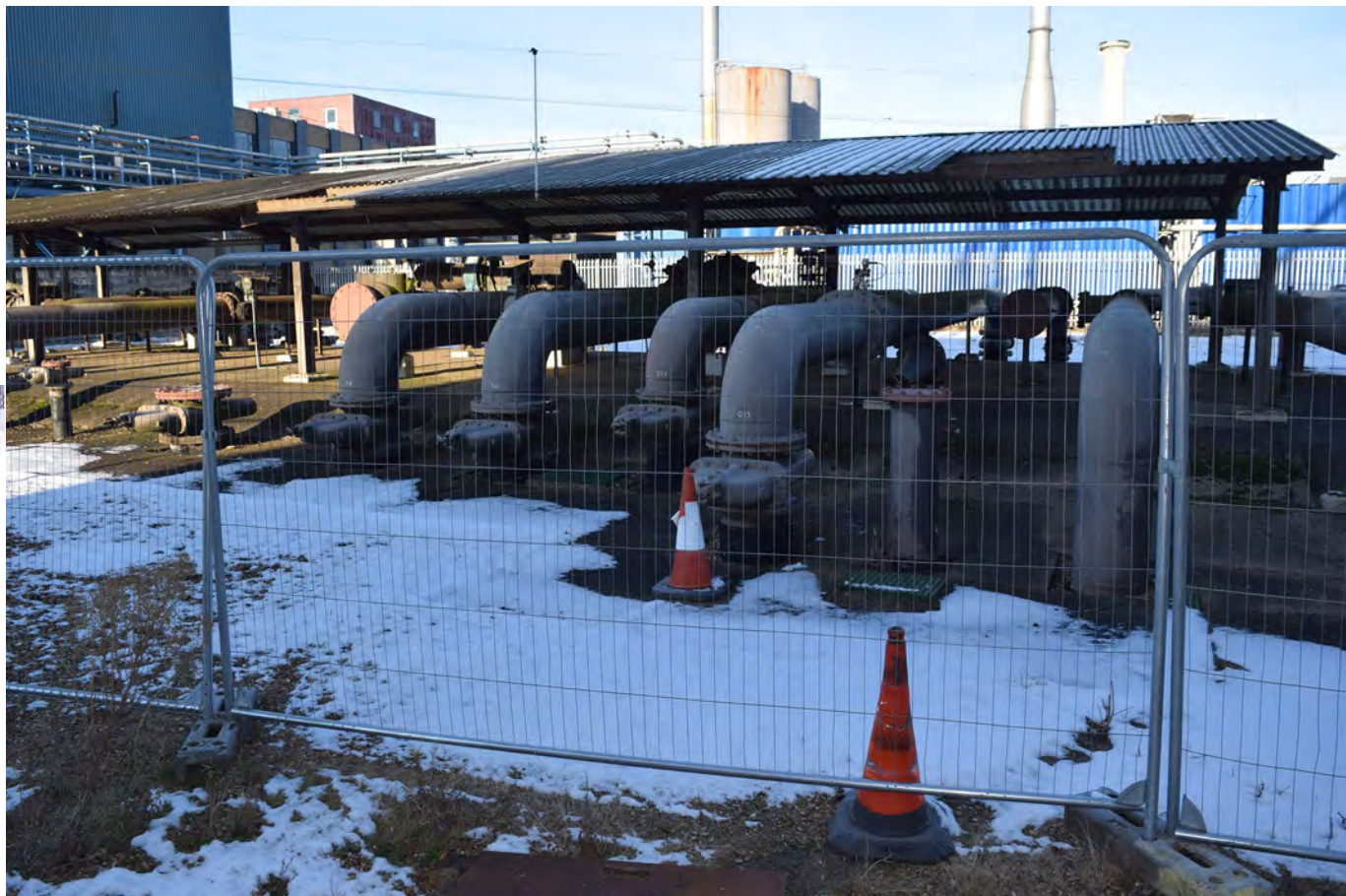
Plate 62: Plant to north-east of gasworks
