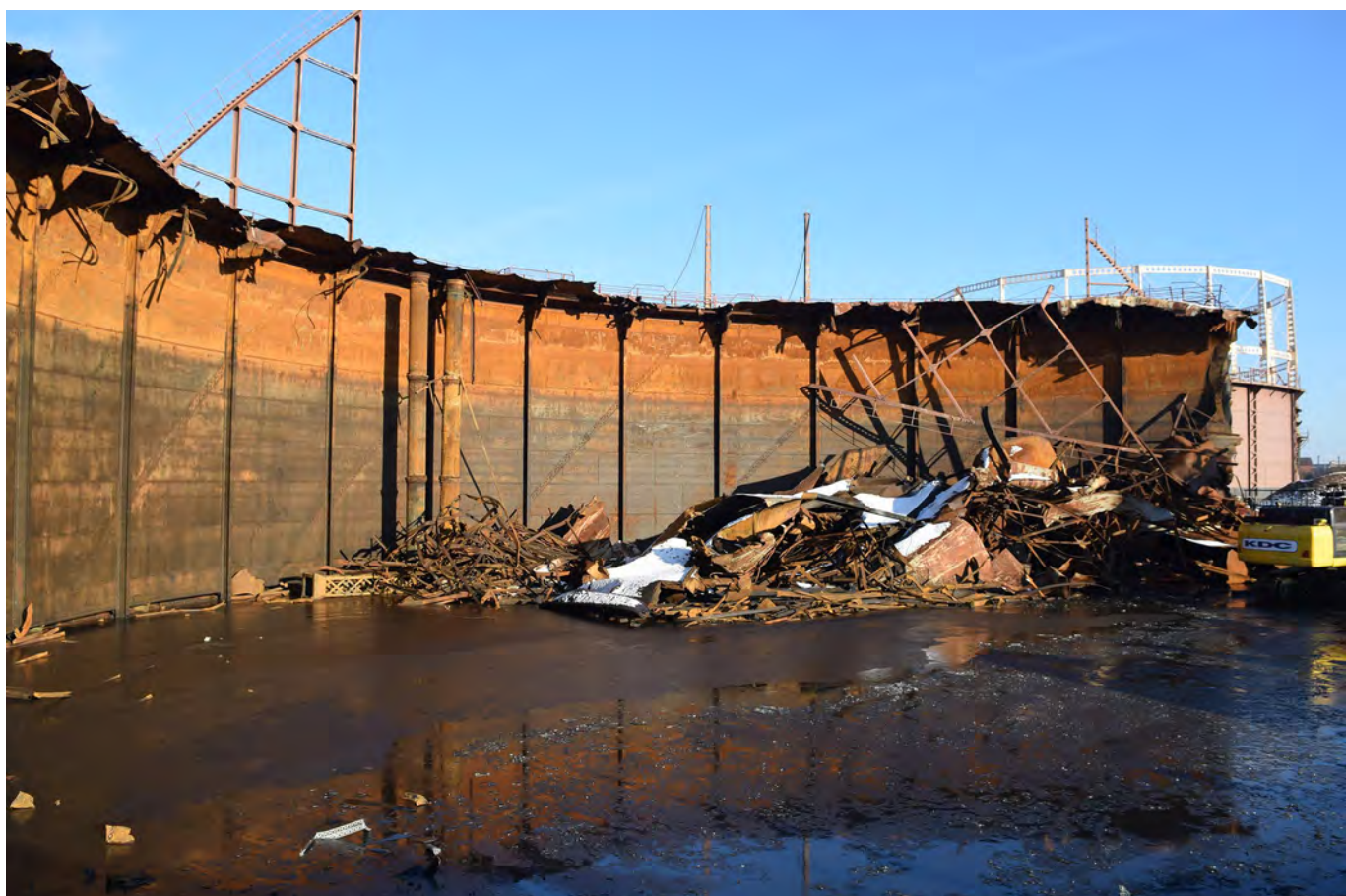
Plate 42: General view of Holder 71 during demolition
