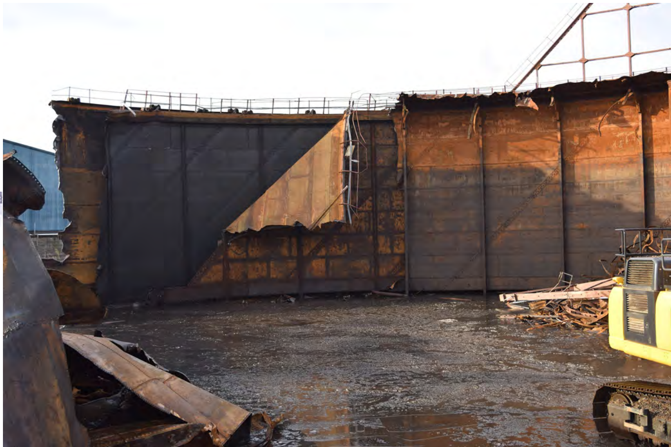
Plate 43: General view of Holder 71 during demolition
