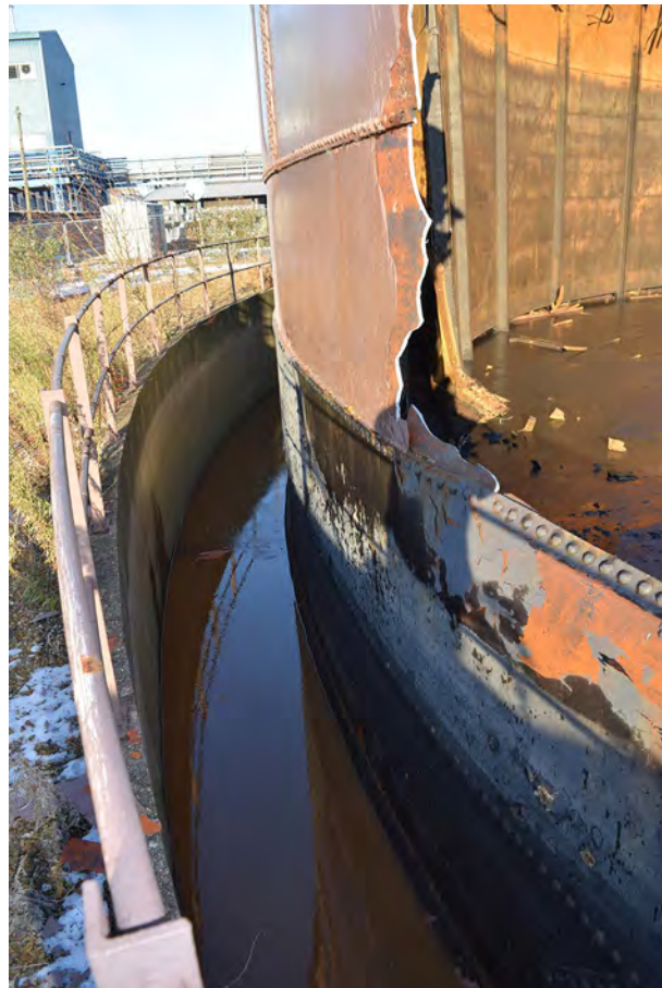
Plate 55: Trench around Holder 71
