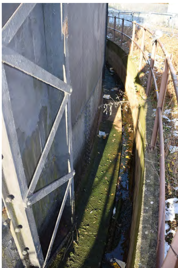
Plate 31: Trench around Holder 70
