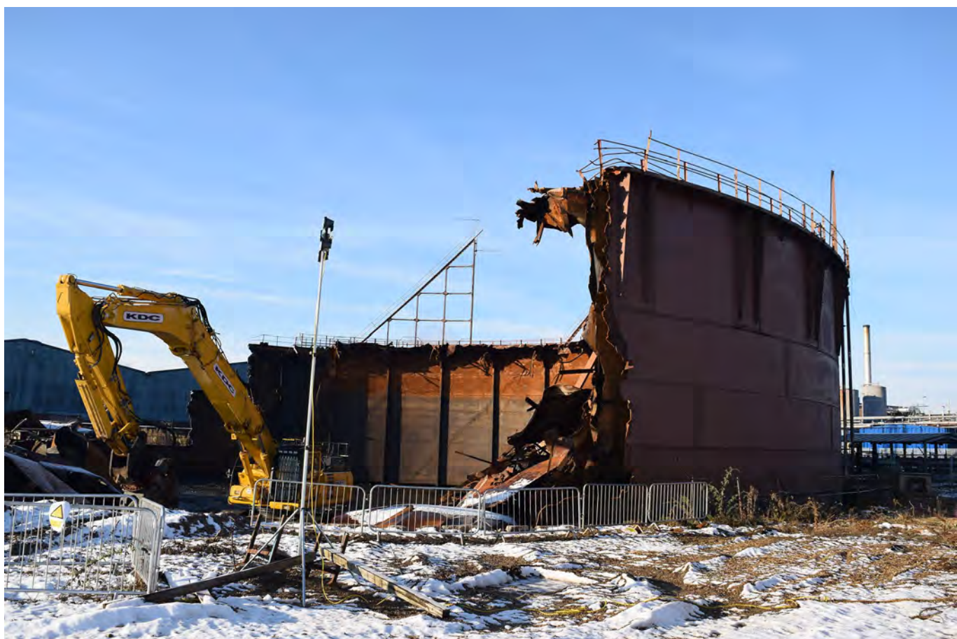
Plate 46: General view of Holder 71 during demolition
