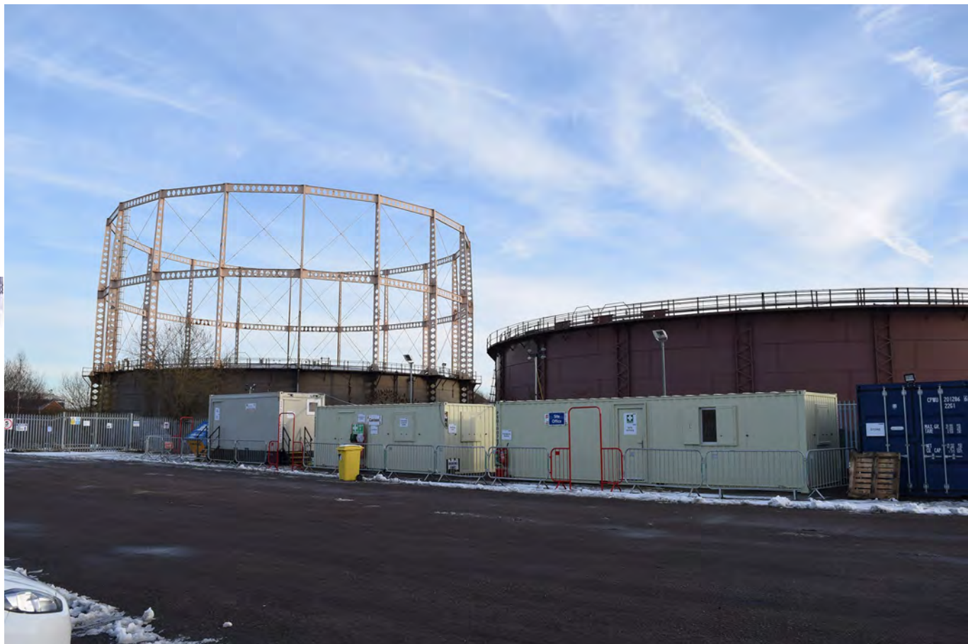
Plate 1: Holders 69 and 70 from north-west
