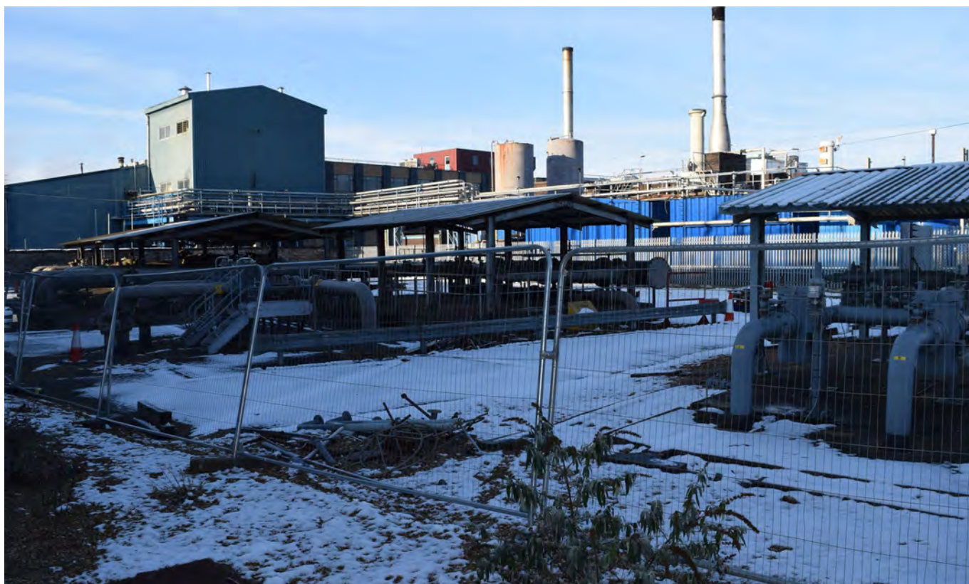
Plate 61: Plant to north-east of gasworks
