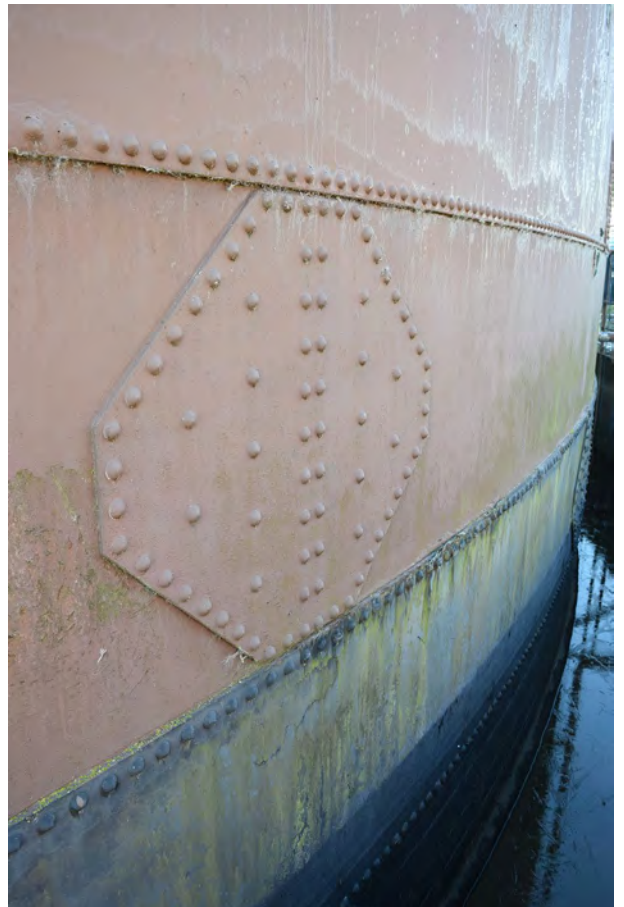
Plate 59: Junction plate to side of Holder 71
