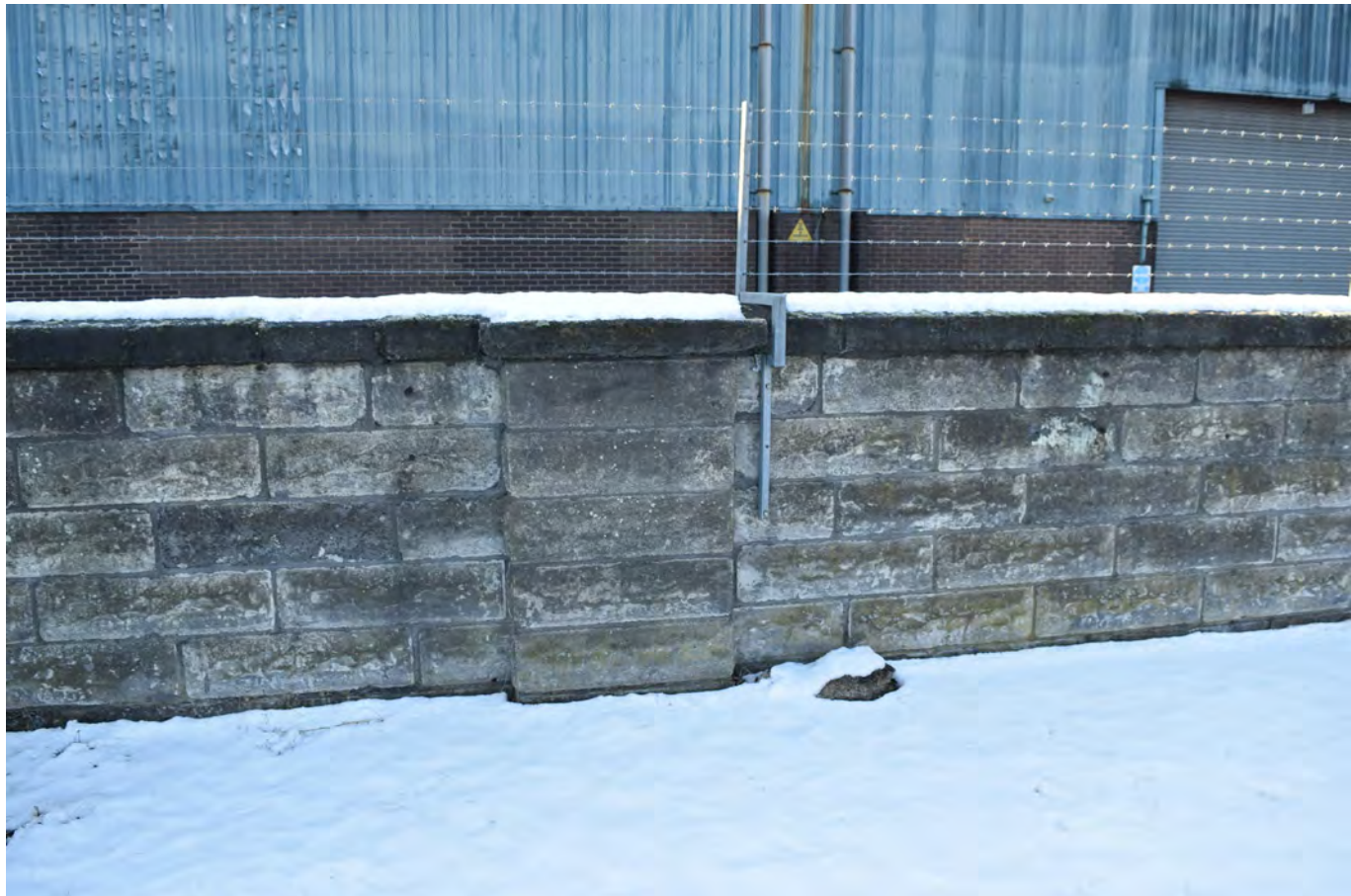
Plate 65: Typical section of wall to west side of site
