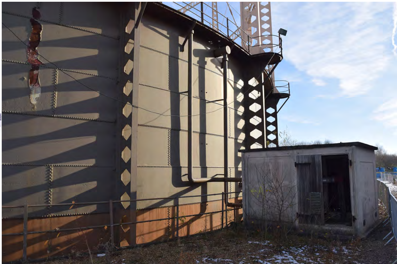
Plate 17: Plant building to west of Holder 69
