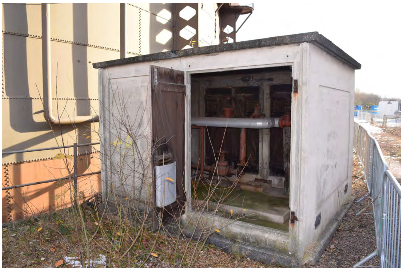
Plate 18: Plant building to west of Holder 69
