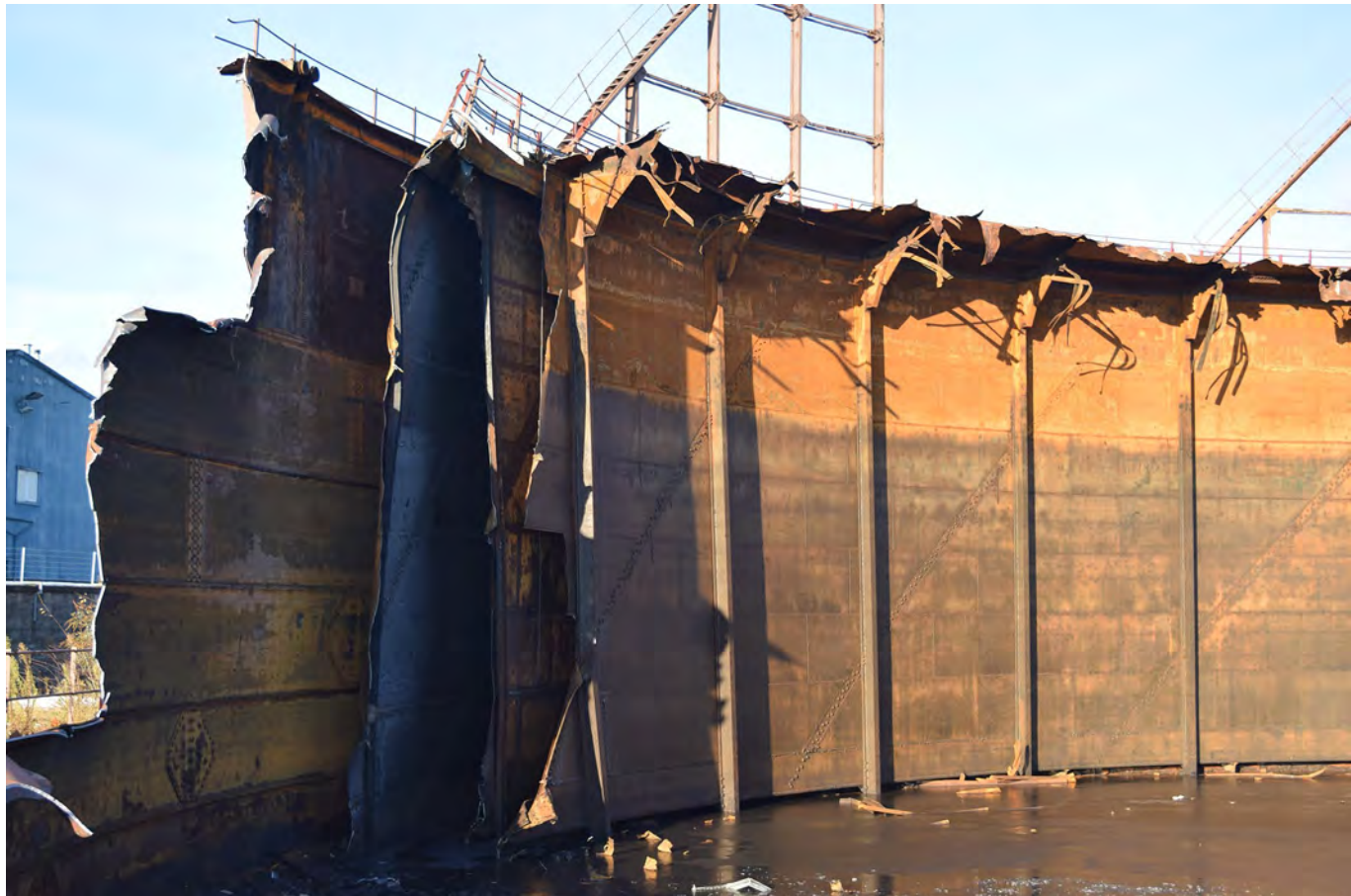
Plate 44: General view of Holder 71 during demolition
