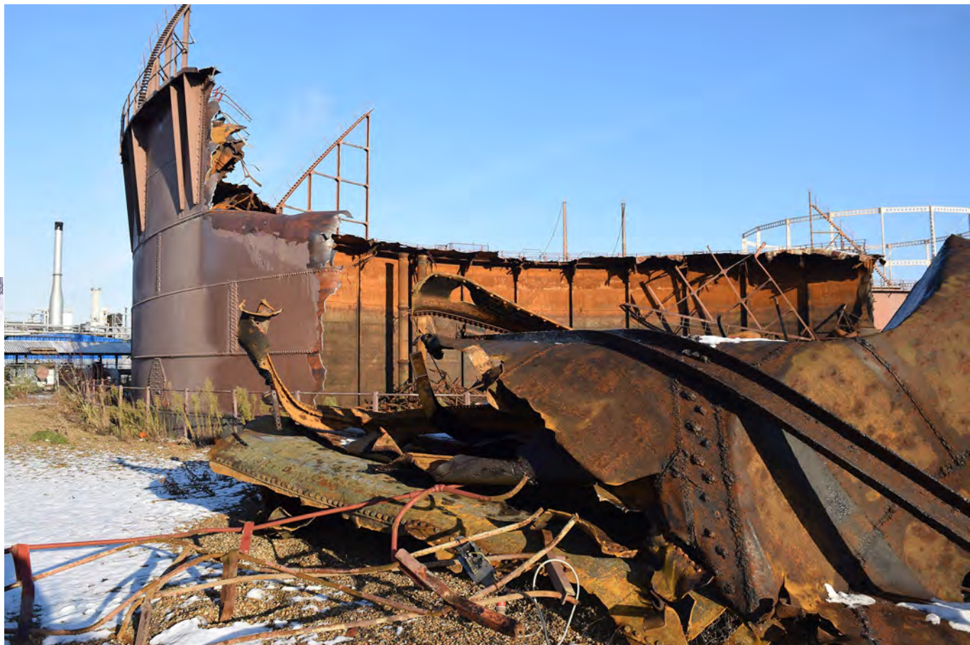
Plate 45: General view of Holder 71 during demolition
