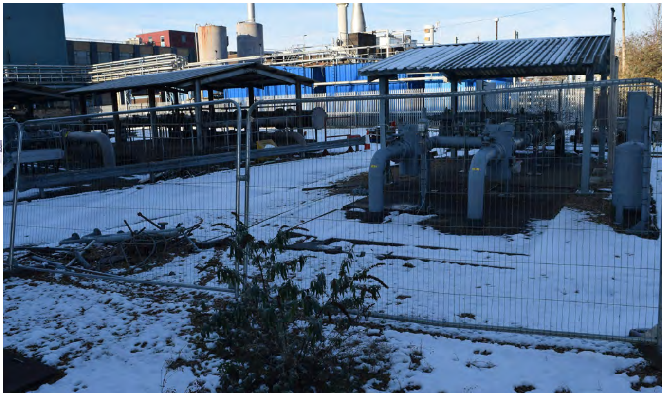
Plate 60: Plant to north-east of gasworks
