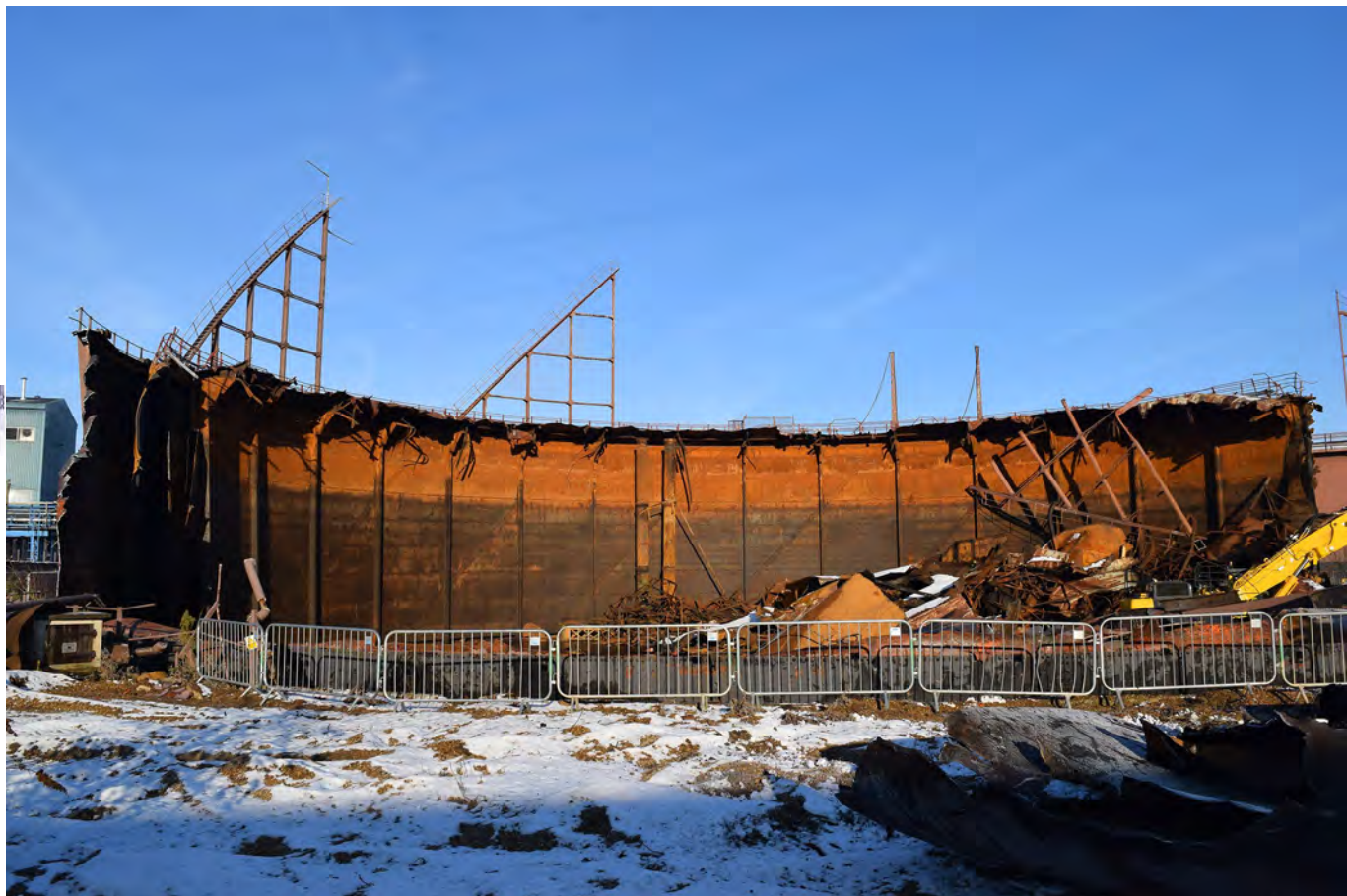
Plate 41: General view of Holder 71 during demolition
