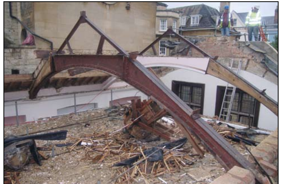
Plate 48: Roof of former lecture room during dismantling
