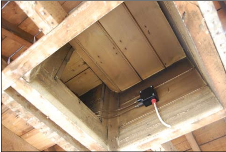
Plate 45: Underside of duct in ceiling of lecture room
