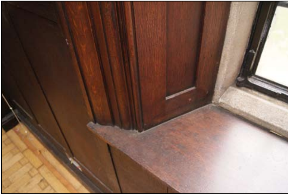
Plate 37: Window jamb detail in former lecture room
