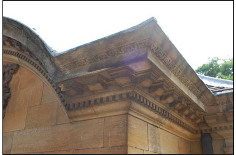
Plate 2: Eaves detail at north-west corner of main building
