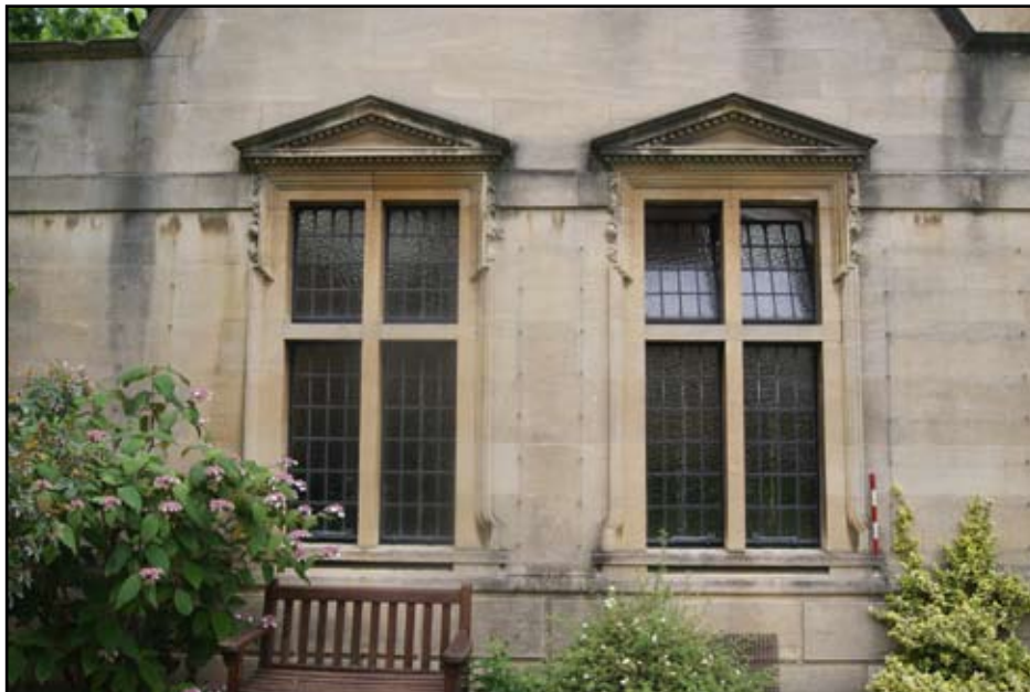
Plate 11: Windows in west wall of former lecture room
