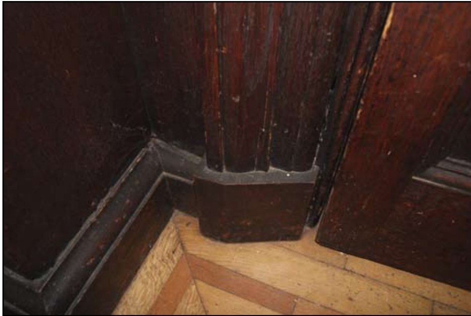
Plate 41: Skirting detail in former lecture room
