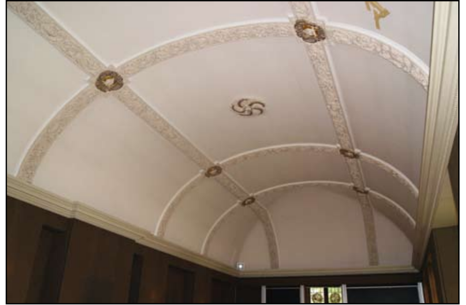
Plate 30: First floor of main building (Oakeshott Room)
