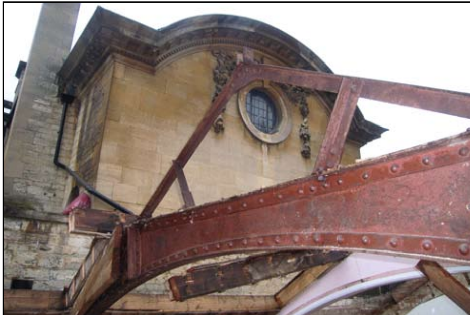
Plate 51: Truss in former lecture room
