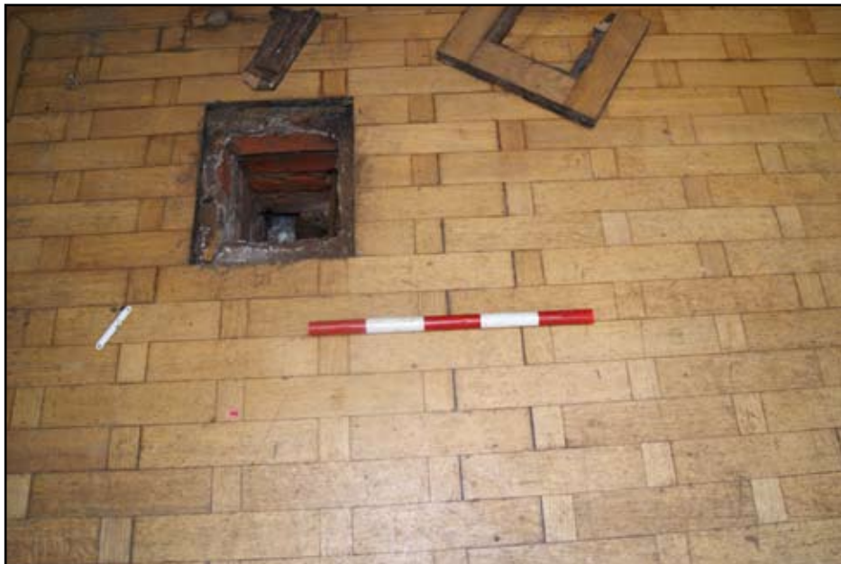
Plate 43: Floor in former lecture room
