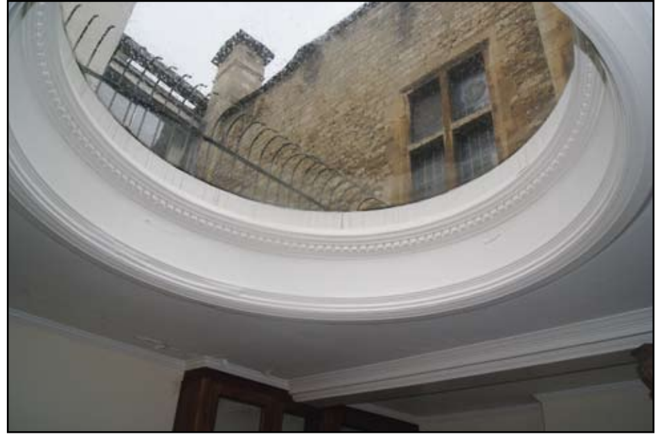
Plate 58: Roof light above lobby by foot of stairs
