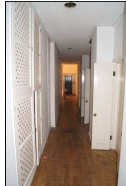
Plate 28: Ground floor corridor along east side of main building
