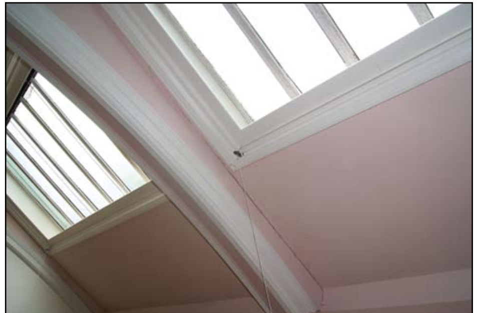
Plate 44: Roof lights in former lecture room
