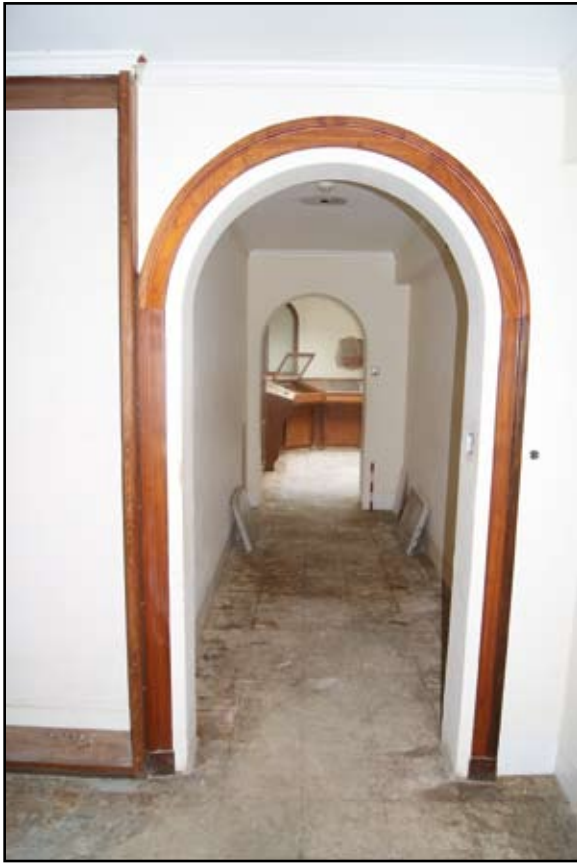
Plate 66: Arched corridor between lobbies to east of building
