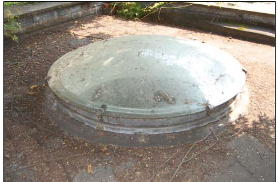
Plate 24: Domed roof light from above
