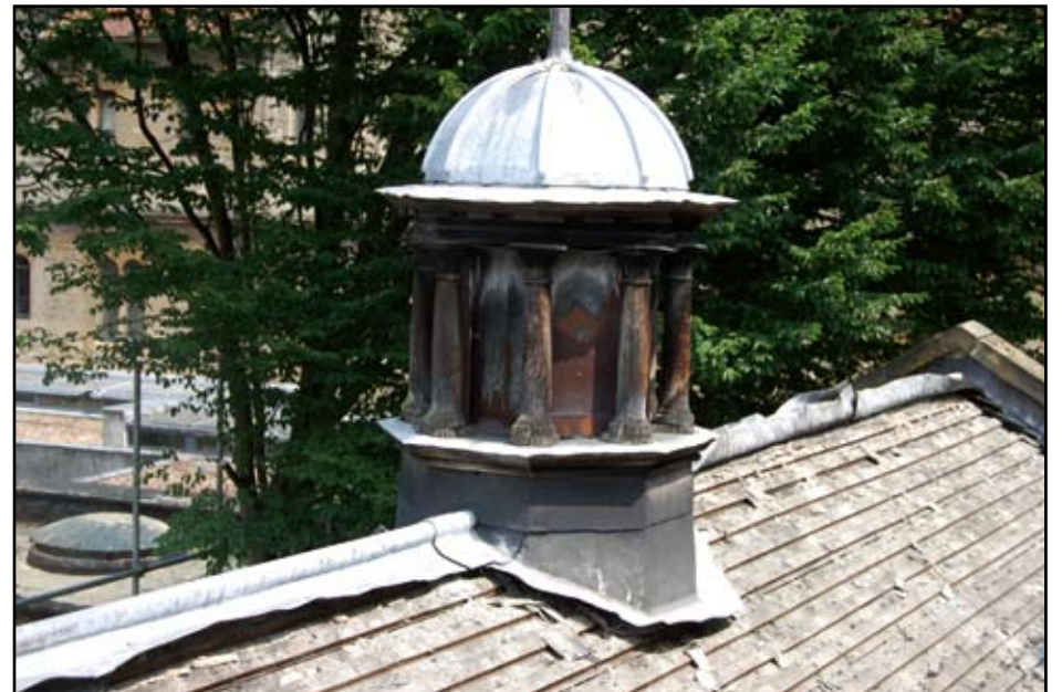
Plate 16: Cupola on former lecture room
