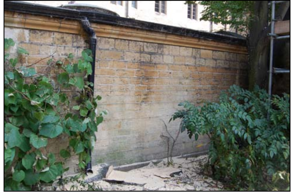
Plate 22: Wall of corridor along east side of Fellows' Garden
