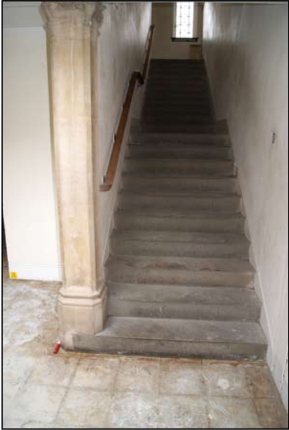
Plate 61: Stairs between main building and former lecture room
