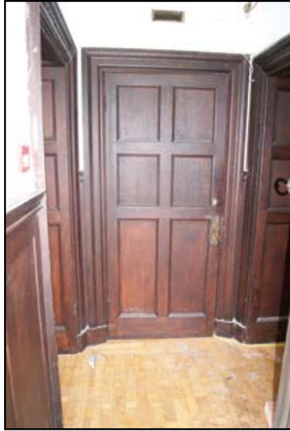
Plate 25: Typical 6-panel door in entrance lobby
