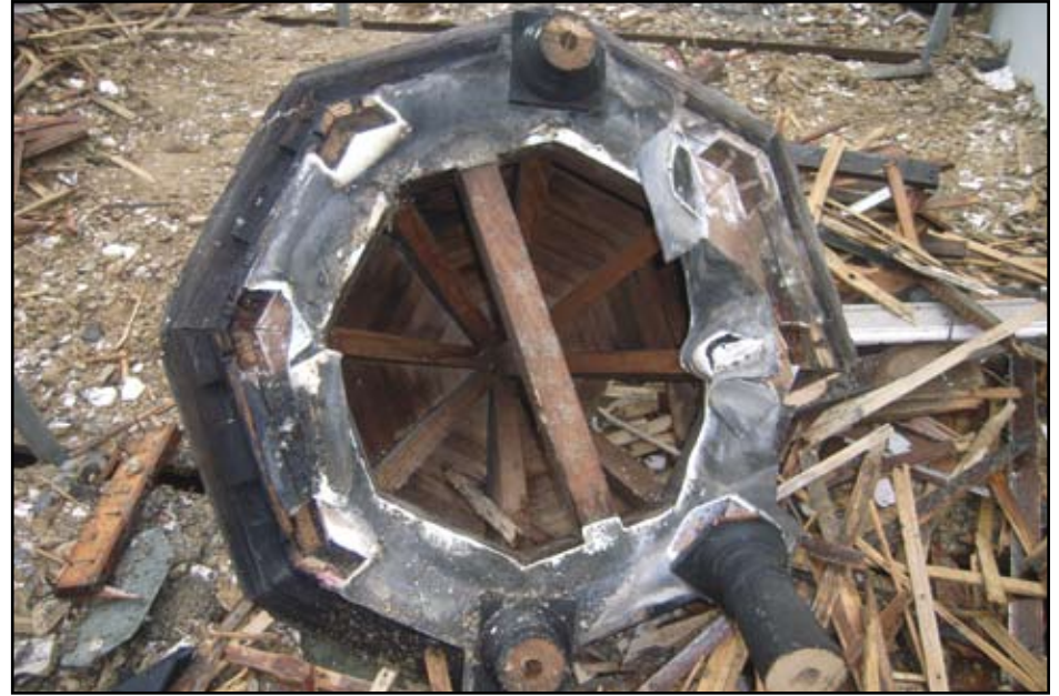
Plate 18: Part of ex-situ cupola during demolition
