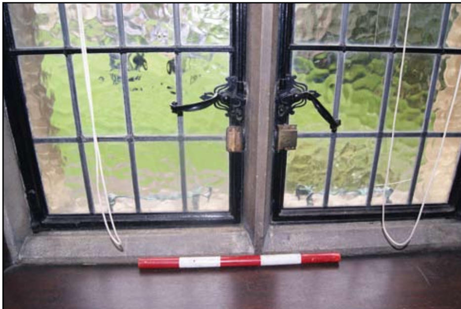
Plate 35: Window detail in former lecture room
