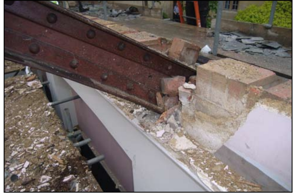
Plate 50: Eaves detail of roof in former lecture room
