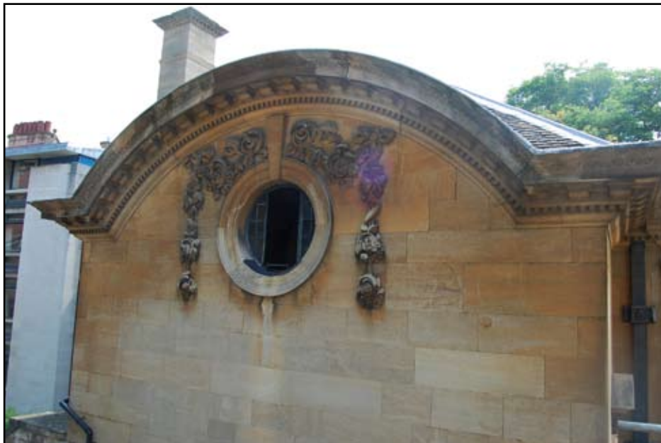
Plate 3: North face of main Garden Building
