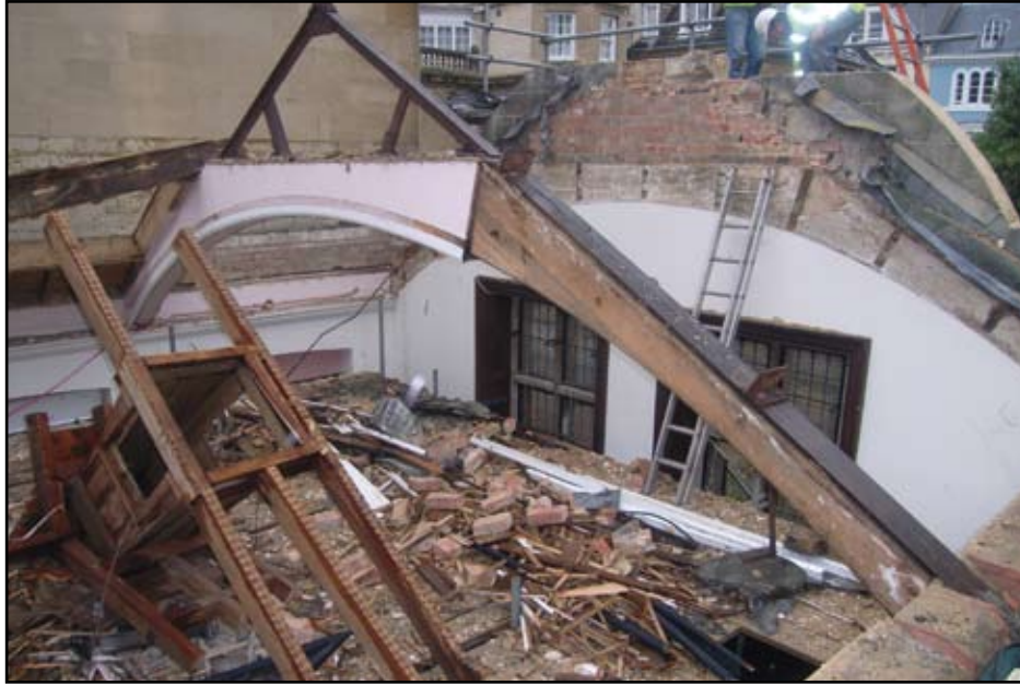
Plate 49: Roof of former lecture room during dismantling
