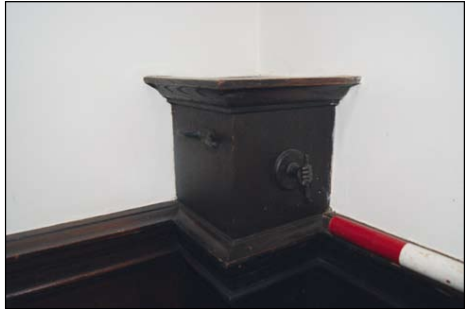
Plate 42: Vent detail in former lecture room
