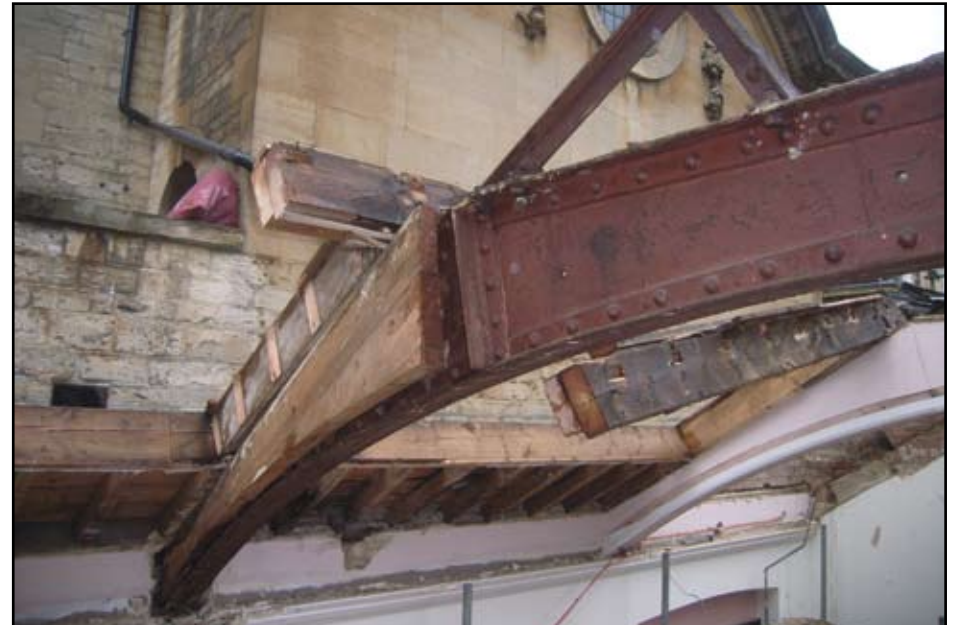
Plate 52: Truss in former lecture room
