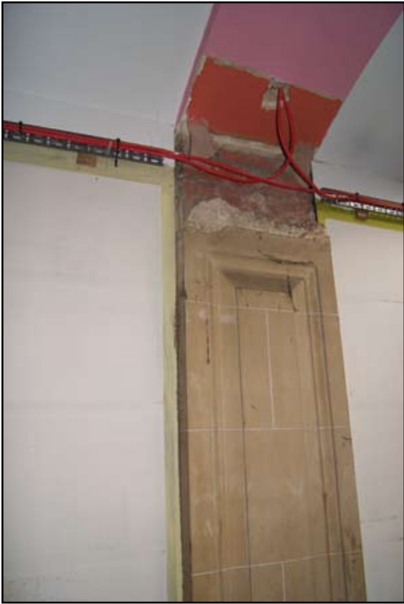
Plate 65: Pilaster detail in corridor to east of Fellows' Garden
