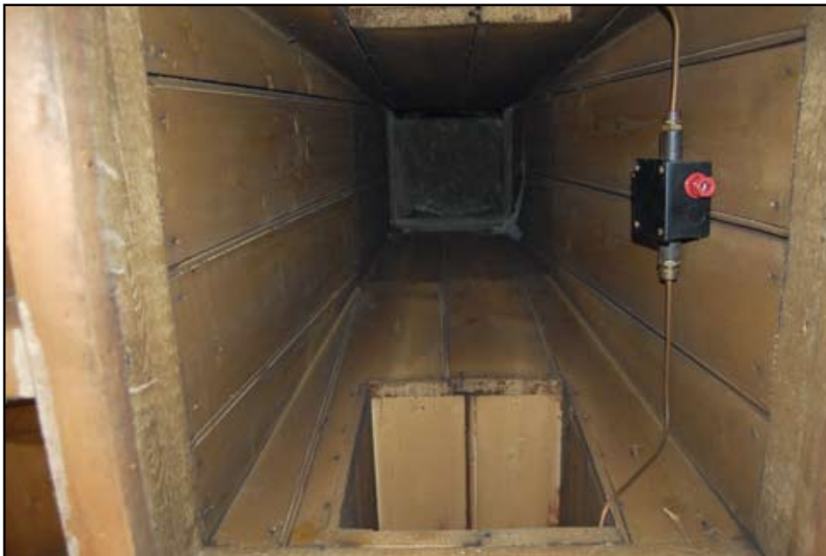
Plate 47: Vertical duct rising to cupola
