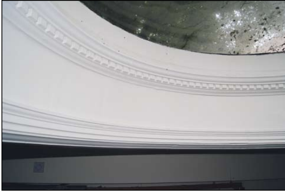
Plate 57: Detail of roof light by foot of stairs
