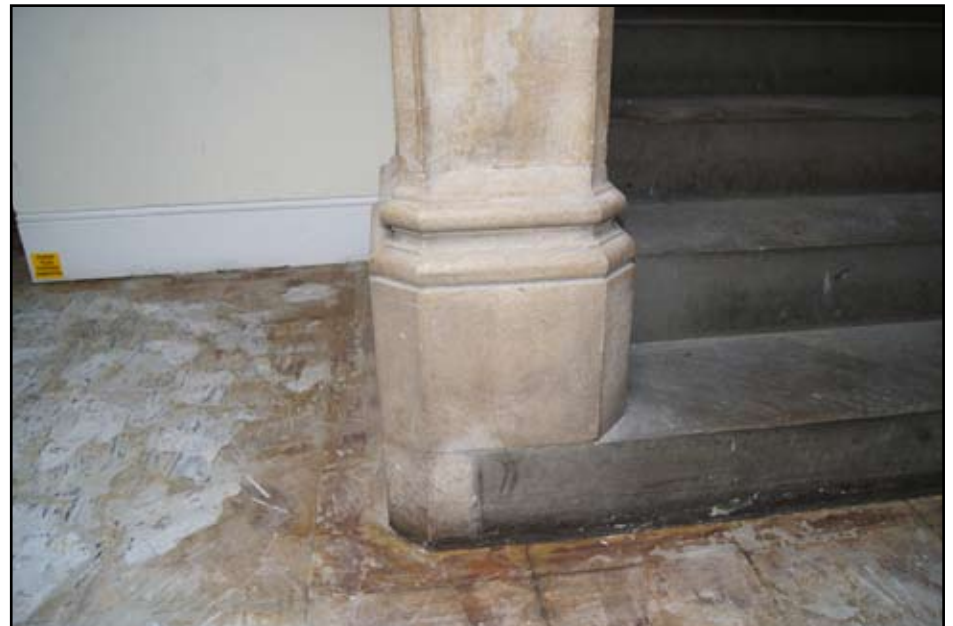
Plate 60: Column base by stairs
