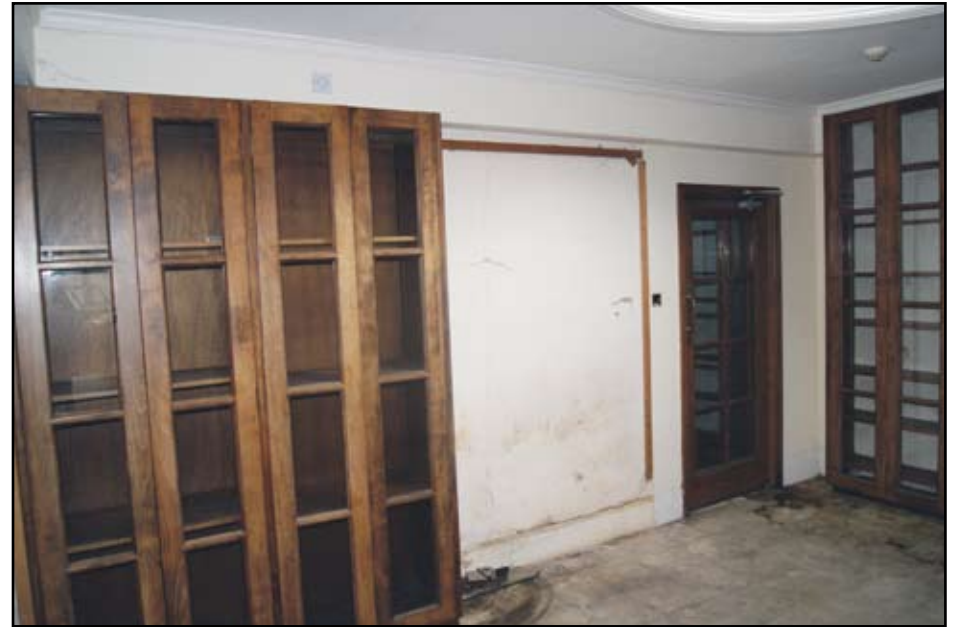
Plate 54: Lobby to east of former lecture room
