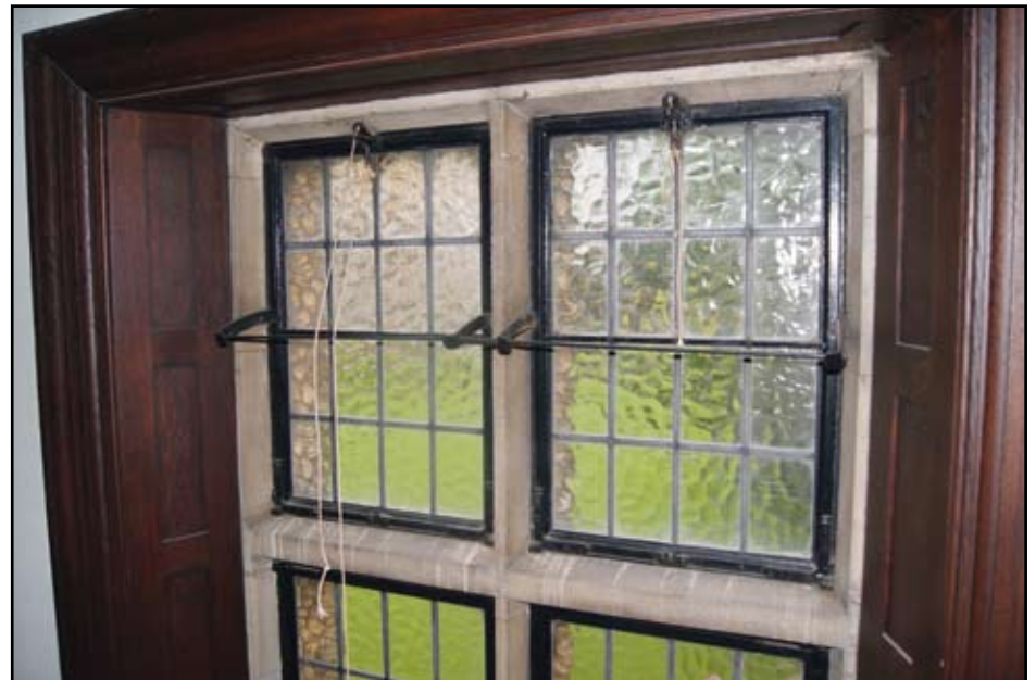
Plate 36: Window detail in former lecture room
