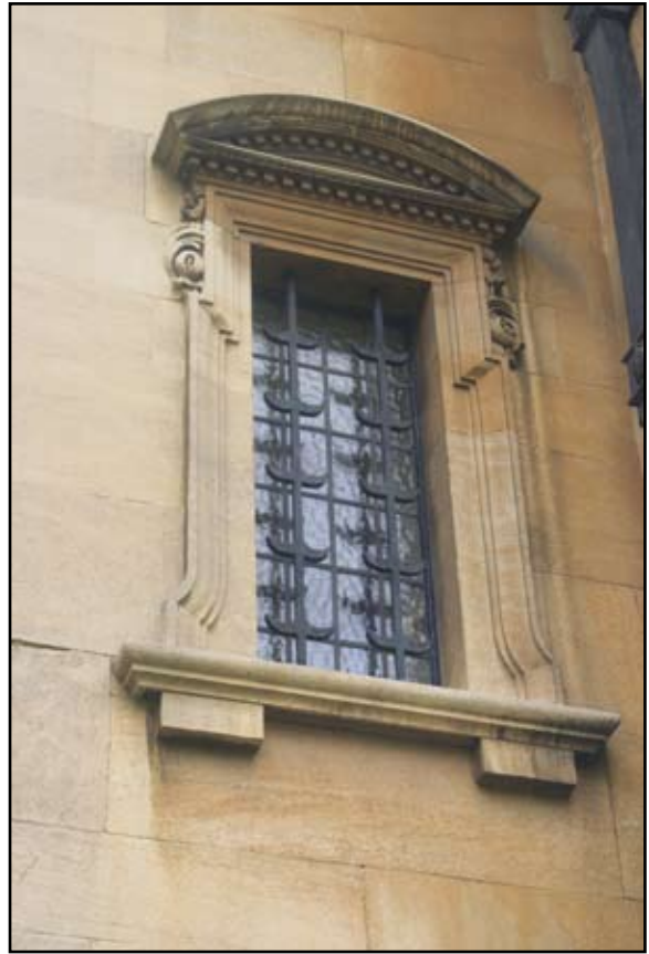
Plate 6: First floor window in west wall
