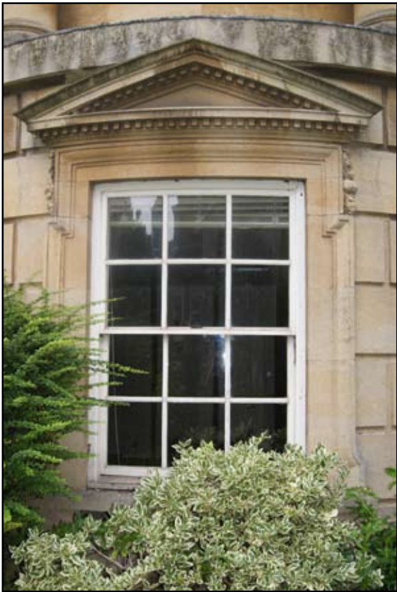
Plate 7: Replaced ground floor window in west wall
