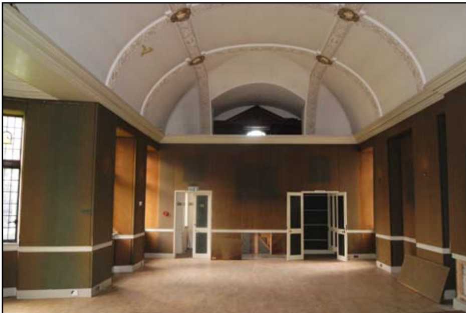
Plate 31: First floor of main building (Oakeshott Room)
