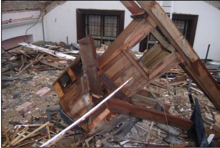
Plate 17: Ex-situ cupola structure during demolition
