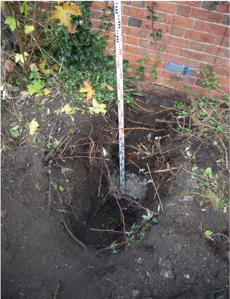
Plate 8: Test pit for engineer at north end of Trench 3 showing chalk foundation of the south wall of Provost Cells.
