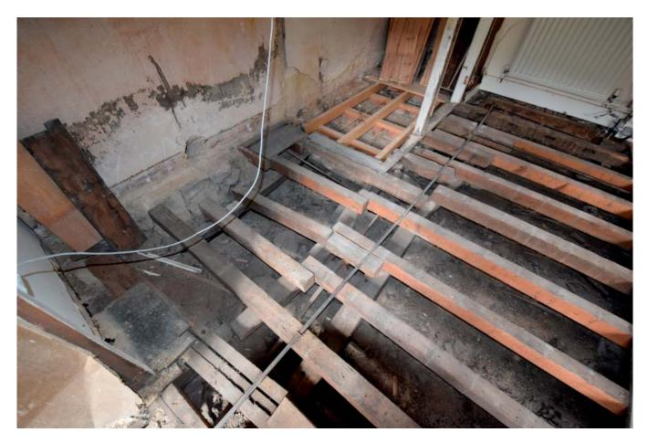
Plate 14: Exposed section of joists
