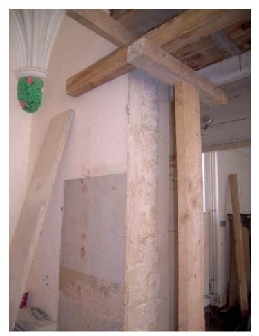
Plate 37: Opening created in wall between passage and Events Office
