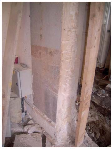
Plate 36: Opening created in wall between passage and Events Office
