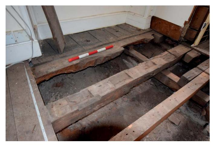
Plate 12: Former wall plate reused with trenches to top
