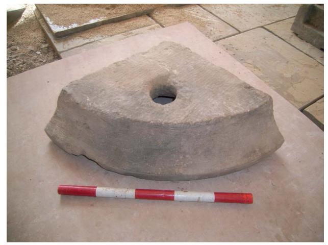
Plate 50: Underside of reused drainage hopper found in wall
