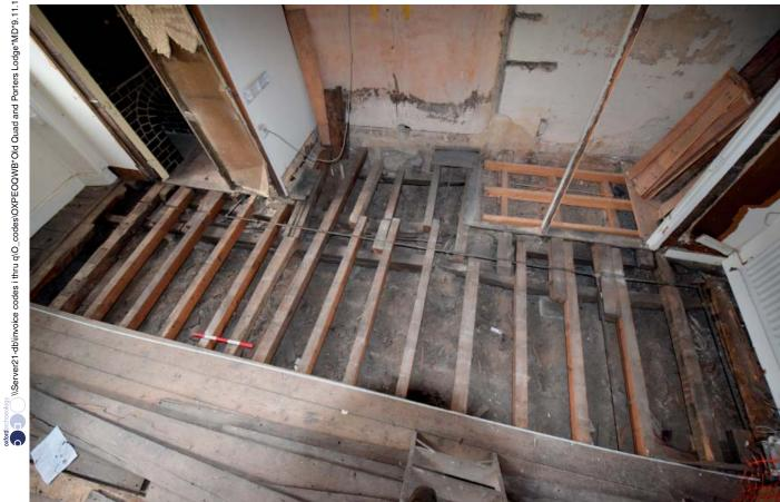
Plate 11: Exposed joists in Events Office
