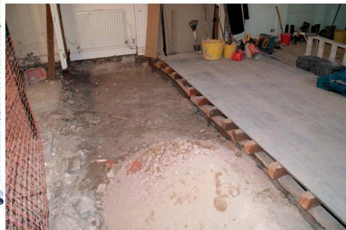
Plate 25: Area of removed joists in Events Office
