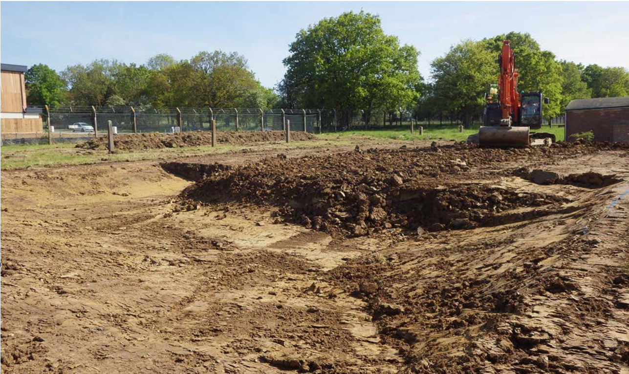
Plate 1: Pond B under construction
