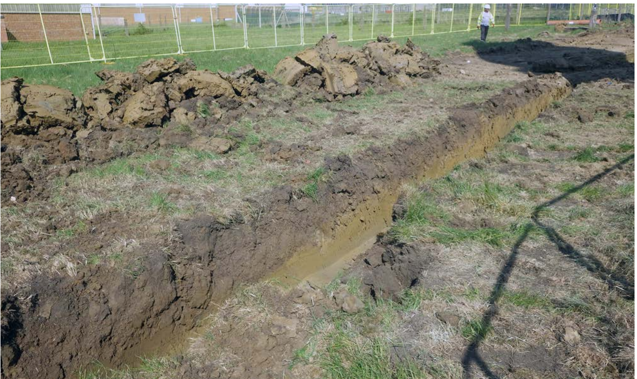
Plate 4: Pond B drainage pipe trench
