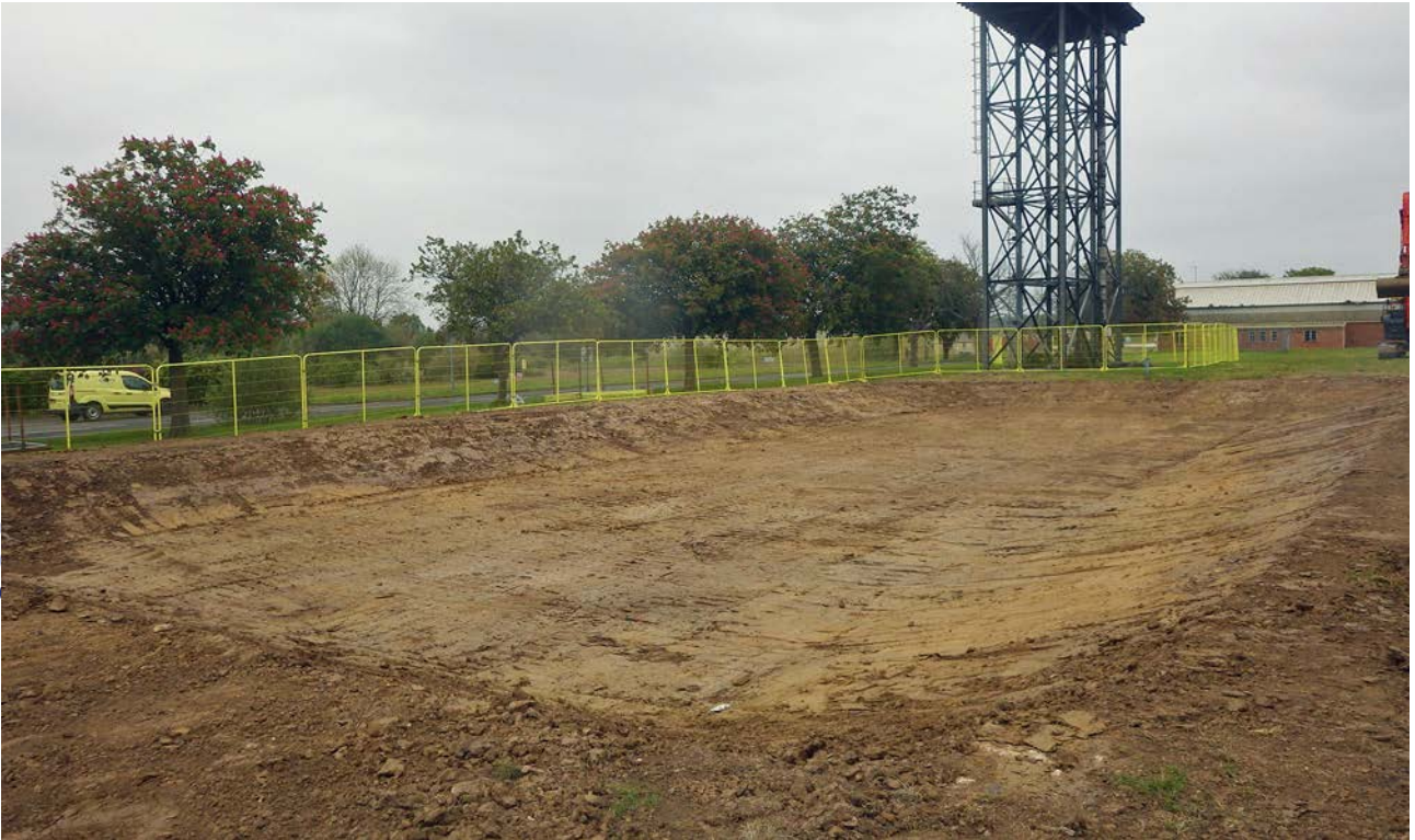
Plate 3: Pond B following excavation
