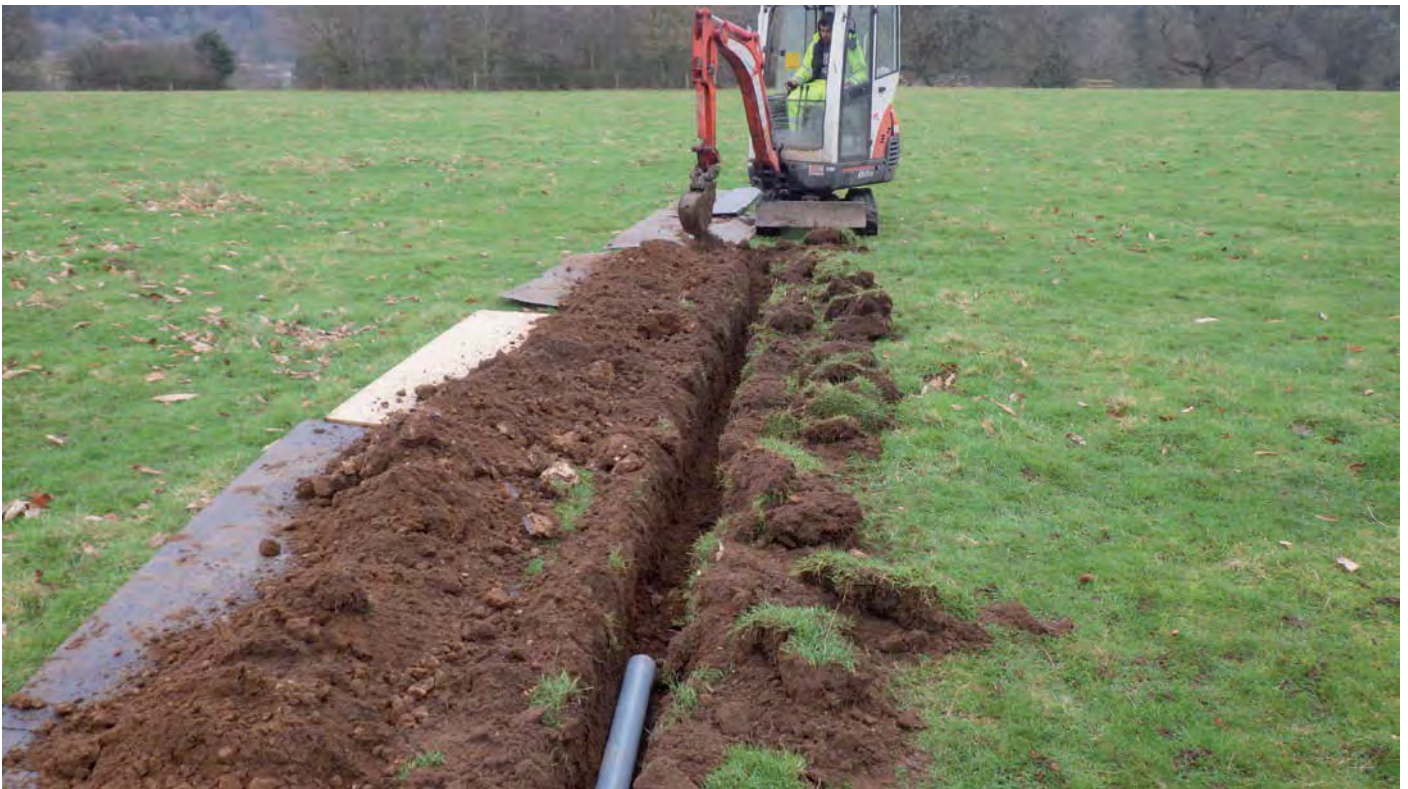
Plate 2 Excavation trench through sub-soil, looking east
