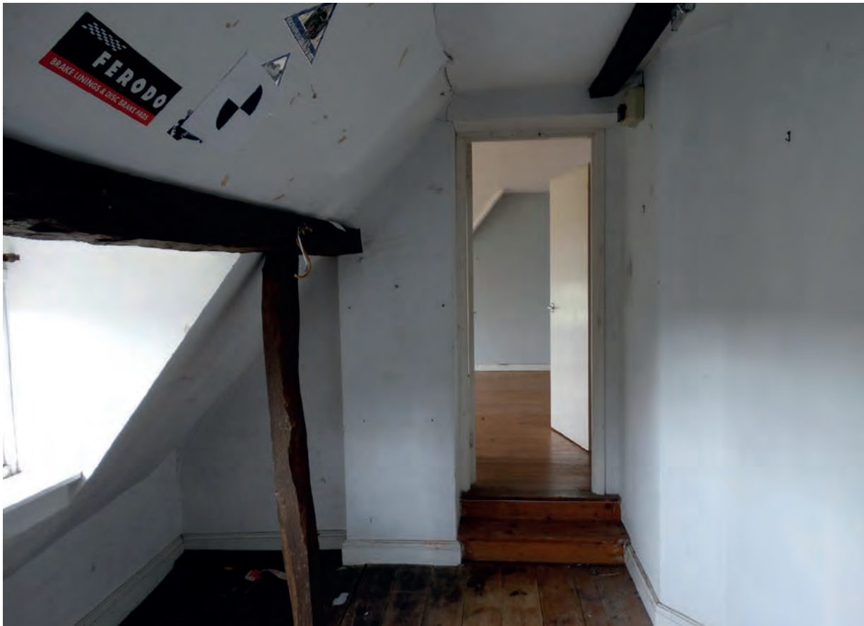
Plate 96: The dressing room, looking north
