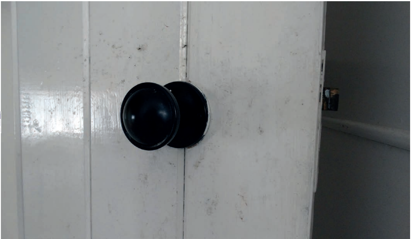
Plate 86: The door knob of bathroom 1
