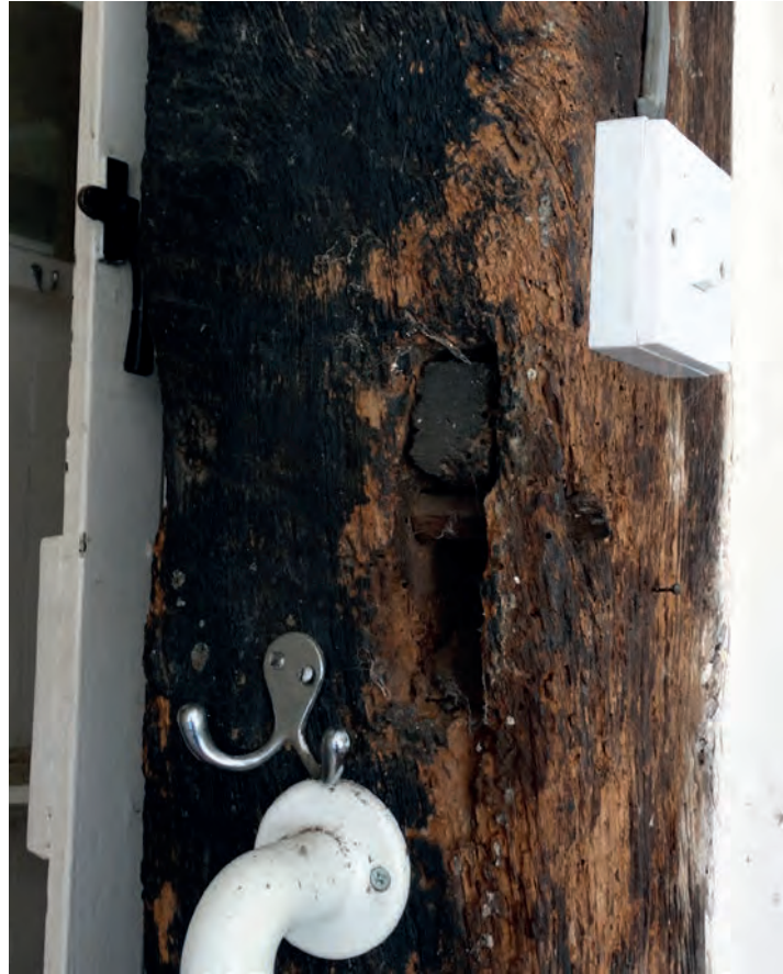
Plate 48: The redundant mortice in the post
