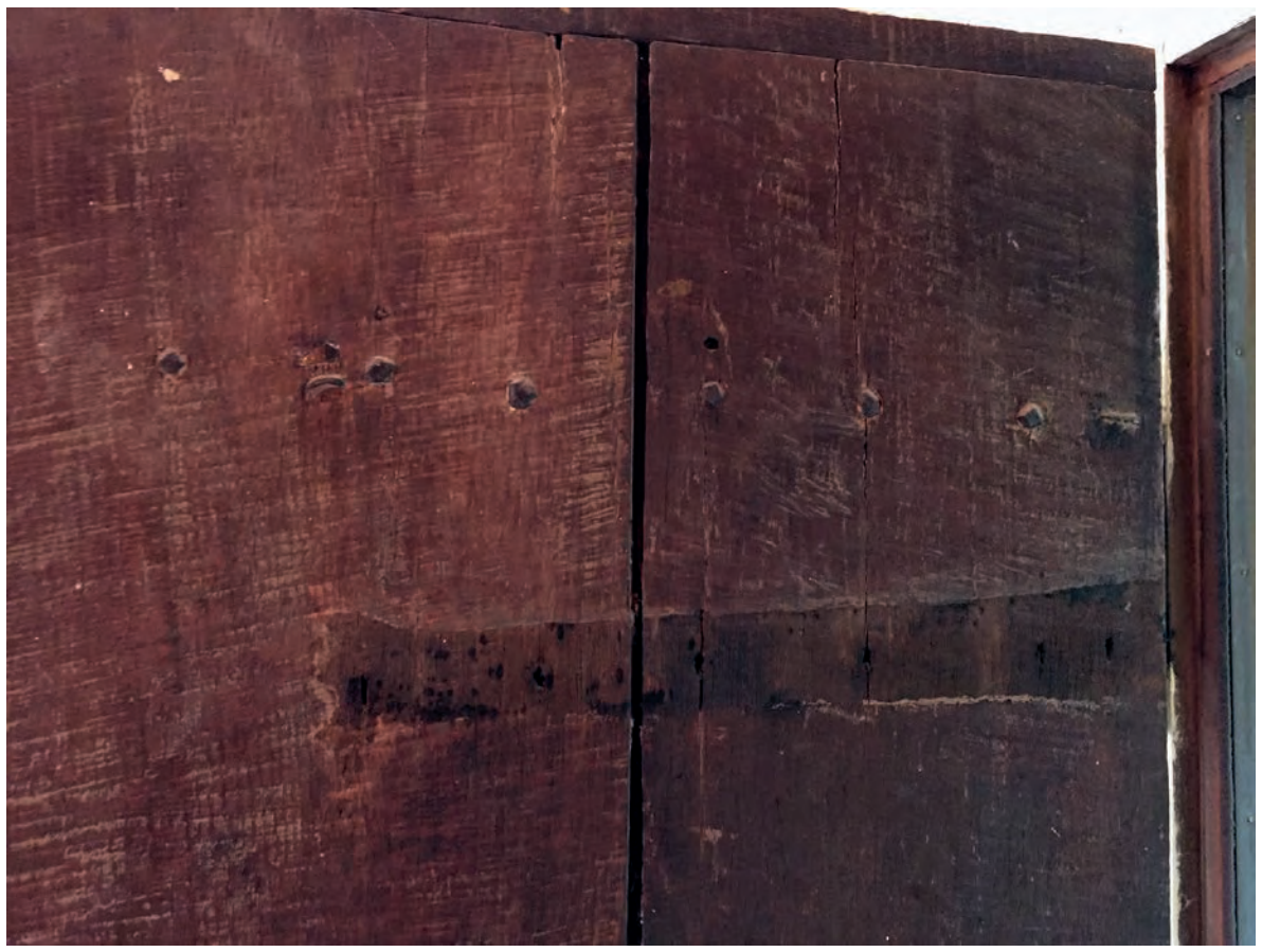
Plate 126: The scar of the early strap hinge
