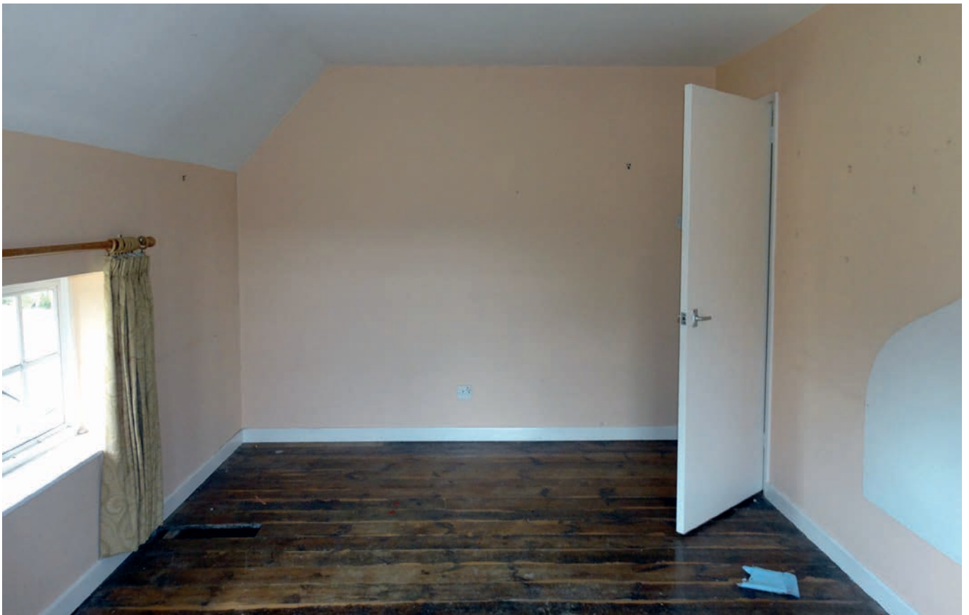
Plate 99: The south wall of bedroom 2
