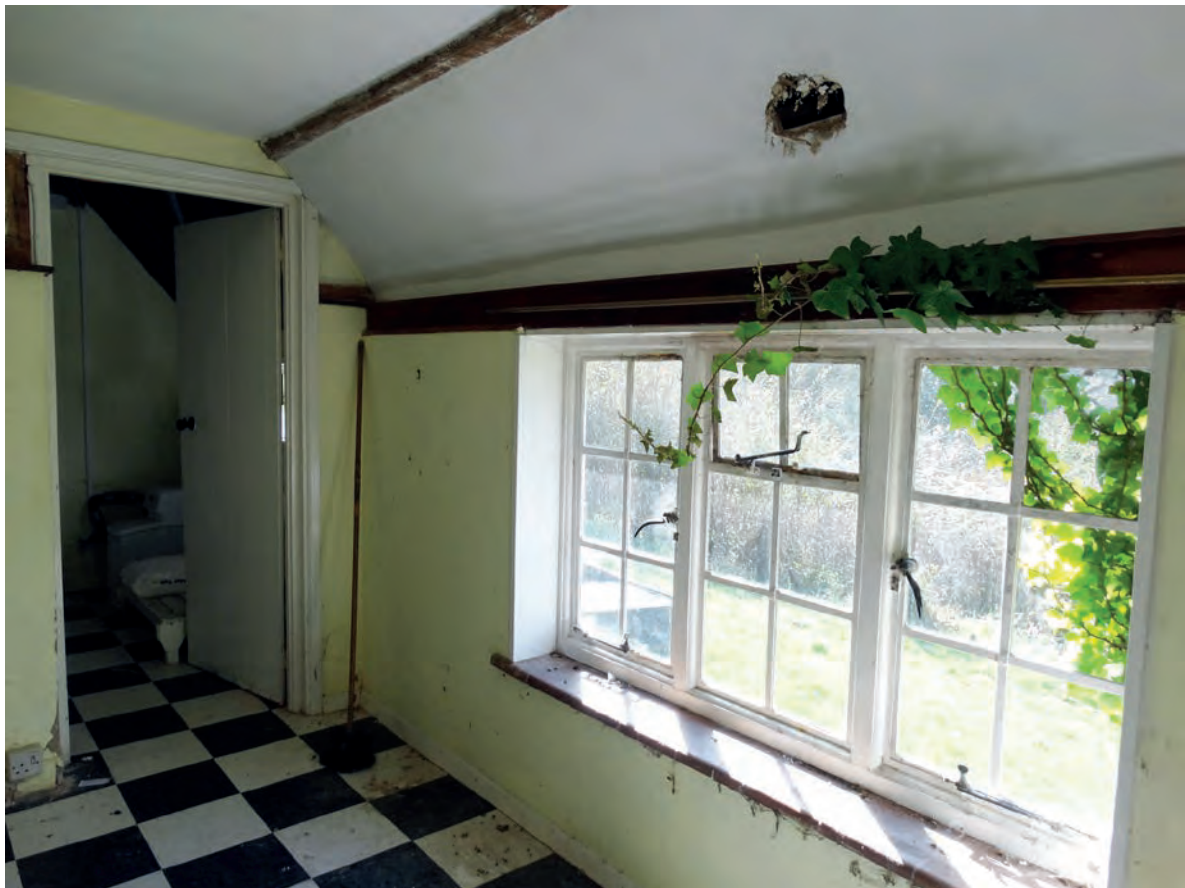
Plate 80: The west wall of the utility room
