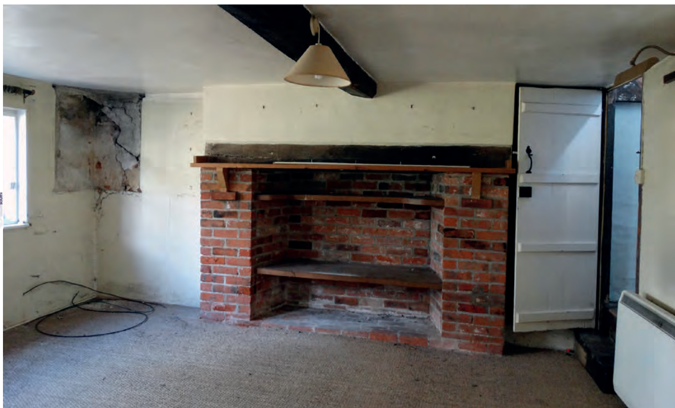
Plate 67: The south wall of sitting room 2
