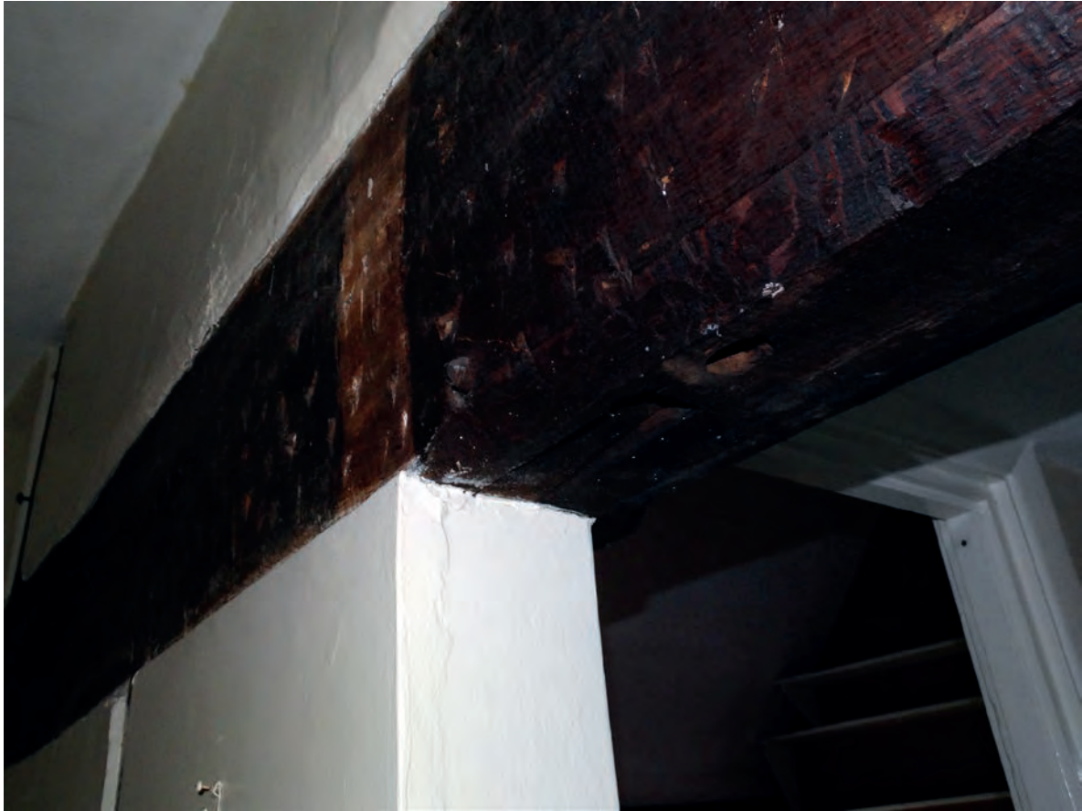
Plate 103: The redundant mortice and stave hole in the doorway between corridors 1 and 2
