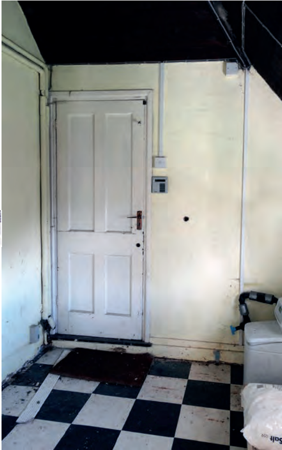
Plate 83: The south wall of lobby 2
