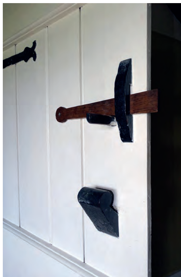
Plate 54: The door furniture to the sitting room 1 side of the door to lobby 1
