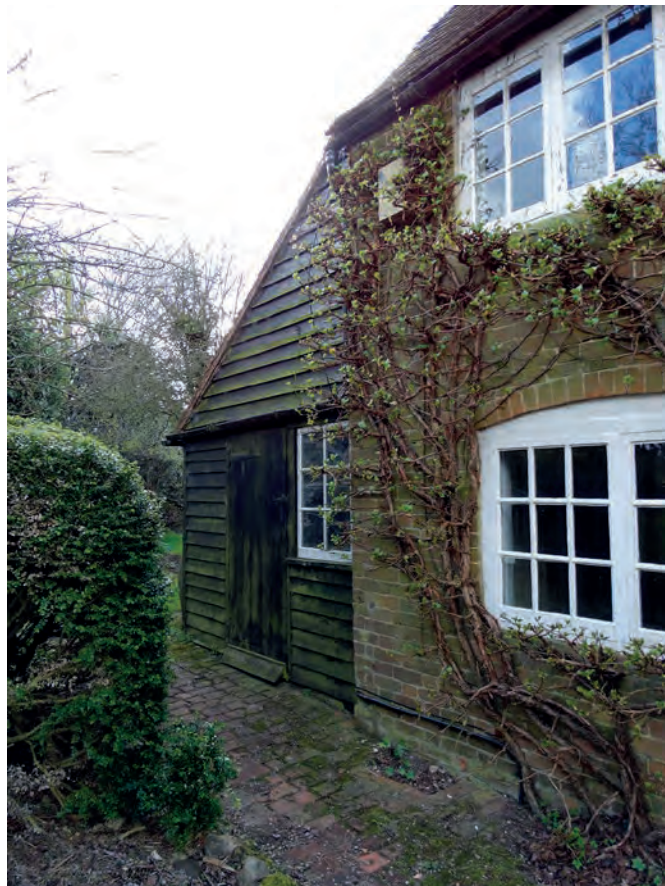
Plate 9: The timber-clad lean-to to the south elevation
