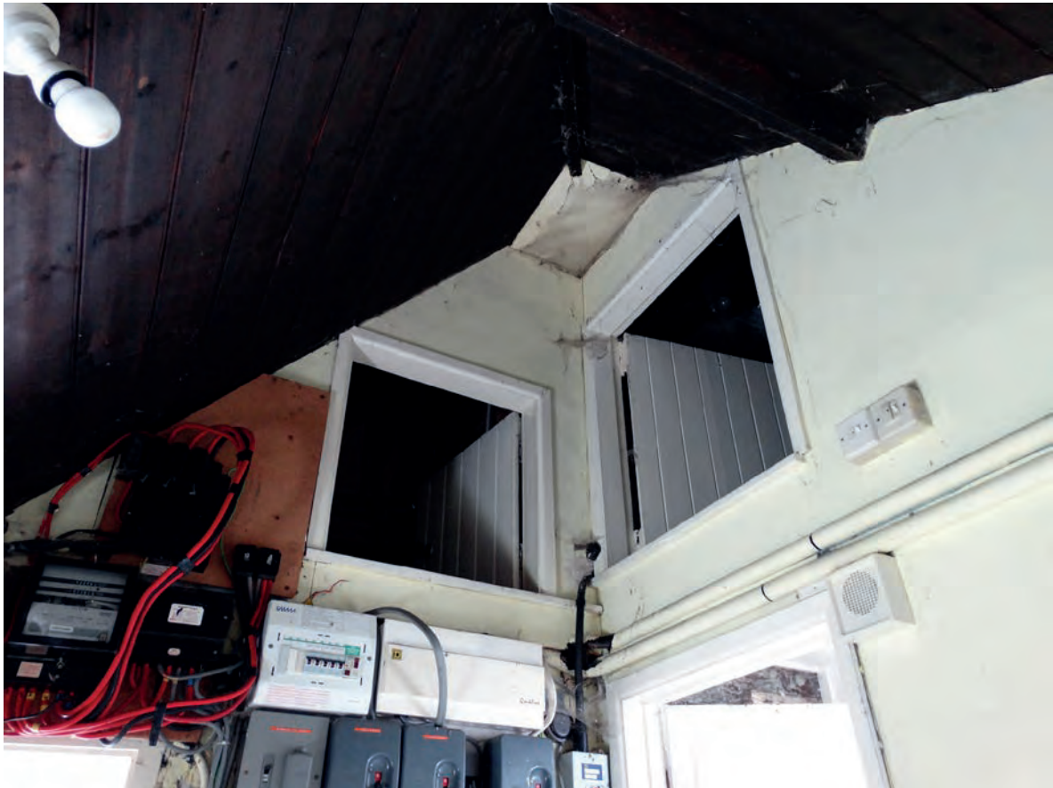
Plate 82: The access hatches in lobby 2
