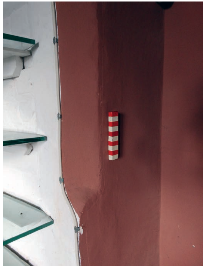
Plate 118: The chamfer of the fireplace in bedroom 4
