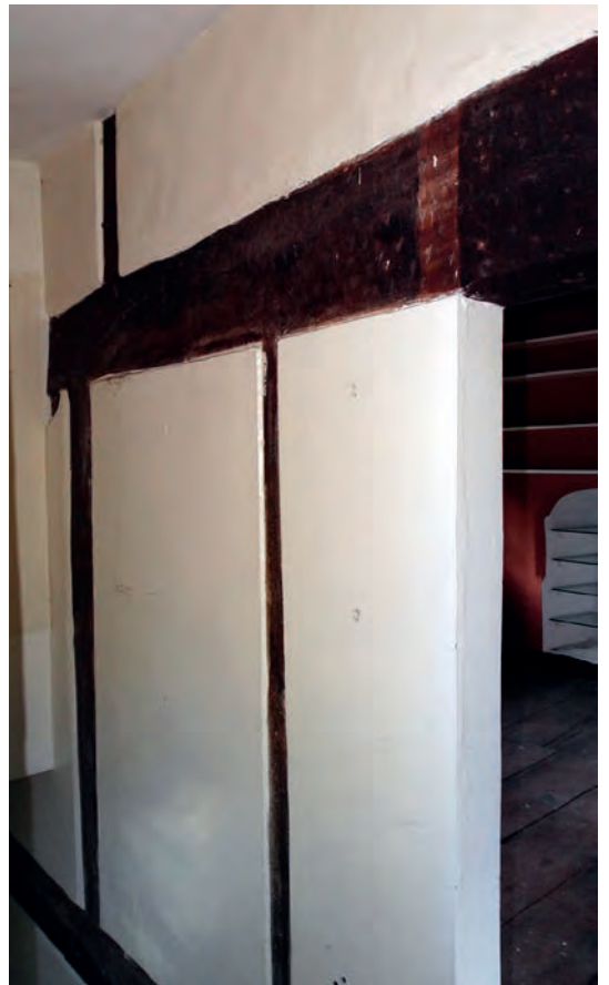
Plate 101: The timber frame above the modern staircase
