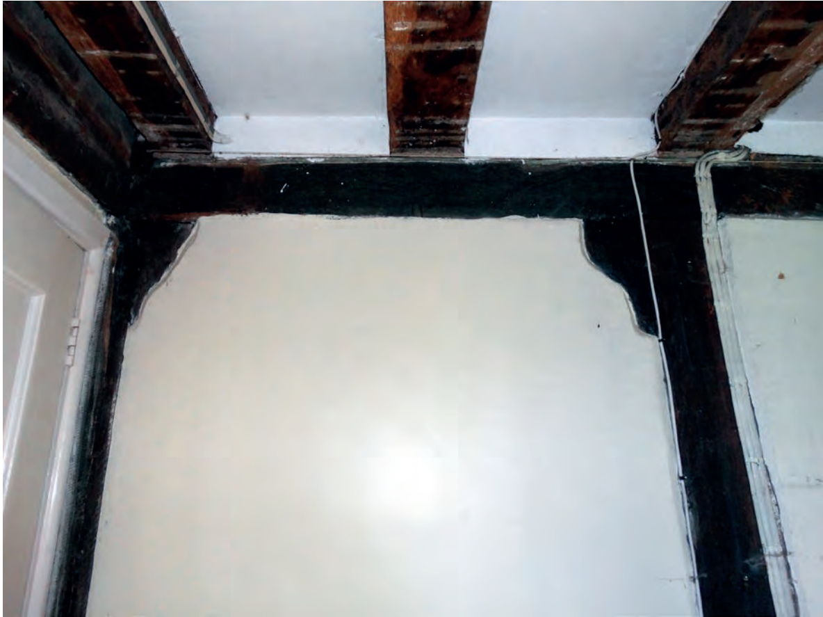
Plate 26: The blocked doorway in the west wall of the entrance hall
