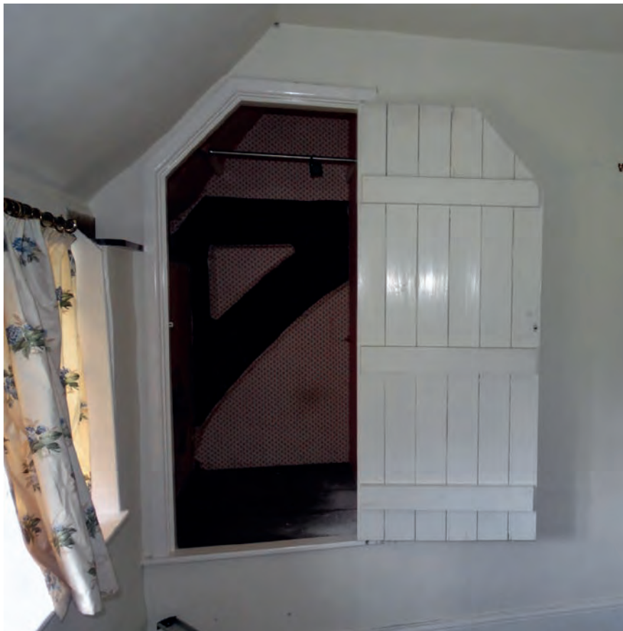
Plate 106: The south wall of bedroom 3
