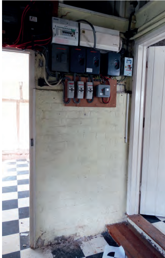
Plate 81: The north wall of lobby 2
