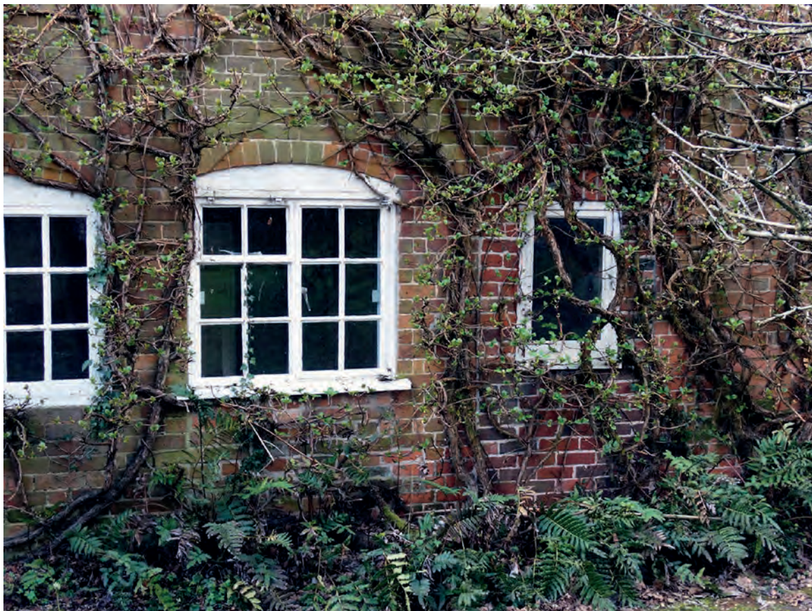
Plate 12: The two partially blocked openings in the east elevation
