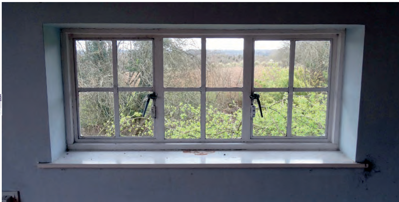
Plate 94: The window in the north wall of bedroom 1
