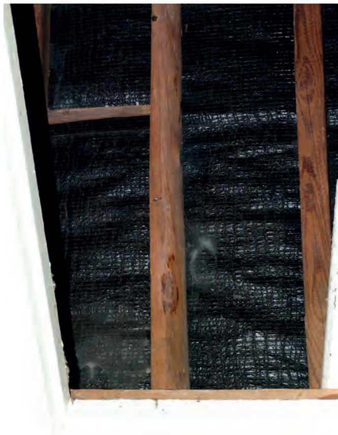
Plate 7: The modern sarking felt to the roof above the Study
