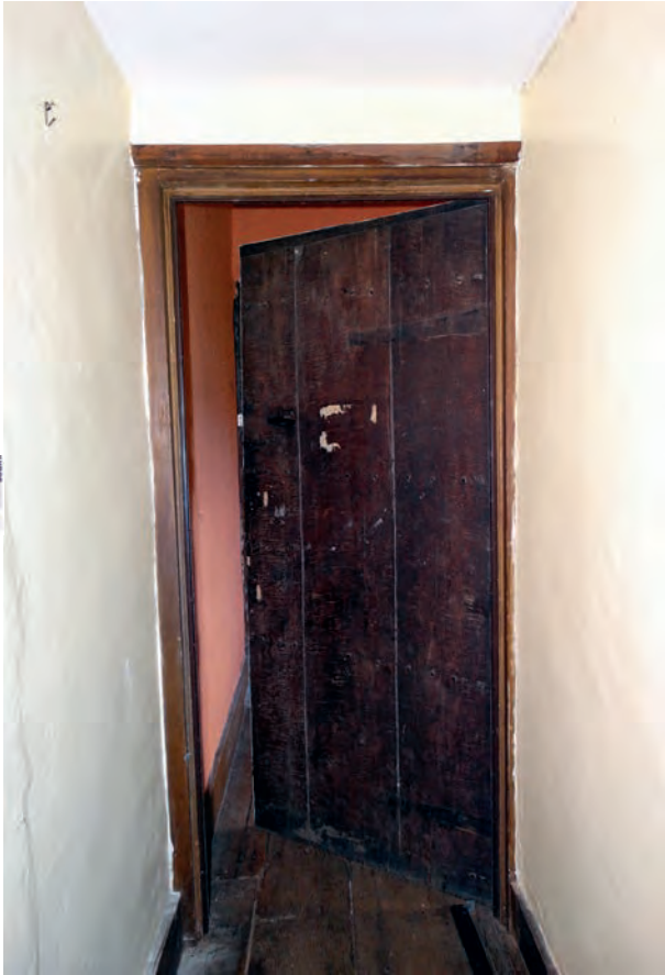
Plate 125: The early door between corridor 2 and bedroom 5
