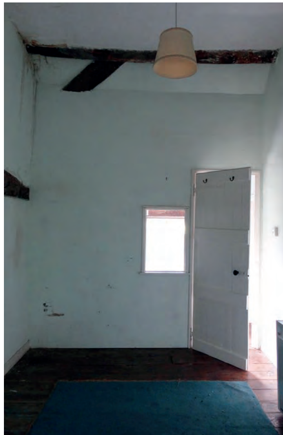
Plate 138: The west wall of bedroom 6
