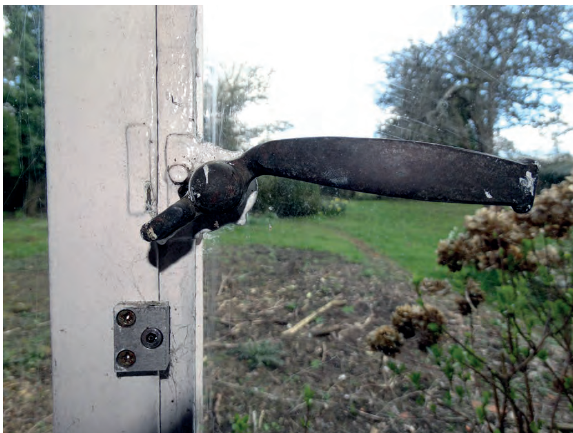
Plate 33: An example of one style of gun metal handle
