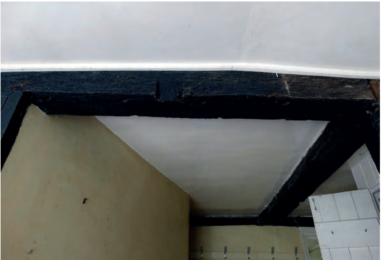
Plate 49: The stave holes above the doorway between the kitchen lobby 1
