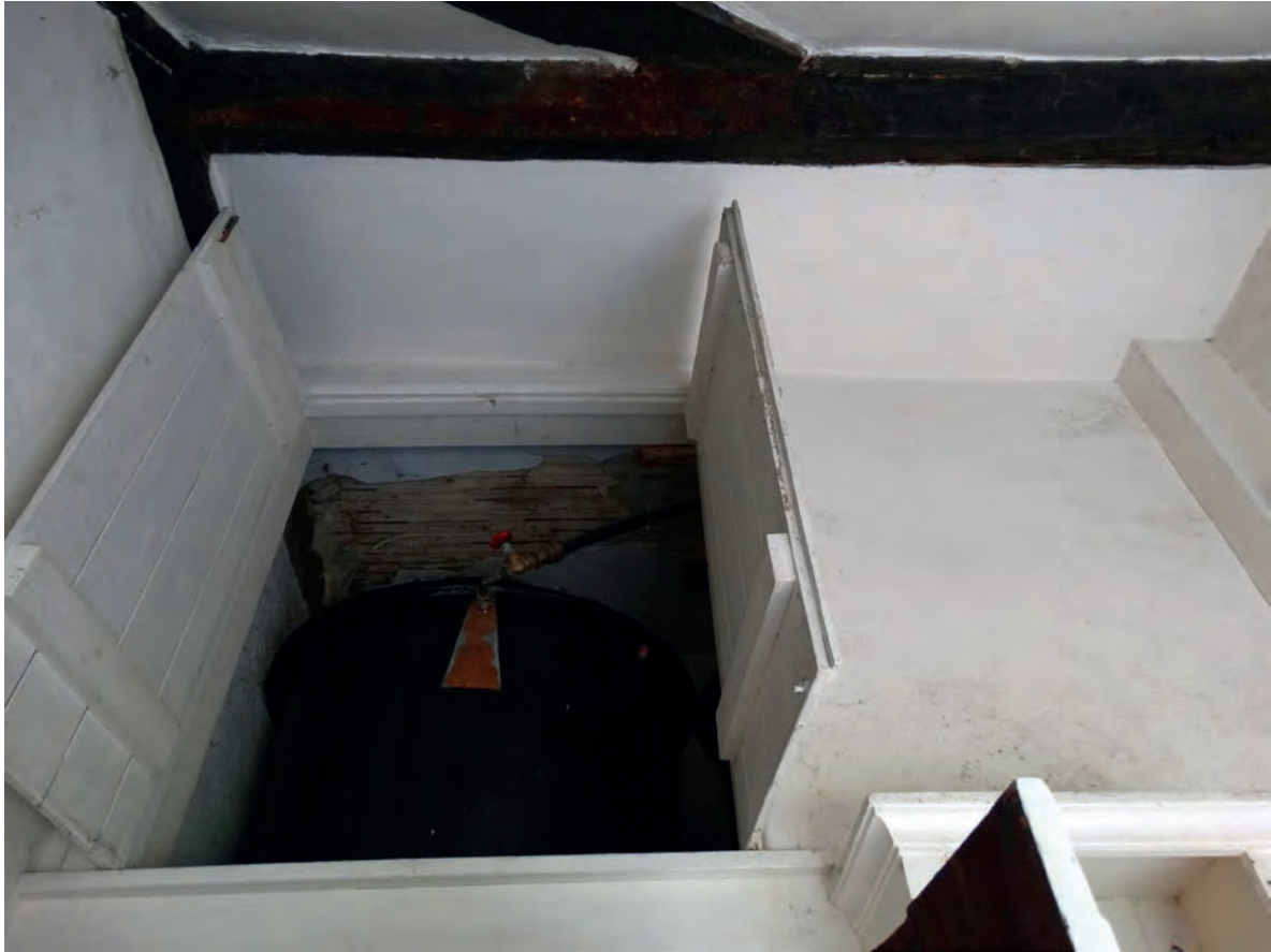
Plate 112: The water tank cupboard and visible timbers in bathroom 2
