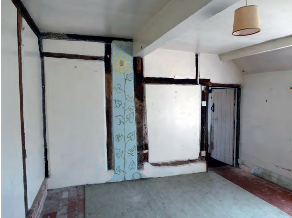
Plate 40: The south wall in the dining room
