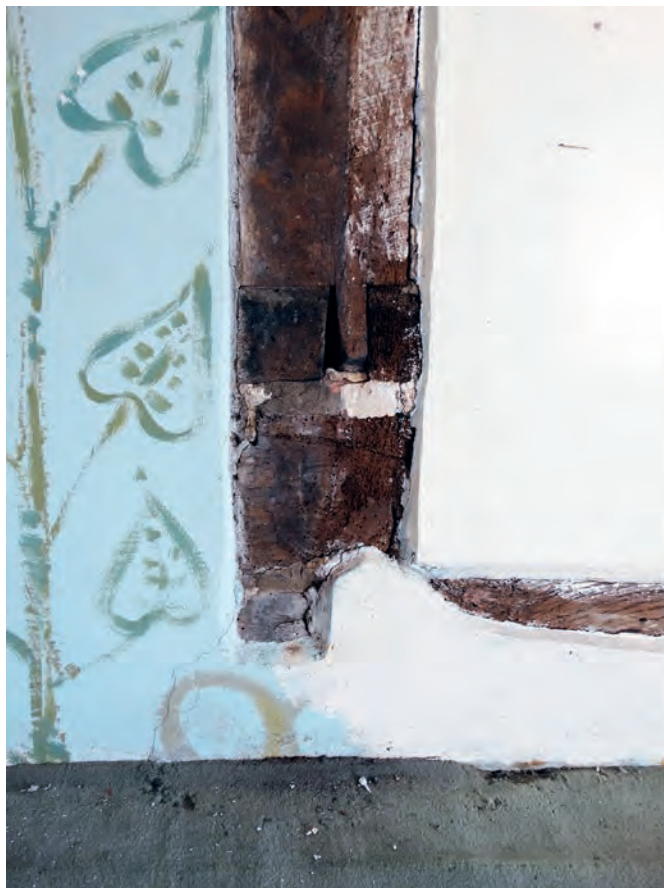
Plate 42: The cut timbers in the south wall
