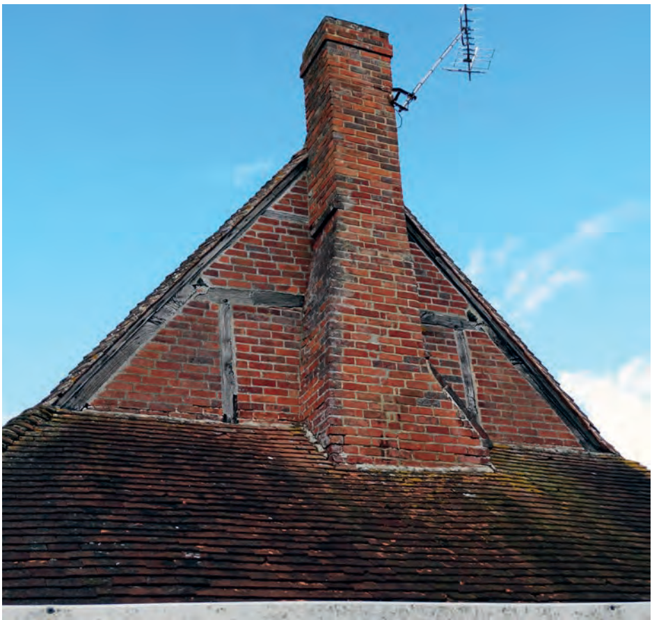
Plate 18: The timber frame visible in the south elevation
