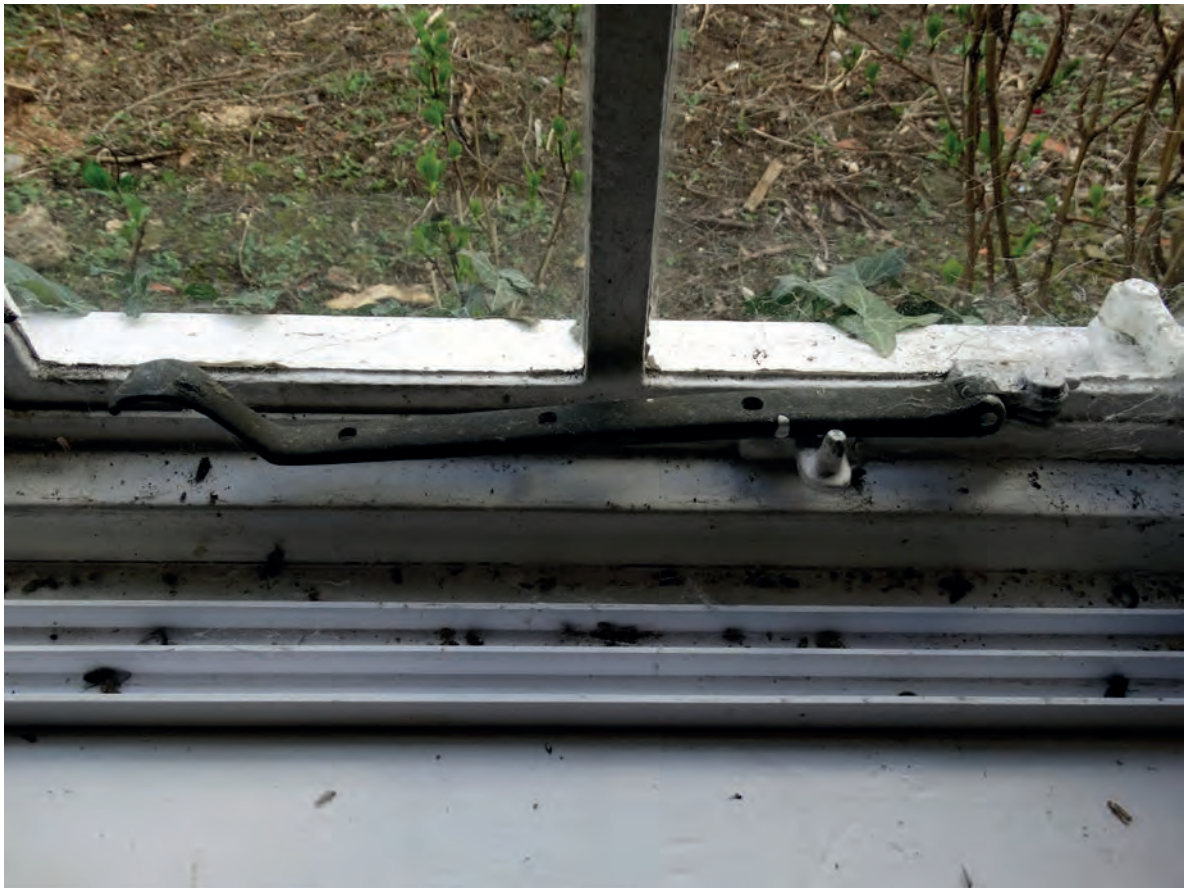
Plate 34: An example of a gun metal peg stay
