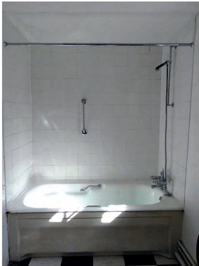
Plate 85: The south wall of bathroom 1
