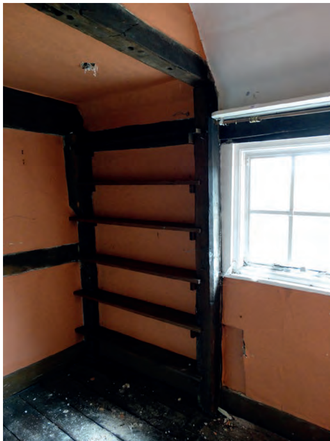
Plate 119: The west wall of bedroom 5
