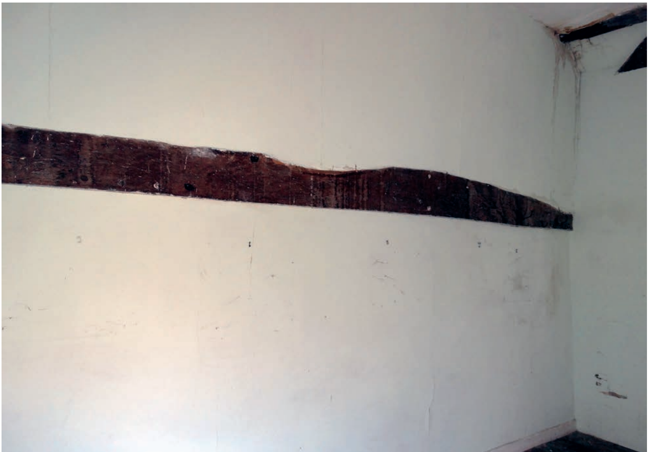
Plate 143: The substantial, but irregularly shaped, southernmost tie beam
