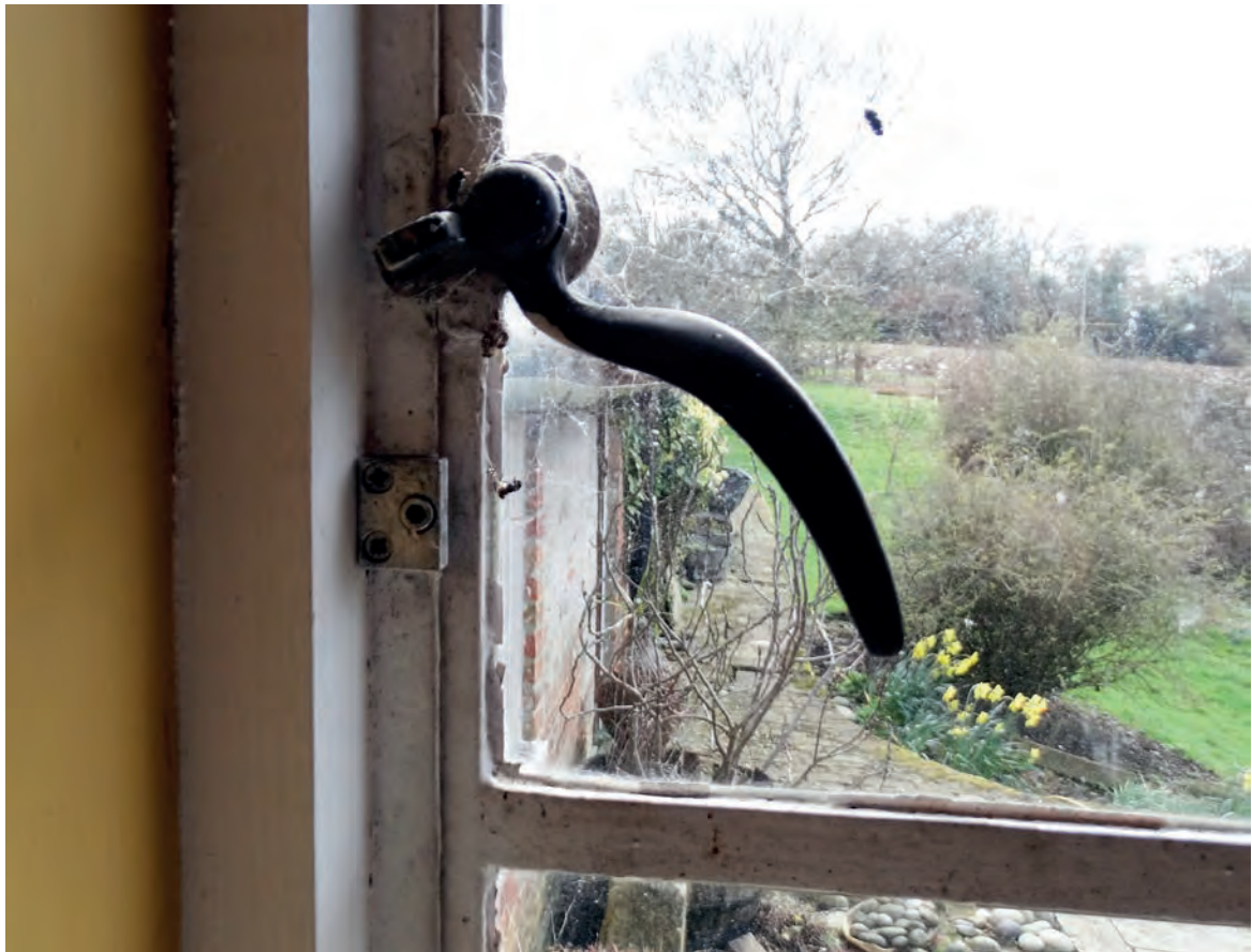
Plate 36: An example of one style of gun metal handle
