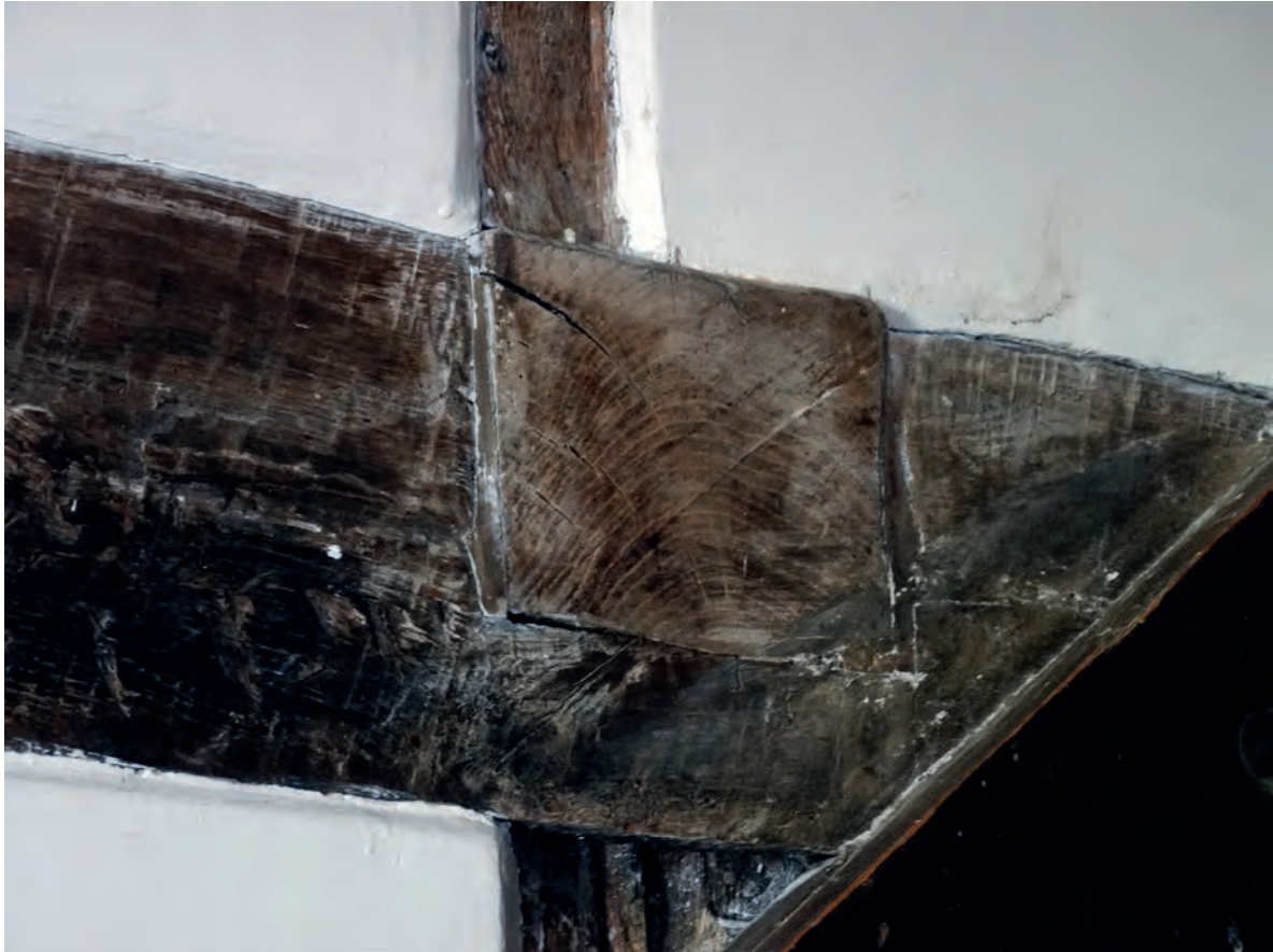
Plate 22: The beam cut to allow installation of the staircase
