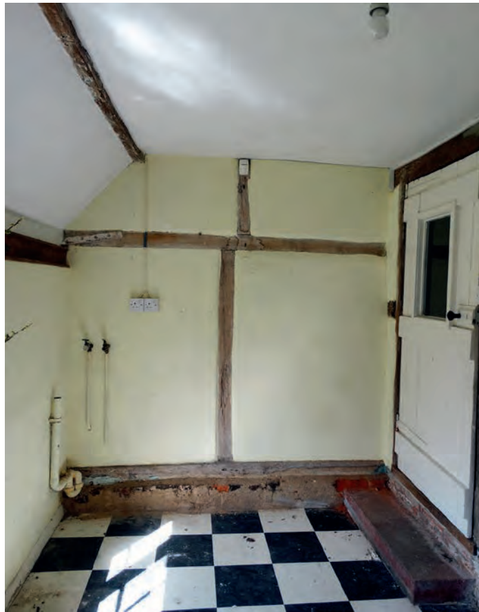
Plate 79: The north wall of the utility room
