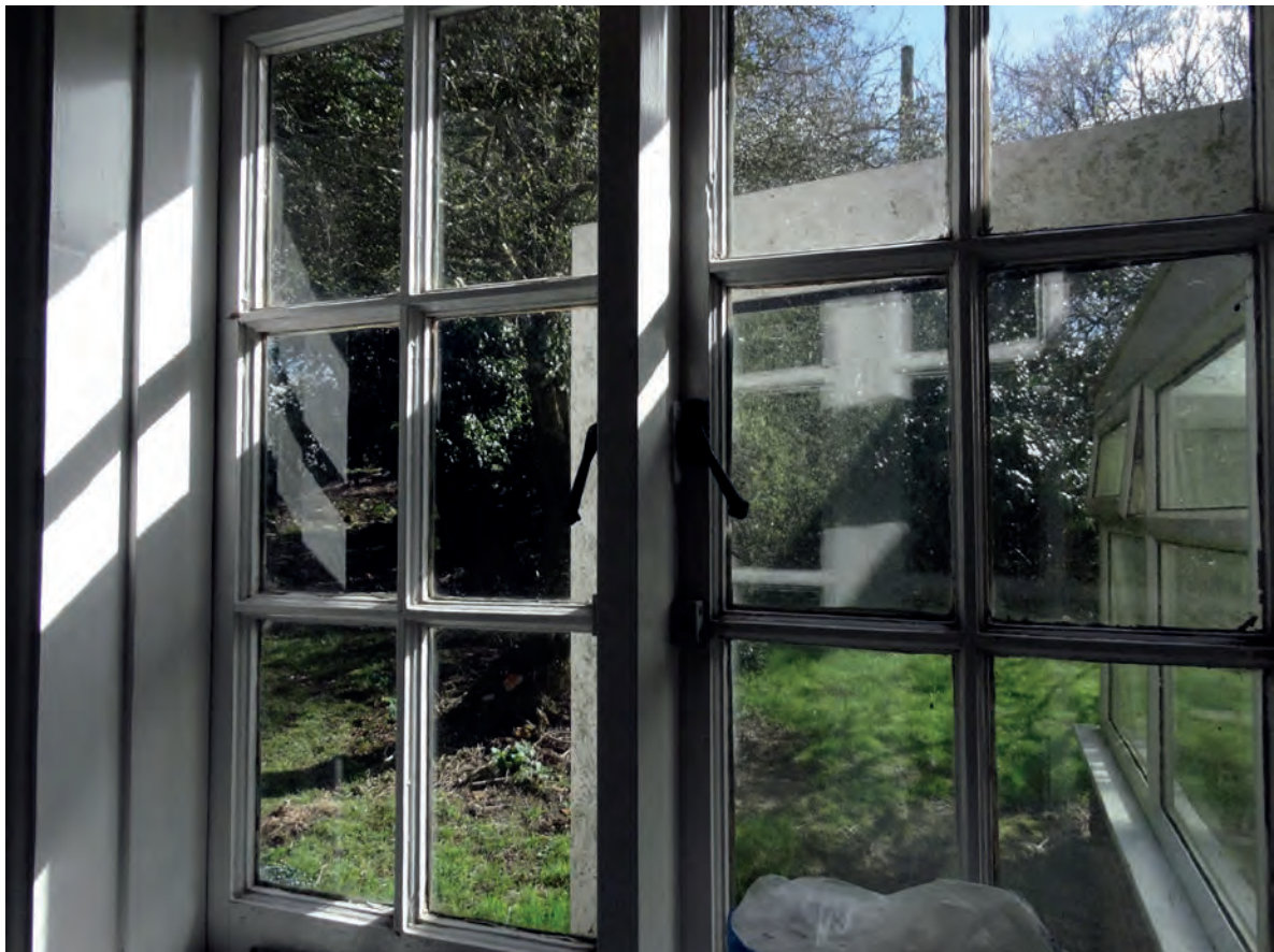
Plate 87: The window in bathroom 1
