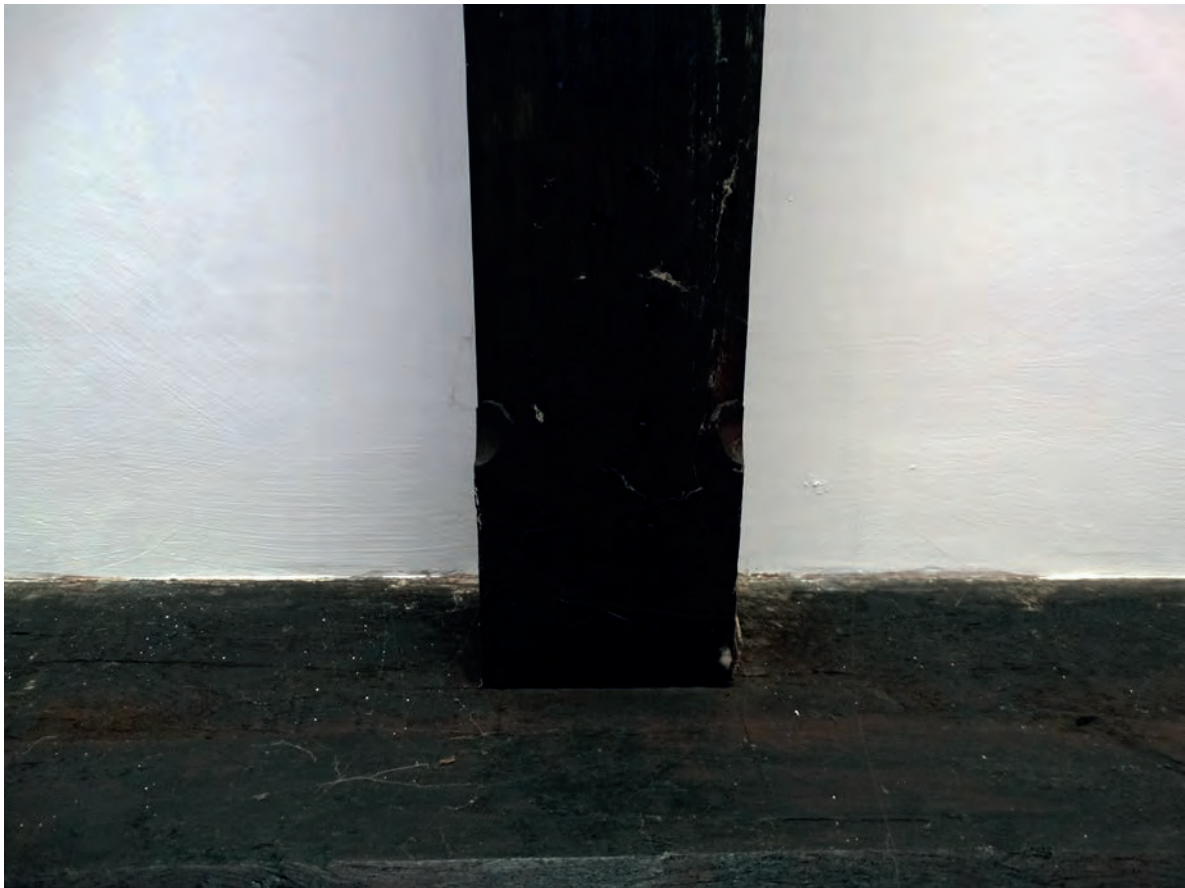
Plate 61: An example of a chamfered and stopped joist in sitting room 1
