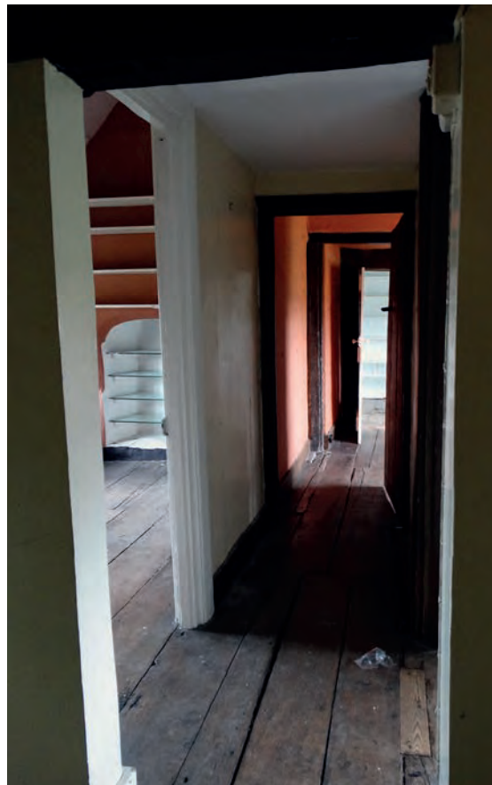
Plate 113: Corridor 2, looking south
