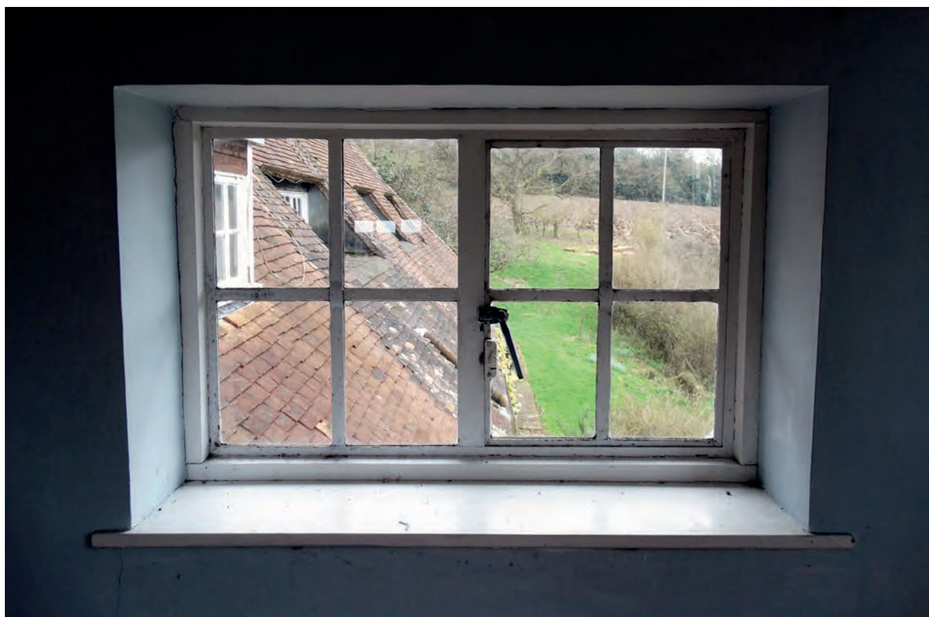
Plate 93: The window in the south wall of bedroom 1
