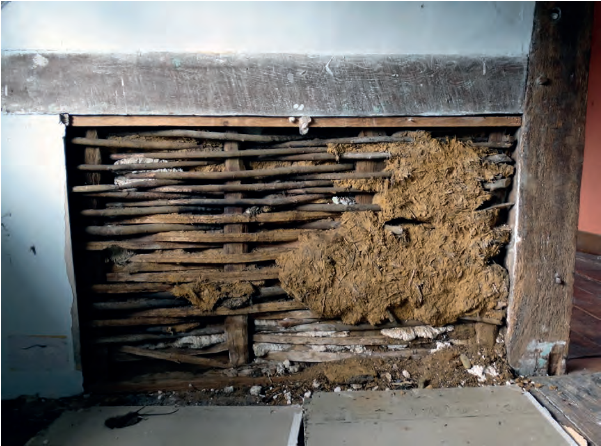
Plate 137: The wattle and daub panel behind modern plaster board
