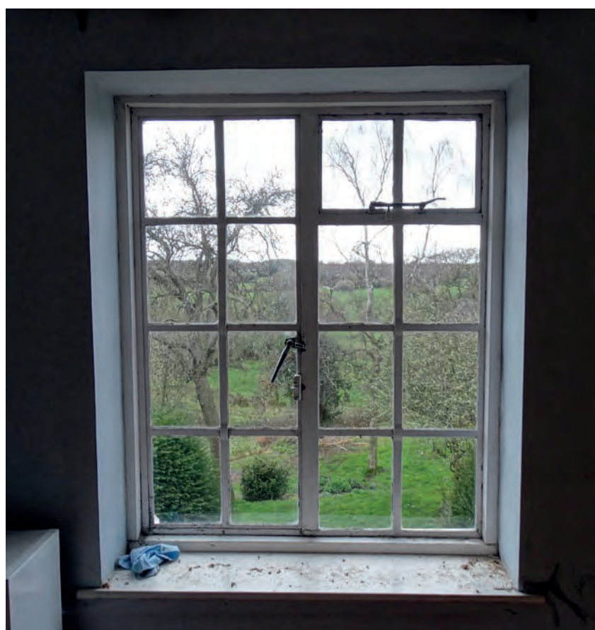
Plate 91: The southernmost window in the west wall of bedroom 1
