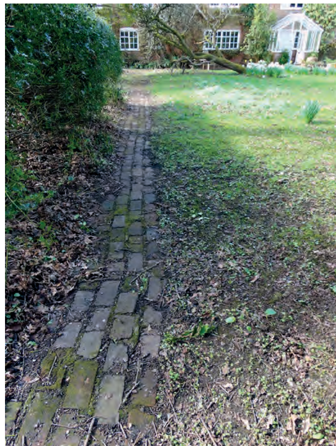
Plate 3: Footpath to the central and southern bays
