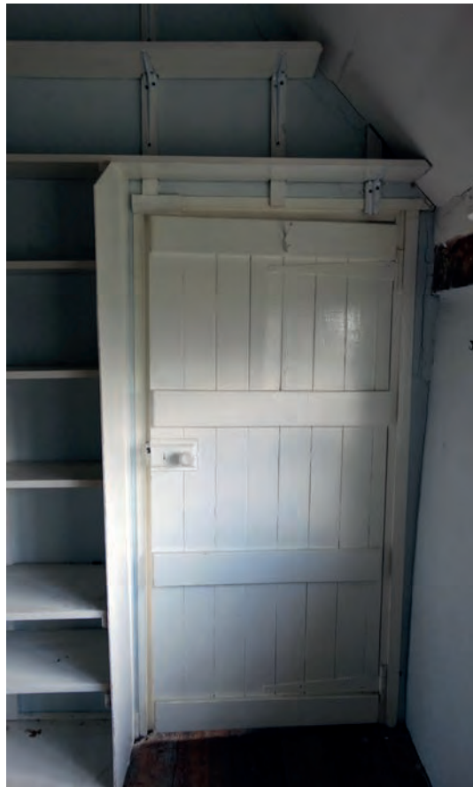
Plate 131: The door between the rear staircase landing and the study
