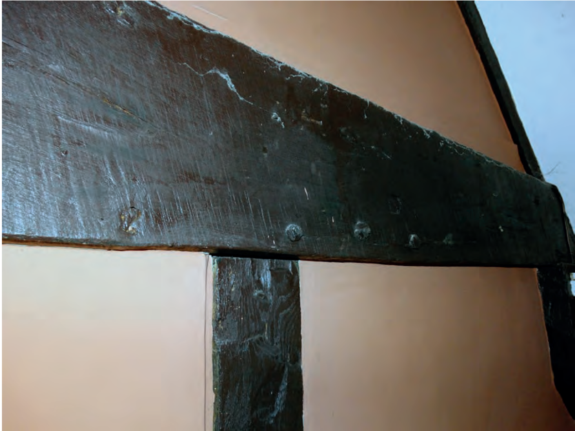
Plate 116: The sawn and hewn timbers
