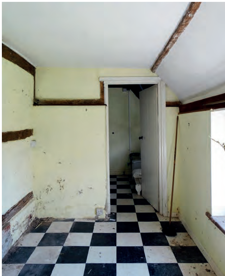
Plate 77: The south wall of the utility room
