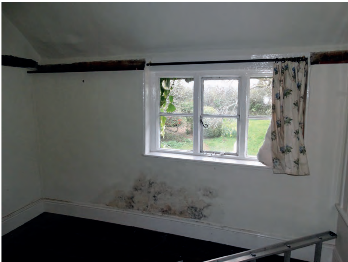
Plate 107: The east wall in bedroom 3
