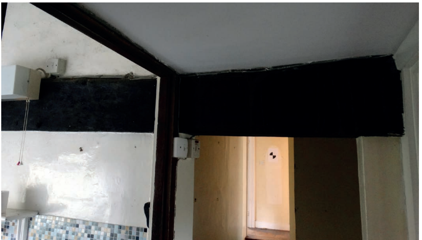
Plate 111: The tie beam between the north and central bays
