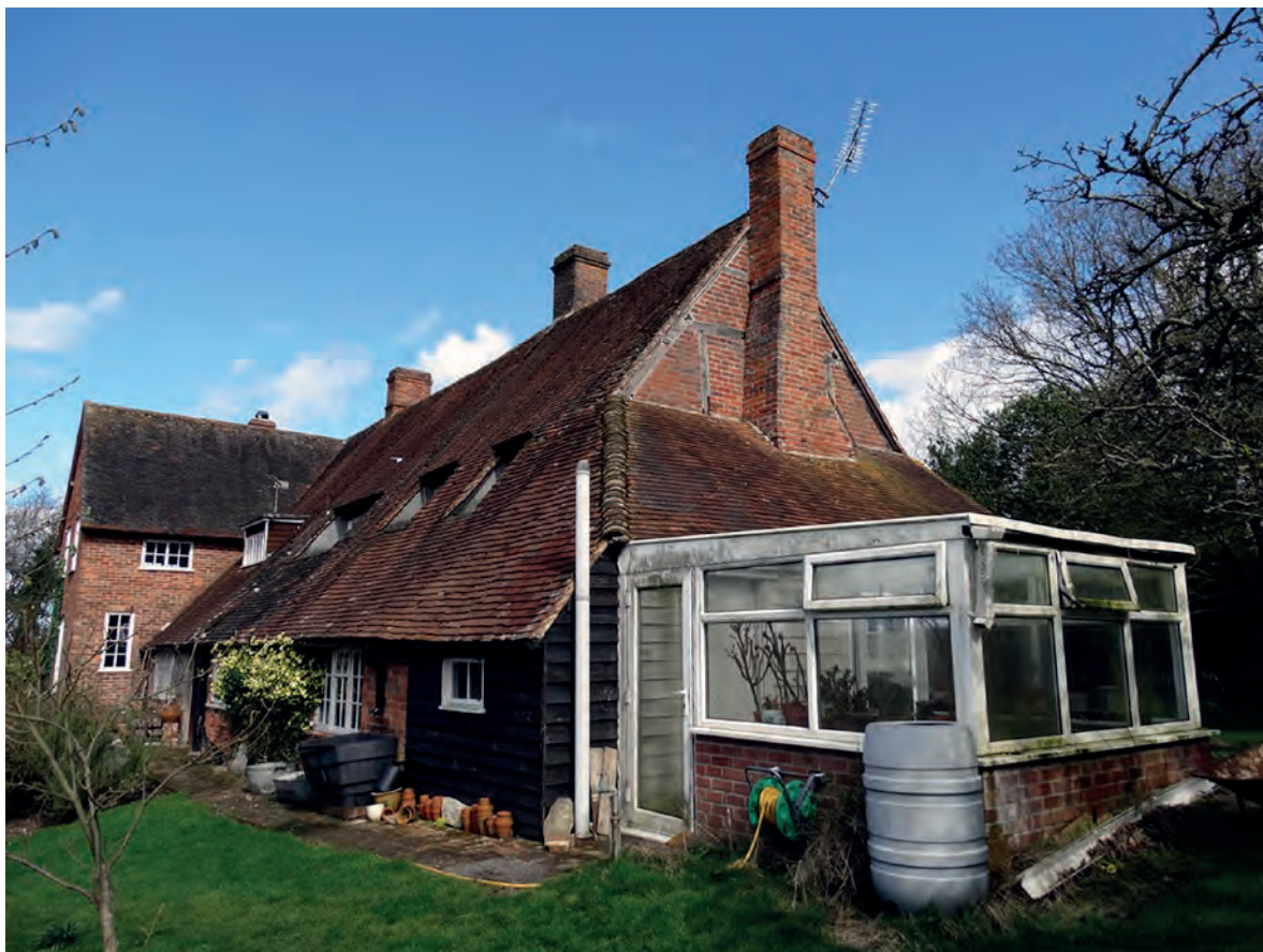
Plate 13: The south and west elevations
