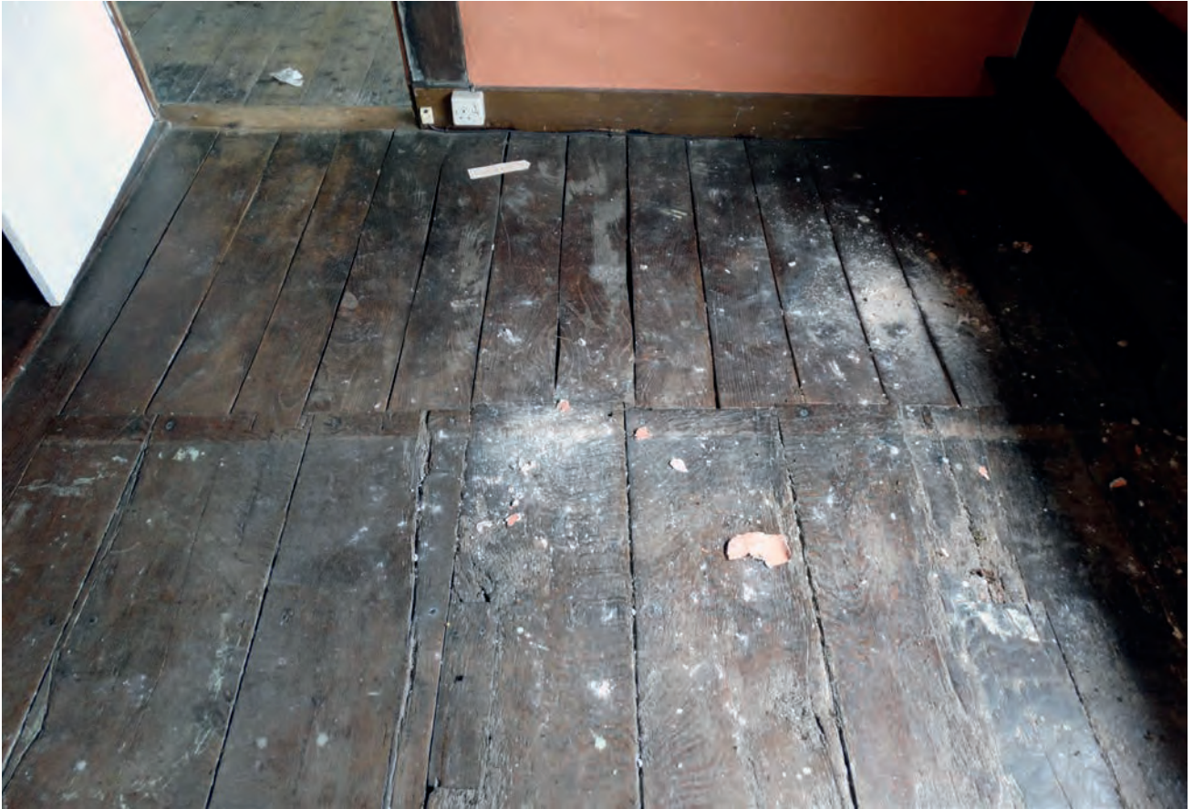
Plate 121: The floorboards in bedroom 5
