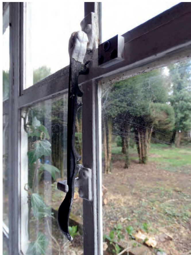
Plate 35: An example of a gun metal night ventilator stay
