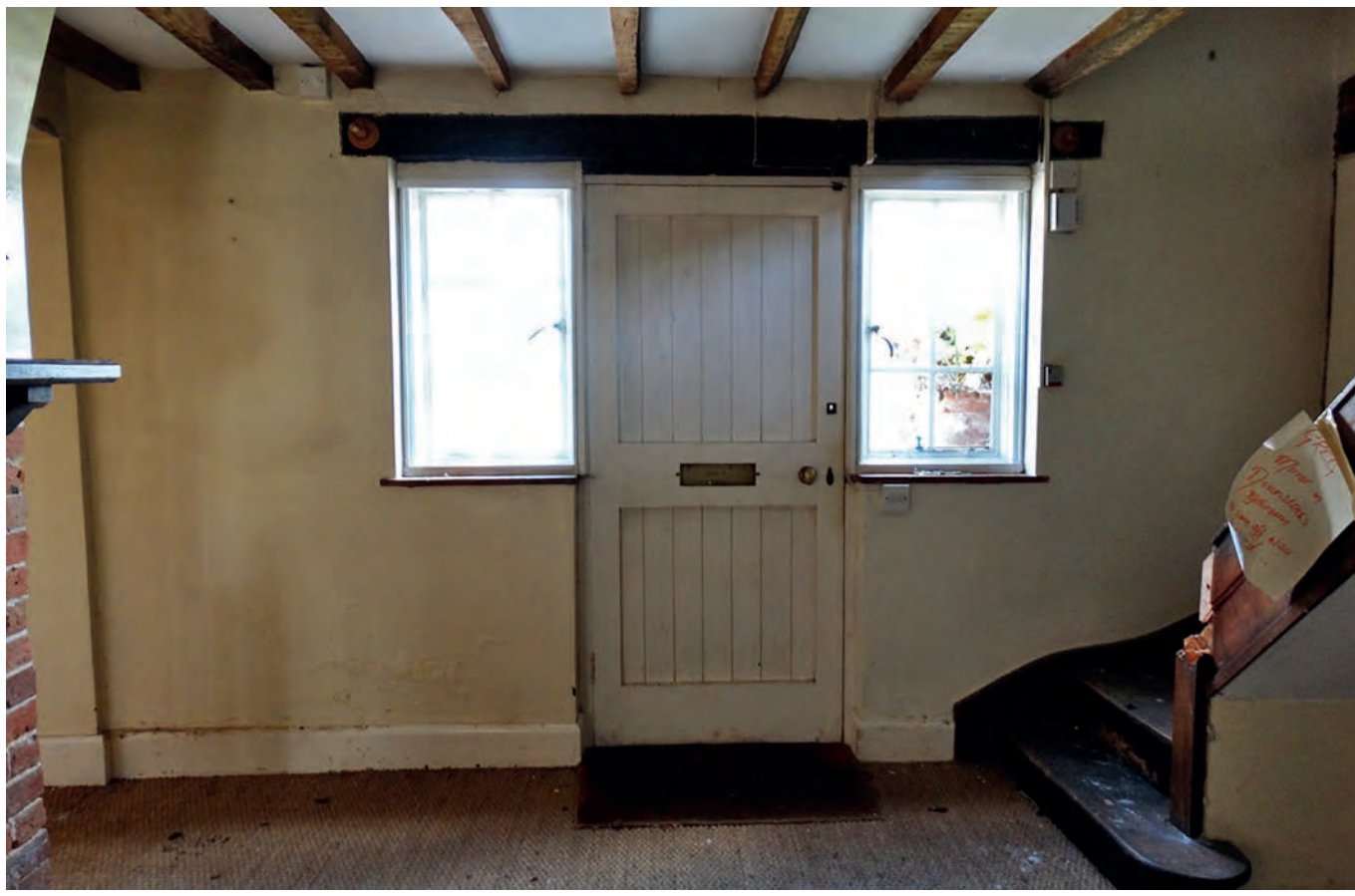
Plate 19: The entrance door in the east wall of the entrance hall
