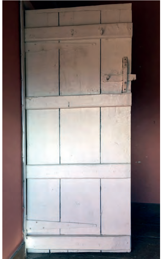
Plate 127: The early door between corridor 2 and bedroom 5
