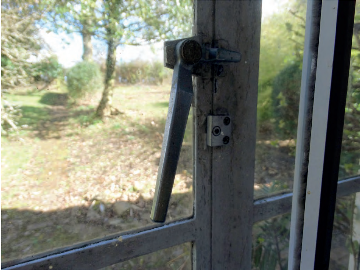
Plate 65: The handle of the metal-framed window in sitting room 2
