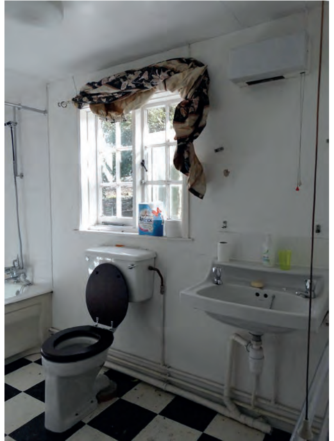
Plate 84: The west wall of bathroom 1
