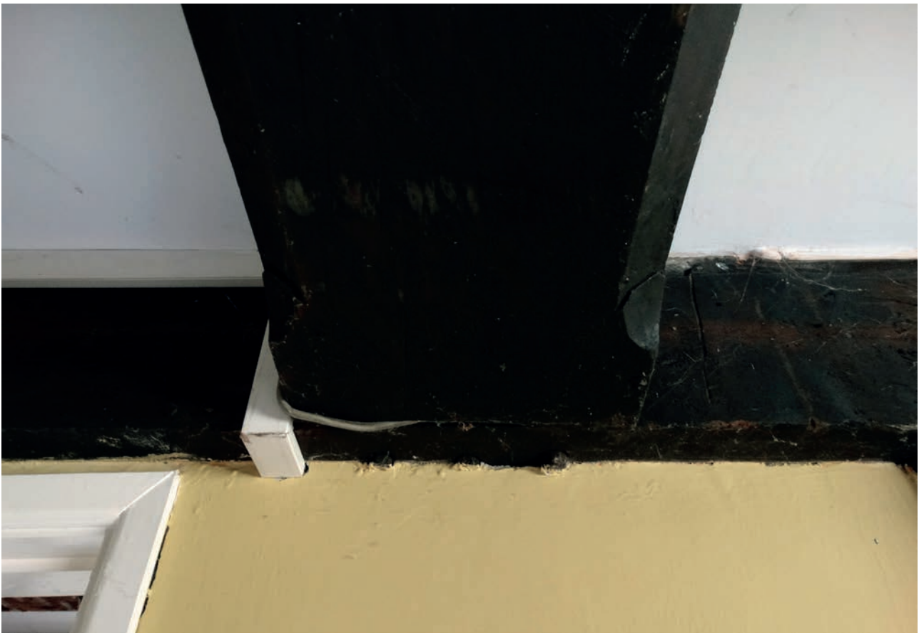
Plate 60: The chamfered and stopped beam in sitting room 1
