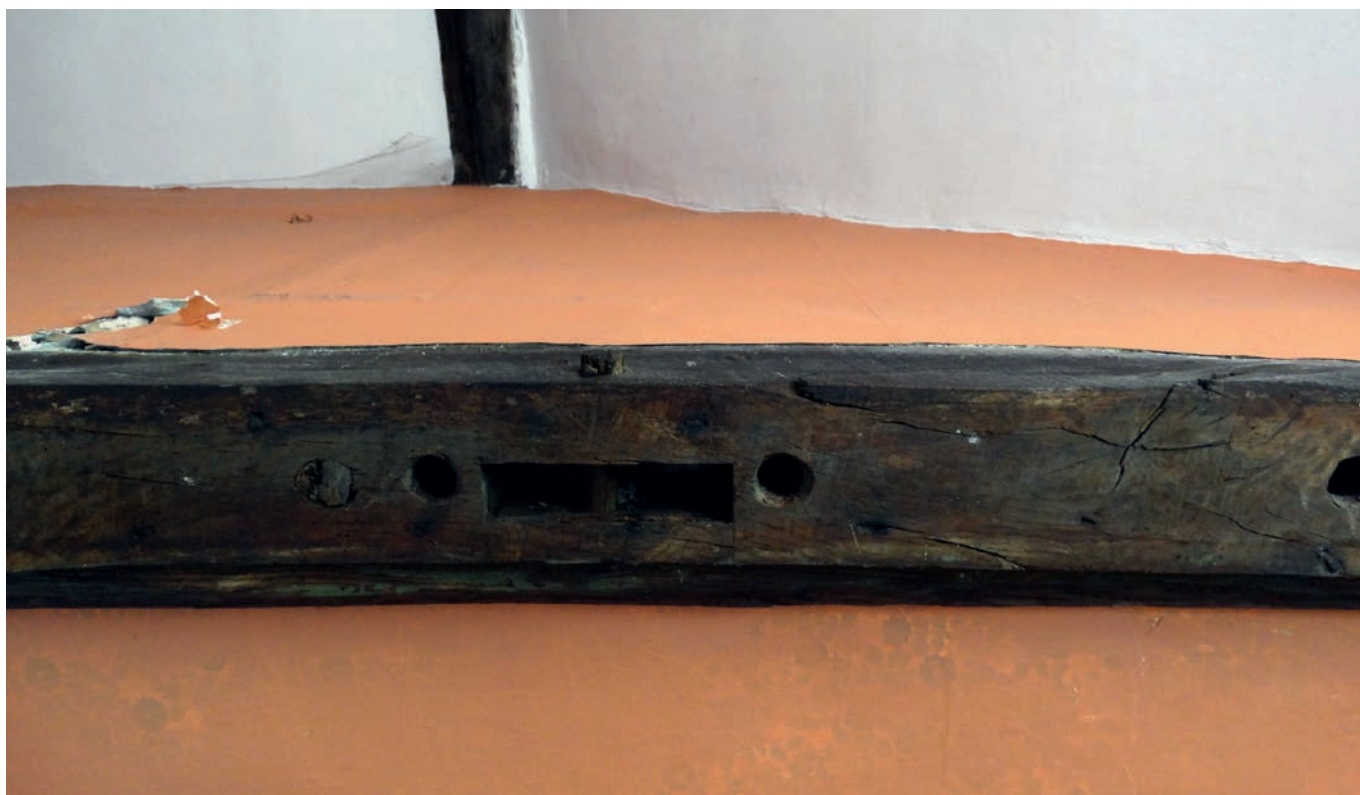
Plate 120: The redundant mortice and staves
