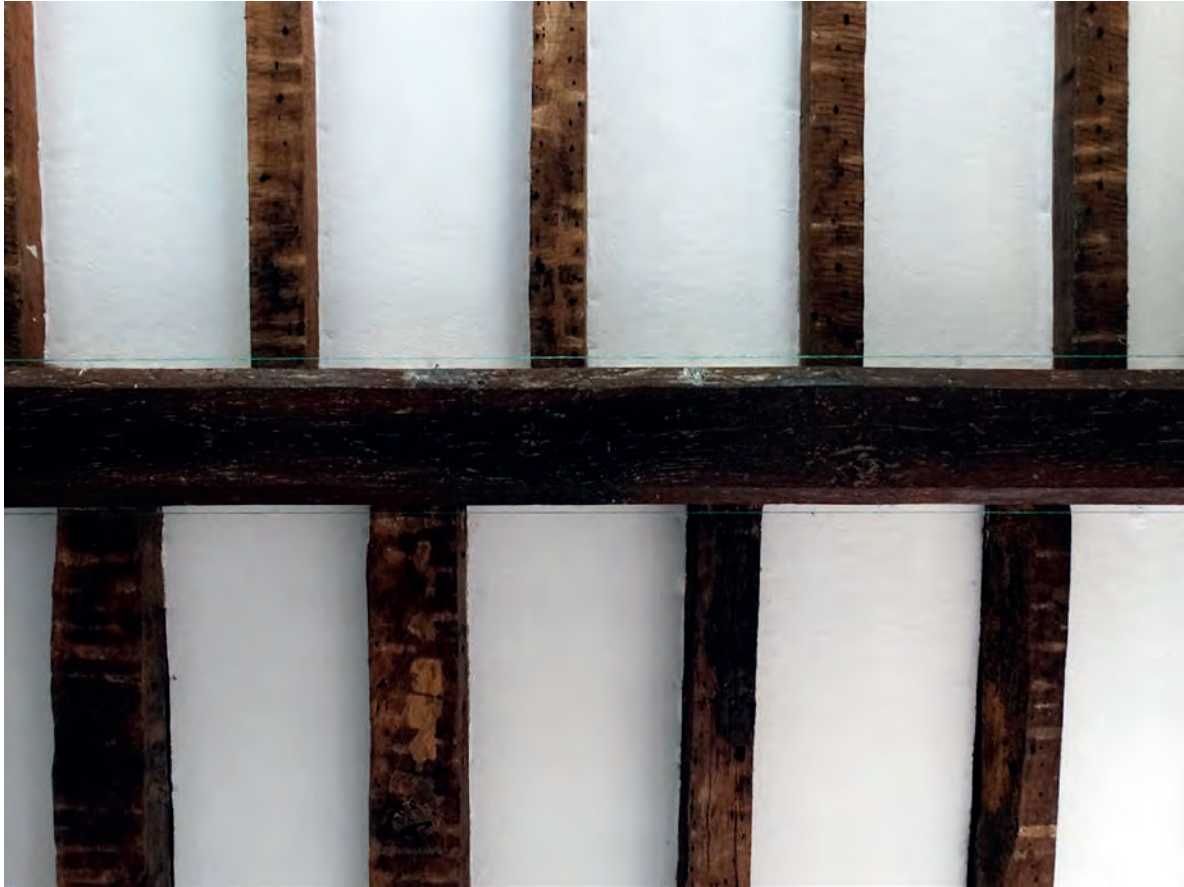
Plate 24: The arrangement of the joists in the entrance hall
