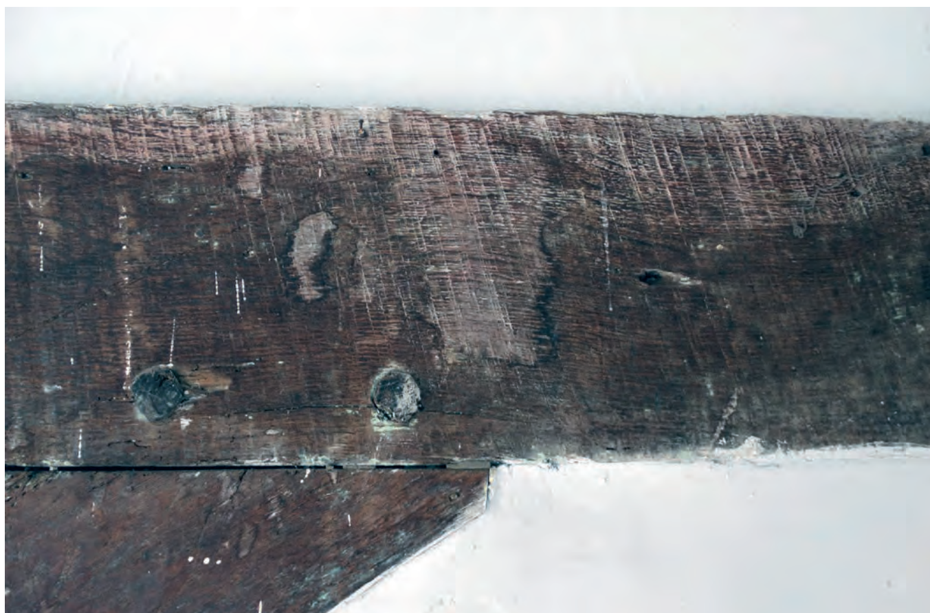
Plate 136: The saw marks
