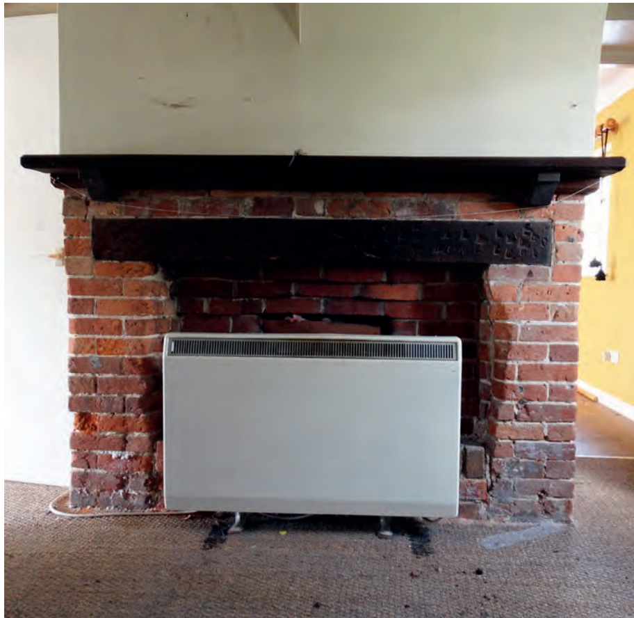
Plate 20: The fireplace in the entrance hall
