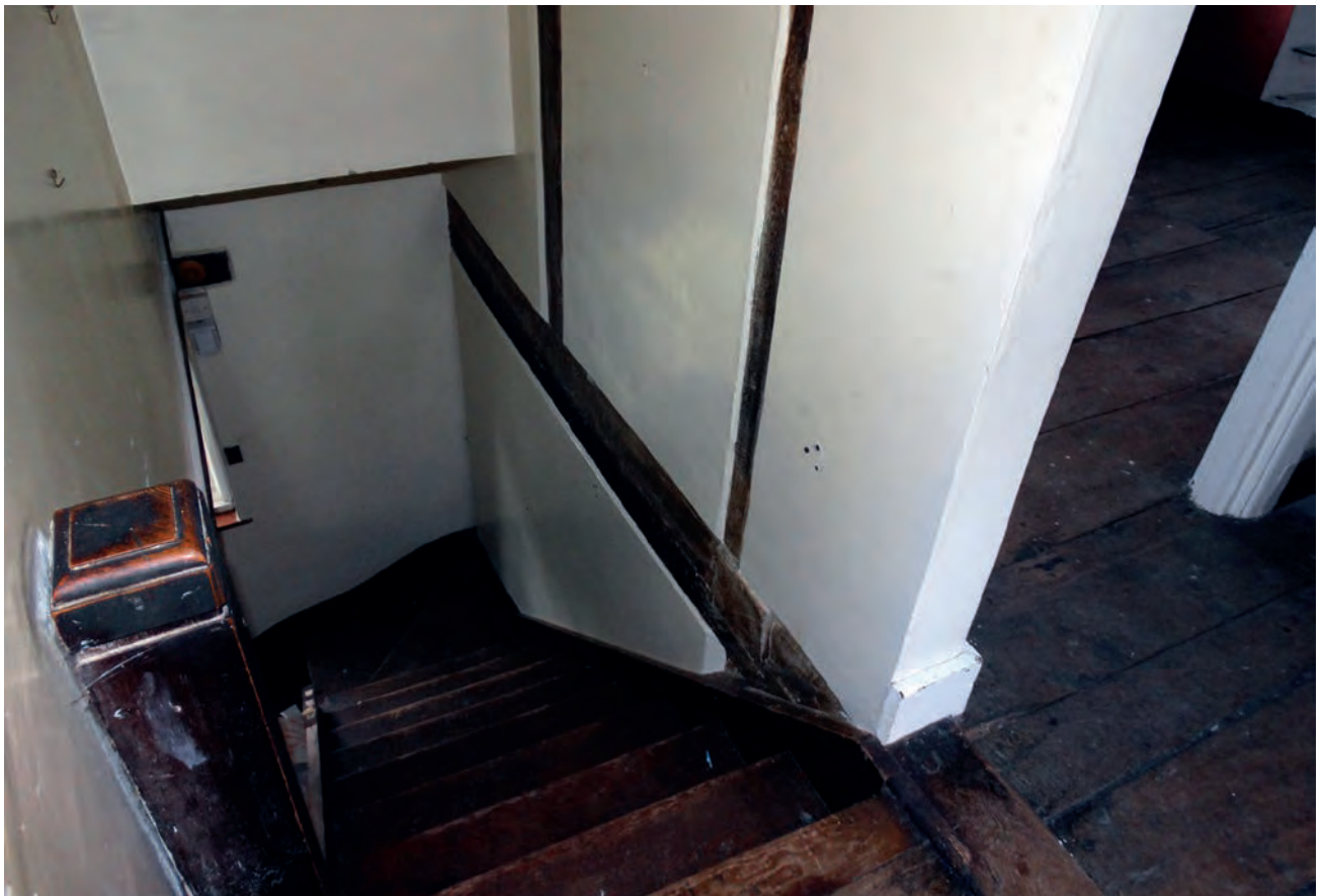
Plate 102: The timber frame above the modern staircase
