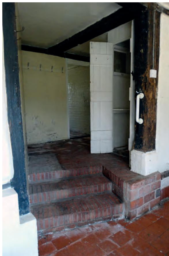
Plate 47: The original post and later steps between the kitchen and lobby
