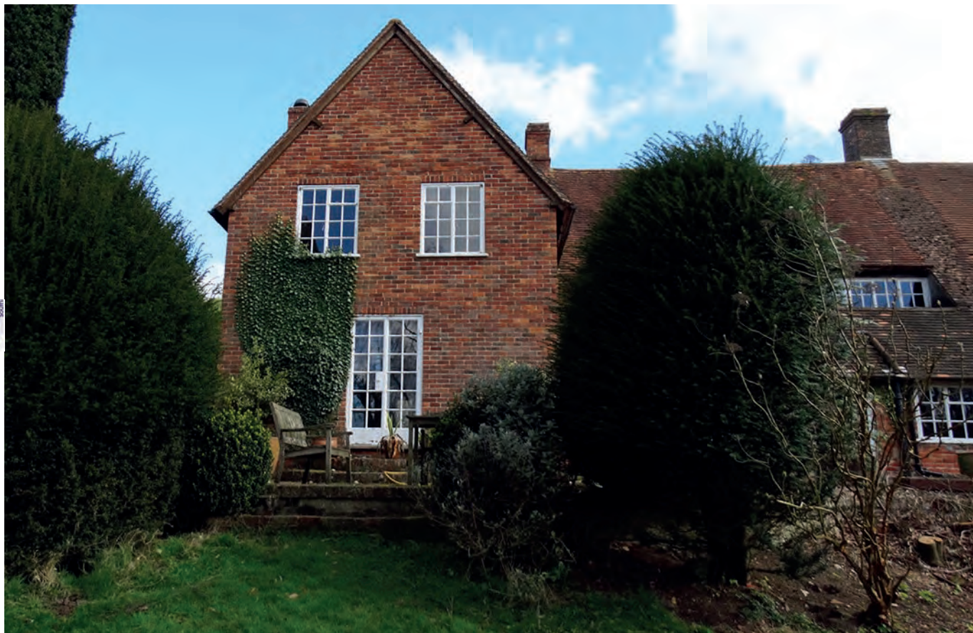
Plate 14: The west elevation of the 1974 extension
