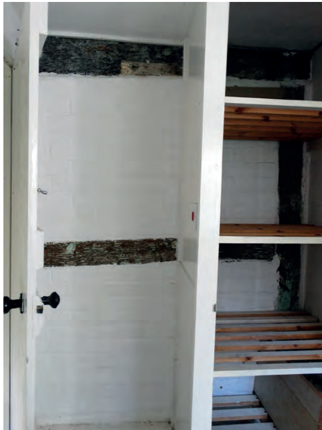
Plate 88: The visible frame in the east wall of bathroom 1
