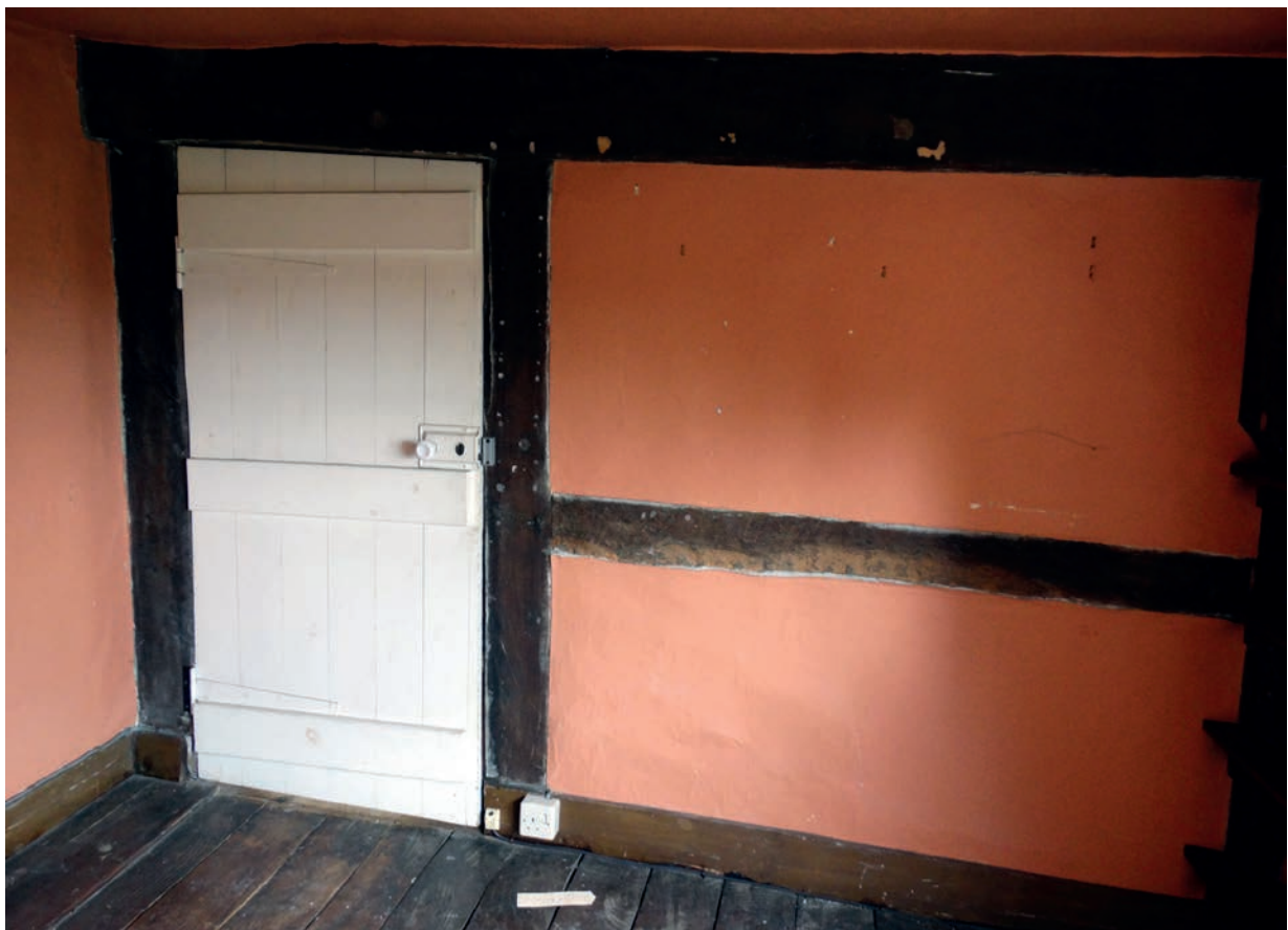
Plate 124: The south wall of bedroom 5
