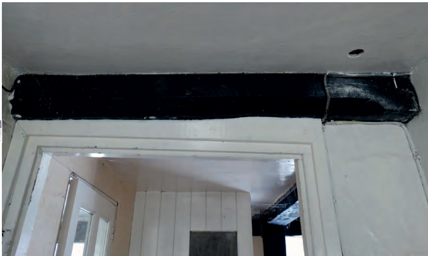
Plate 63: The chamfered and stopped beam in the pantry
