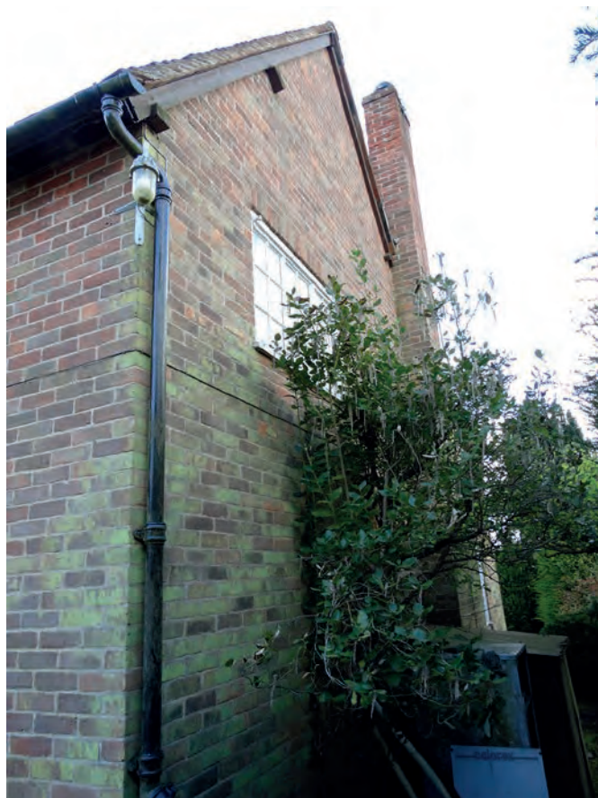
Plate 15: The north elevation
