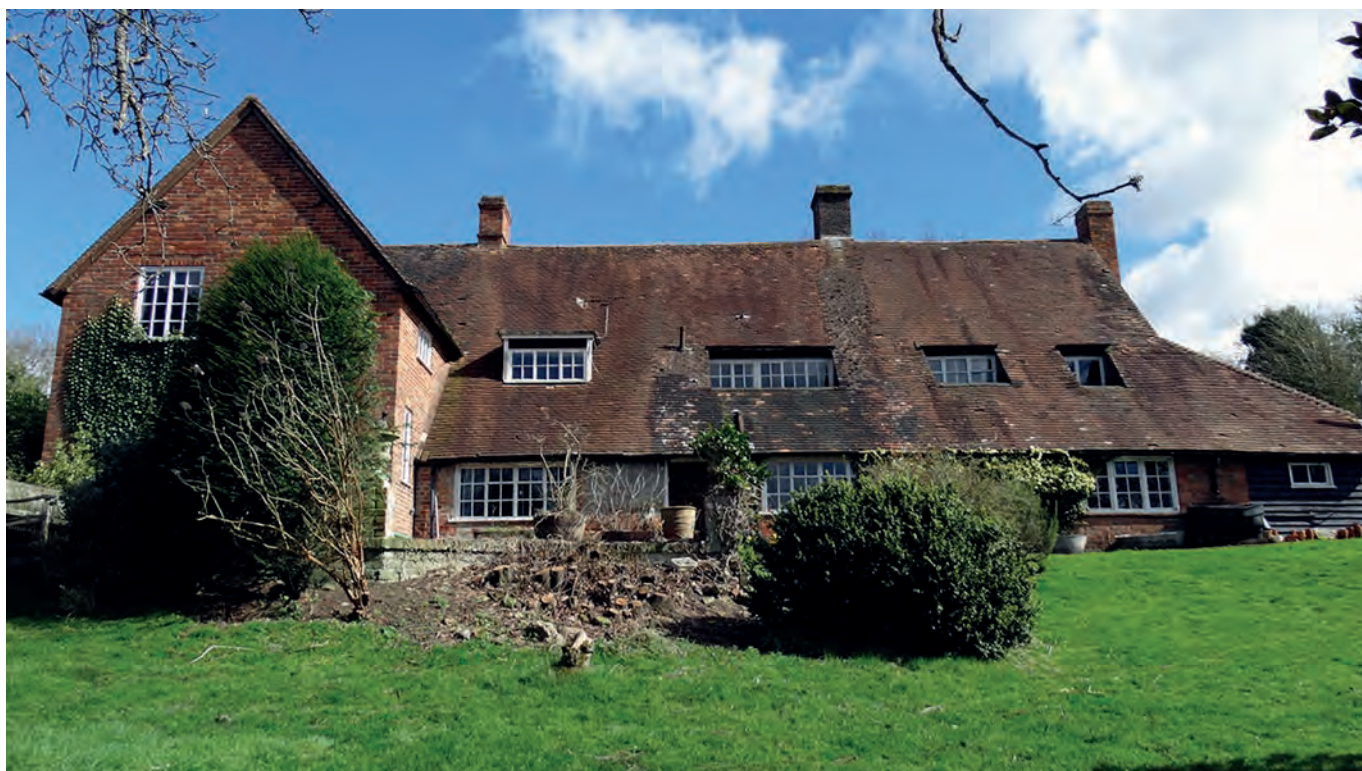
Plate 5: Rear, west-facing elevation
