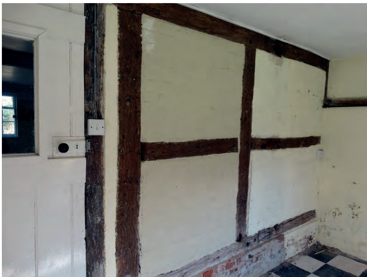
Plate 78: The east wall of the utility room
