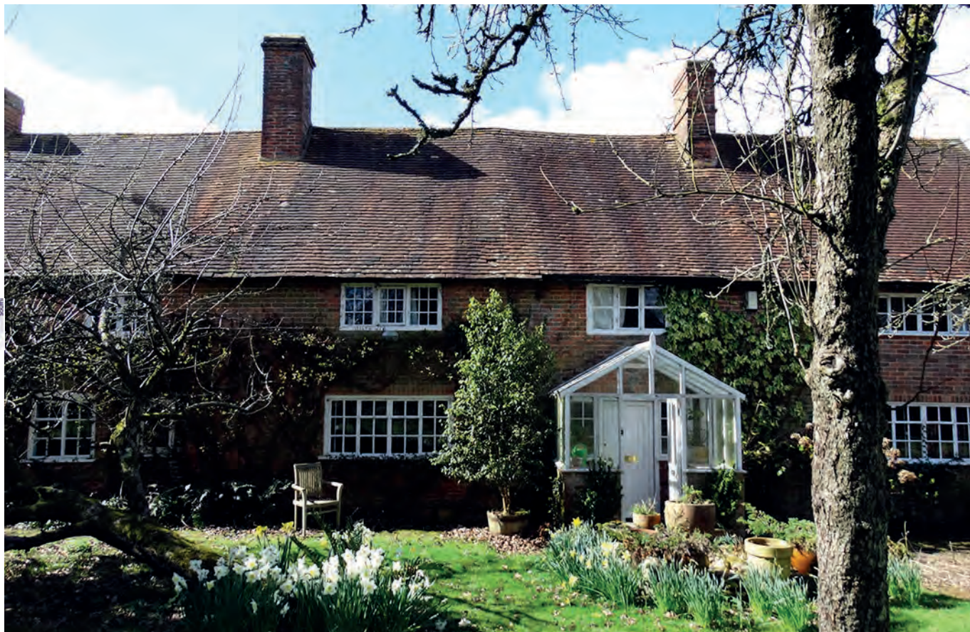
Plate 10: The north and central bays of the original building
