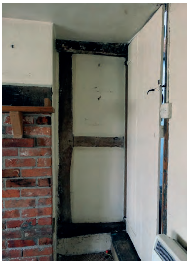
Plate 68: The timber frame visible in the south wall
