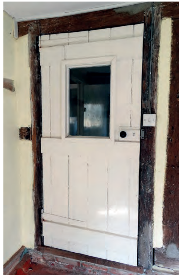
Plate 76: The door between sitting room 2 and the utility room
