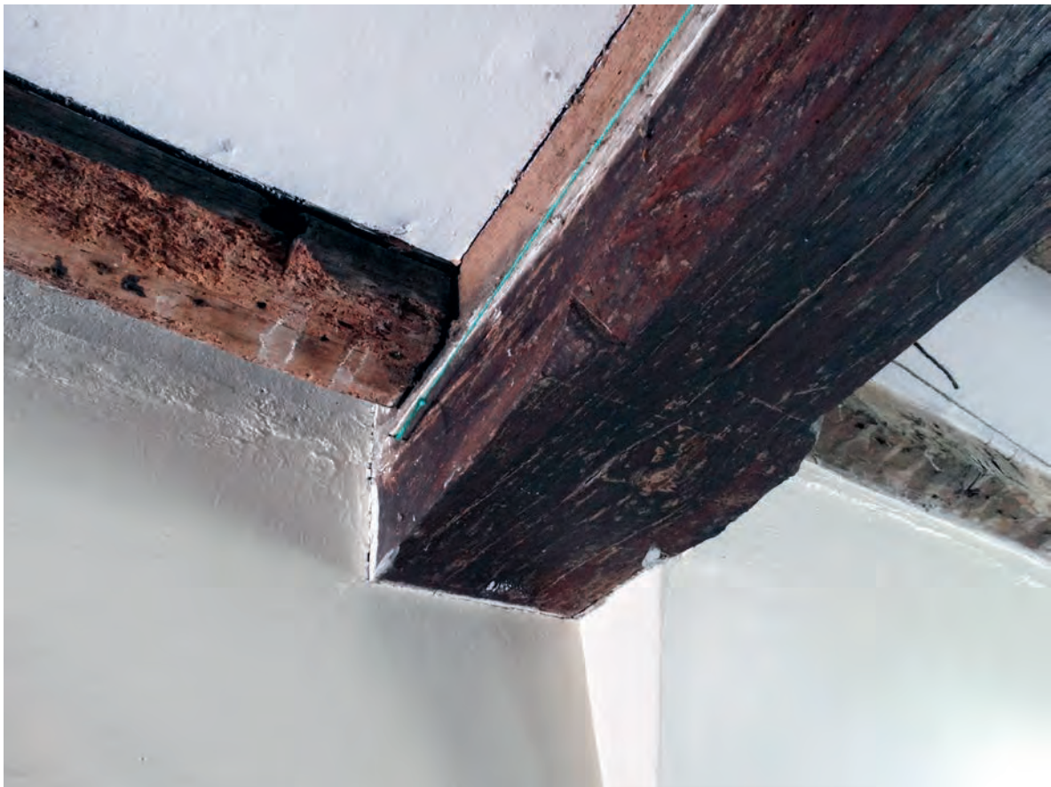
Plate 23: The chamfered and stopped beam above the fireplace
