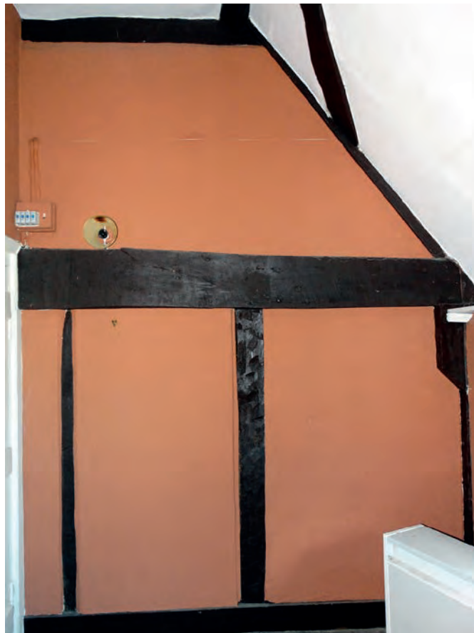
Plate 115: The north wall of bedroom 4
