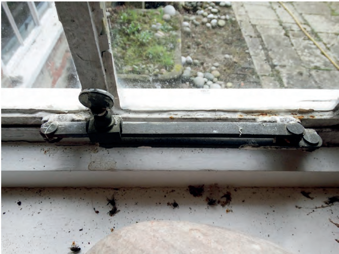
Plate 37: An example of a gun metal sliding stay
