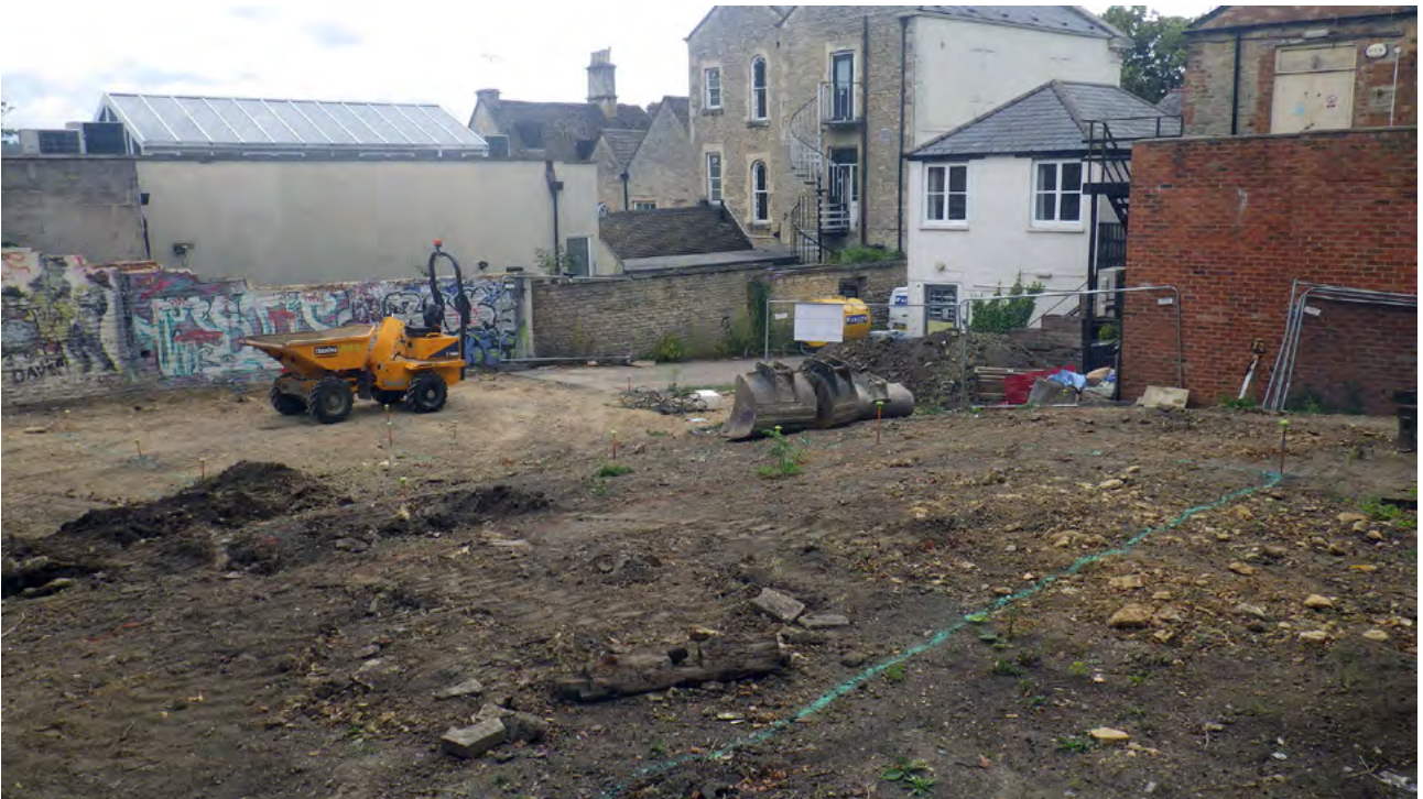
Plate 4: Site overview, looking north-east
