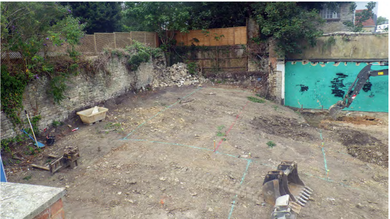
Plate 2: Site overview, looking west
