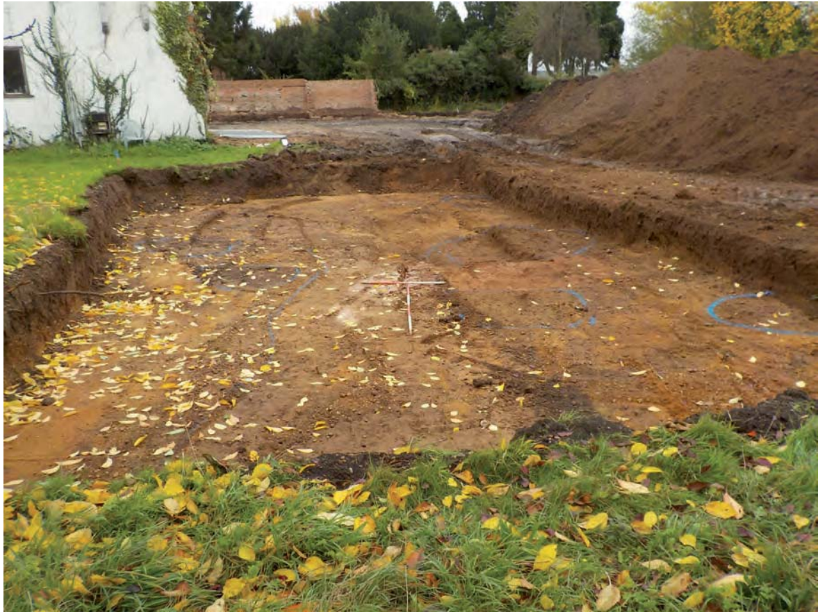
late 3: eneral shot of Trench 3 facing north
