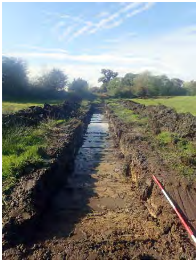
Plate 5: Trench 45, view to NW
