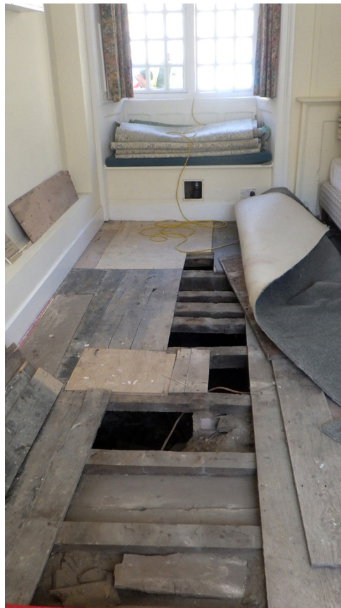
Plate 9: Floor 16 and basement structure 19, internal, view to east
