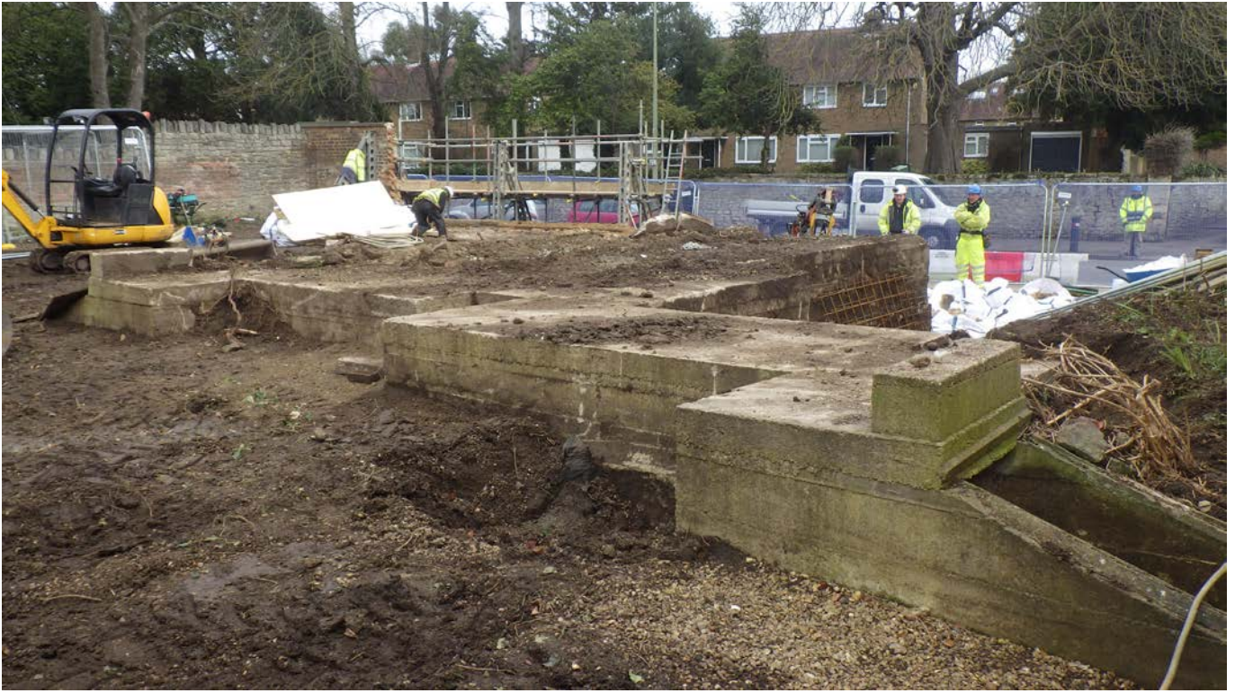
Plate 15: Air-raid shelter exposed before demolition, looking north-east
