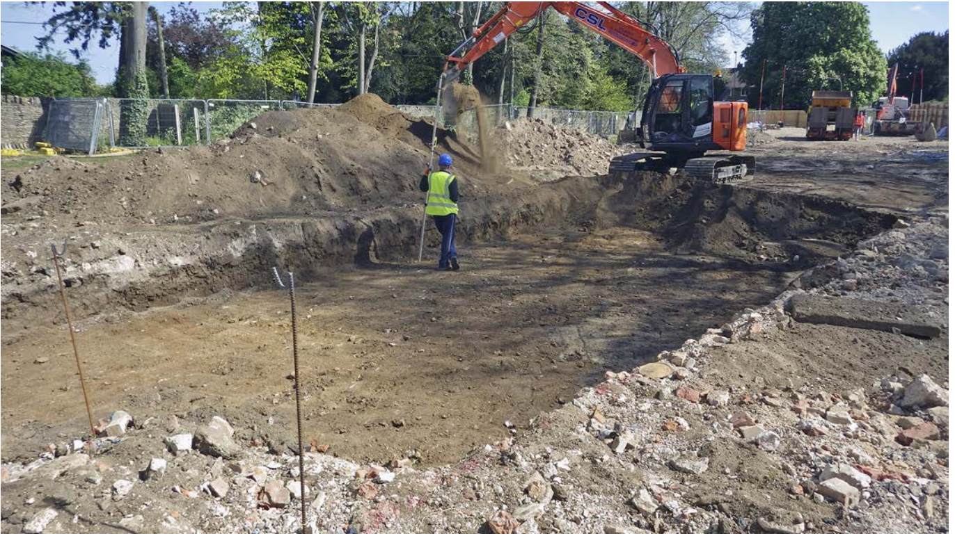
Plate 17: Stripping of the footprint of the new building, looking north-east
