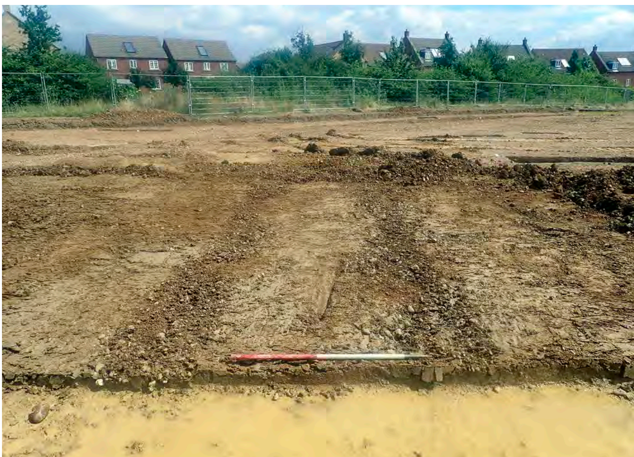
Plate 12: Potential wheel ruts 1079 below trackway/road surface 1021, looking north-east
