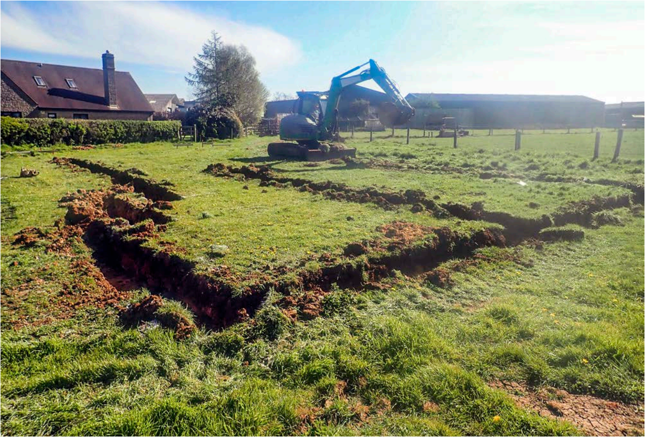
Plate 1: General shot of groundworks
