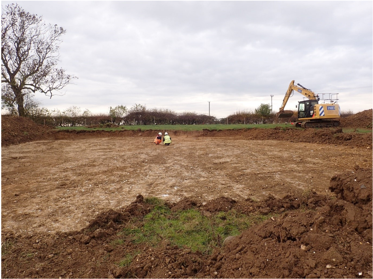
Plate 9: Mitigation excavation during stripping
