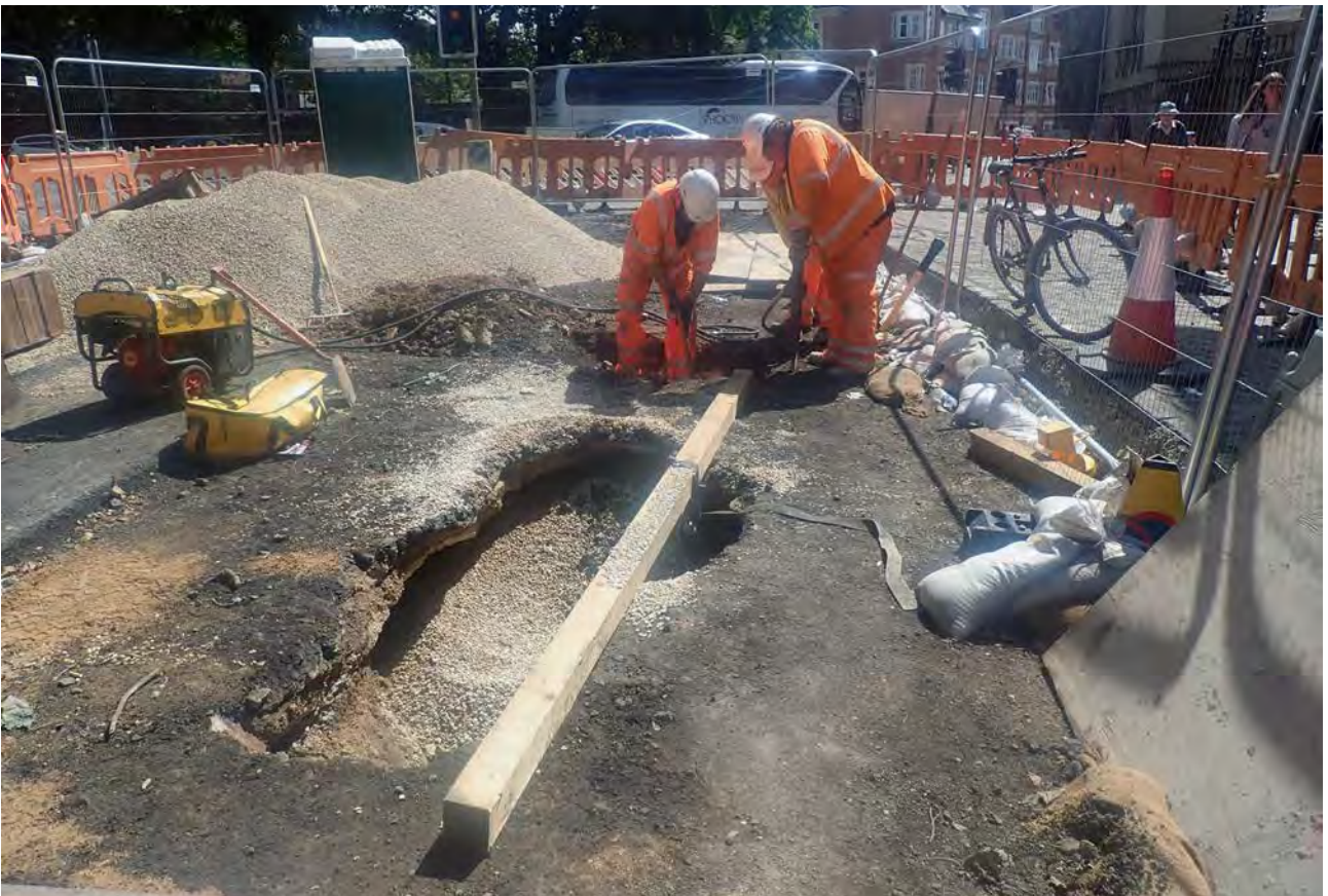
Plate 2: Backfilling void 1
