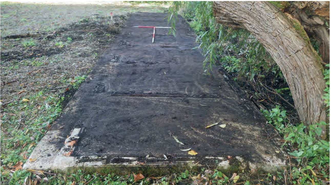
Plate 4: Structure 2, brick foundations of locker rooms visible, facing west
