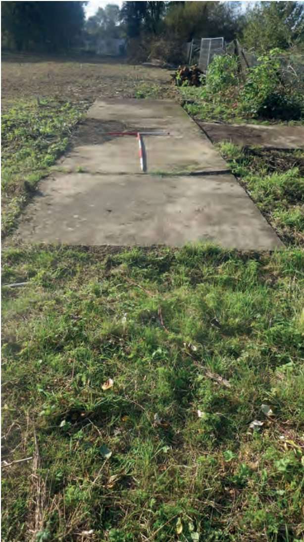
Plate 6: Structure 6, facing west
