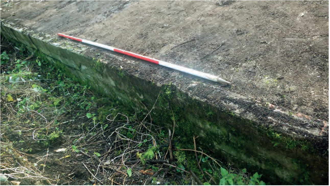
Plate 5: Structure 2, foundation of outer wall
