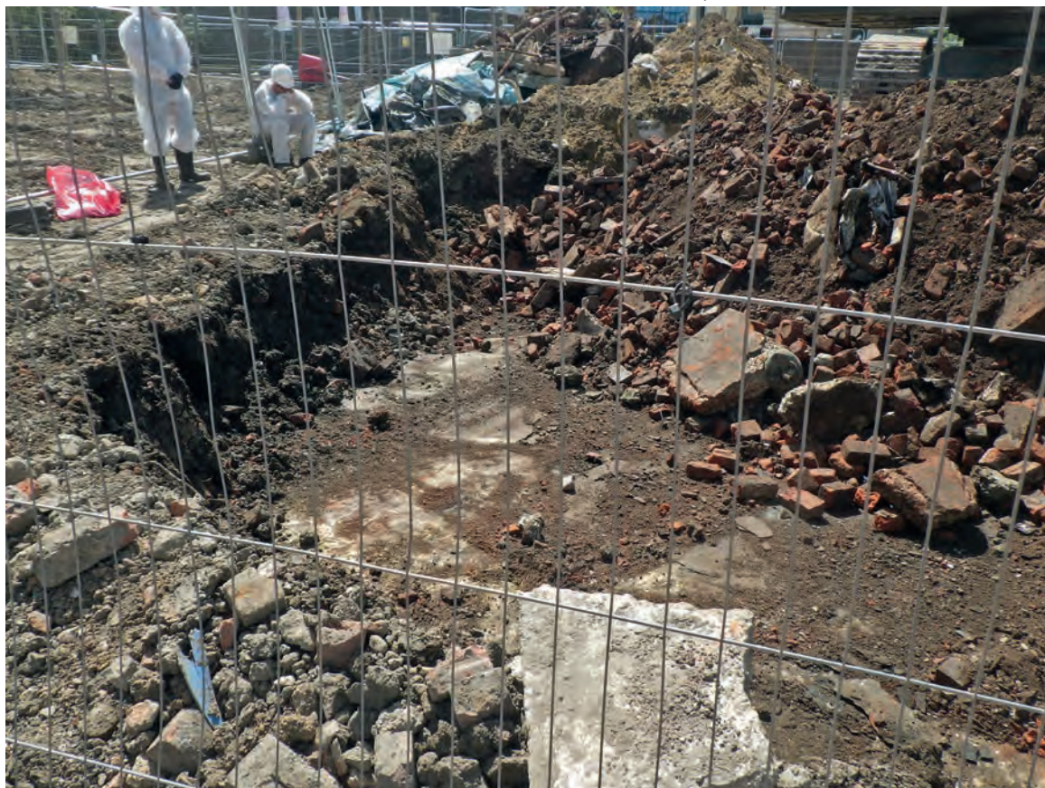
Plate 4: Trench 16, view to E
