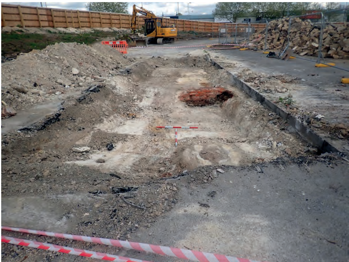
Plate 2: Trench 10, view to N
