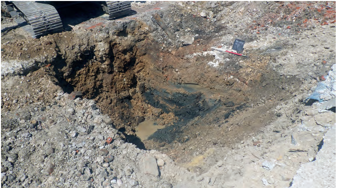
Trench 13 view to NW
