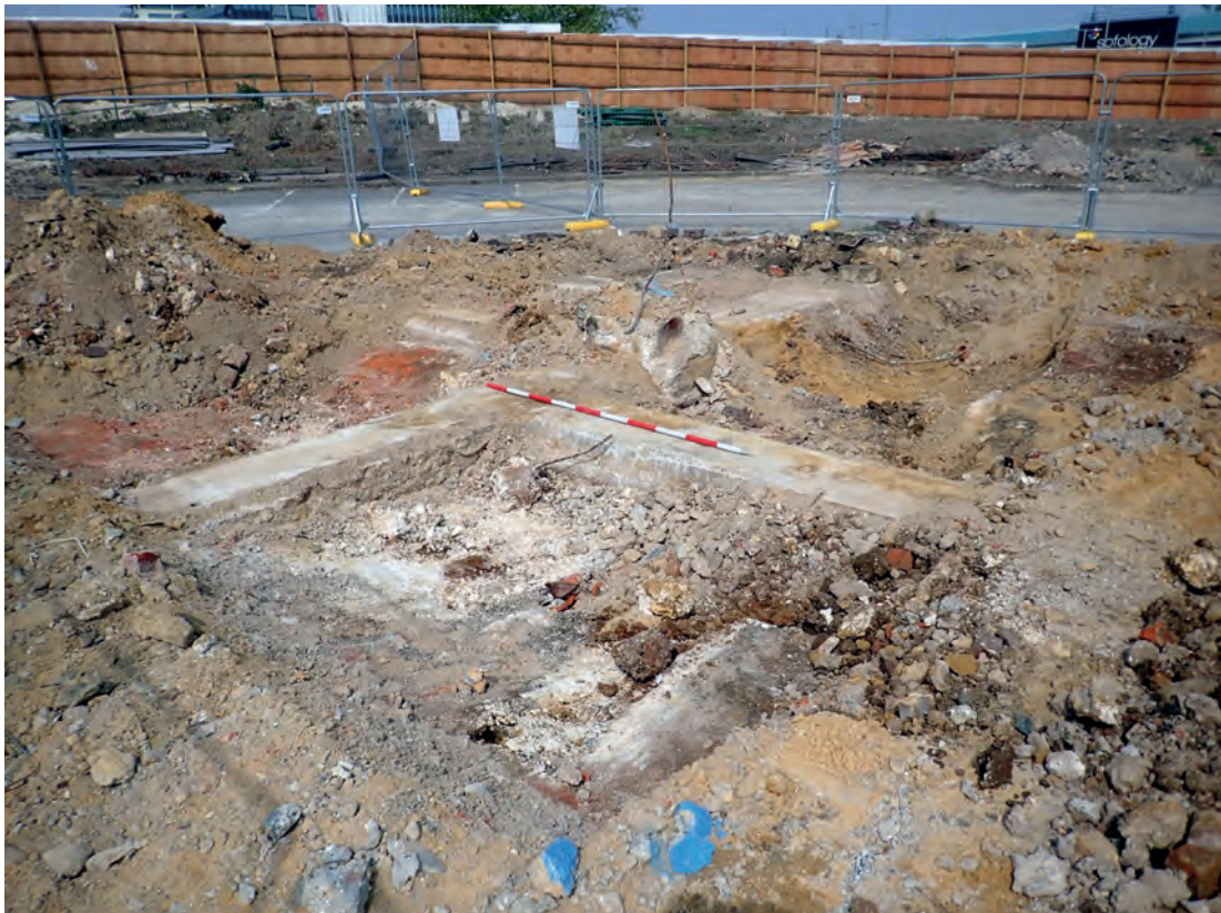
Trench 12a, view to NW
