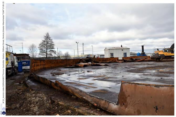
Plate 37: The partially demolished Gasholder 4
