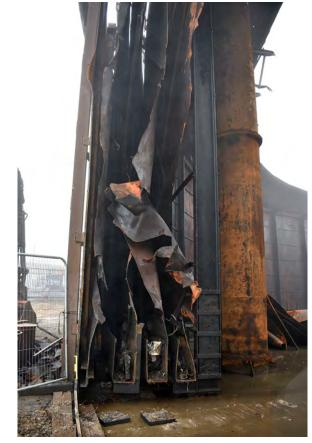
Plate 33: A section through the tank and lifts of Gasholder 4
