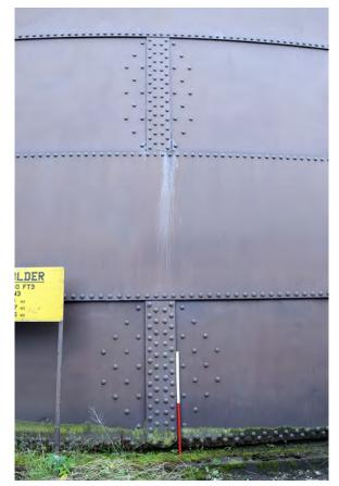
Plate 8: Example of the riveting of Gasholder 3
