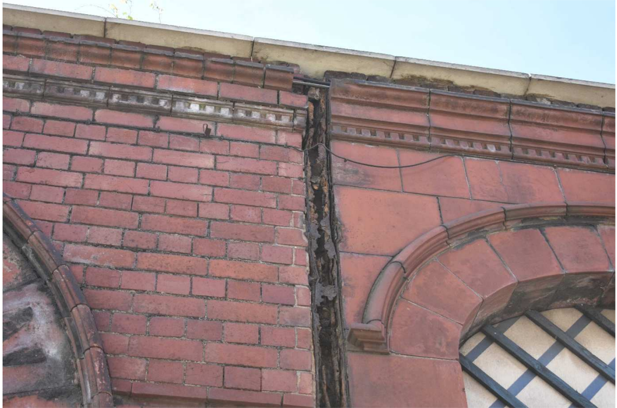
Plate 30: Junction between phases on north side of wall
