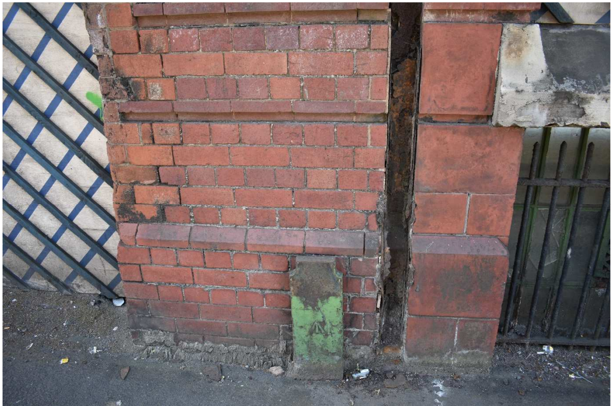
Plate 29: Junction between phases on north side of wall
