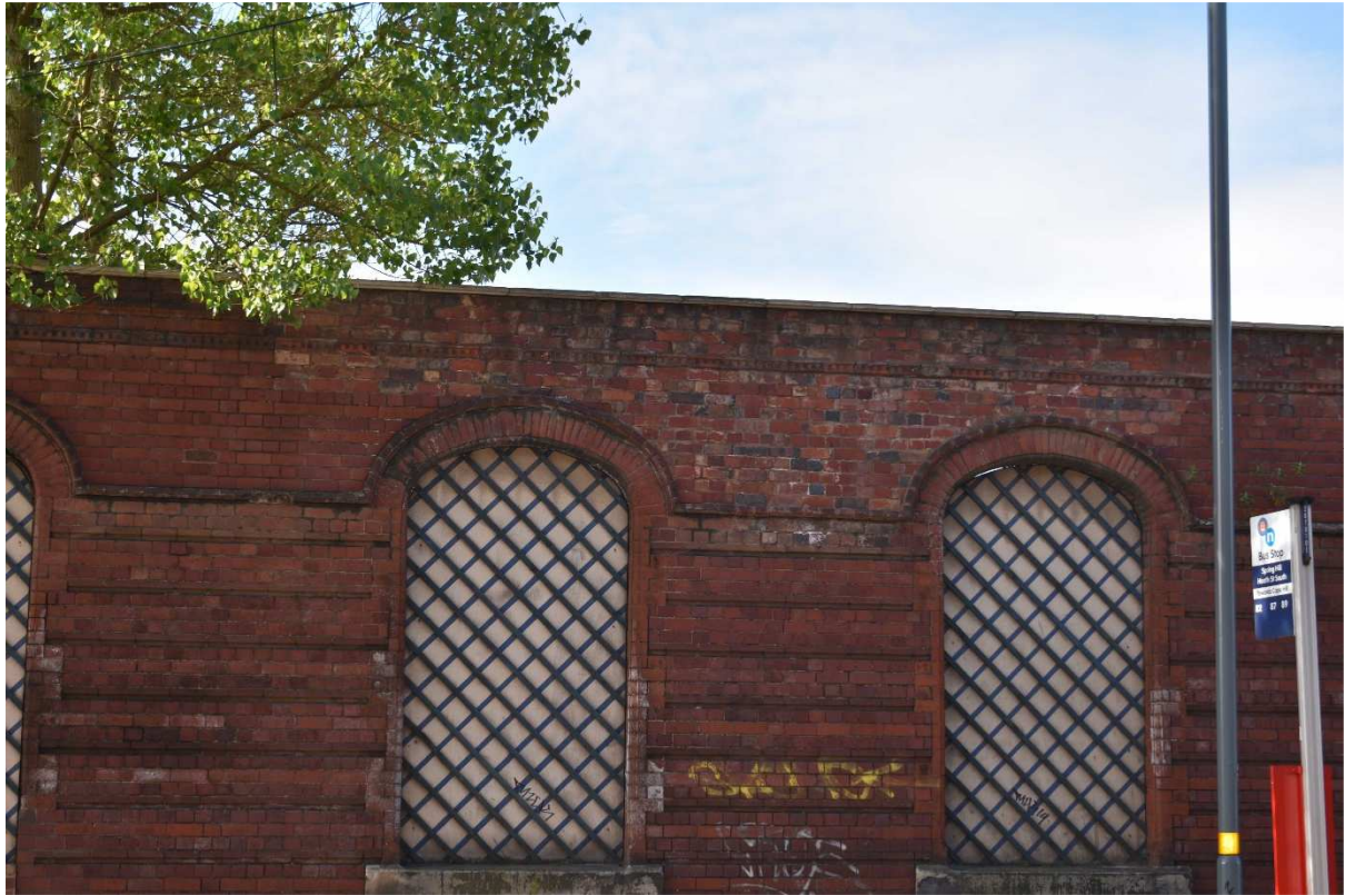
Plate 22: Bays in north side of wall, rebuilt brickwork over windows
