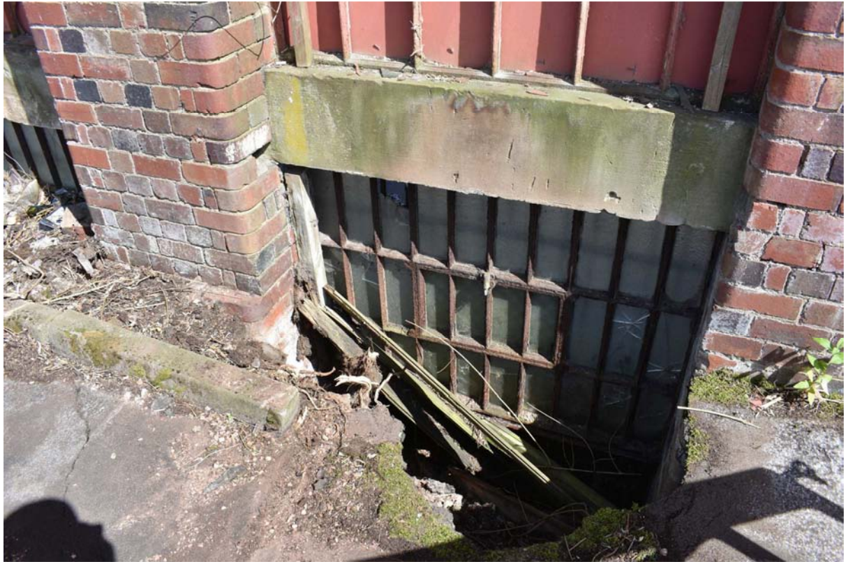
Plate 52: South side of former basement window
