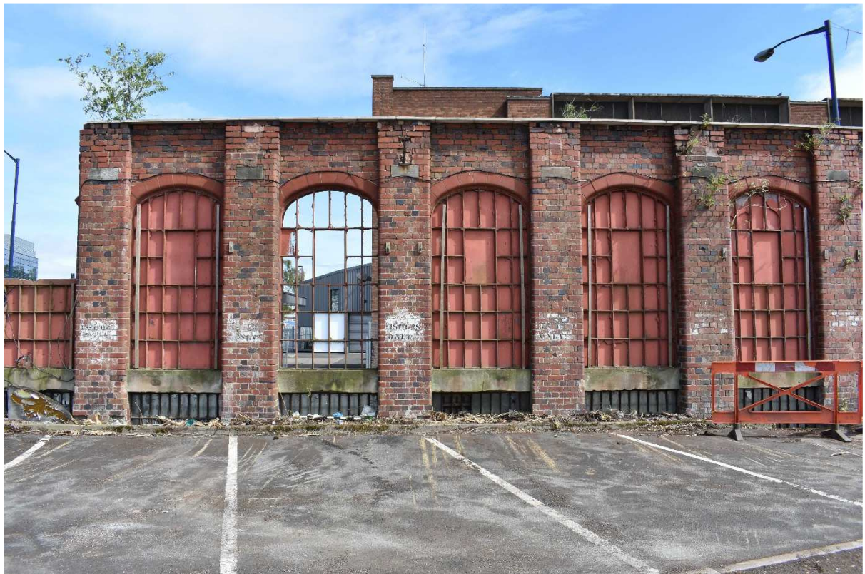
Plate 47: Western section of south face of wall
