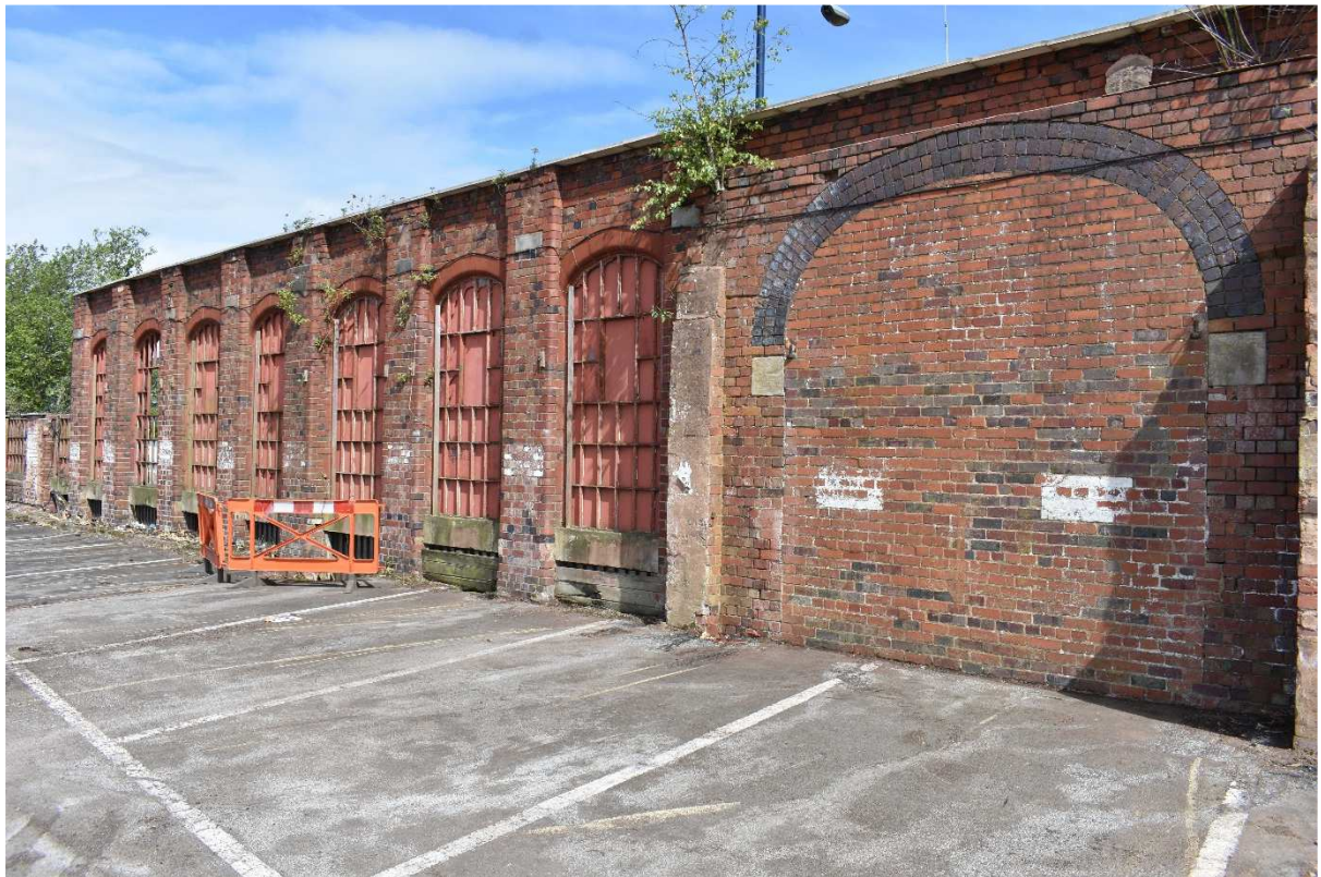
Plate 35: South side of wall looking to north-west
