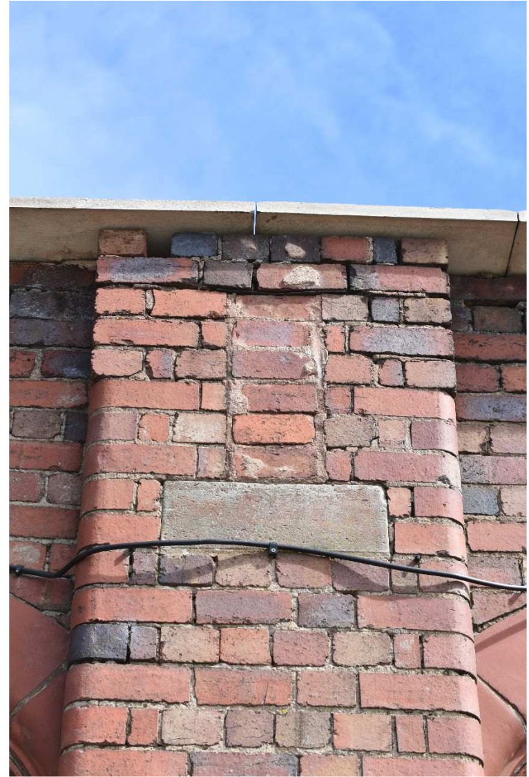
Plate 51: infilled socket from former truss end
