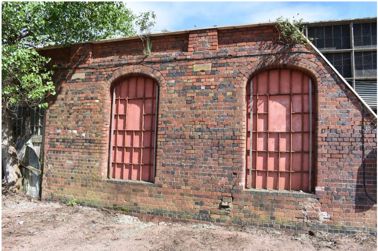
Plate 43: Typical bays in east half of wall
