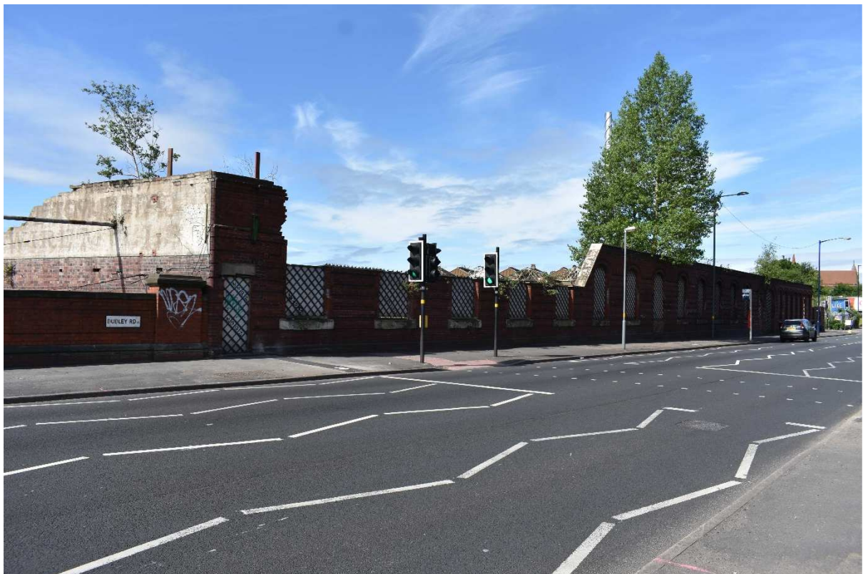
Plate 27: General view of wall from north-east
