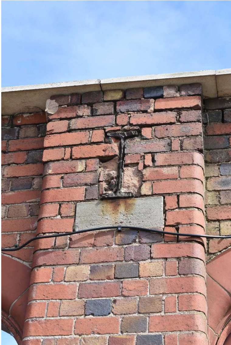
Plate 50: Truncated roof truss (early 20 th -century extension)
