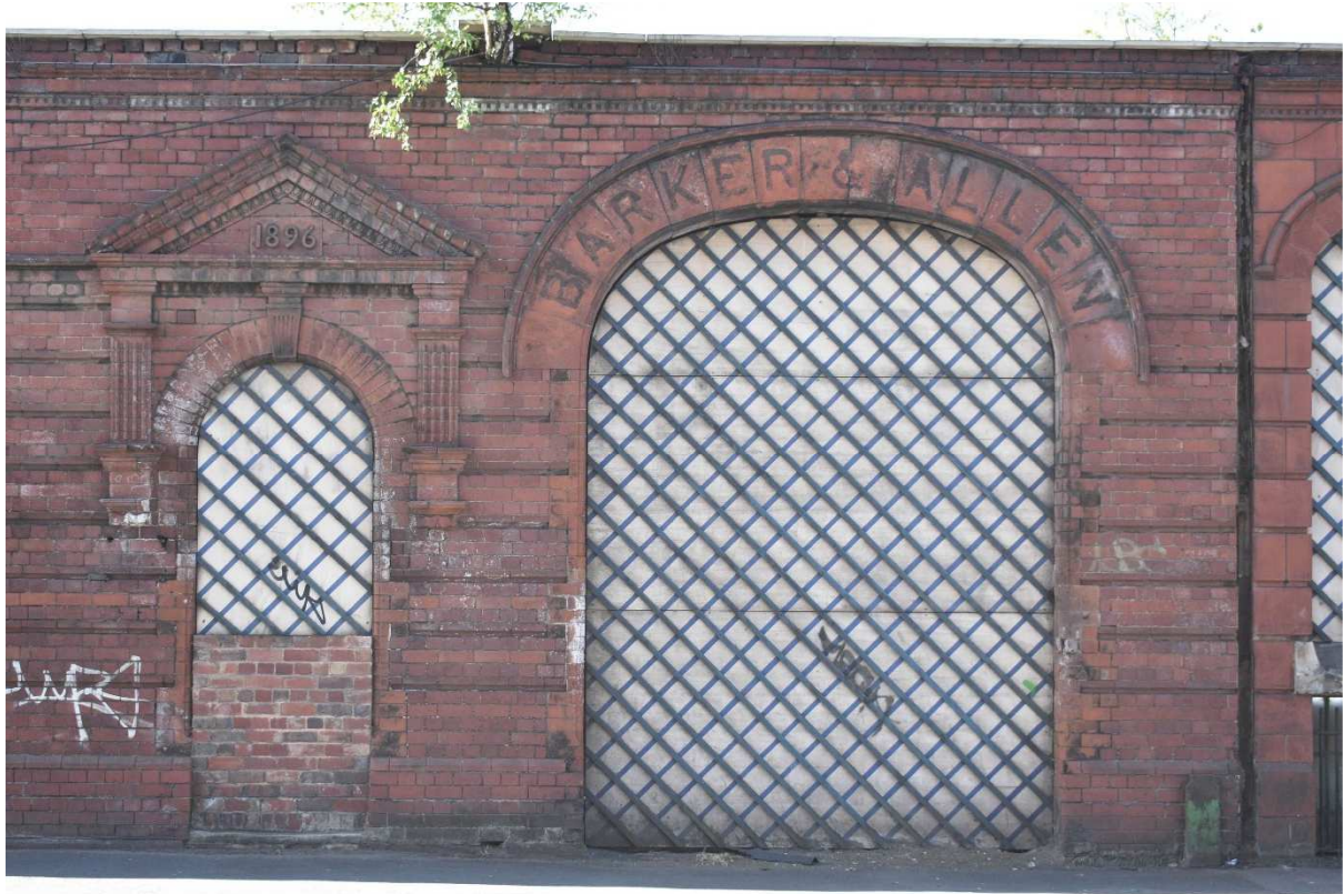
Plate 18: Archway and doorway, north side of wall
