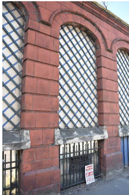
Plate 33: Typical bays in western extension
