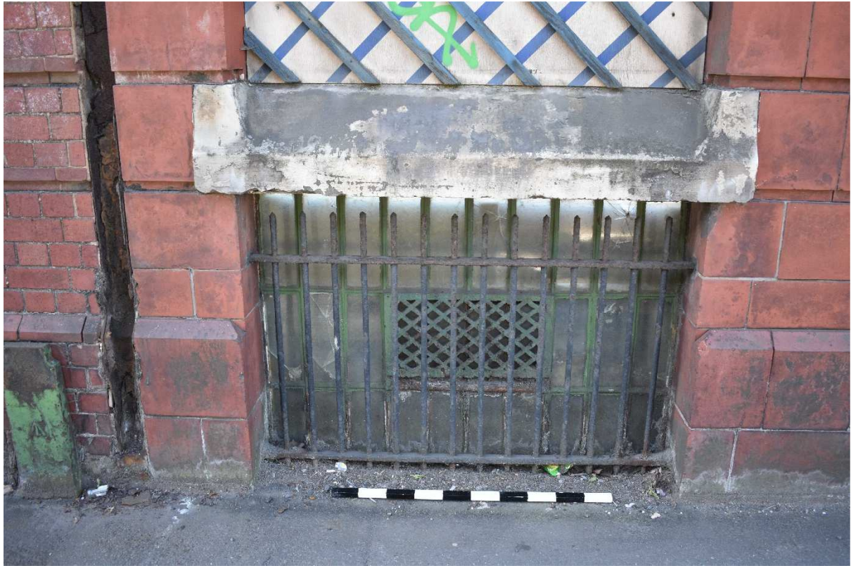
Plate 32: North side of former basement window
