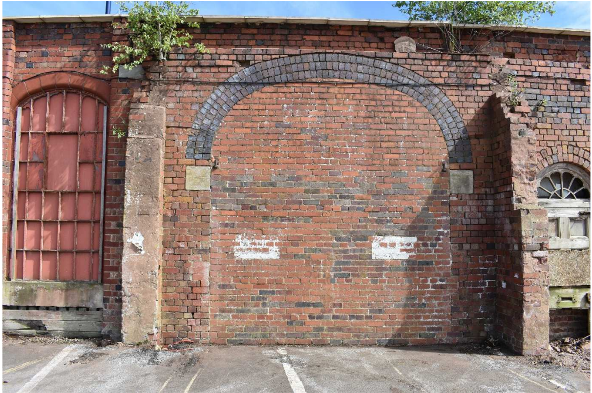
Plate 36: South side of blocked archway
