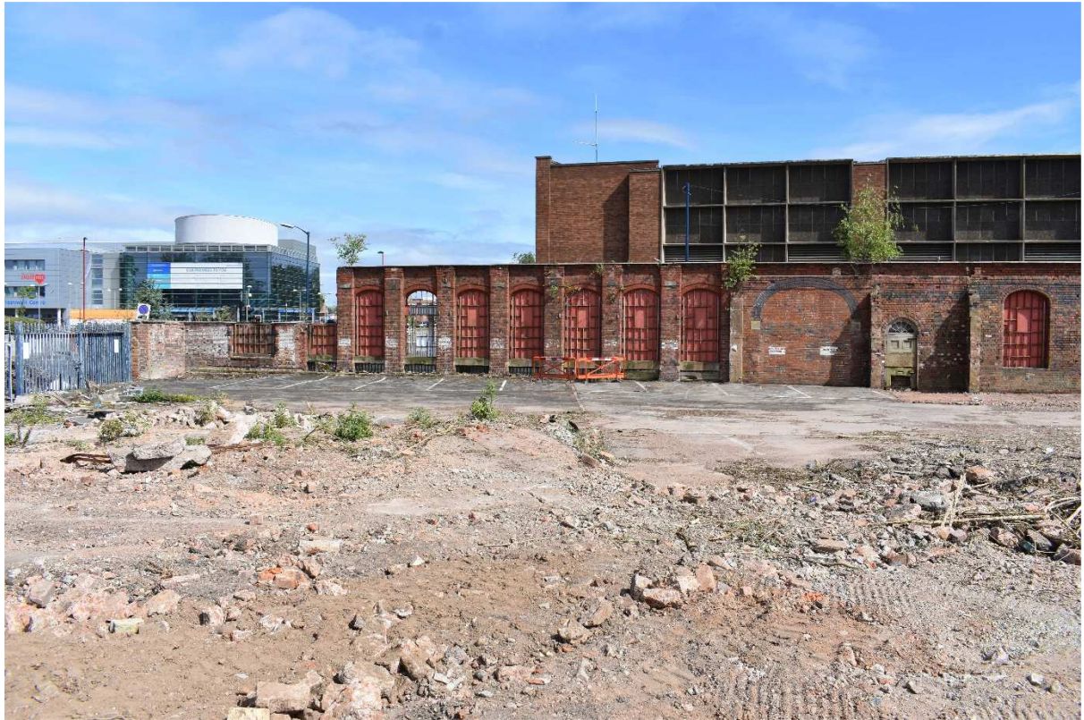
Plate 34: South side of wall, western part
