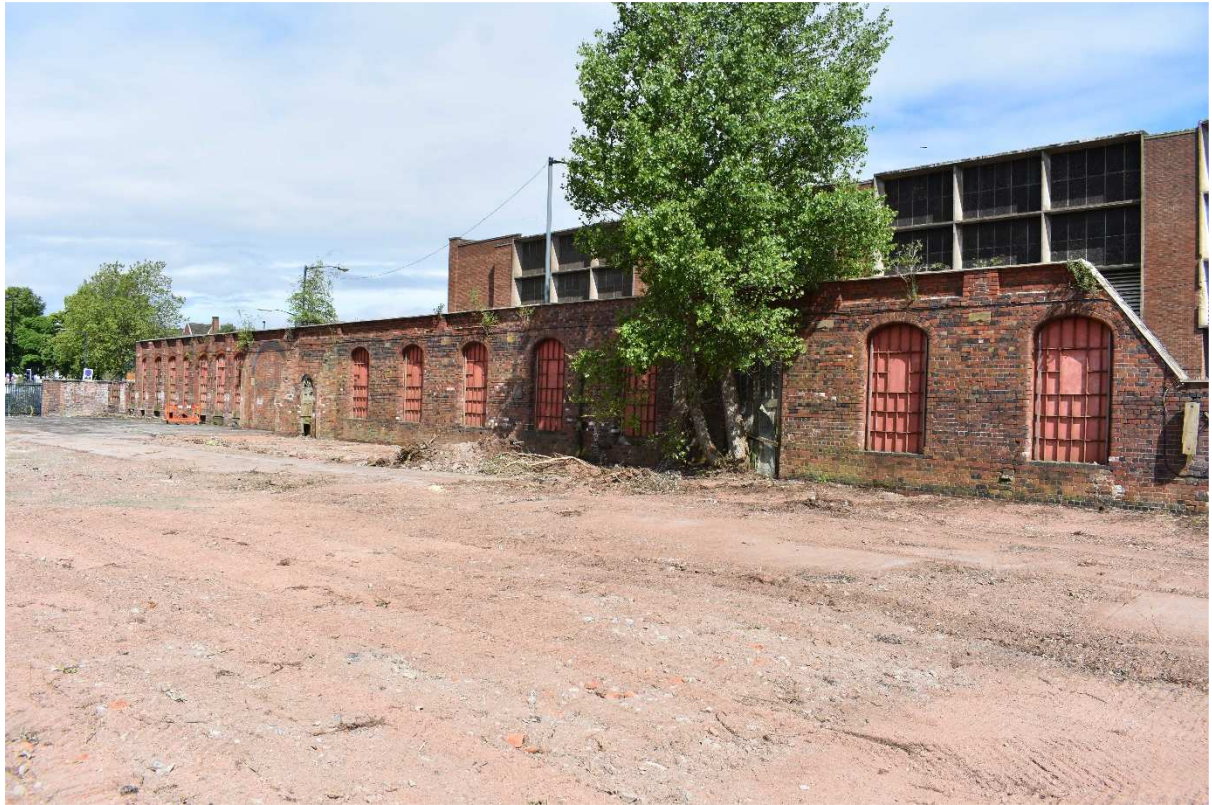
Plate 42: General view of wall looking north-west
