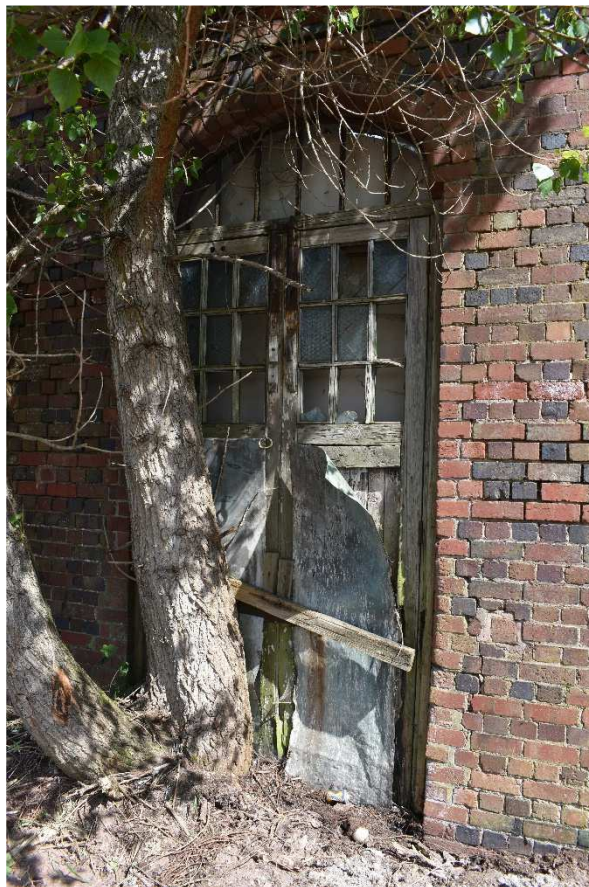
Plate 41: Former doorway in eastern part of all
