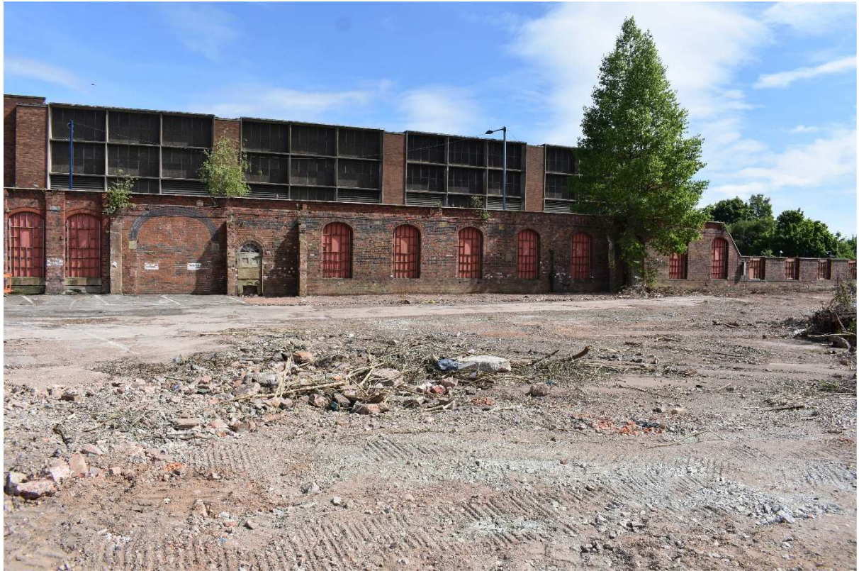
Plate 40: Eastern part of south side of wall
