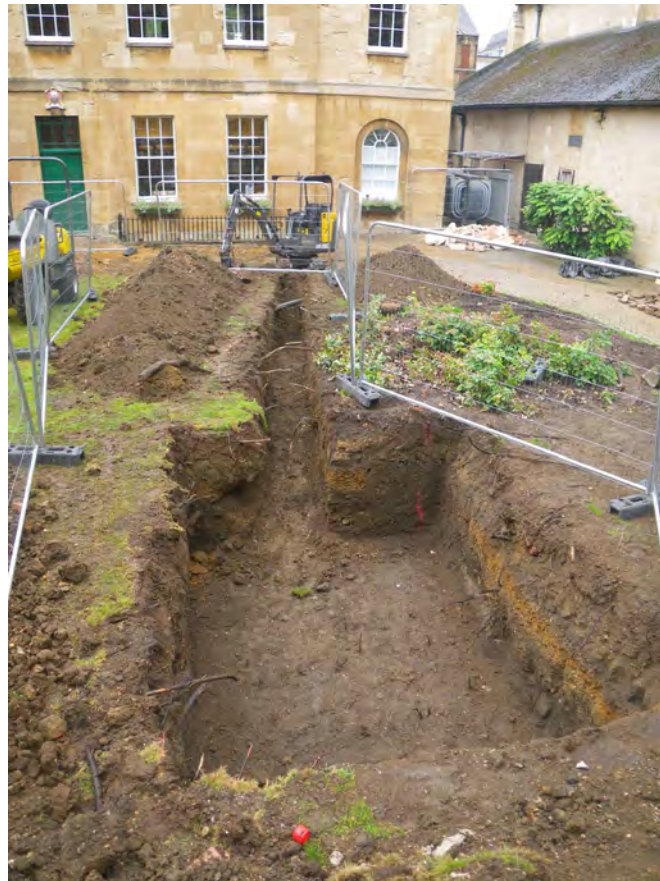
Plate 2 Soakaway and service run general shot
