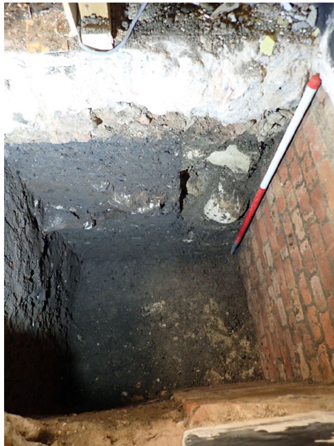
Plate 2: Test Pit 2, looking north
