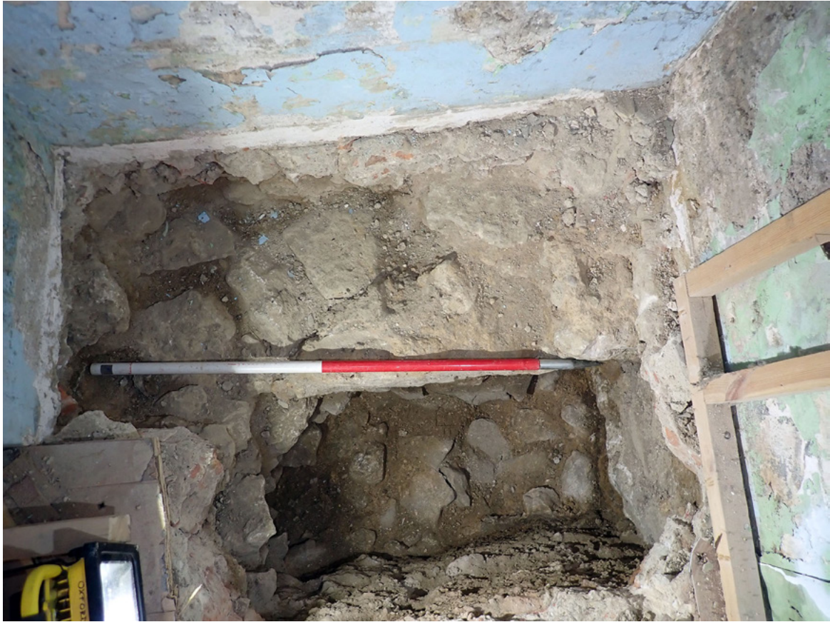
Plate 7: Test Pit 8, vertical shot of wall 800 overlying rubble core of Medieval Town Wall 804
