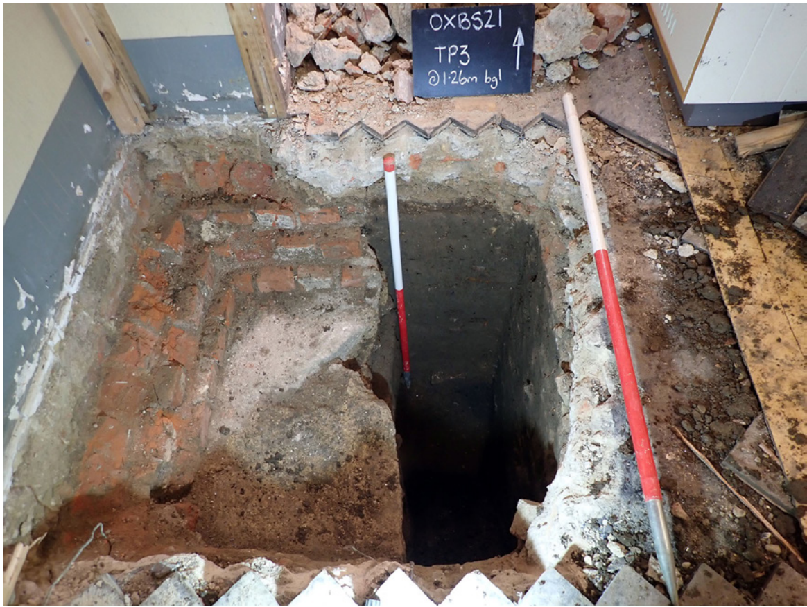
Plate 3: Test Pit 3, looking north
