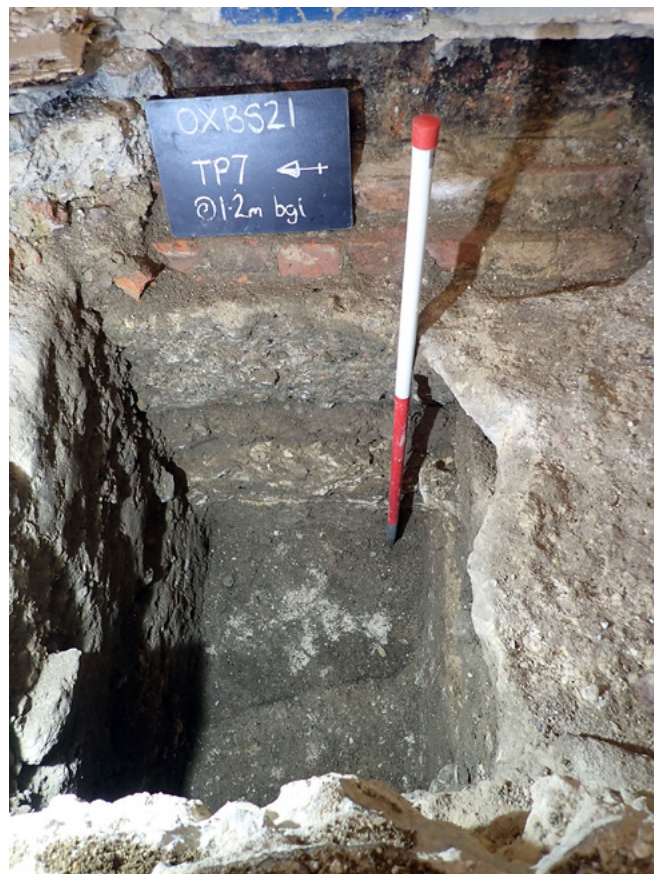
Plate 6: Test Pit 7, looking west
