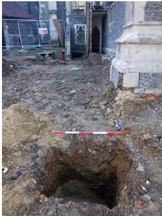
Plate 2: Test Pit 1, looking east
