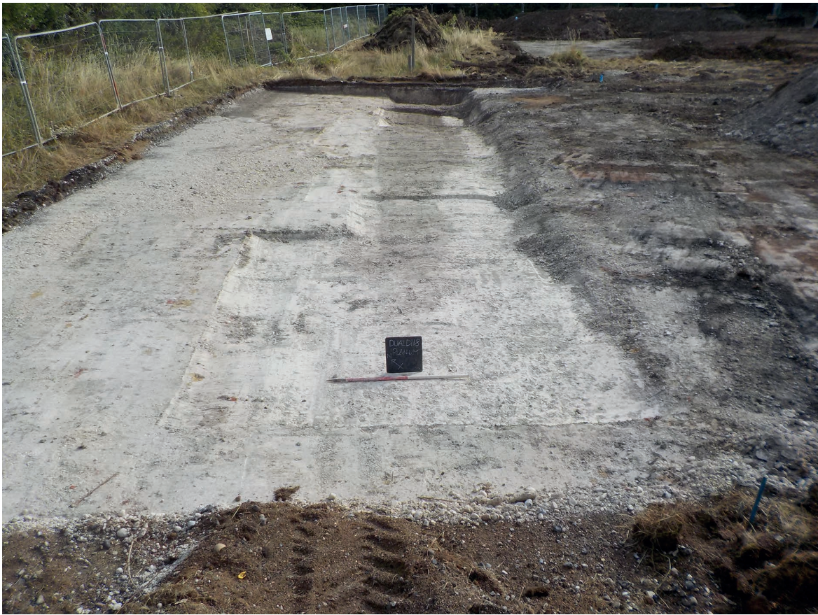
Plate 1: Attenuation tank area-strip showing ditch 1005=1013
