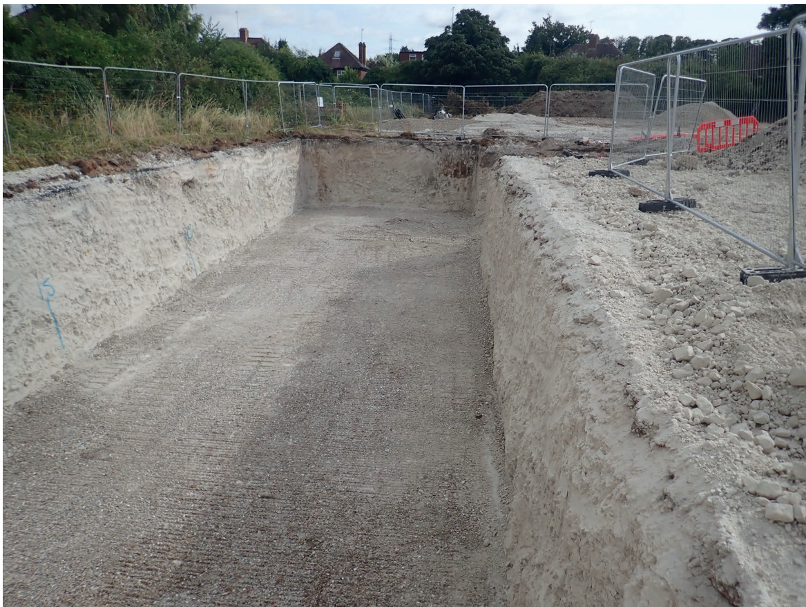
Plate 5: Attenuation tank, post-excavation
