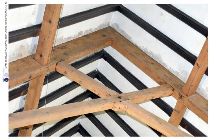
Plate 42: Detail of scissor brace roof
