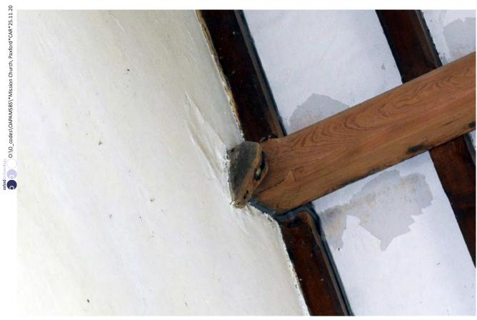
Plate 46: Pulley wheel for cord at west end of church
