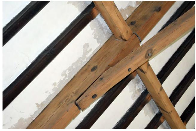
Plate 43: Detail of scissor brace roof
