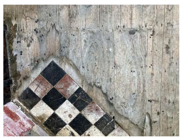
Plate 64: Small section of surviving primary floorboards by fireplace hearth (photo provided by Geoff Bolam)
