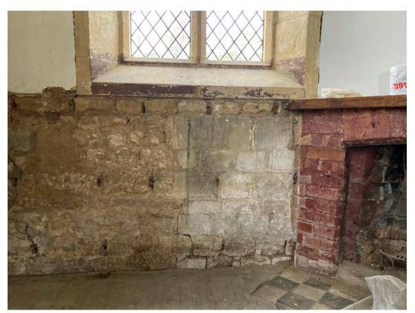
Plate 66: North wall of school room after removal of boarding (photo provided by Geoff Bolam)
