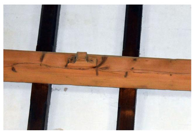
Plate 45: Detail of guide bearer for cord fixed to purlin
