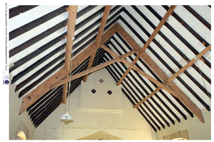
Plate 40: Scissor brace roof looking east
