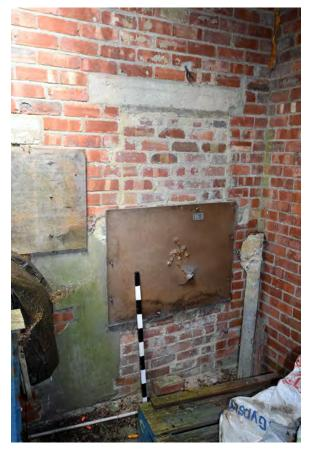
Plate 36: Blocked doorway at east end of north wall in Building 5
