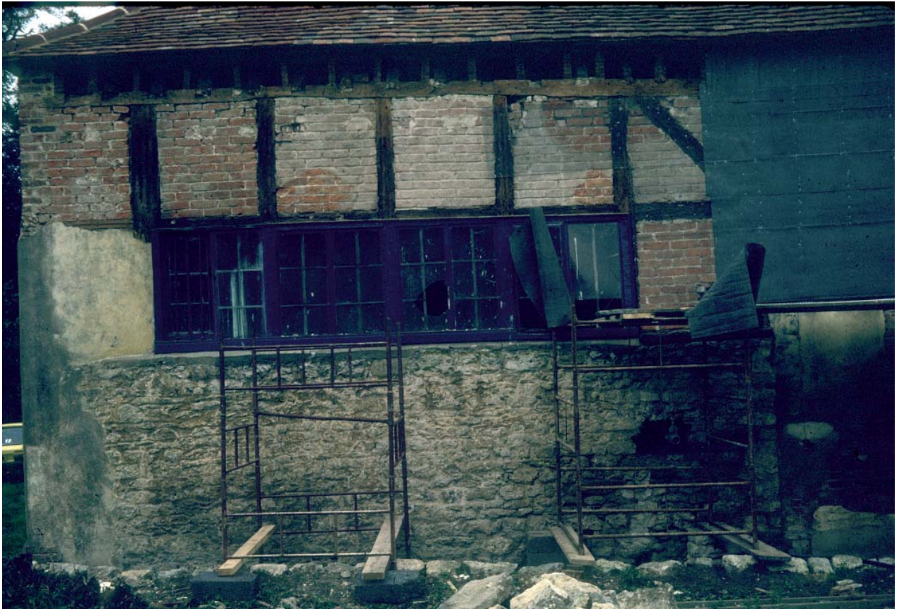
Plate 3: Exposed frame at south end of east elevation during 1980s works (courtesy of Julian Munby)
