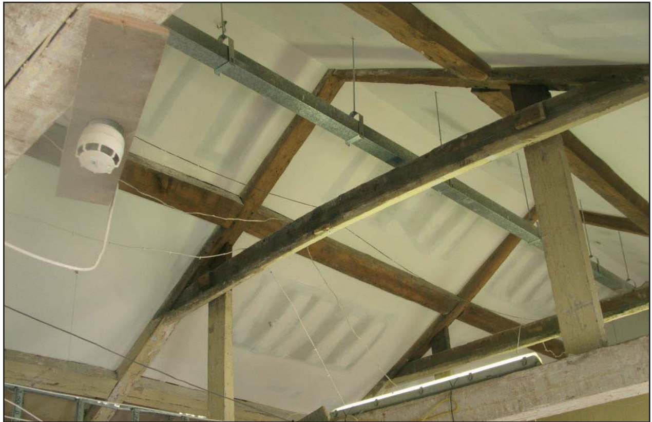
Plate 12: Typical open roof truss (west face of truss 11)
