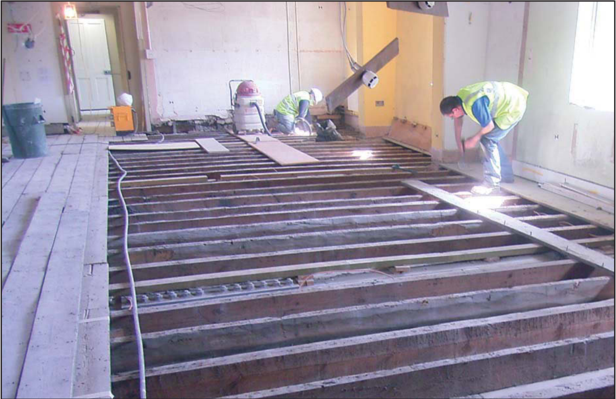
Plate 9: First floor joists on south side of east barrack room
