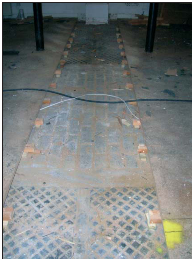
Plate 14: Stable floor view NE, see figure 26
