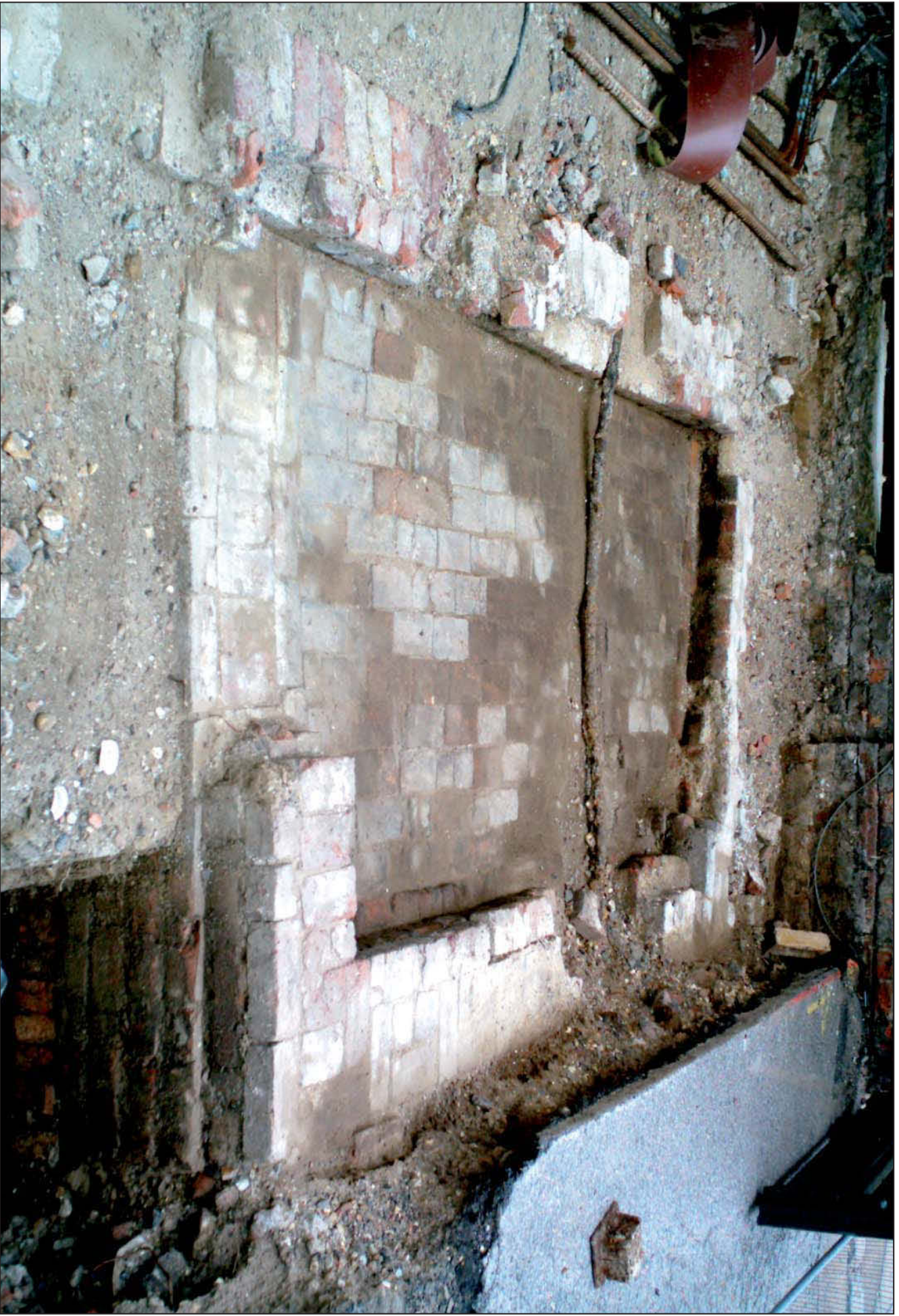
Figure 14: Soil pit 1070, looking South
