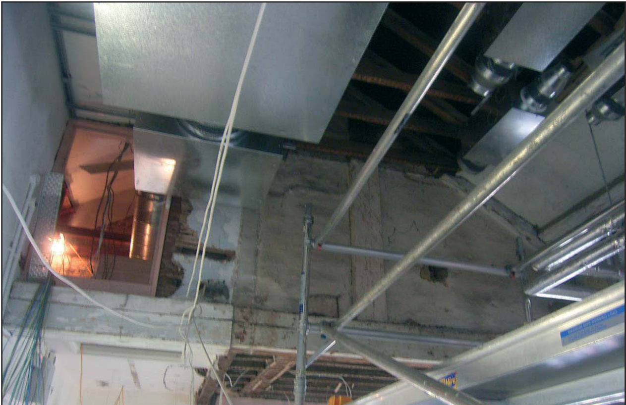
Plate 10: East elevation of closed truss (truss 2) with primary stairwell ceiling joists behind
