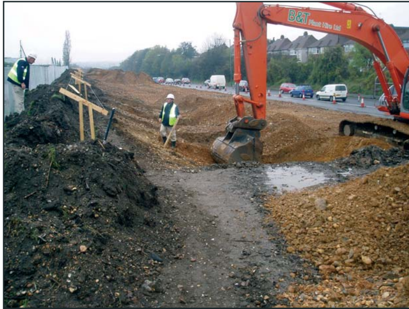
Plate 1: Groundworks in progress
