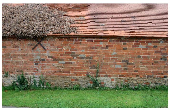
Plate 8 Signs of repair to the plinth of the west elevation
