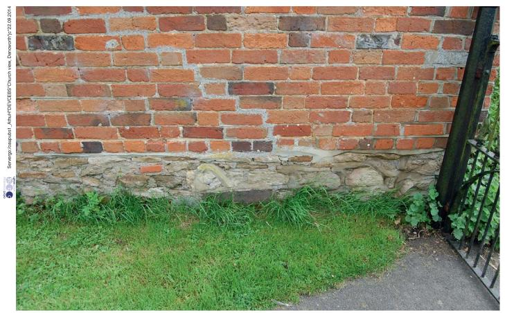
Plate 9 Repaired cracking in the west elevation
