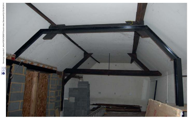
Plate 21 Structural steel frame in the store room
