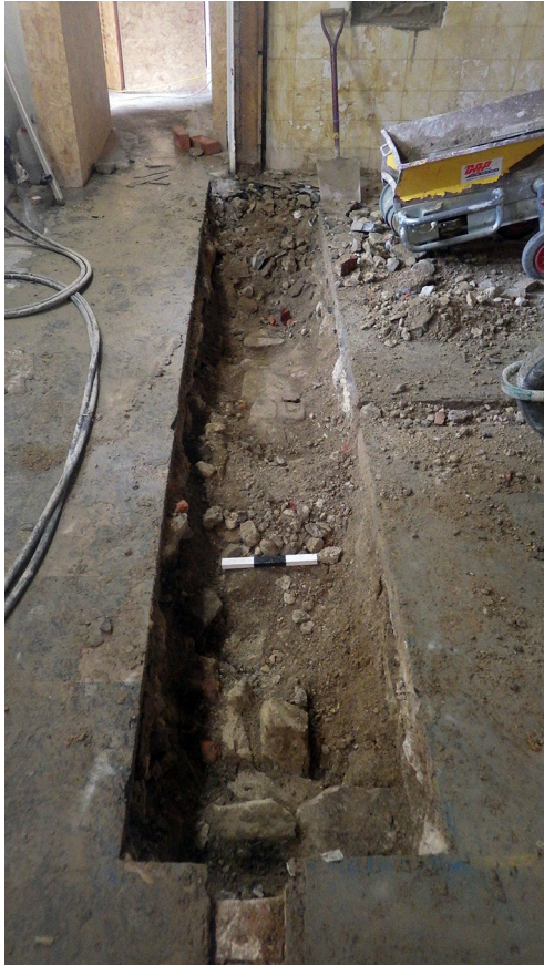
Plate 1: Wall 400, looking north
