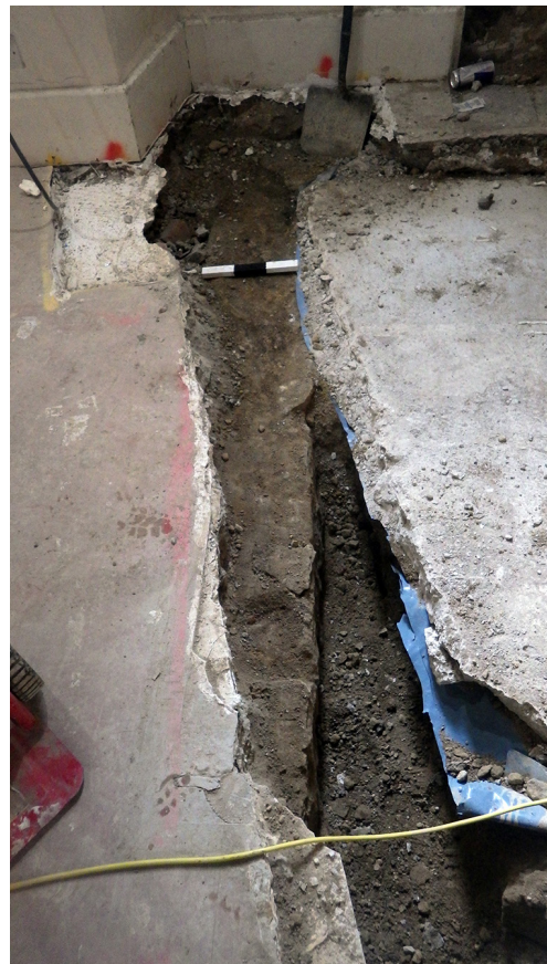
Plate 4: Wall 404, looking north
