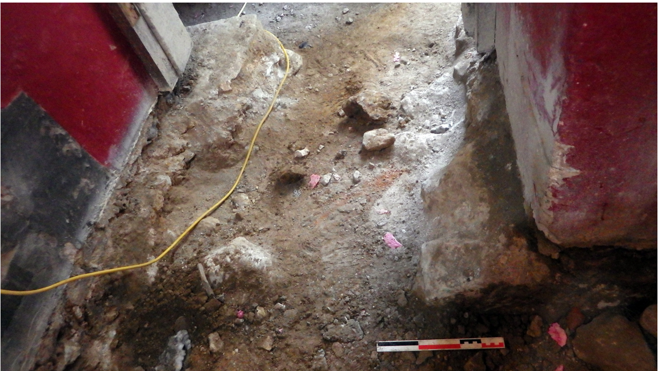
Plate 6: Wall foundation 406, looking south
