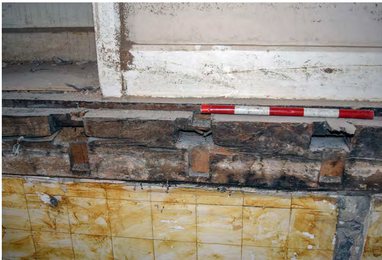
Plate 62: Primary first floor joist at north end of Chaplains III
