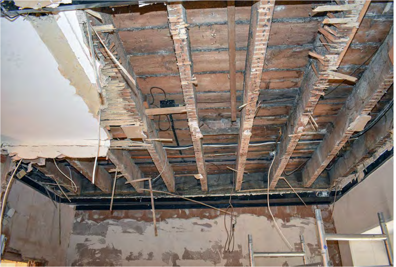
Plate 66: Underside of first floor joists in Chaplains III
