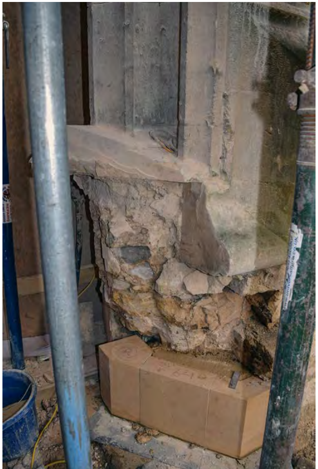
Plate 51: Works to doorway in South Range of Great Quad
