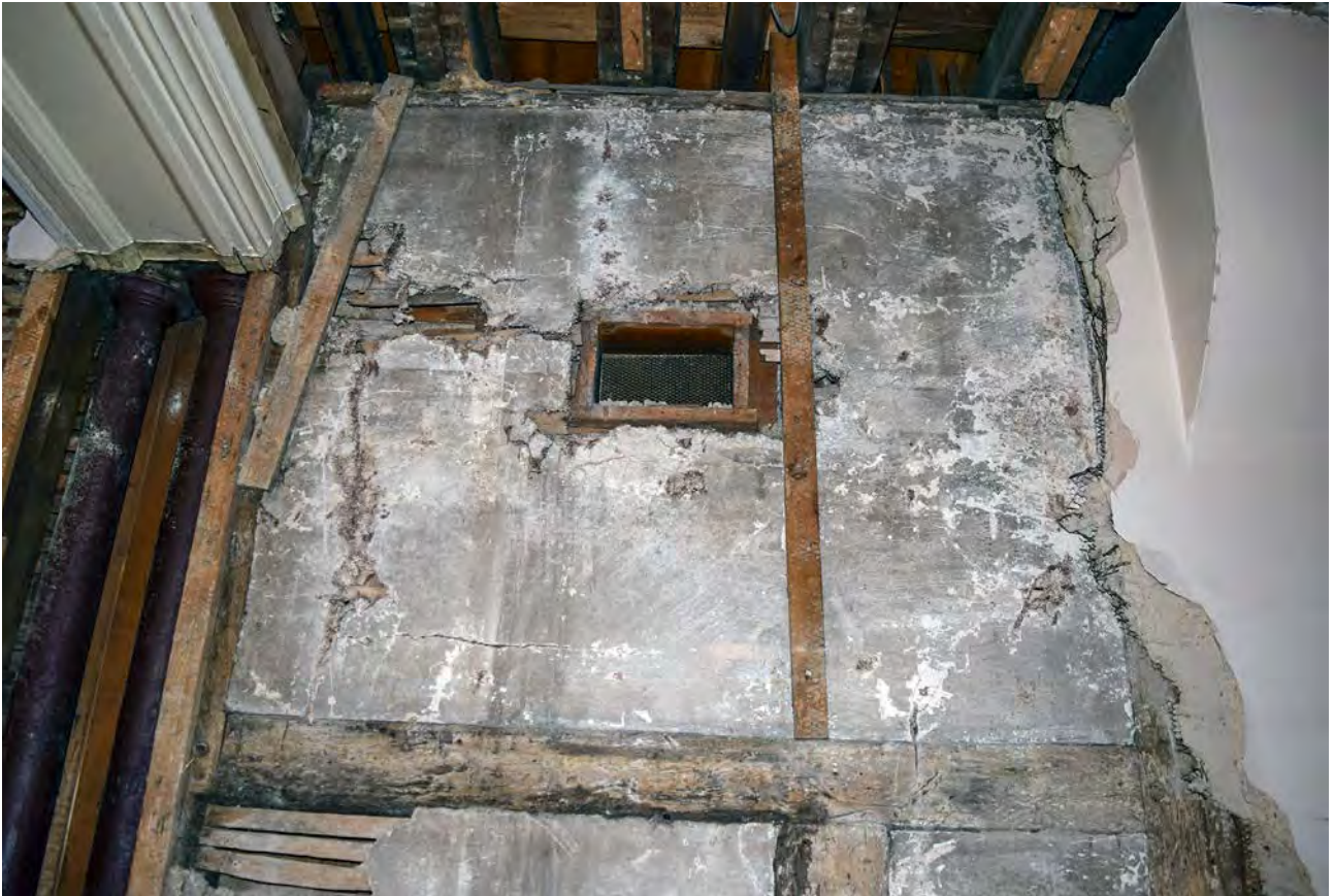
Plate 18: 16th century frame exposed on north side of Old Bursary
