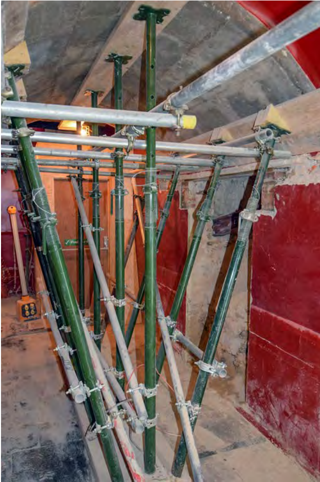
Plate 38: Passage during works to form doorway in east wall
