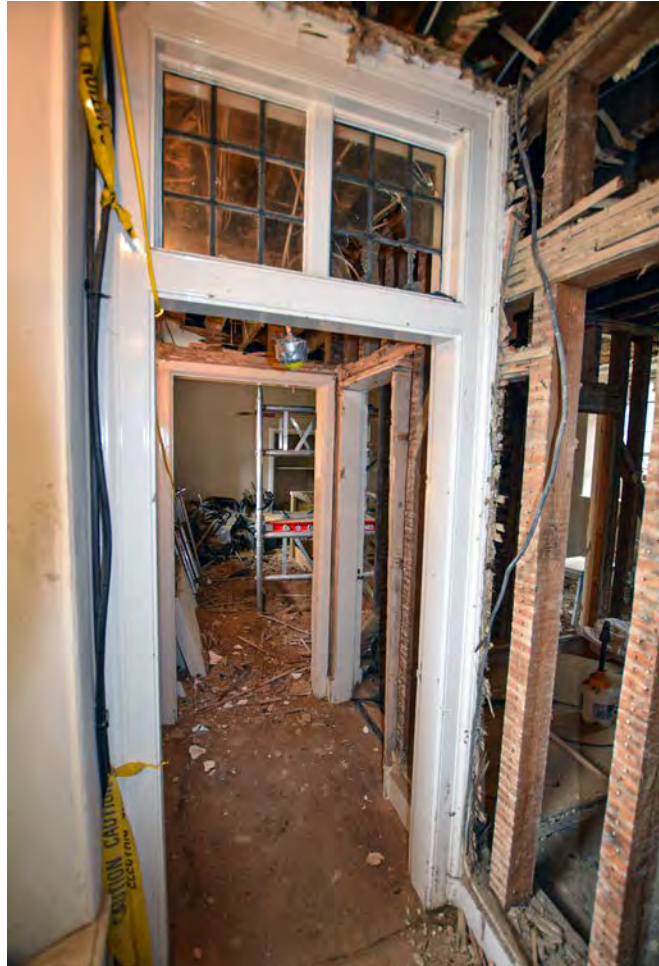
Plate 91: Exposed frame of corridor lobby at first floor of Chaplains III
