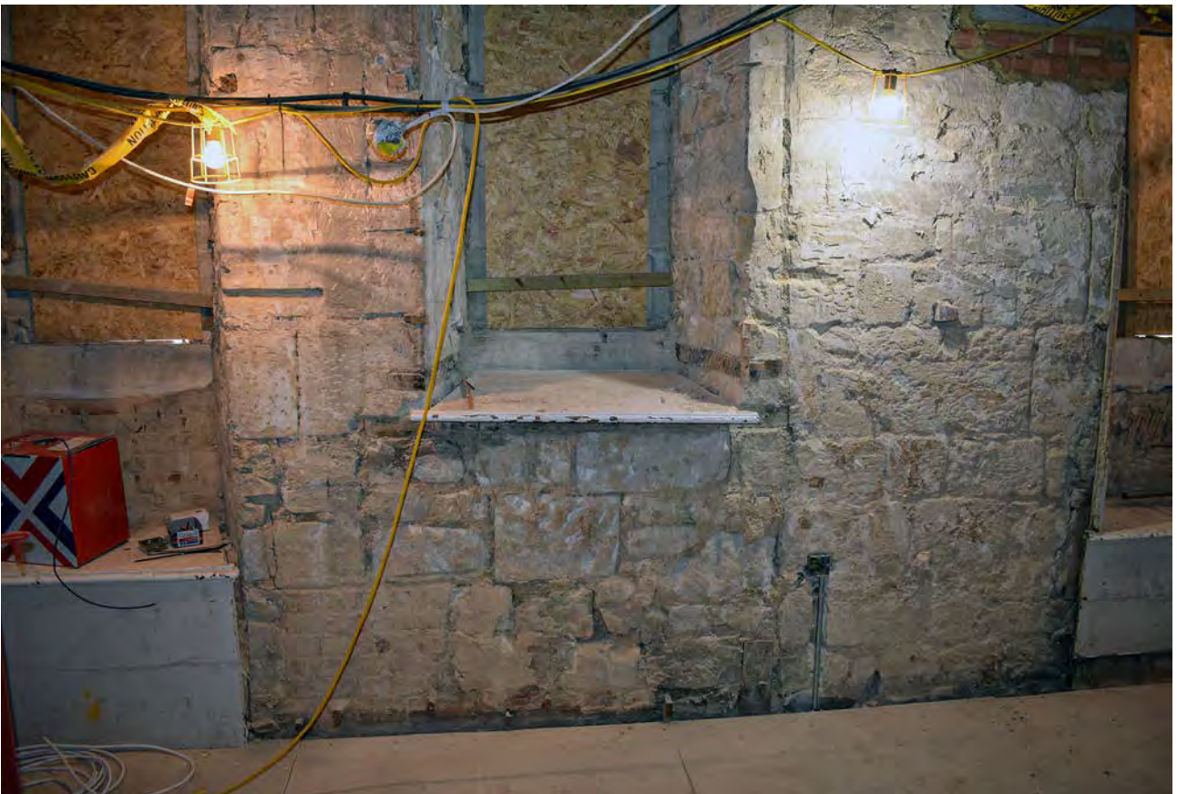
Plate 106: Part of west wall at first floor of Chaplains III
