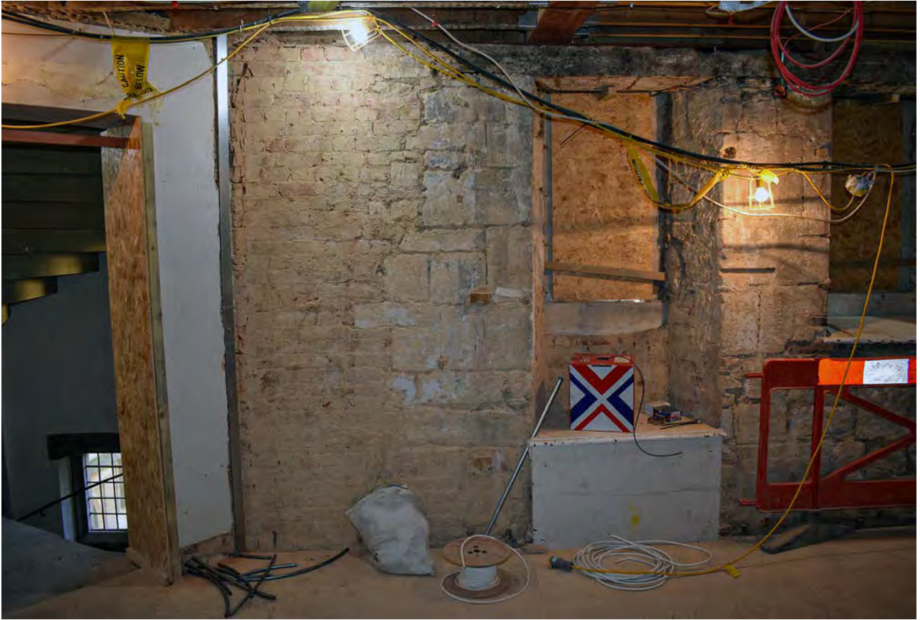
Plate 101: Part of exposed west wall of Chaplains III by staircase
