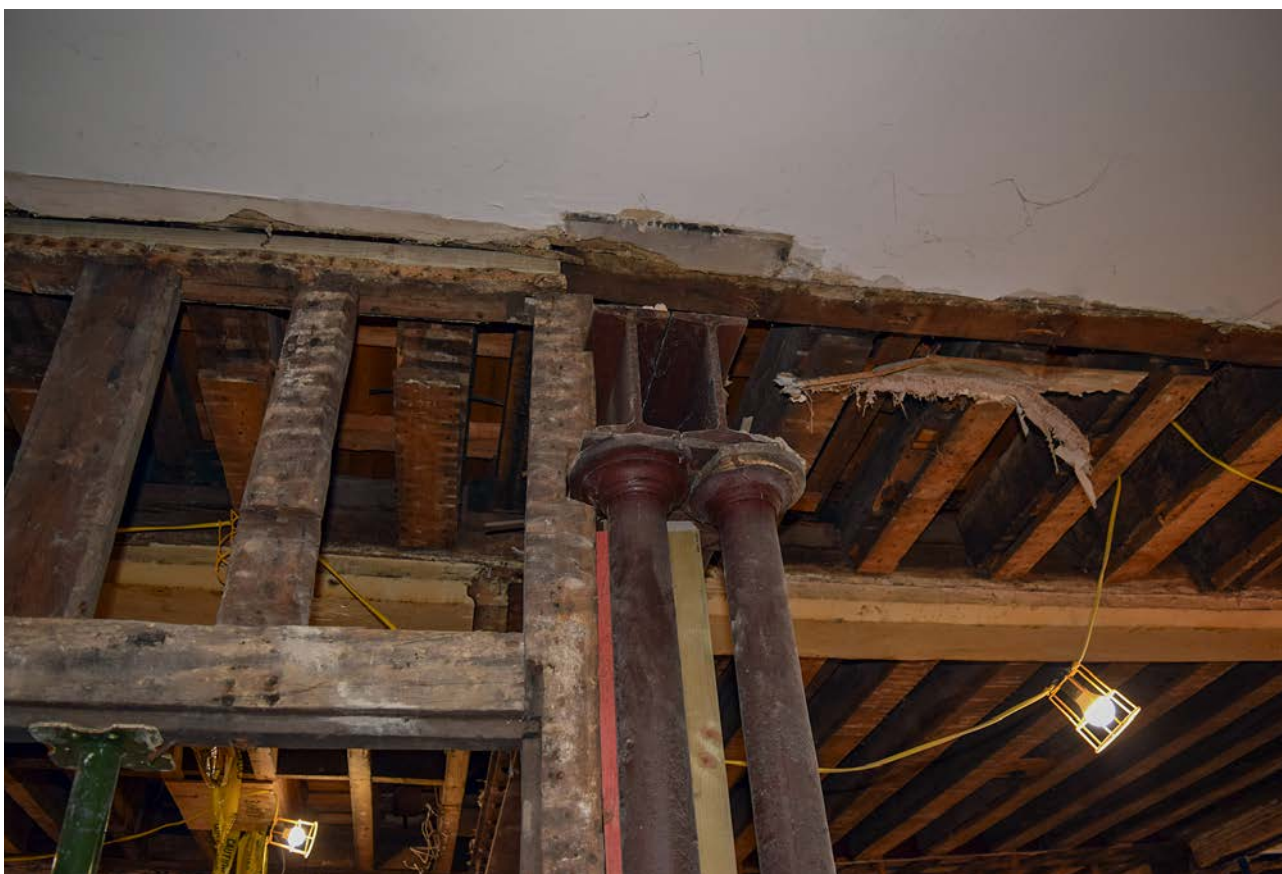
Plate 24: Cast iron columns inserted in 1950s
