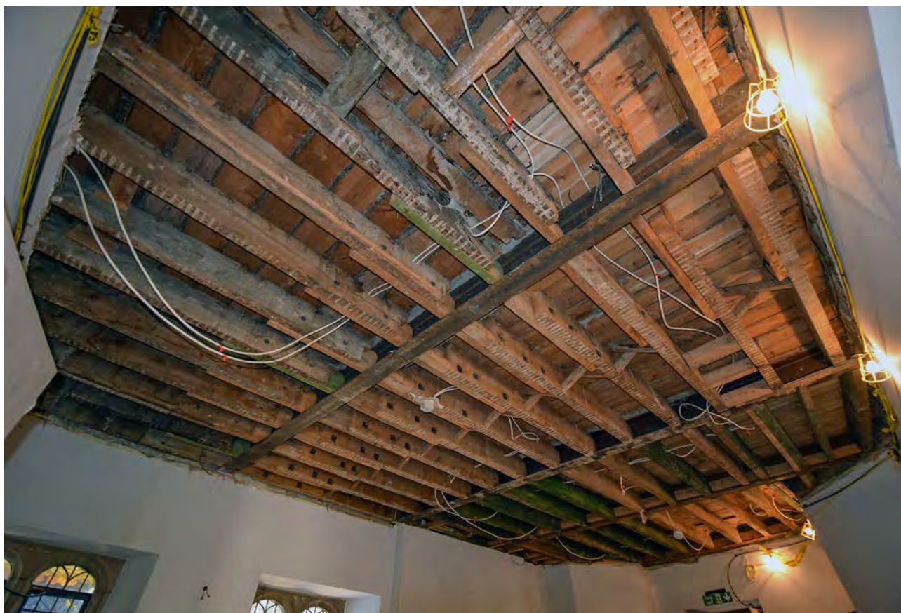
Plate 63: Underside of first floor above Ante Room
