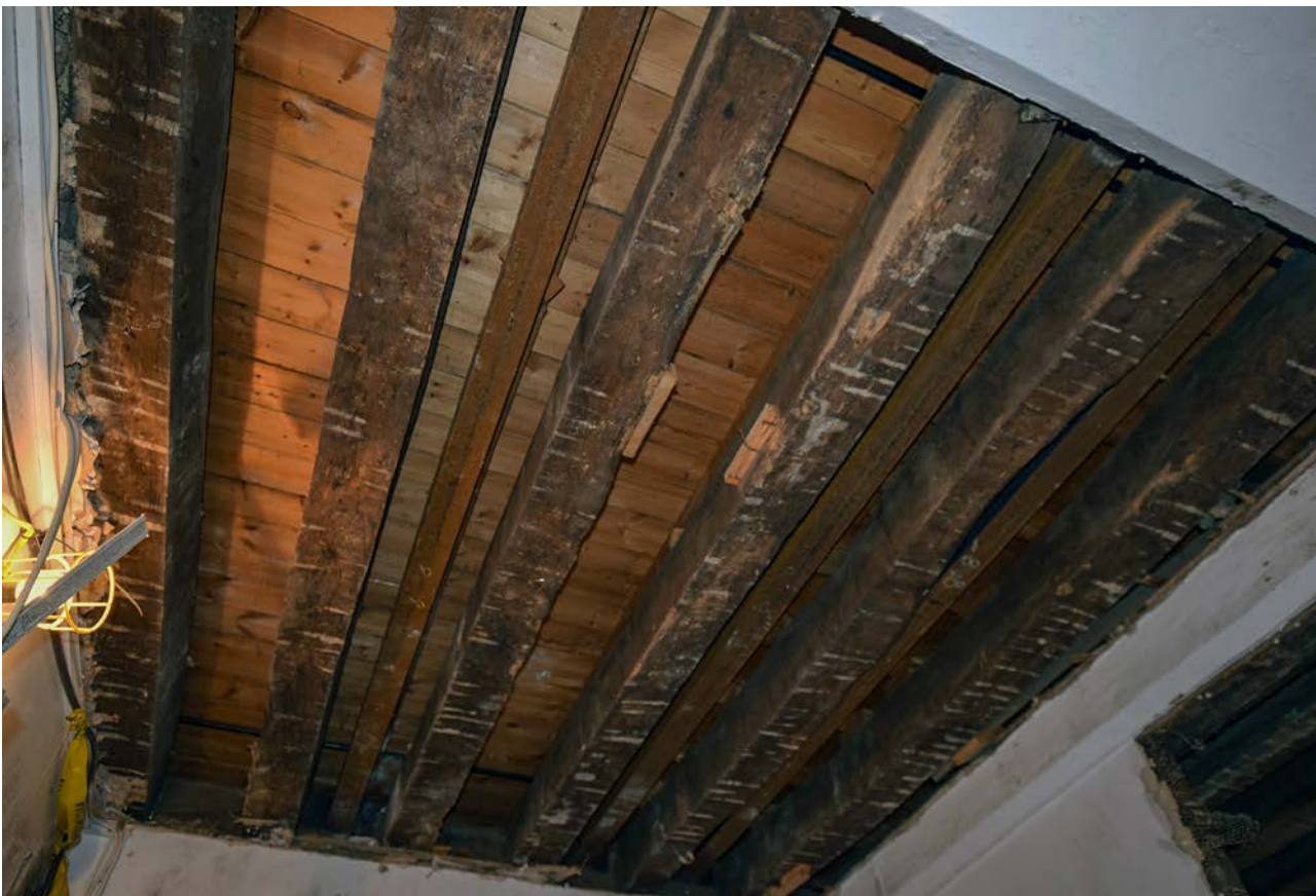
Plate 29: Exposed floor in Linen/Crockery Store
