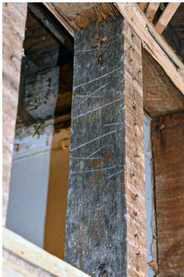
Plate 94: Baltic timber marks to first floor frame
