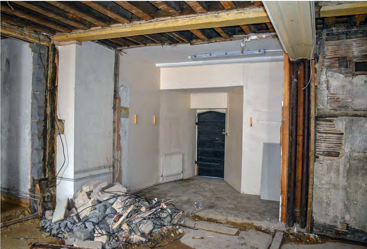
Plate 32: Old Bursary looking north after removal of partition
