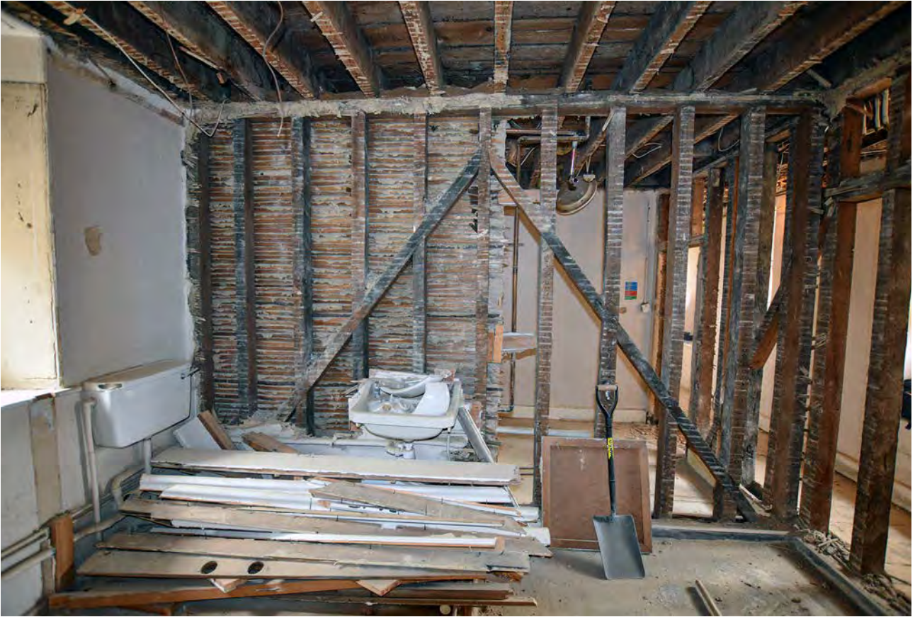
Plate 87: Exposed partition in first floor of Chaplains III
