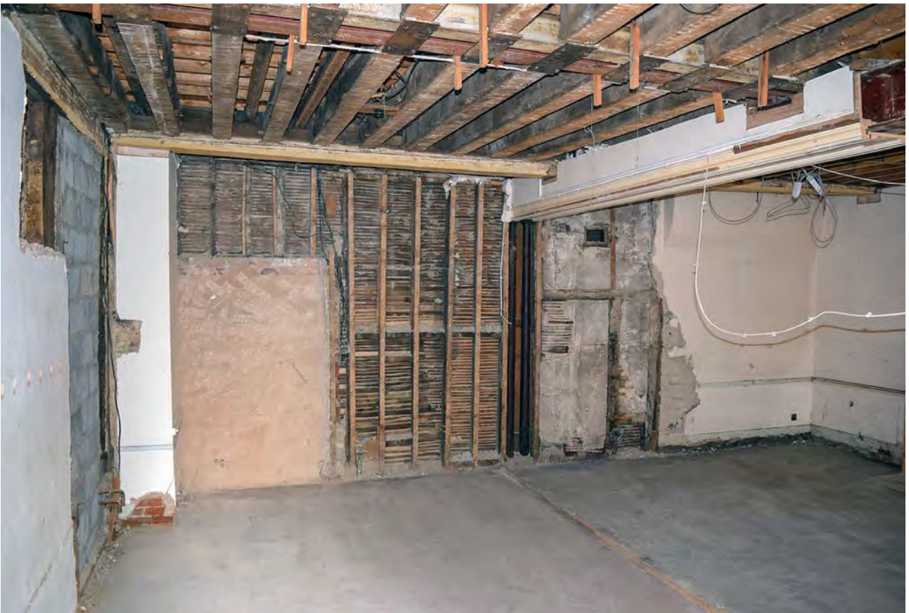
Plate 16: North side of Old Bursary area during works
