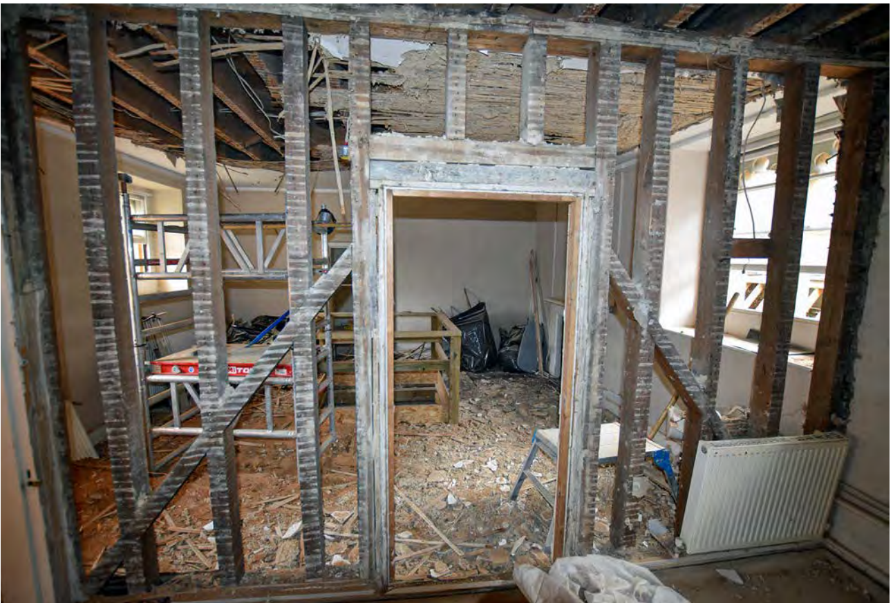
Plate 90: Exposed partition towards north end of Chaplains III
