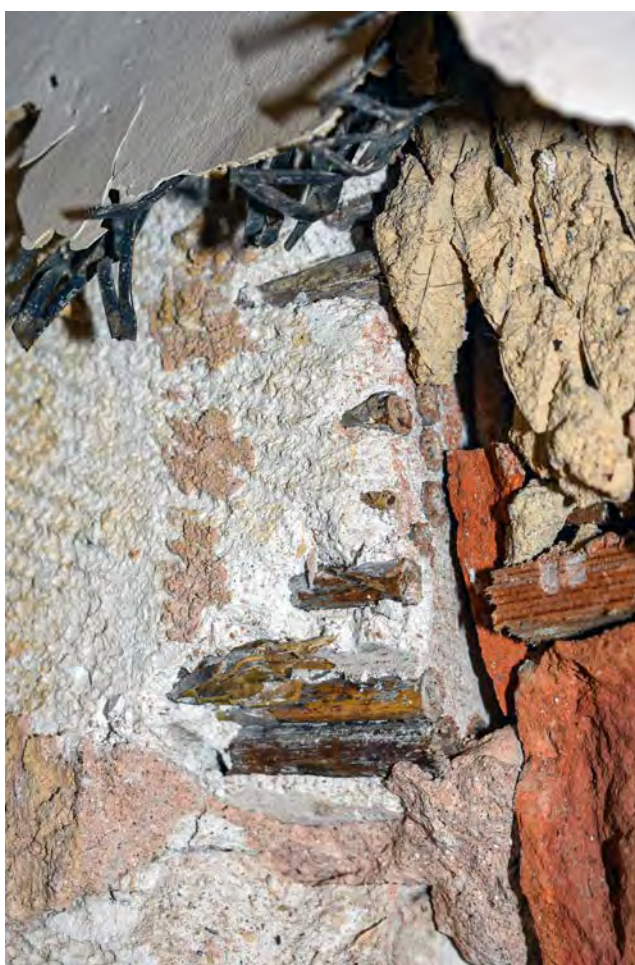
Plate 98: Detail of plaster block partition with reeds
