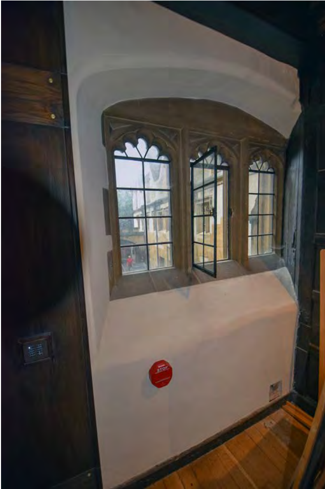
Plate 48: Internal view of window in south wall of Hall
