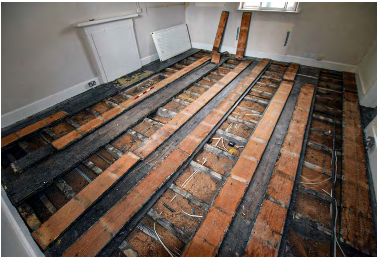
Plate 111: Exposed second floor at north end of Chaplains III
