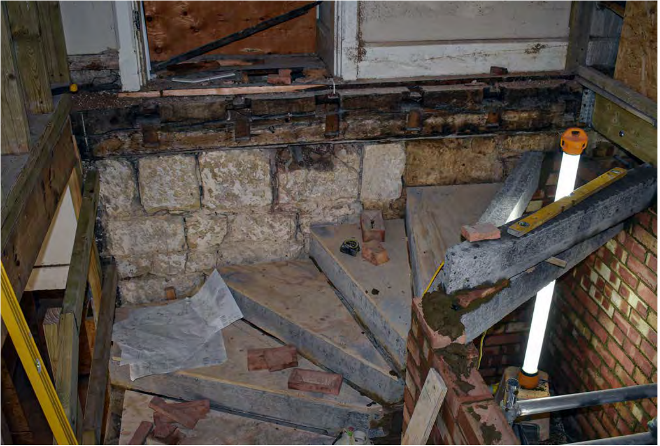
Plate 103: New stairs being constructed at north end of first floor
