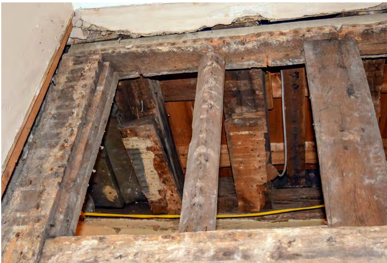
Plate 23: Upper part of 16th-century frame after removal of plaster
