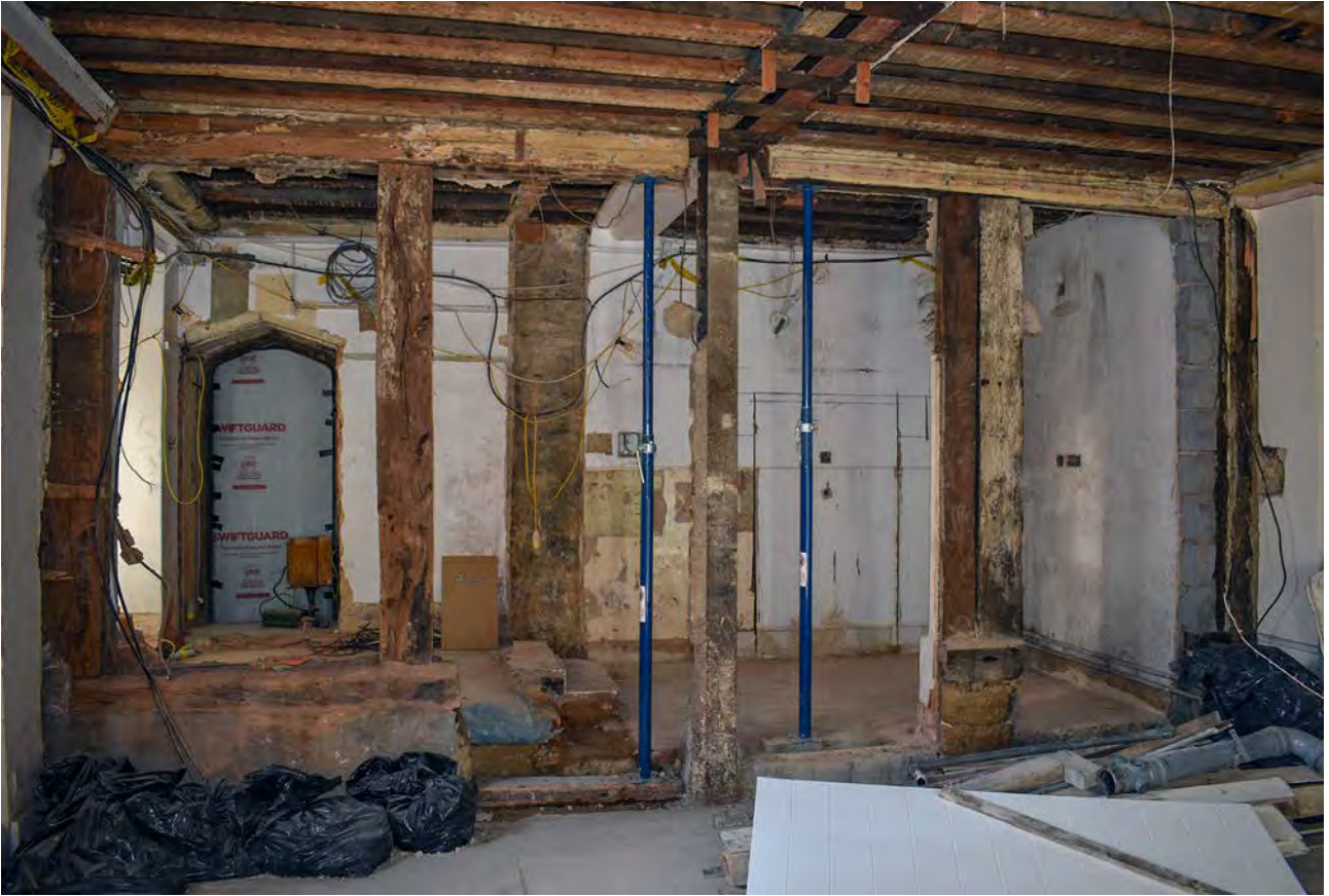
Plate 13: Partition on west side of Old Bursary after removal of infill
