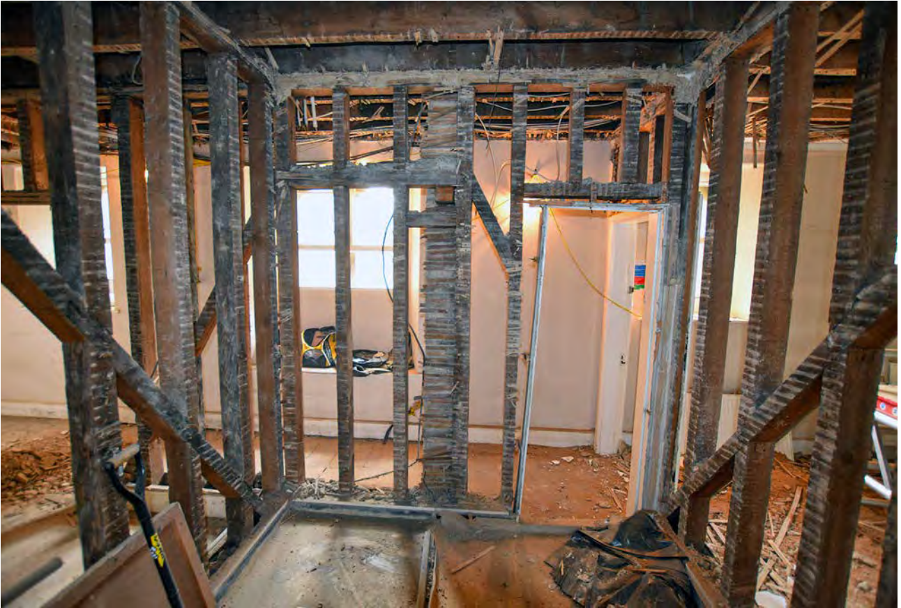
Plate 89: Exposed first floor partition with inserted doorway
