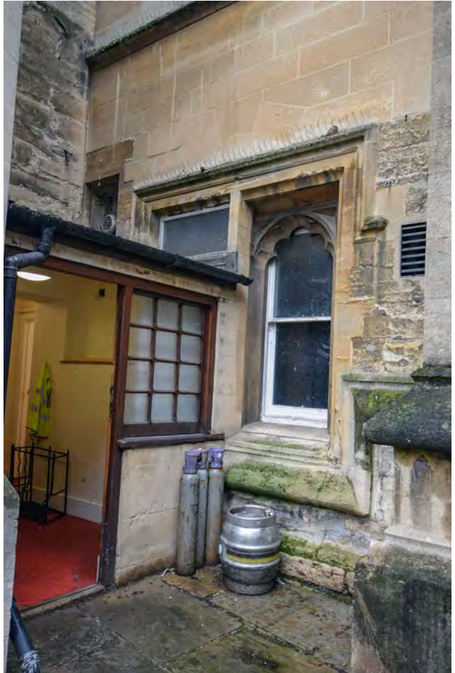
Plate 49: Lobby between Chaplains III and south side of Great Quad
