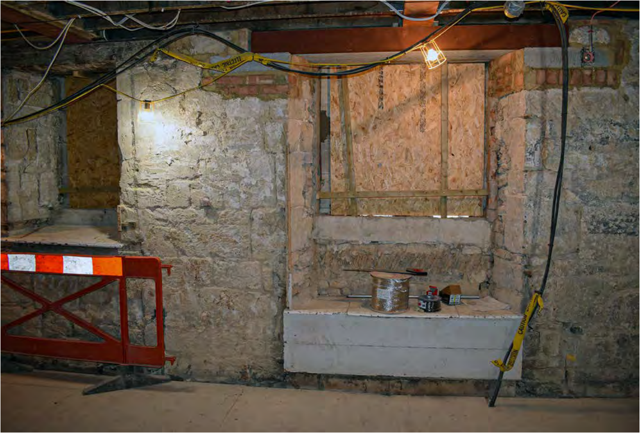
Plate 105: Part of west wall at first floor of Chaplains III
