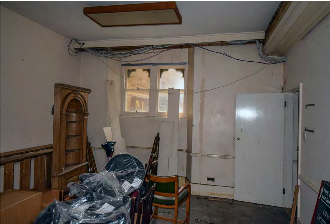
Plate 4: Store in Old Bursary area prior to work looking south
