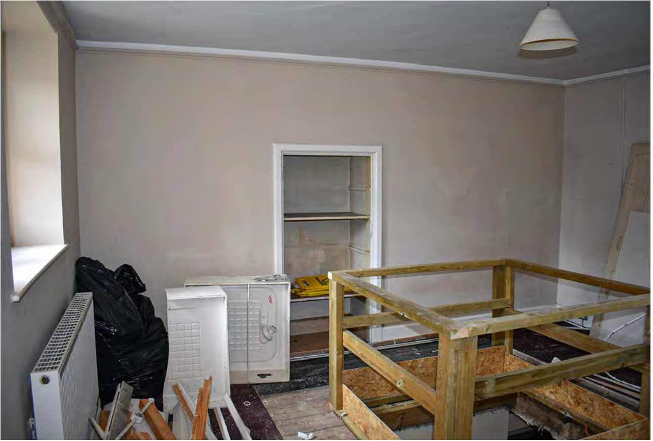
Plate 85: Room at north end of first floor of Chaplains III
