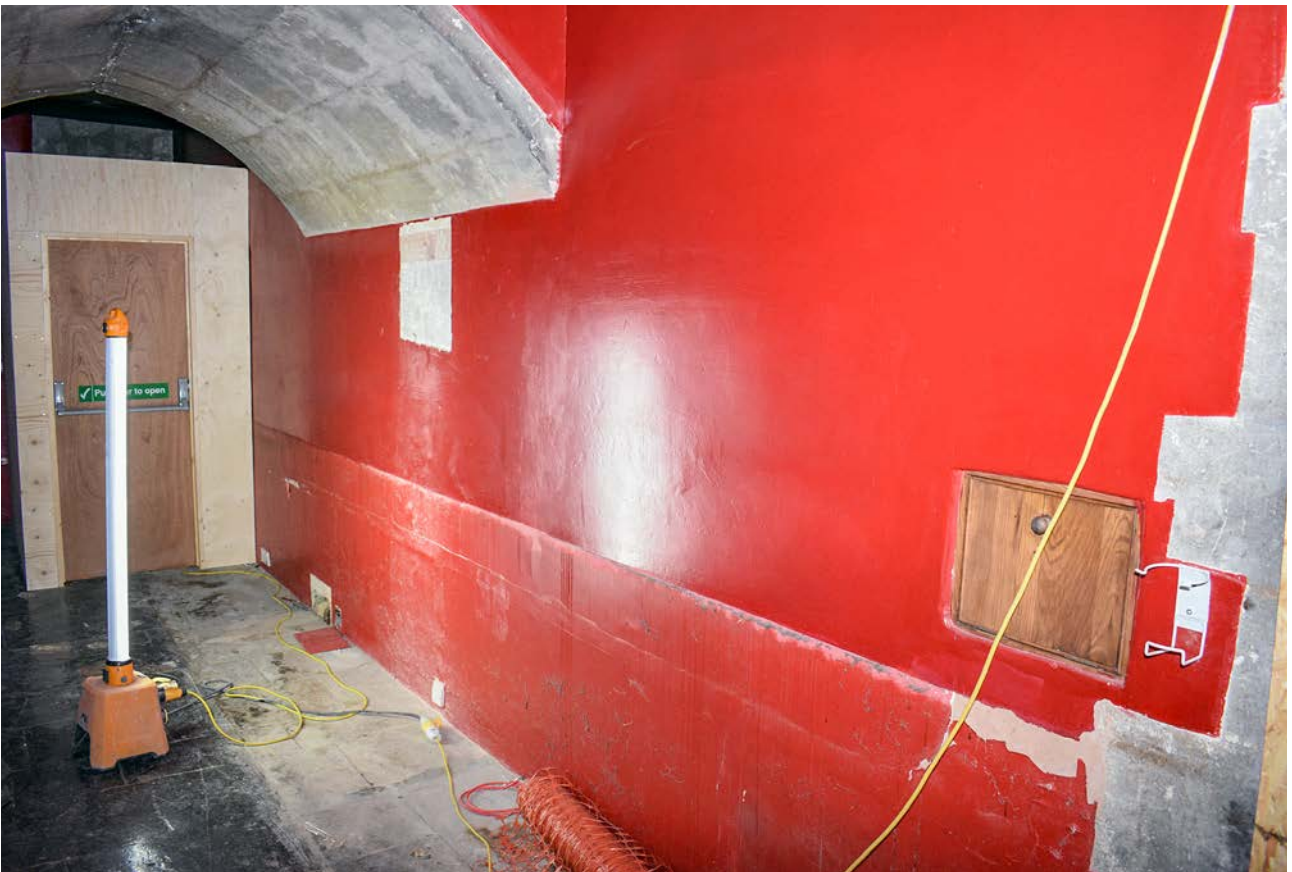
Plate 37: Passage after removal of servery
