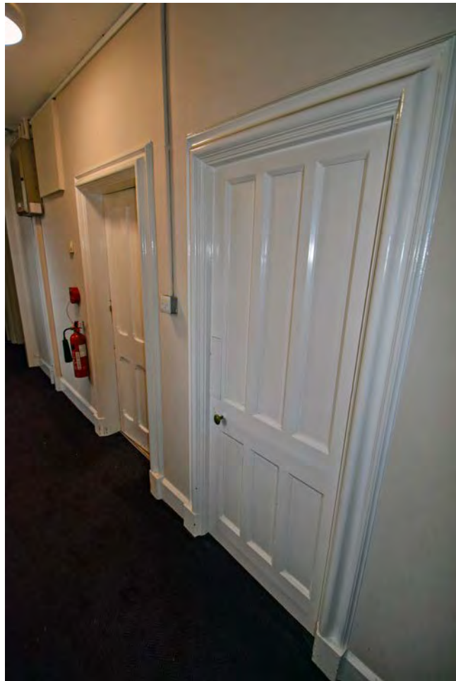
Plate 83: Doors at first floor level in Chaplains III
