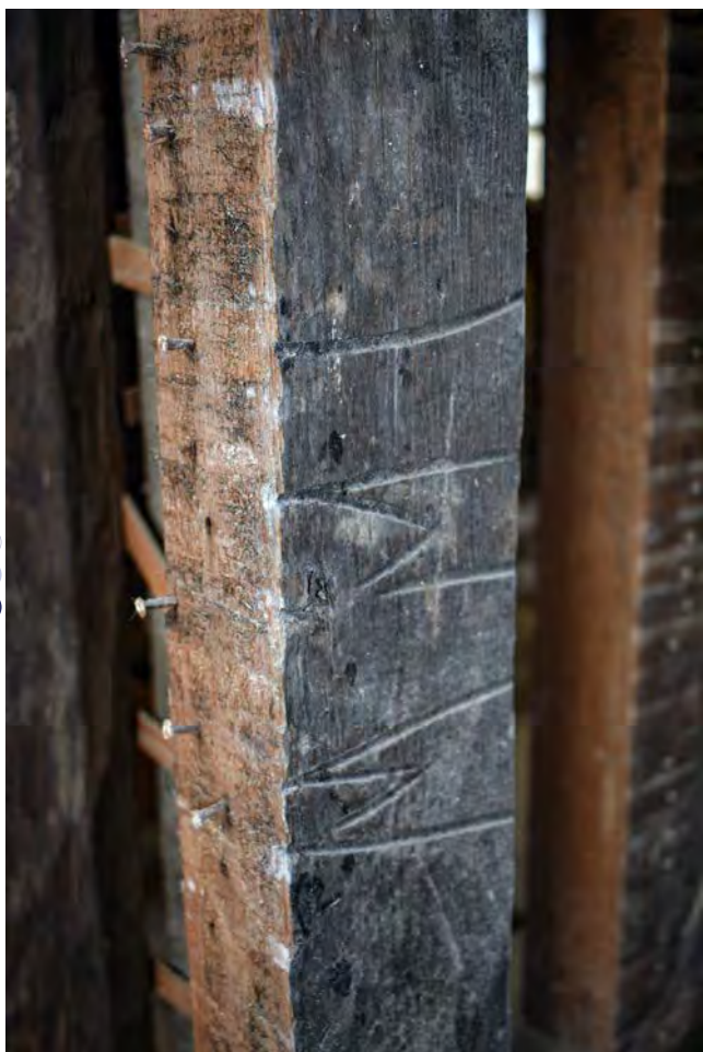
Plate 93: Baltic timber marks to first floor frame
