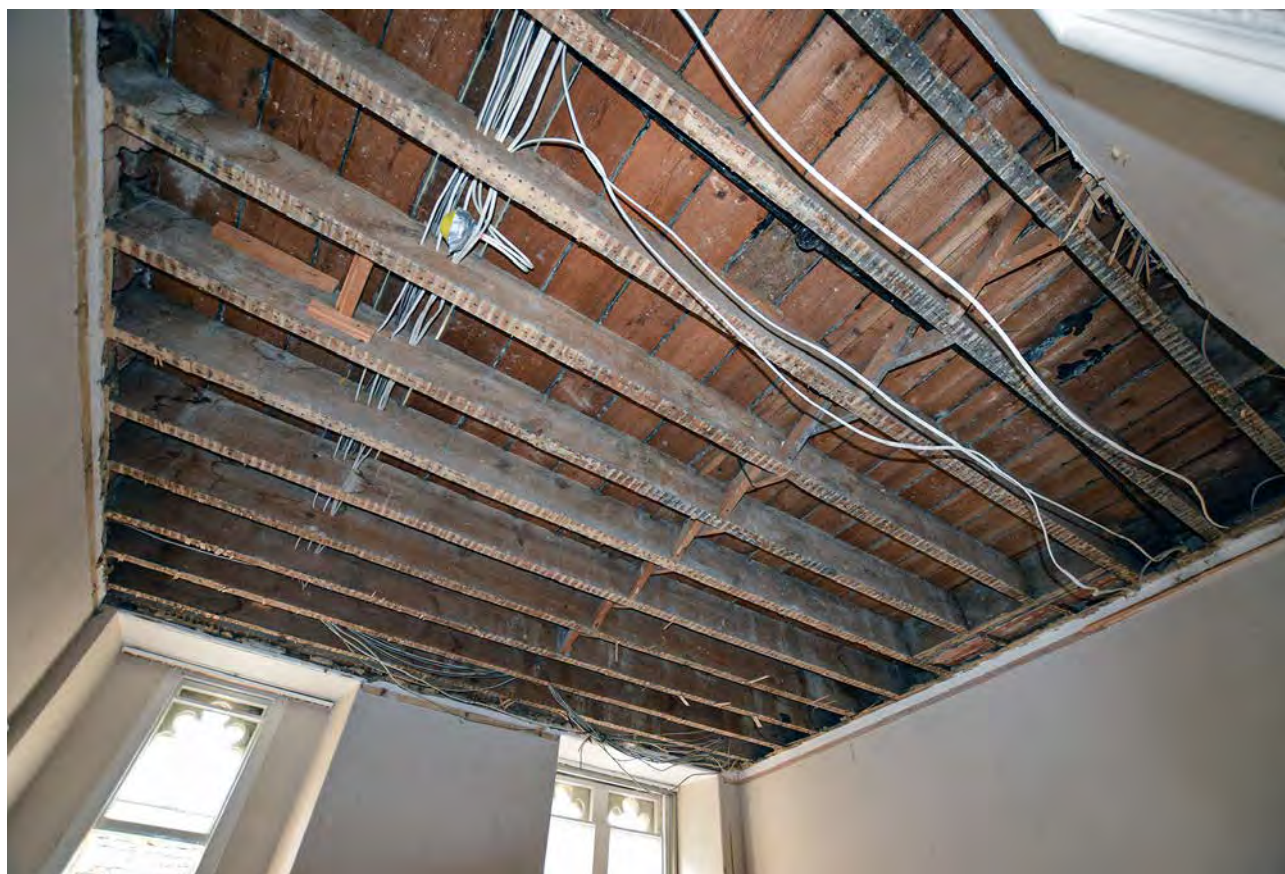
Plate 95: Underside of second floor ceiling in Chaplains III
