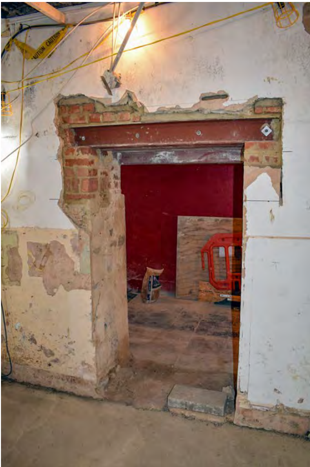
Plate 40: New doorway created in east wall of passage
