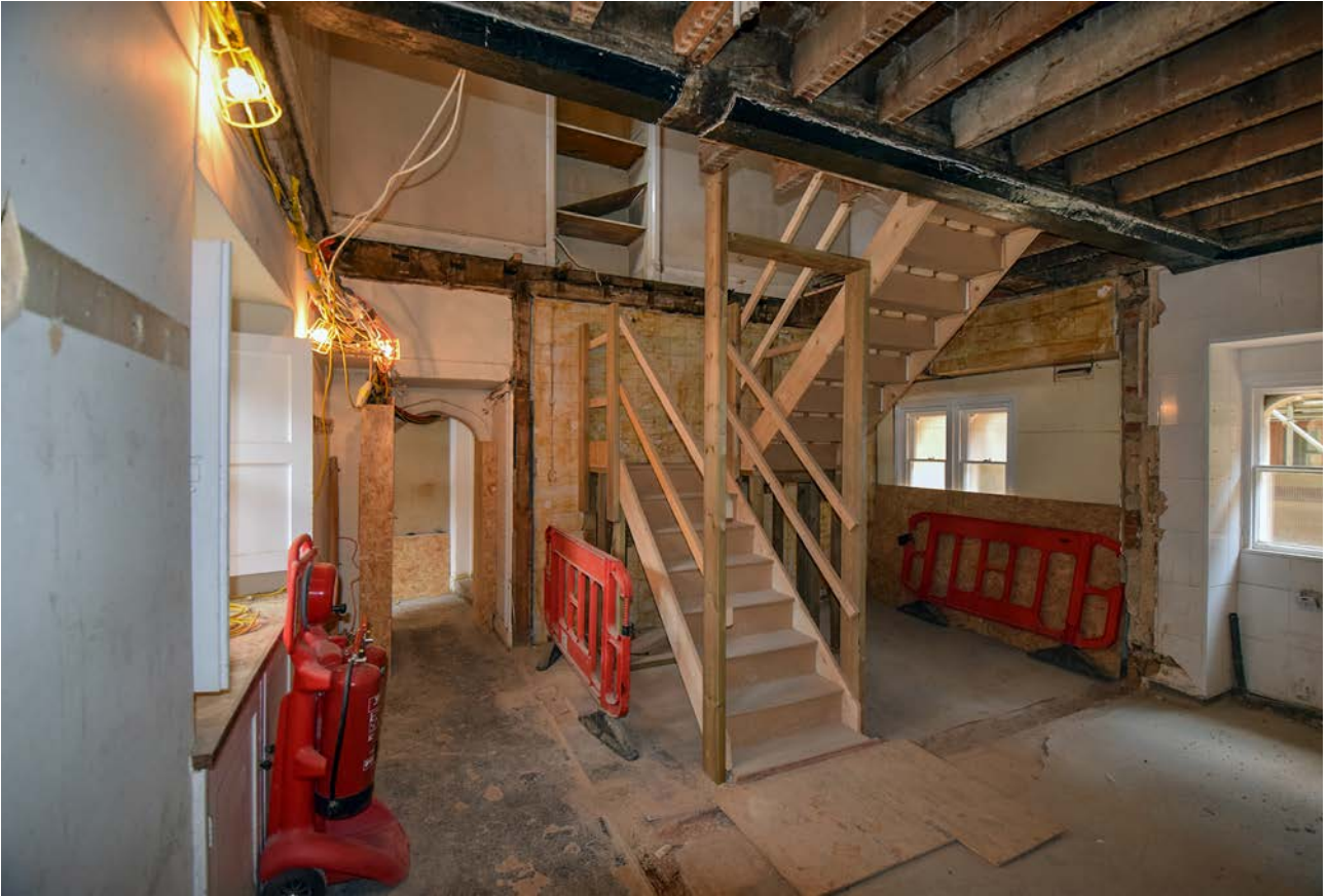
Plate 60: Temporary stairs during works in Chaplains III
