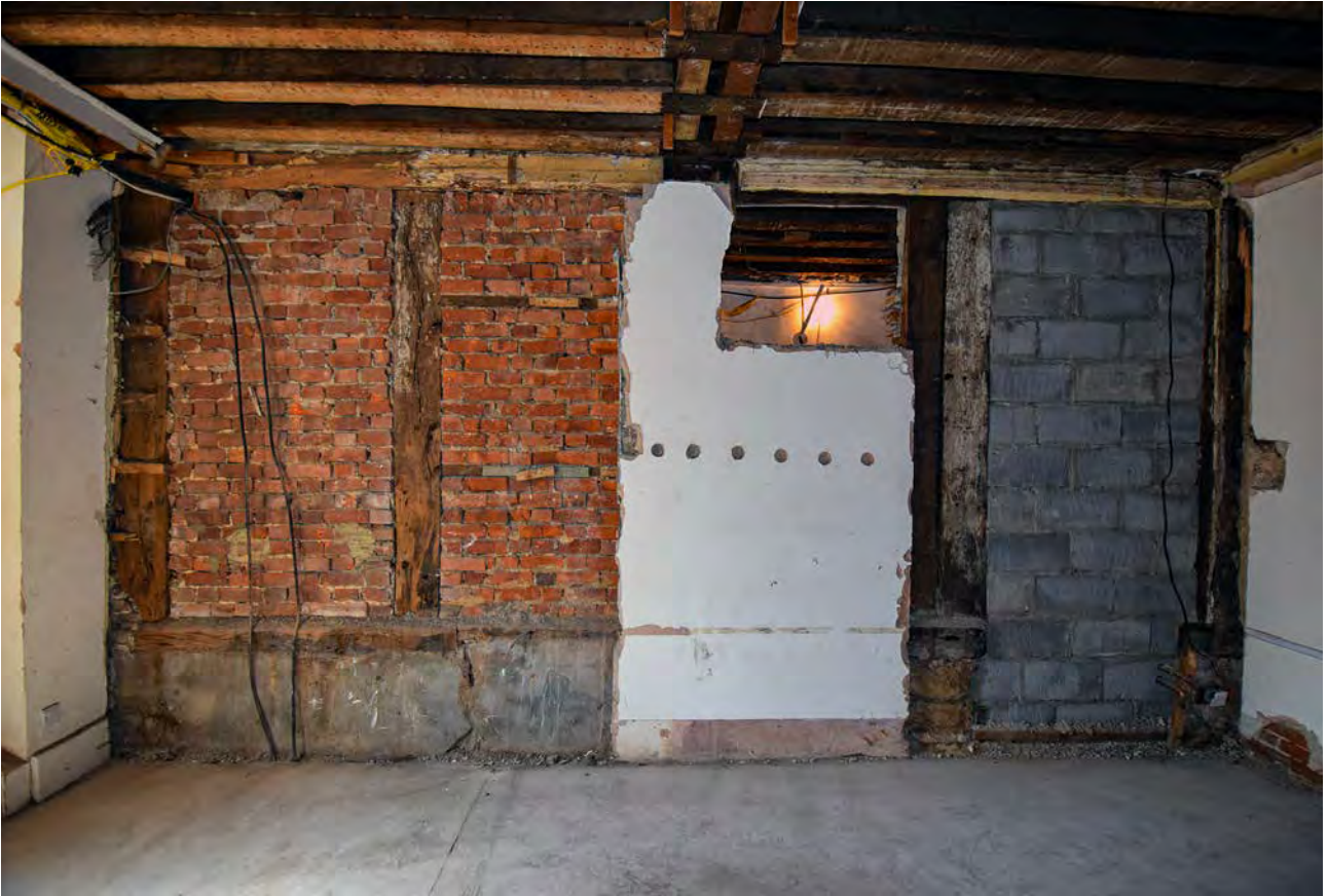
Plate 7: Exposed frame in west wall of Old Bursary
