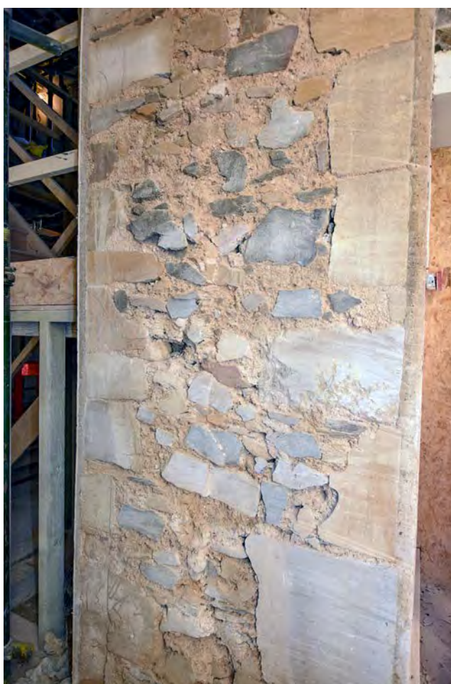
Plate 70: Jamb of new doorway created in north wall of Chaplains III
