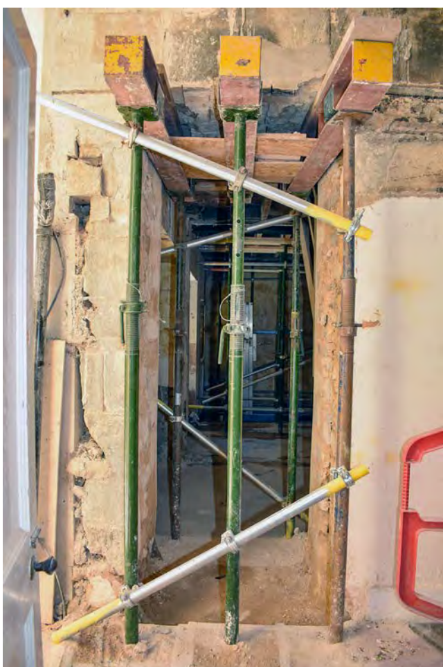
Plate 69: Doorway created in north wall of Chaplains III
