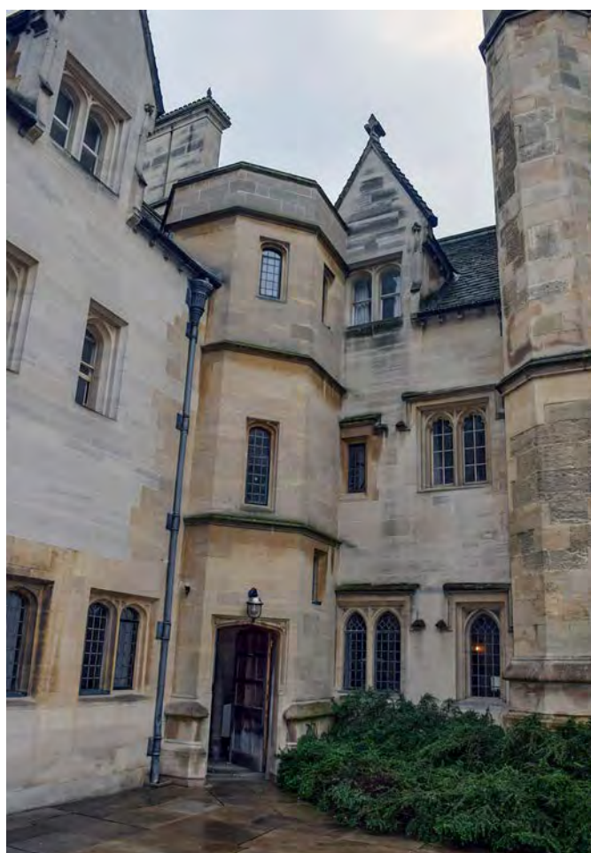
Plate 55: Inserted stair tower in Chaplains III
