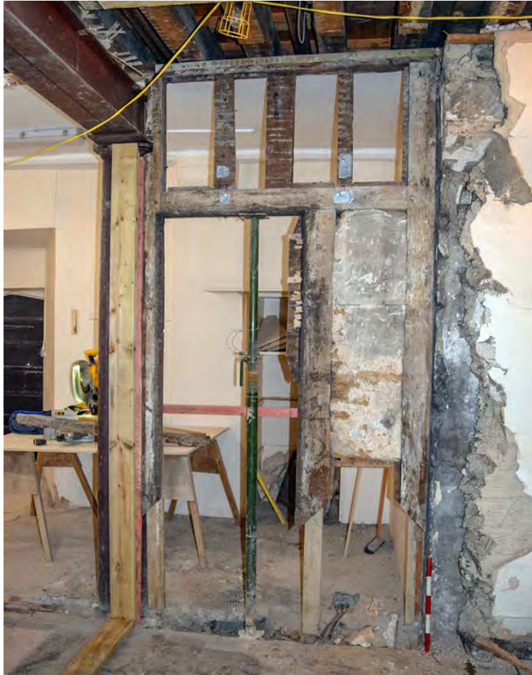
Plate 21: 16th-century frame after works to raise it
