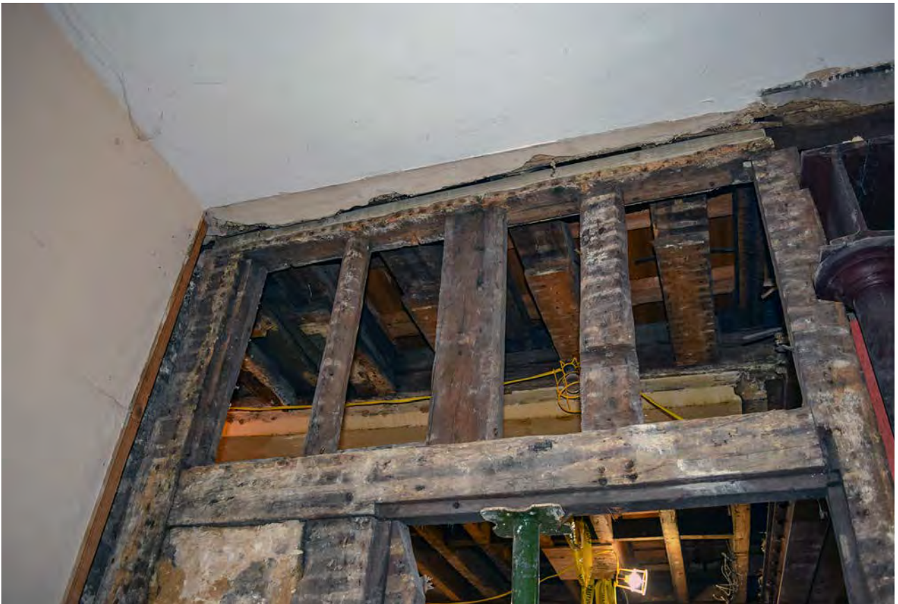
Plate 22: Upper part of 16th-century frame after removal of plaster
