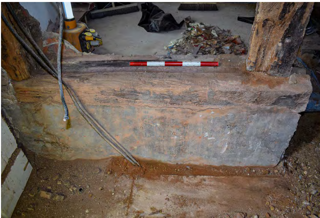
Plate 9: Sole plate of frame after removal of brick infill
