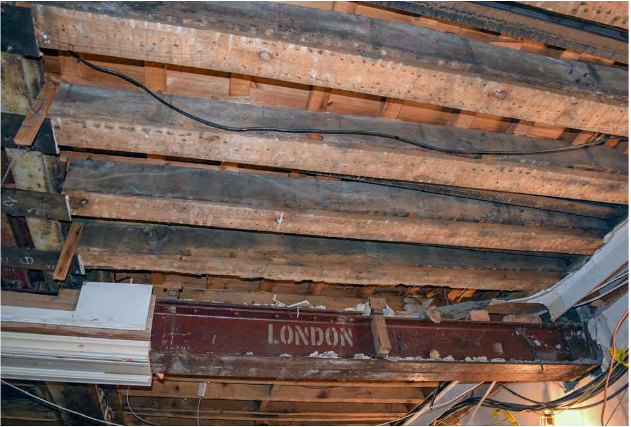
Plate 27: Exposed floor in Old Bursary looking east
