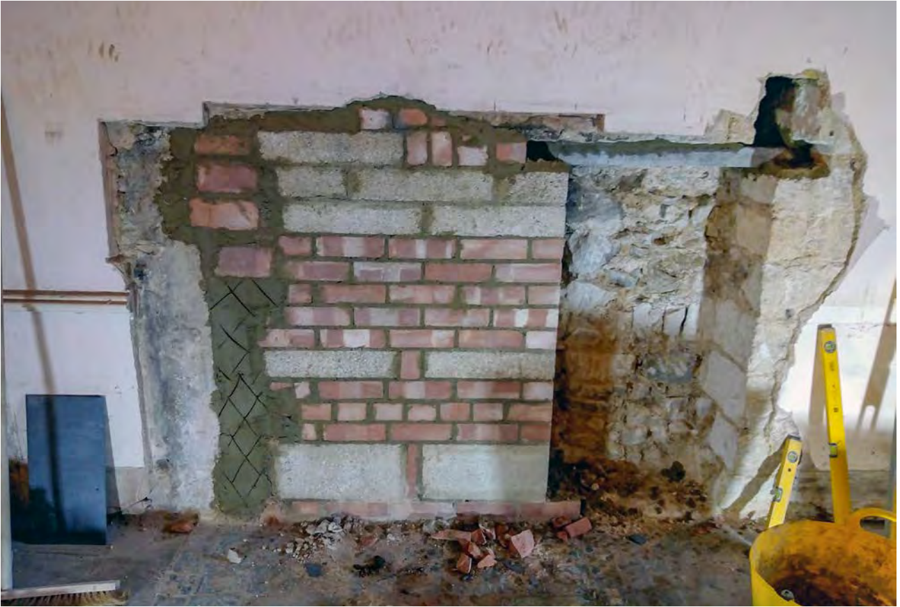
Plate 33: Fireplace on east side of Old Bursary after removal of surround
