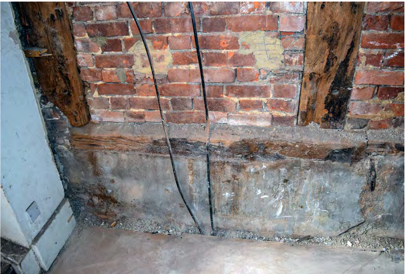
Plate 8: South end of sole plate of frame in west side of Old Bursary
