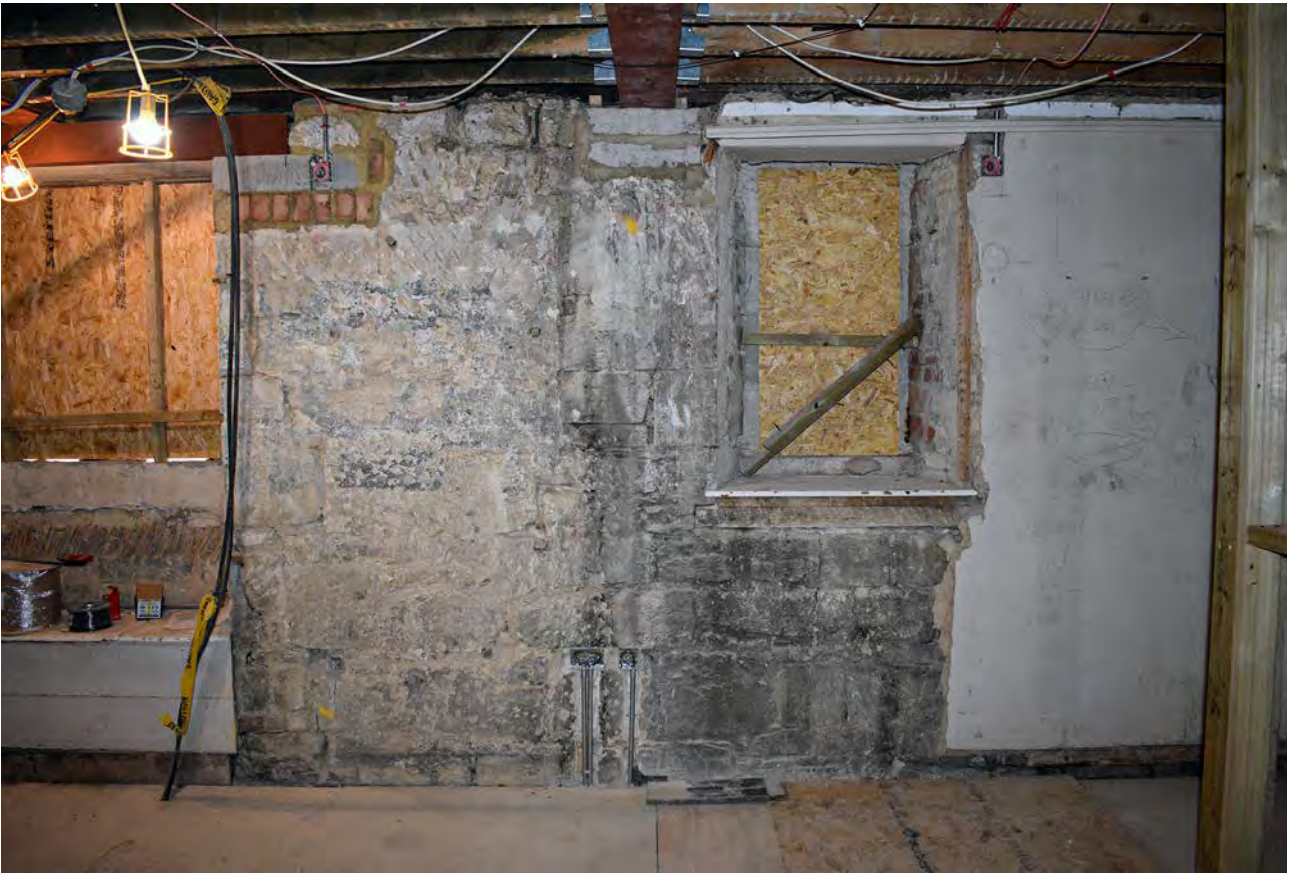
Plate 104: Part of west wall at first floor of Chaplains III
