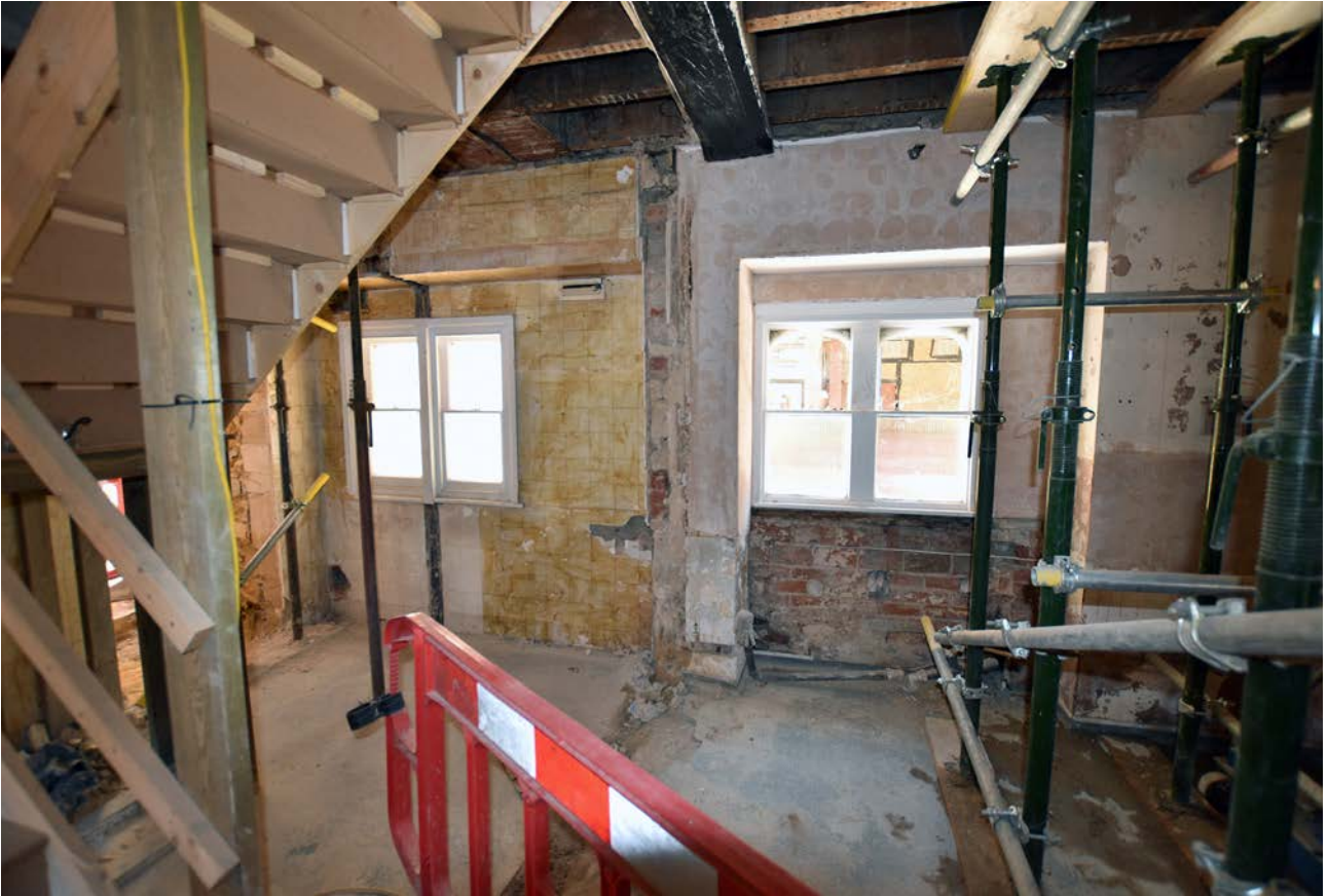
Plate 64: Ground floor of Chaplains III during strip out
