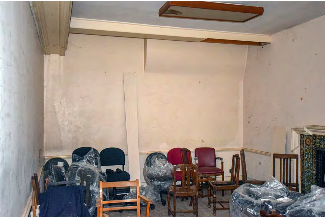
Plate 2: Store in Old Bursary area prior to works looking north
