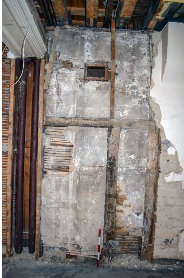
Plate 17: 16th century frame exposed on north side of Old Bursary
