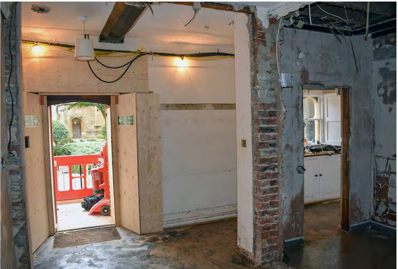
Plate 65: Ground floor of Chaplains III during strip out
