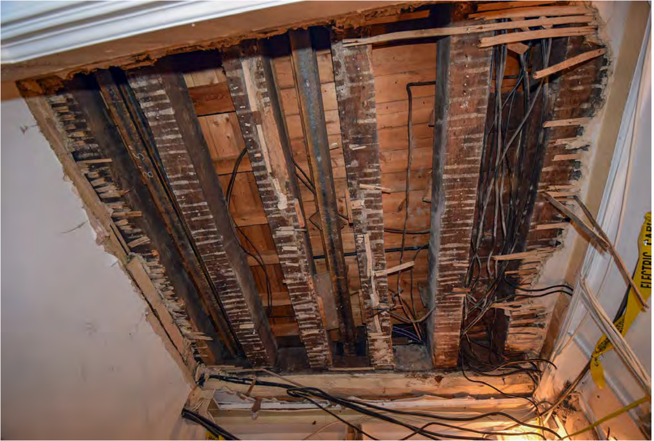
Plate 25: Primary floor joists in Linen Store
