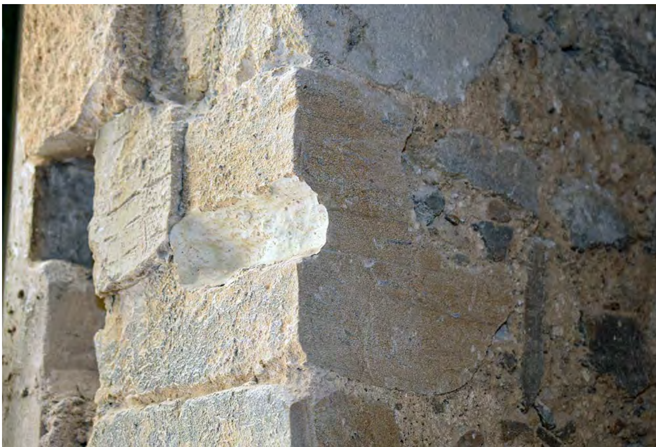
Plate 71: Reused moulded stone in jamb of new doorway
