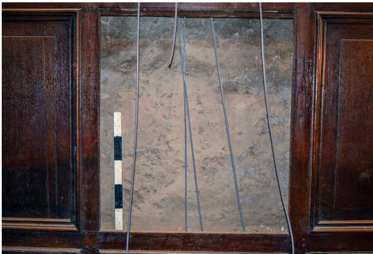
Plate 44: Exposed stone behind removed panel in Winter Common Room
