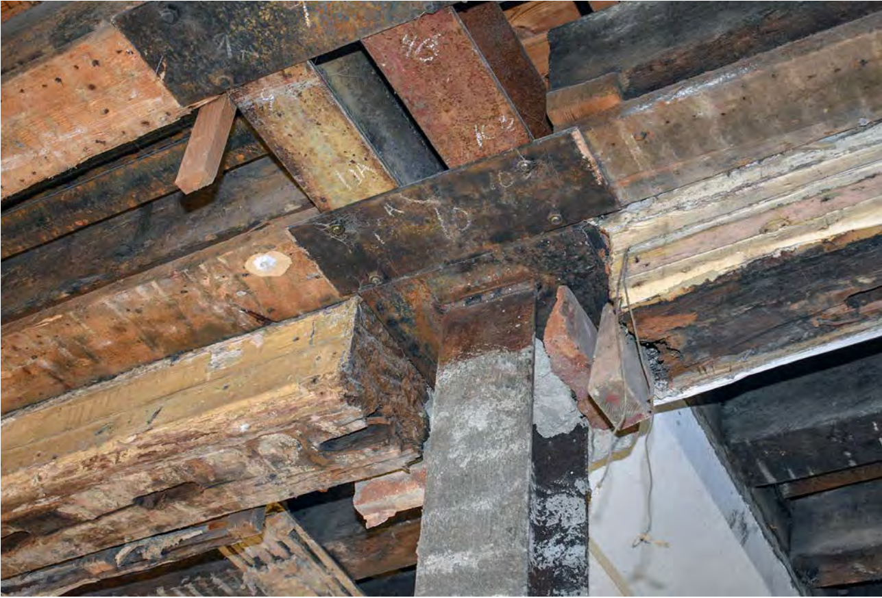
Plate 31: Head of steel column at centre of primary partition
