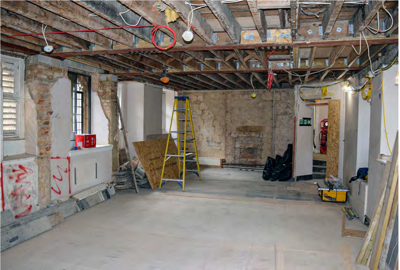
Plate 99: First floor of Chaplains looking south
