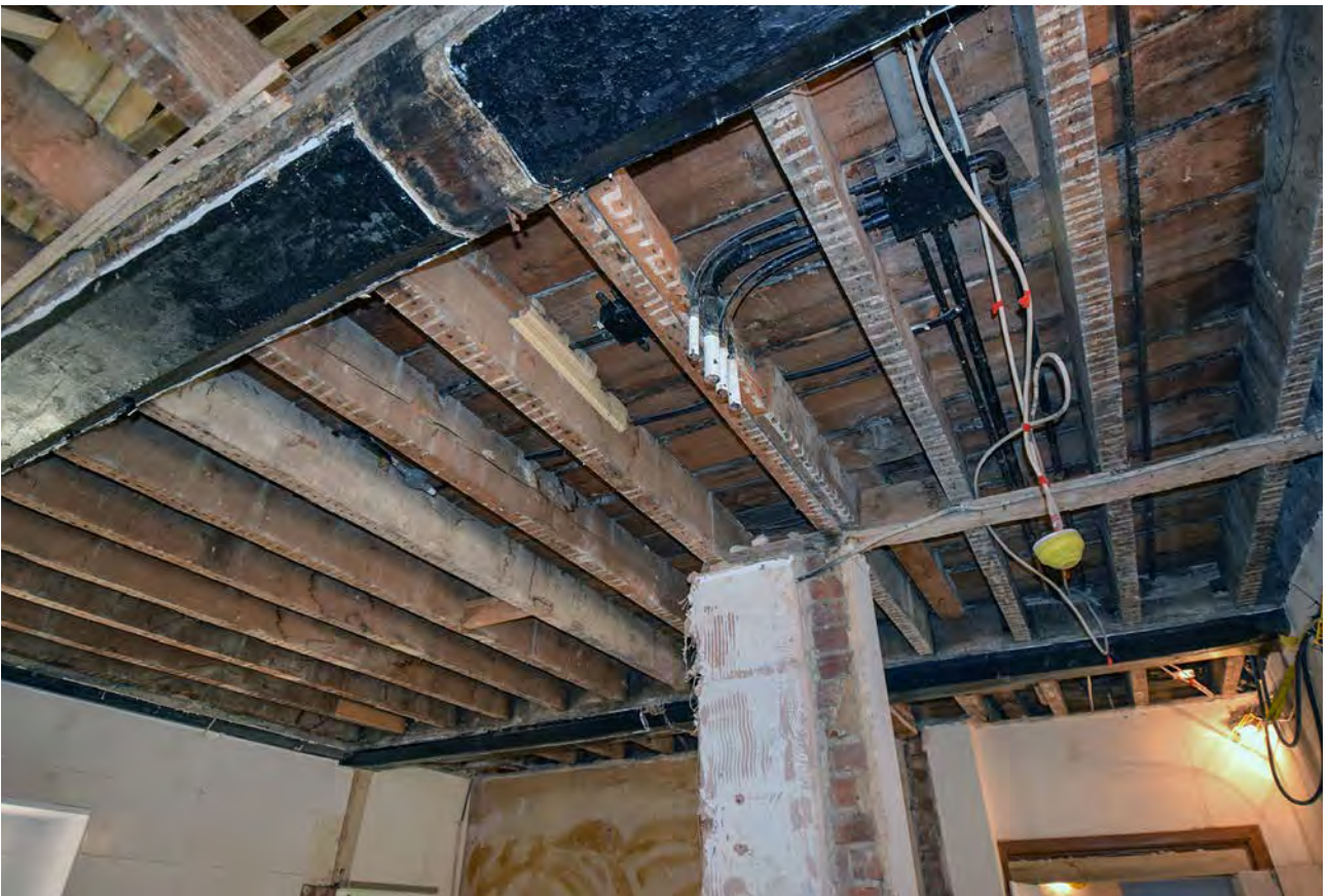
Plate 61: Exposed joists in ground floor of Chaplains III
