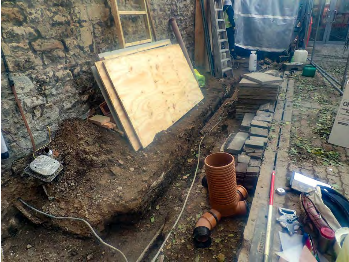
Plate 3: South end of drainage trench
