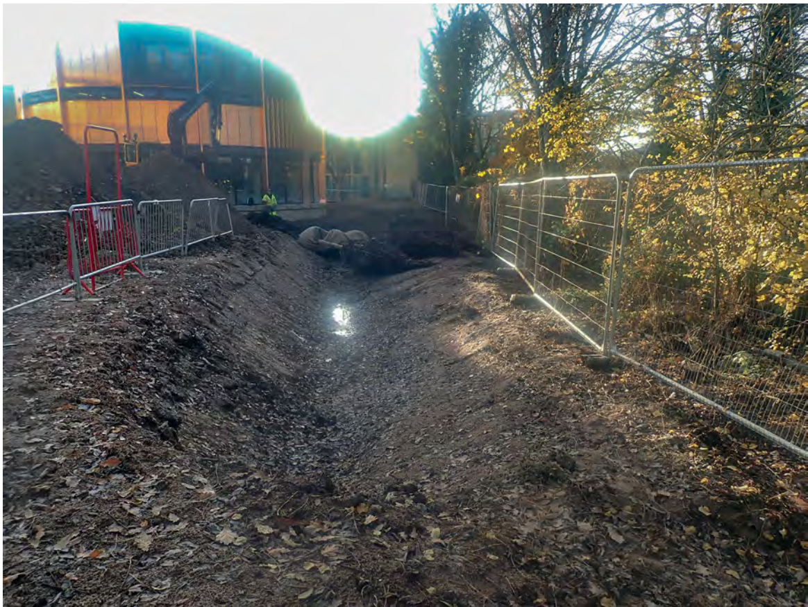
Plate 2: South-West view along ditch
