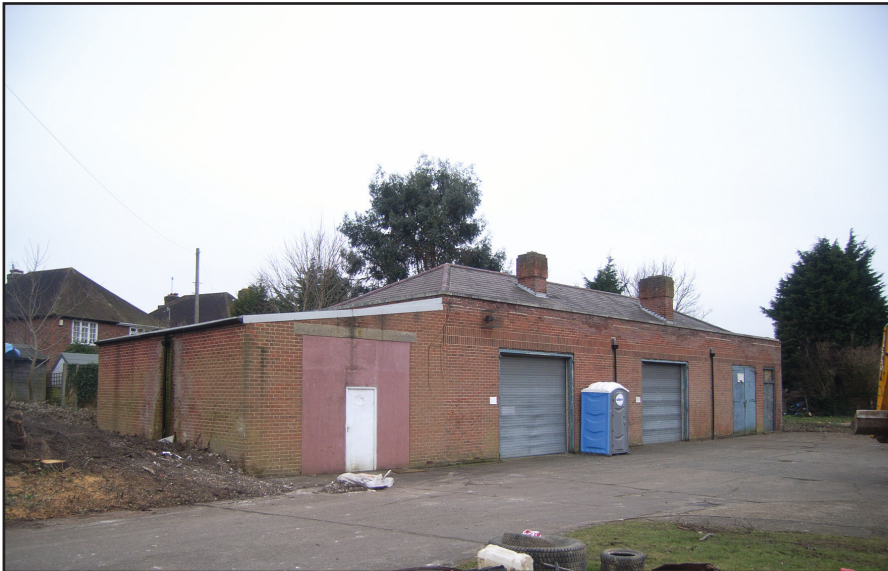
Plate 19: Front of fire station store building
