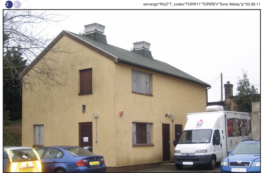
Plate 18: Smoke House from north-west
