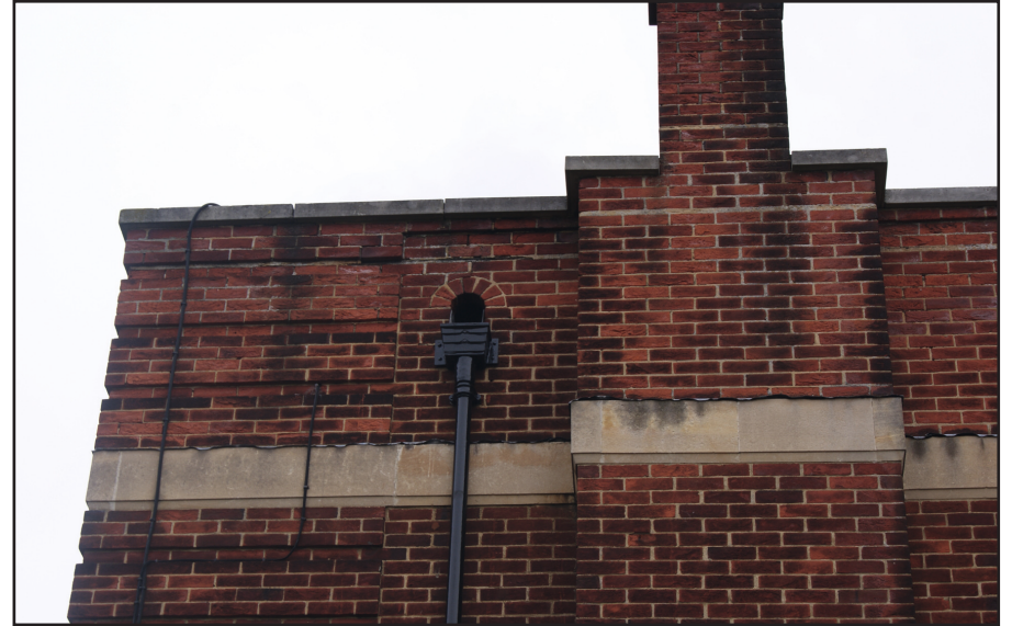
Plate 10: Gutter detail at north end of west elevation
