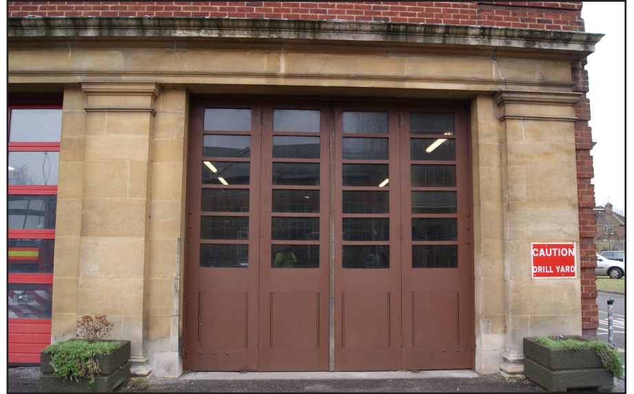
Plate 6: Original doors for fire engines in north elevation
