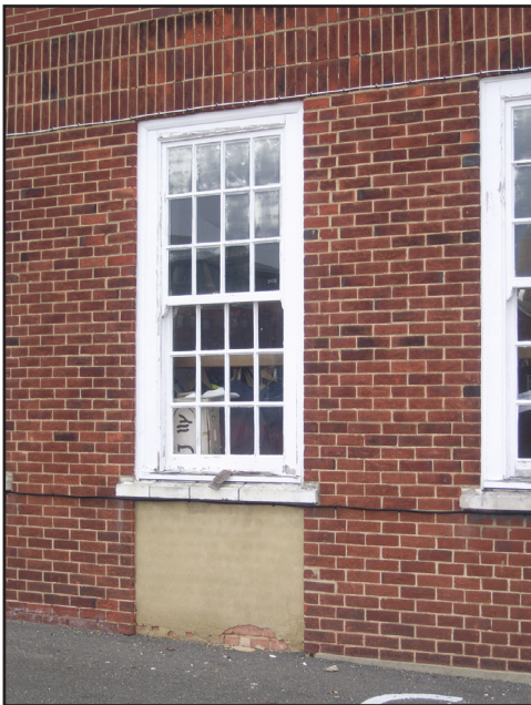
Plate 11: Door converted to window in west elevation
