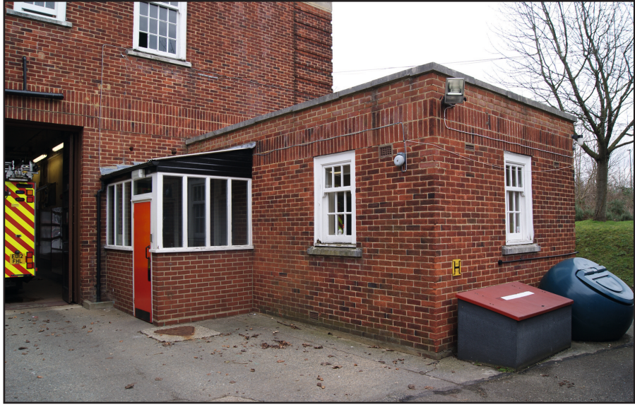
Plate 13: Projection at east end of south elevation
