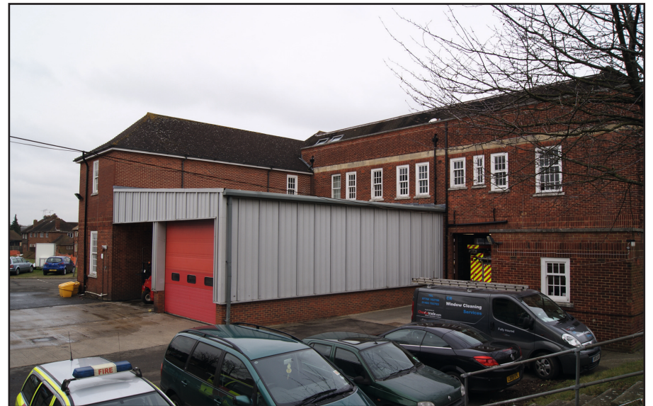
Plate 12: General view of rear of main building (from SE)
