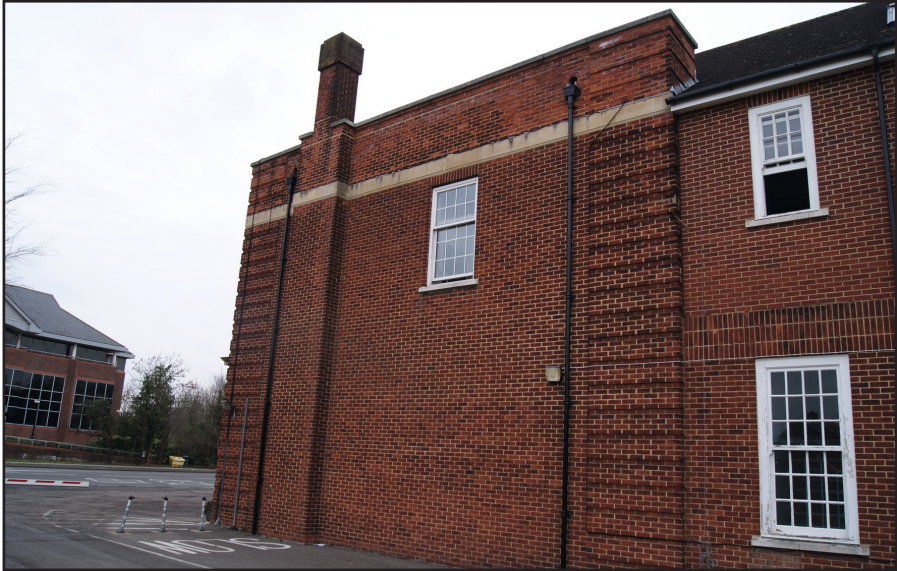
Plate 9: North end of west elevation
