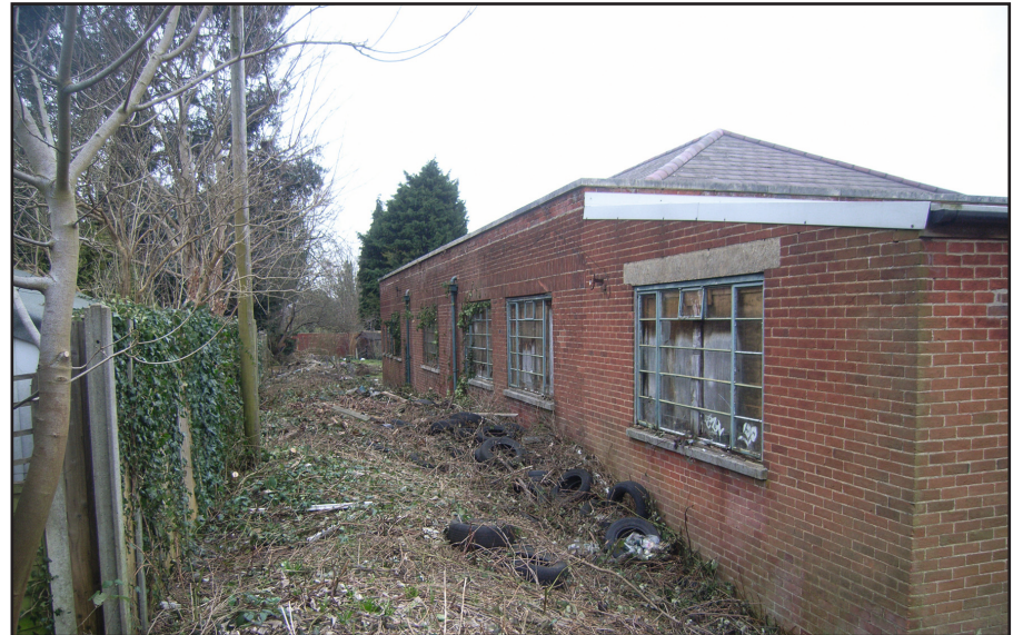
Plate 20: Rear of fire station store building
