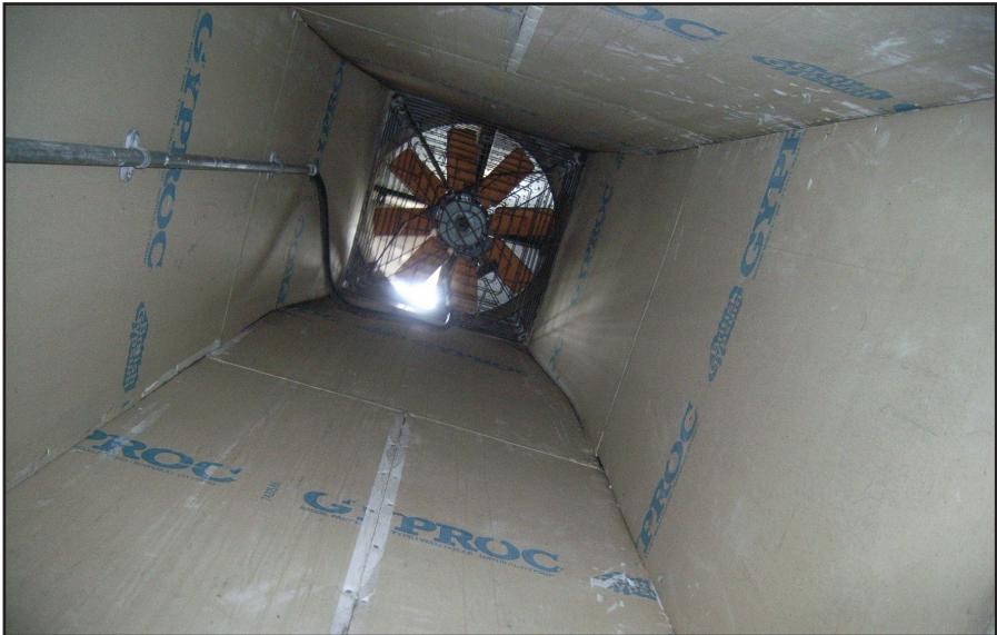
Plate 31: Smoke vent in smoke house
