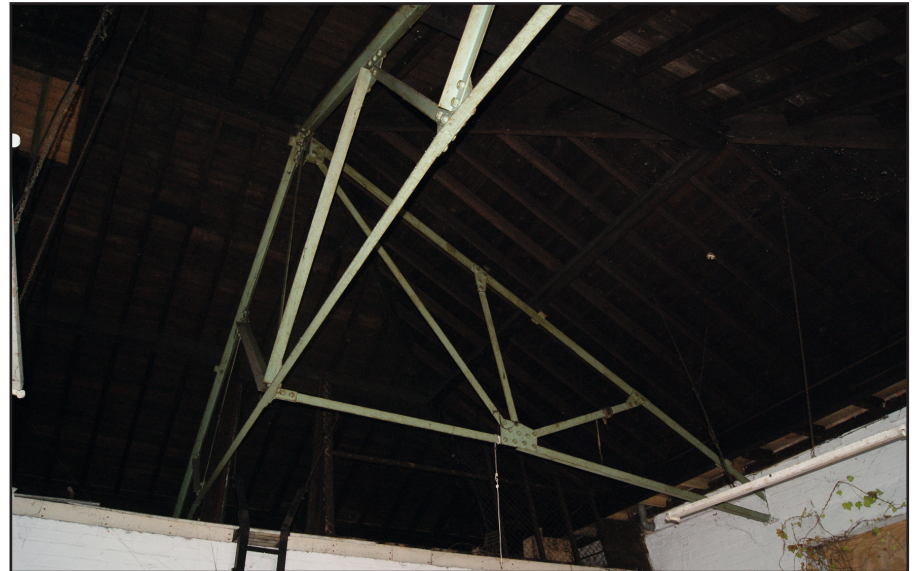
Plate 32: Trusses in store buildings
