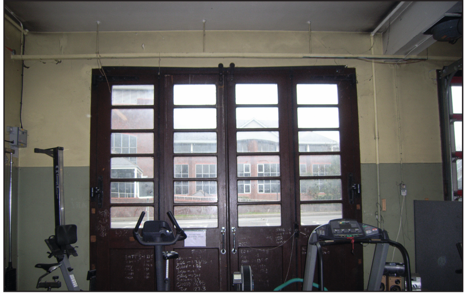
Plate 22: Primary horizontally sliding doors for fire engines
