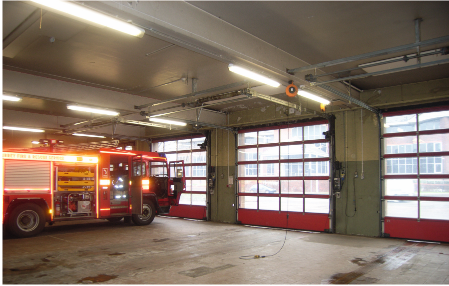
Plate 21: Secondary vertically sliding doors for fire engines
