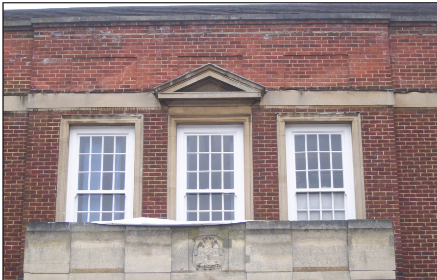
Plate 3: Balcony in north elevation of main building
