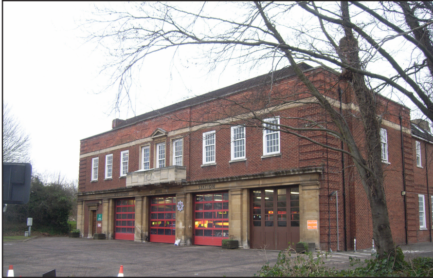
Plate 1: North elevation of main fire station
