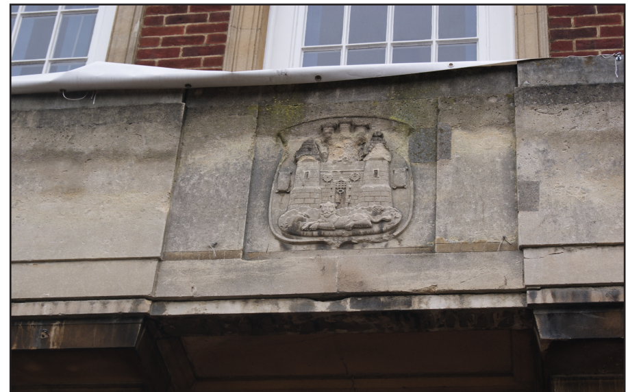
Plate 4: Stone crest on balcony
