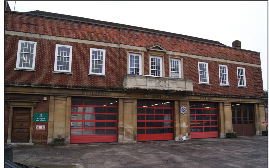
Plate 2: North elevation of main fire station
