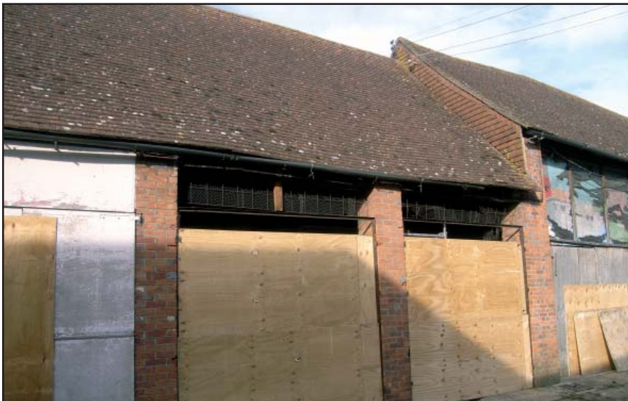
Building 7 and 8, Plate 3
