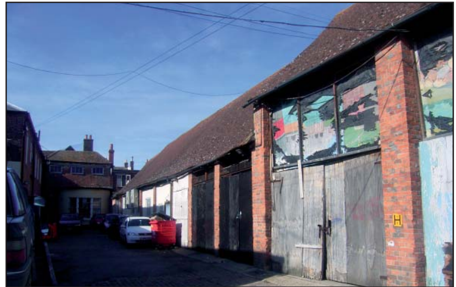
Building 7 and 8, Plate 4
