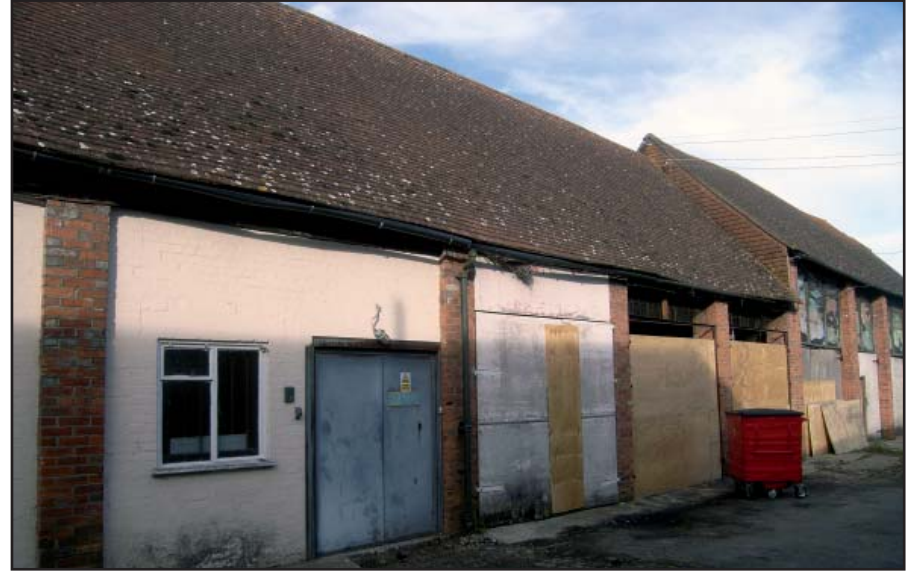
Building 7 and 8, Plate 2
