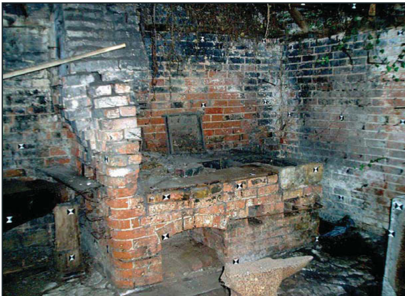
Plate 7: Blacksmith's Workshop: internal north elevation (without artefacts)
