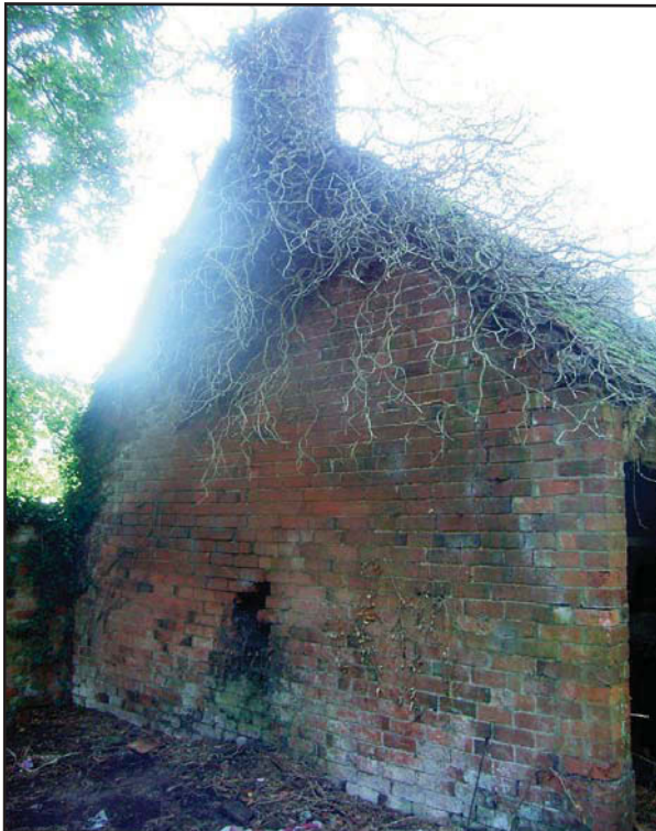
Plate 3: Blacksmith's Workshop: north elevation showing hole in brickwork and west edge rebuild (without artefacts)
