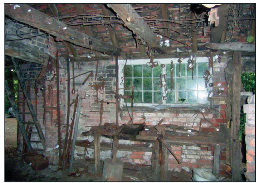
Plate 8: Blacksmith's Workshop: internal west elevation (showing some artefacts)
