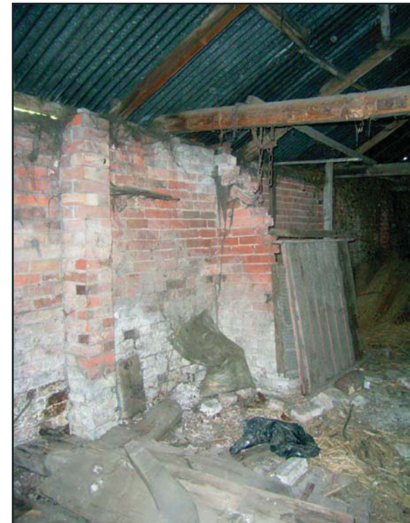
Plate 20: The Store: east elevation, former partition wall
