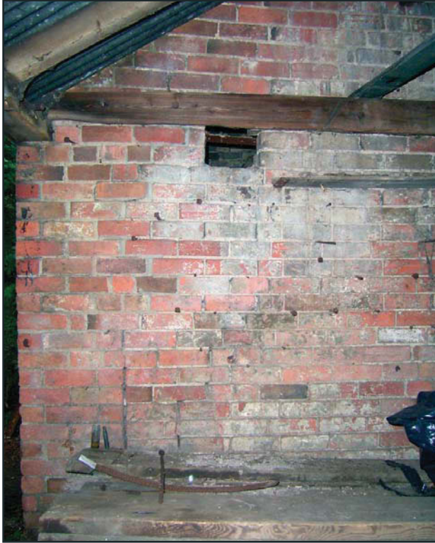
Plate 21: The Store: north elevation, showing phasing to west
