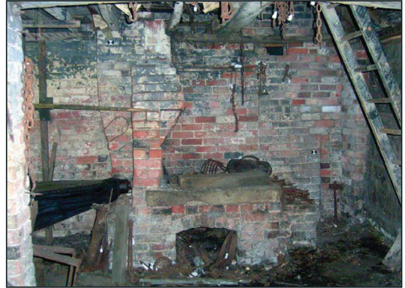
Plate 10: Blacksmith's Workshop: internal south elevation, showing phasing
