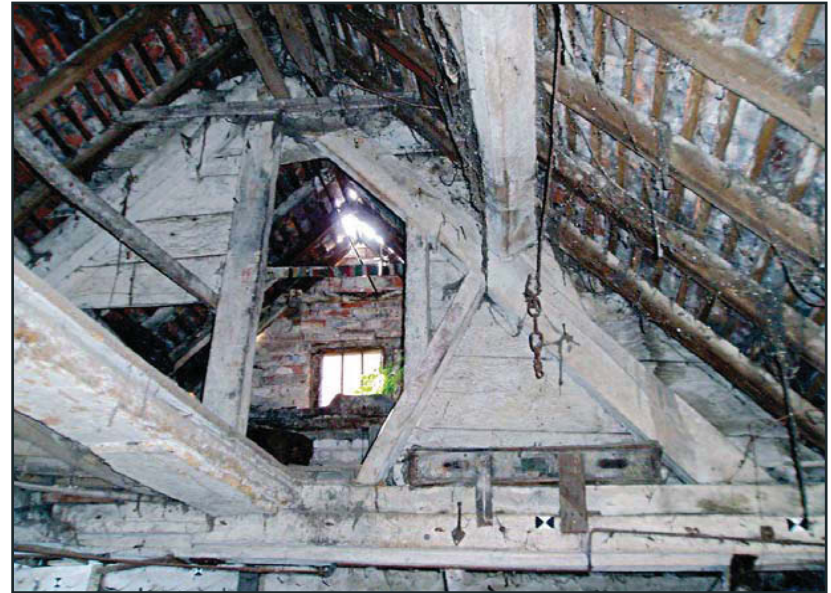
Plate 14: Wheelwright's Workshop: Paint store, south elevation
