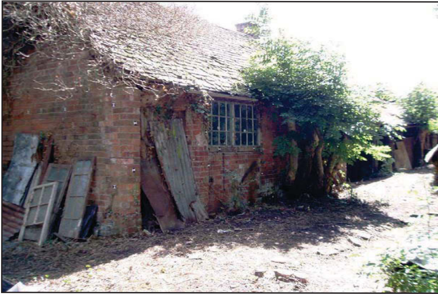
Plate 1: Blacksmith's Workshop: north and west elevations (with artefacts)
