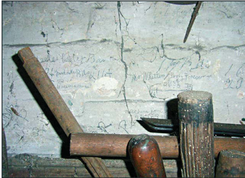
Plate 17: Wheelwright'sv Workshop: internal graffiti on north elevation
