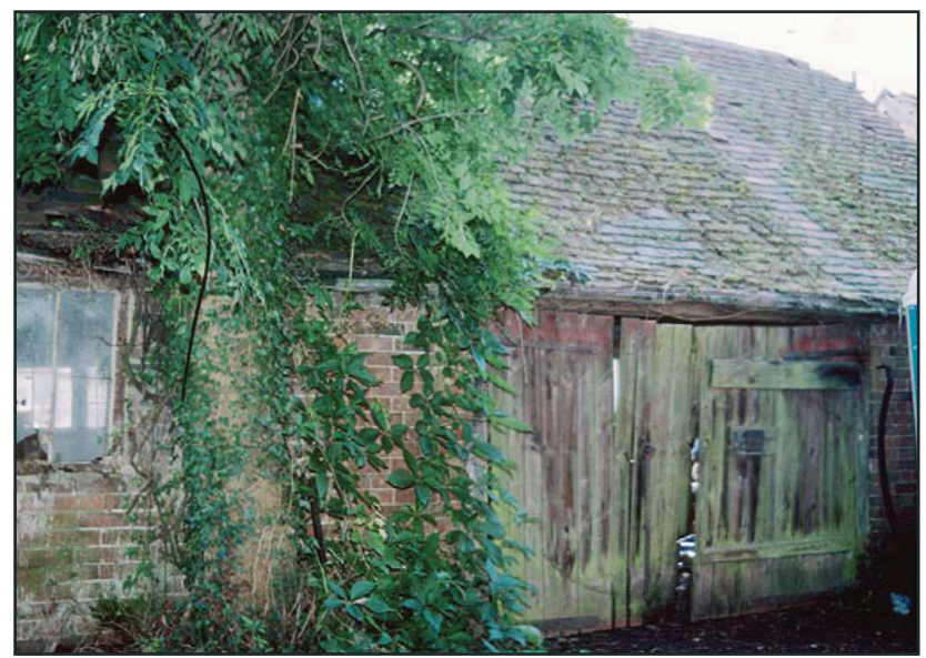
Plate 12: Wheelwright's Workshop: west elevation, entrance door
