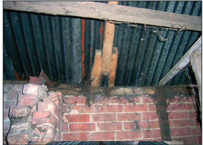
Plate 22: The Store: roof, common rafter
