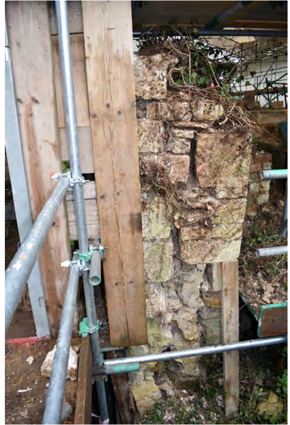
Plate 15: South face of pier (former window jamb) before dismantling
