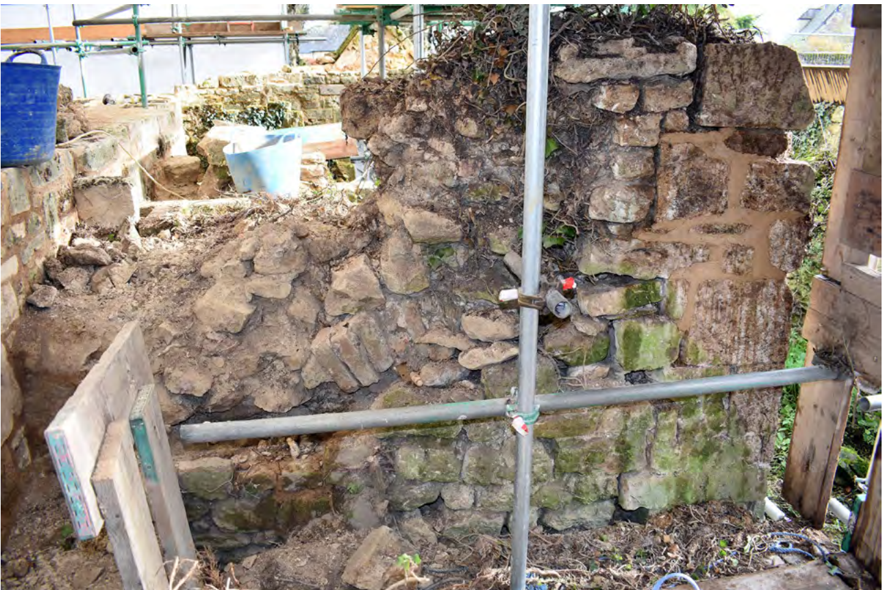
Plate 11: West side of section of wall before dismantling with straps removed
