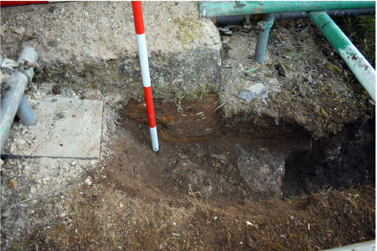
Plate 6: Foundations exposed at point where trench adjoins building
