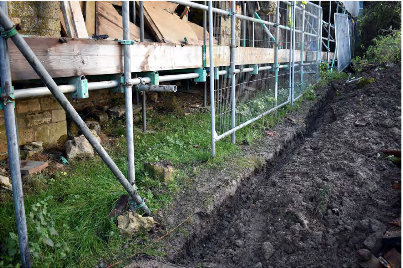
Plate 1: General view of trench to west side of building, looking south
