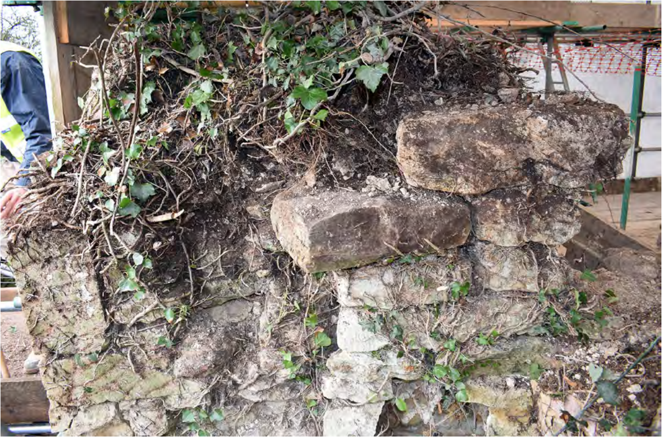
Plate 17: Stonework at top of east side of wall prior to dismantling
