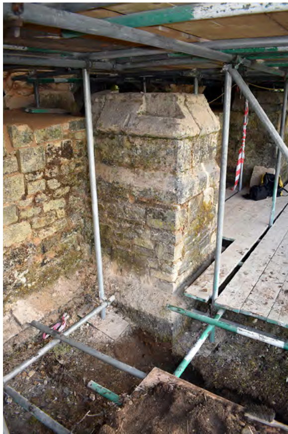
Plate 9: Third buttress from south; with adjoining trench
