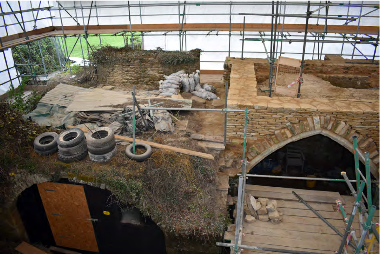
Plate 29: Northern end of range
