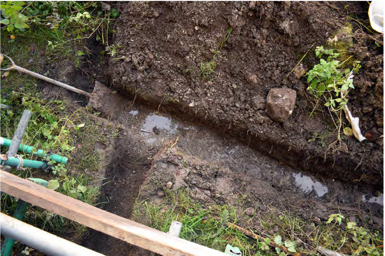
Plate 4: Junction at southern end of drainage trench
