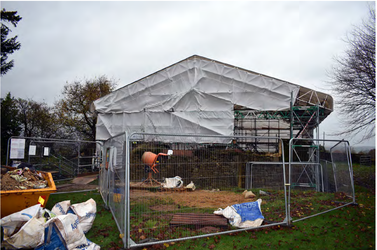
Plate 26: General view towards north during works
