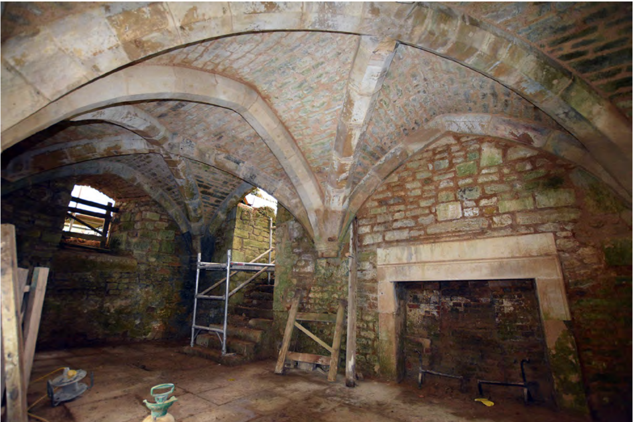
Plate 30: Southern end of undercroft
