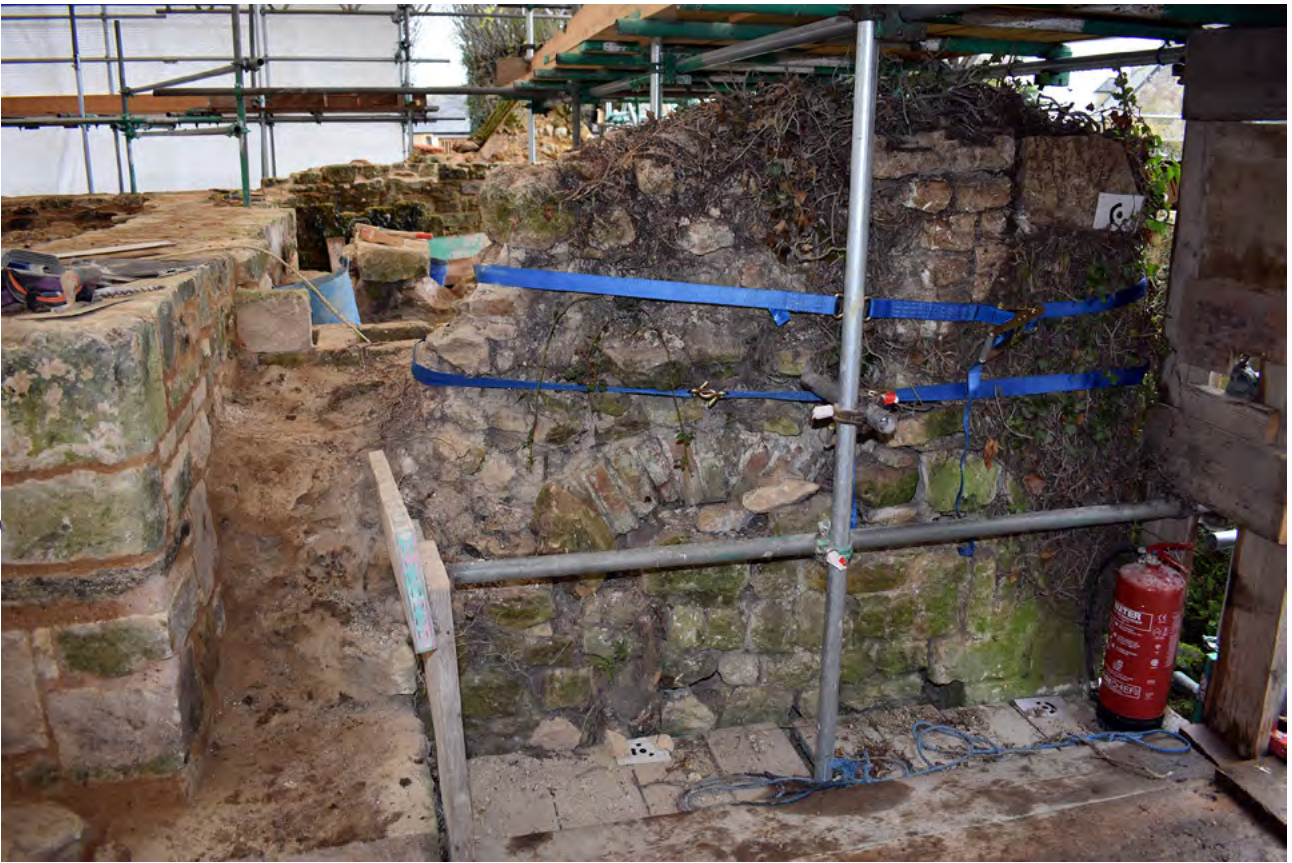
Plate 10: West side of section of wall before dismantling with straps in-situ
