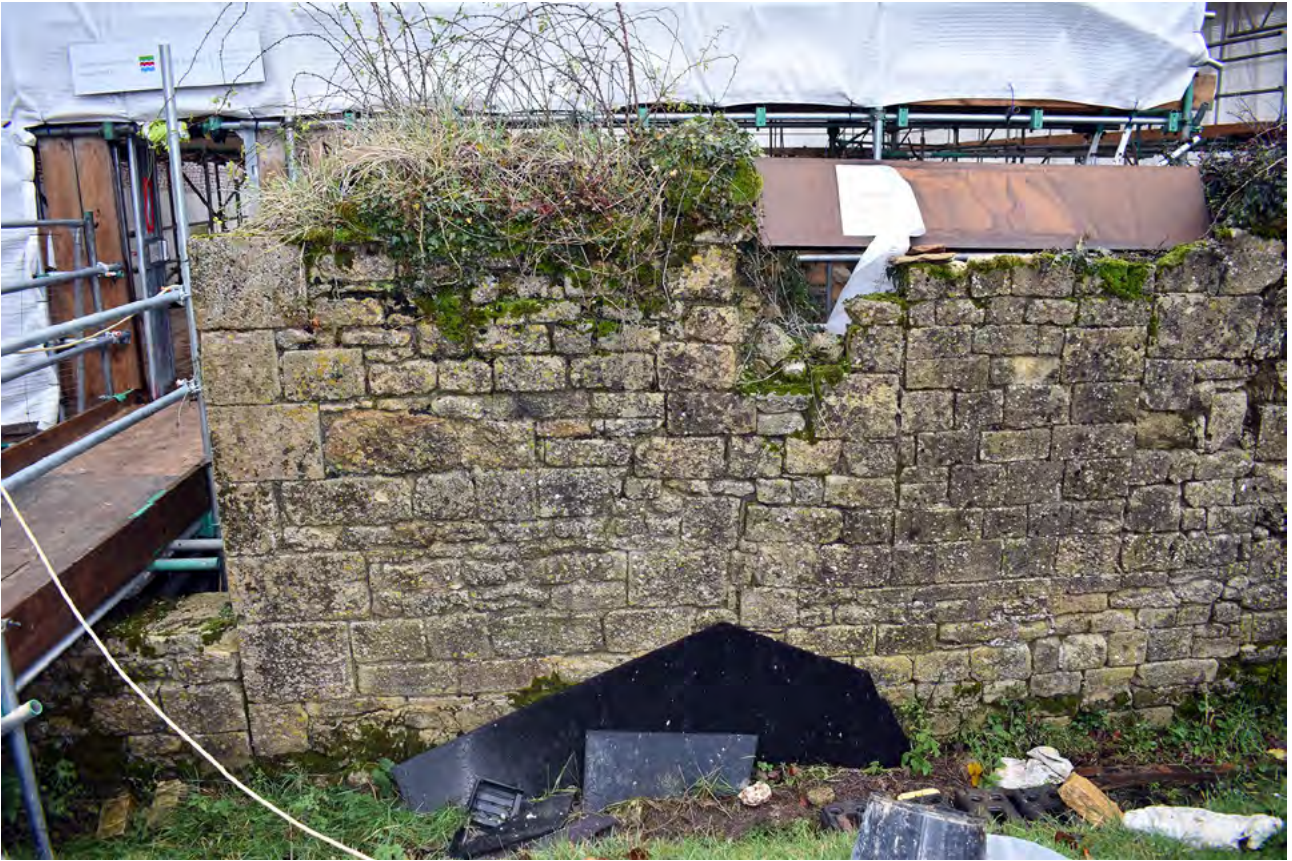
Plate 25: South wall of former Prior's Lodgings
