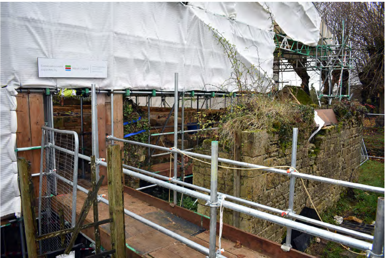
Plate 24: View looking NE towards former Prior's Lodgings
