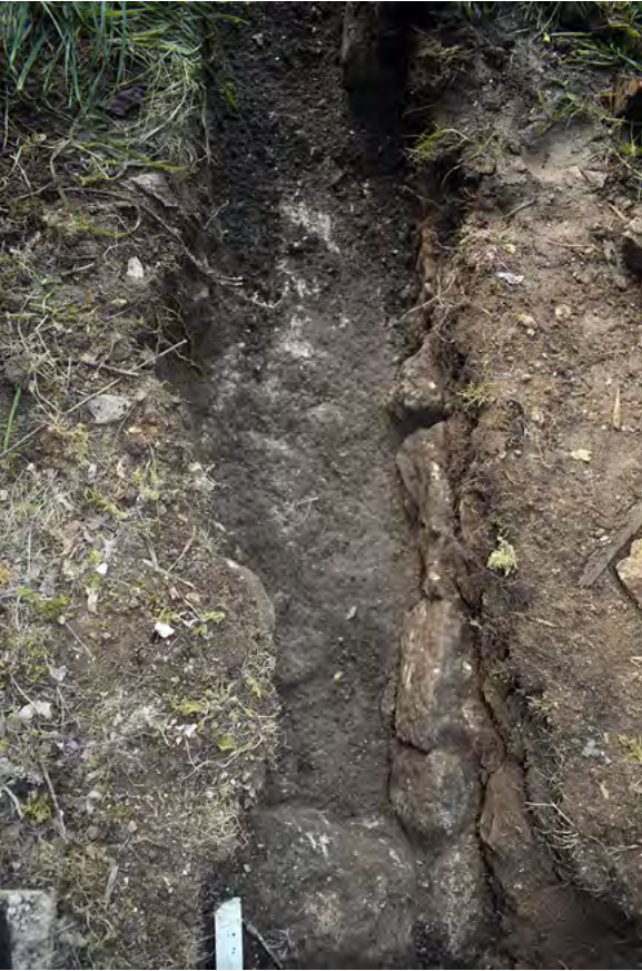
Plate 7: Eastern part of drainage trench looking west
