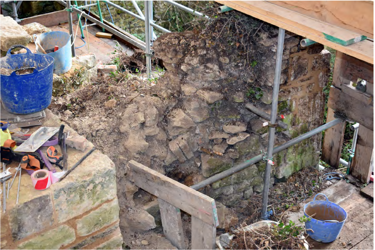
Plate 12: General view of section of wall before dismantling
