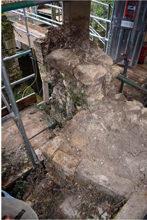
Plate 21: View looking SW towards wall to be dismantled
