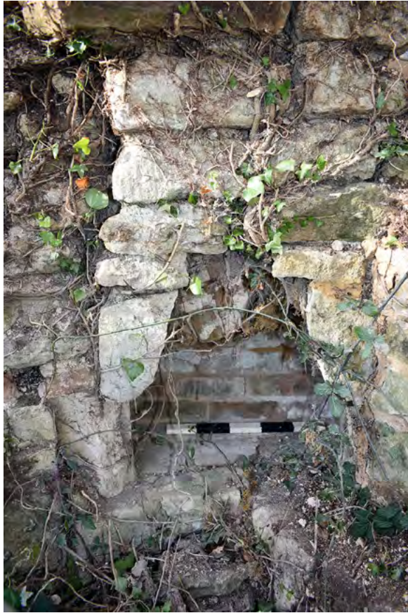
Plate 19: Remains of bread oven in east side of wall
