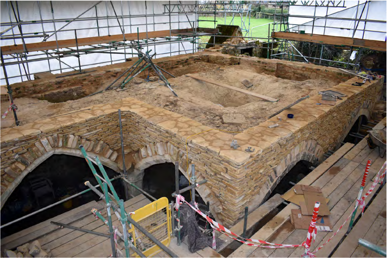
Plate 27: General view towards SE during works
