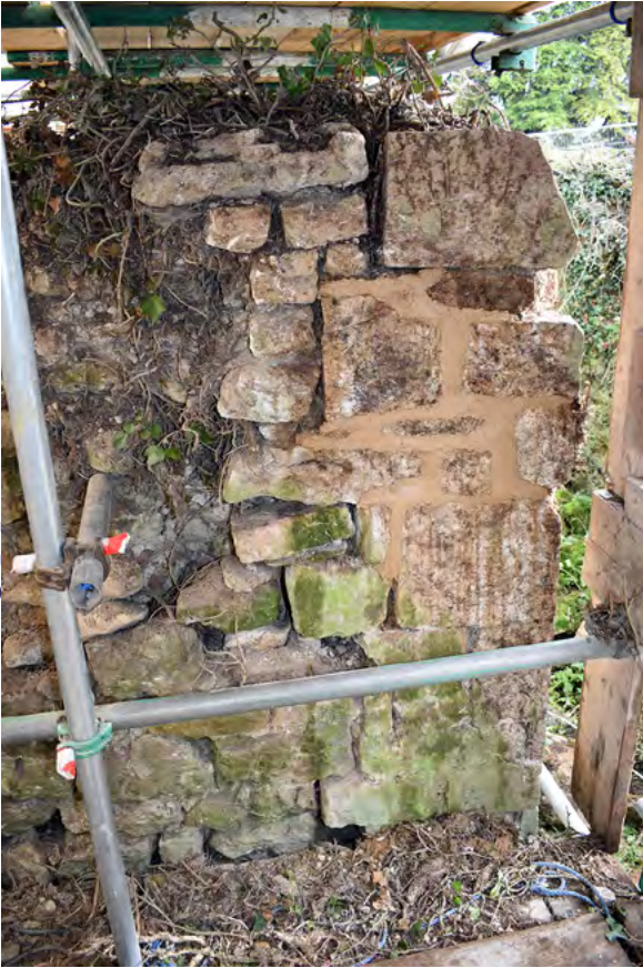
Plate 14: Southern end of west side of wall during dismantling
