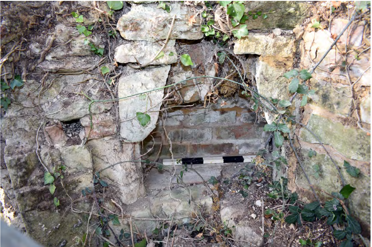
Plate 18: Remains of bread oven in east side of wall
