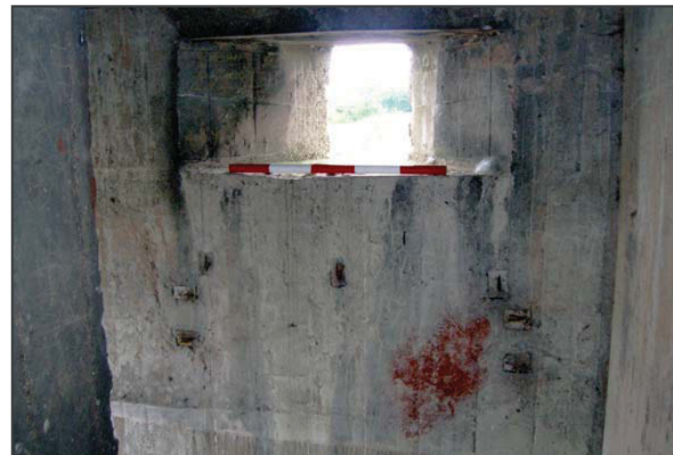
Plate 10: Interior view of south embrasure showing timber fixing blocks below, 0.5m scale
