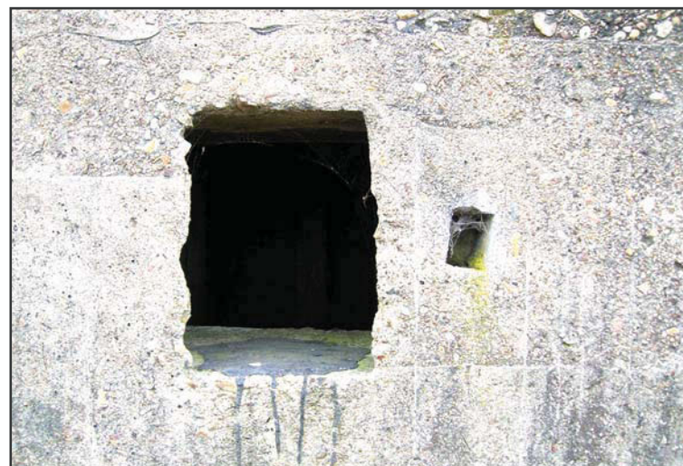
Plate 6: Close up of south facing embrasure
