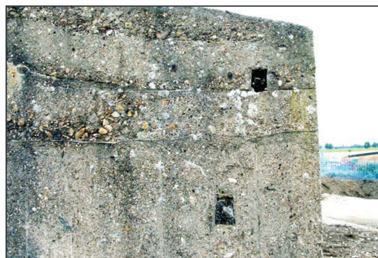
Plate 8: Part of south elevation showing construction phases and timber blocks
