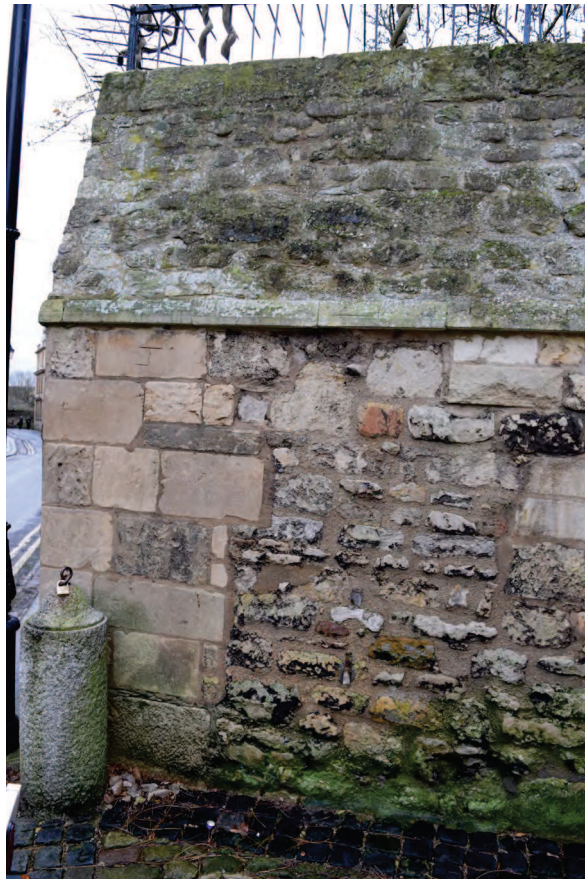
Plate 6: North half of wall facing lay-by off Queen's Lane
