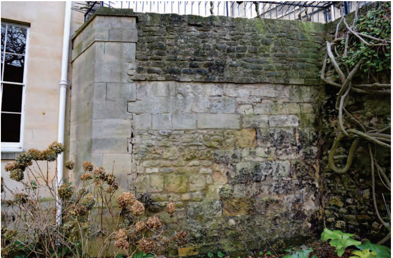
Plate 1: General view of west face of wall
