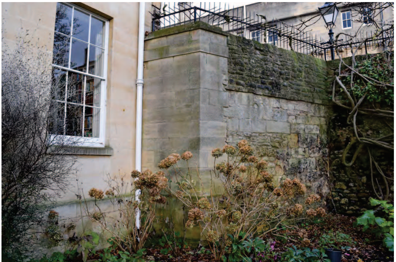
Plate 2: General view of east face of wall
