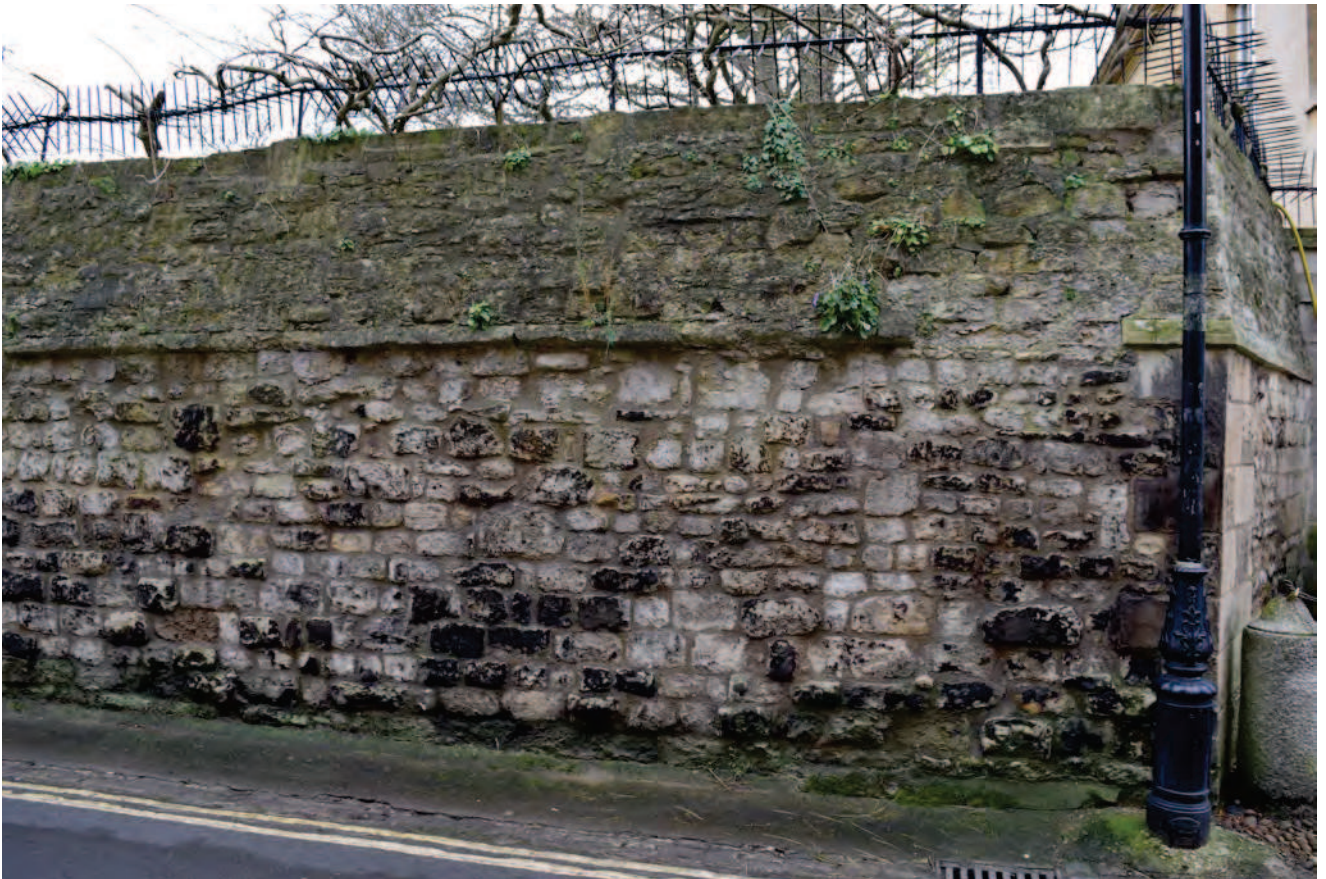
Plate 4: View of main wall along Queen's Lane (outside current works)
